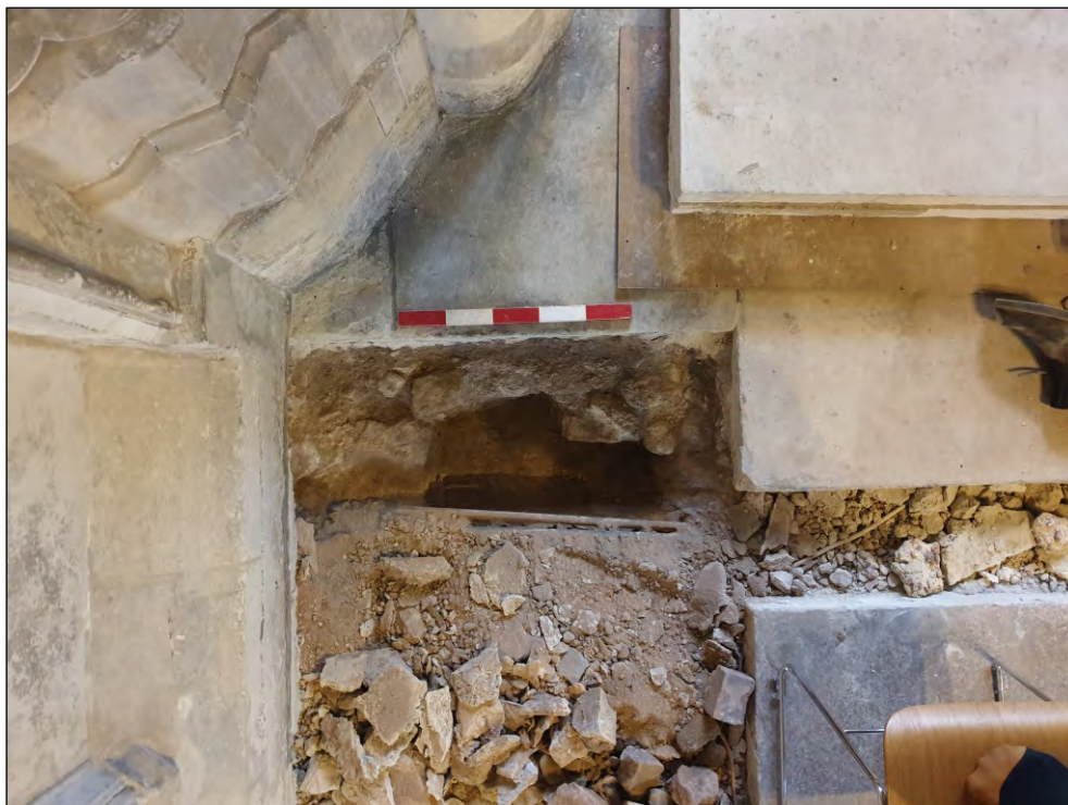
Pl. 6 Close-up of Trench 1 showing pier foundation (103). 0.5m scale. Looking south.
