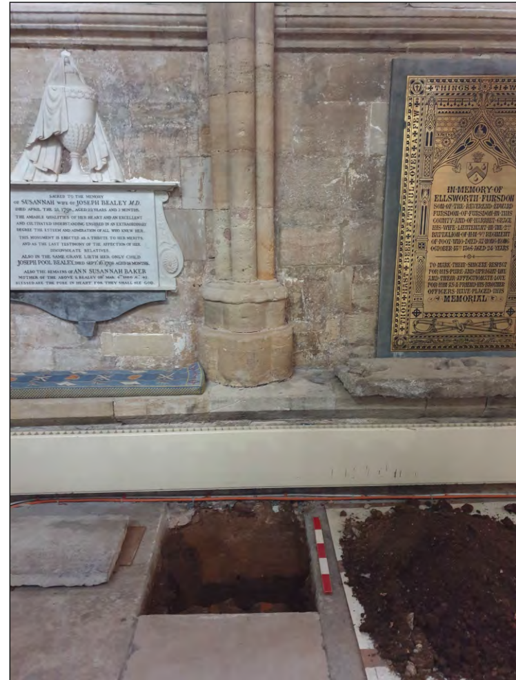
Pl. 36 General view of Trench 18 showing projecting foundation (1807) of possible Norman north wall pier. 0.5m scale. Looking north.
