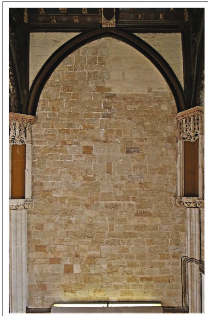
Fig. 5e. Chapter House, south wall: the upper part of Bay 4, showing two periods of masonry ( photo: Hugh Harrison, 20 Oct 2020 ).
