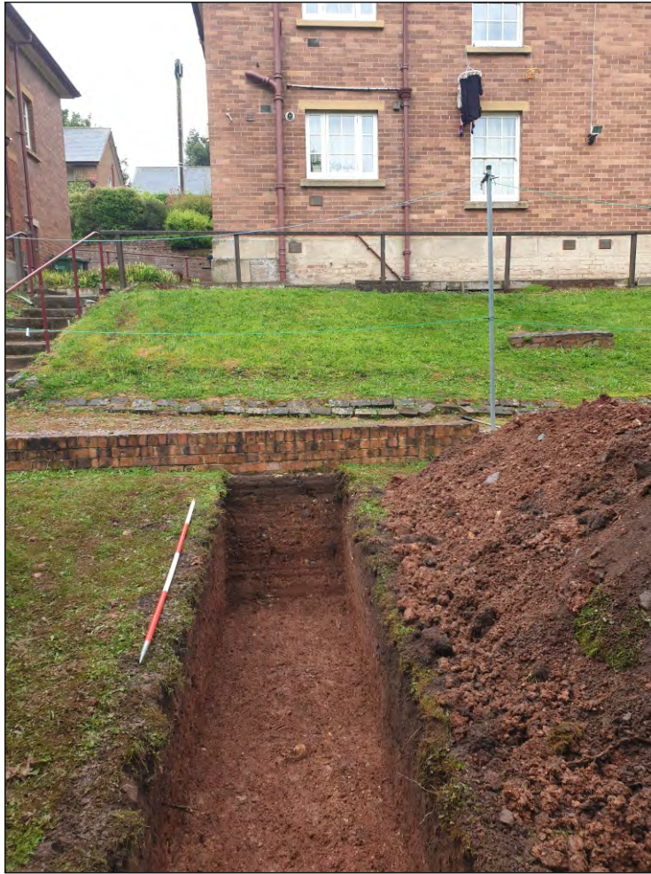
Pl. 11 General view of Trench 3. 2m scale. Looking southeast.
