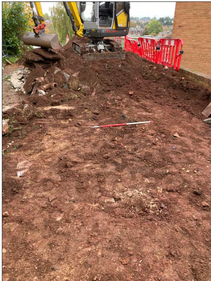
Pl. 4 General view of new bin store excavations. 1m scale. Looking northeast.
