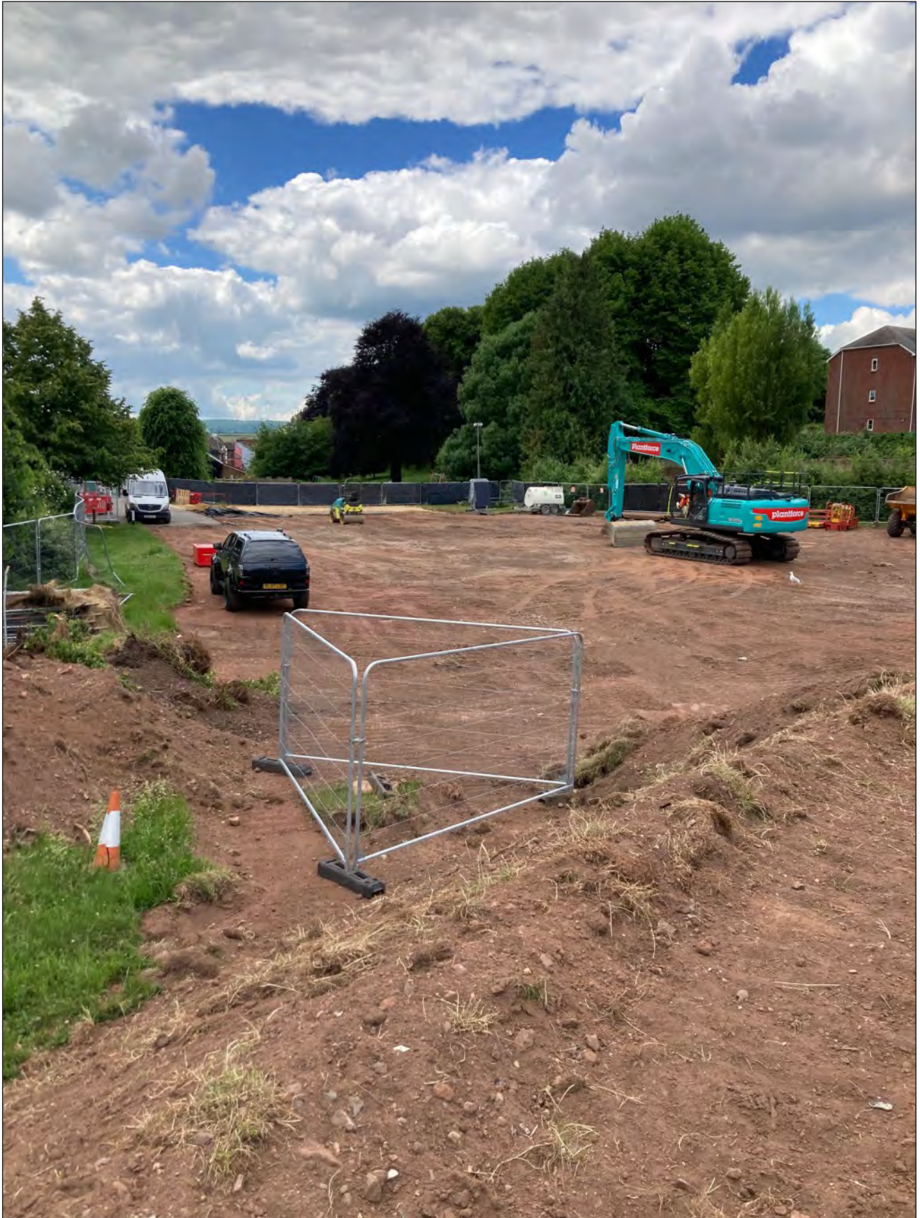
Pl. 1 General view of site. Looking southwest.
