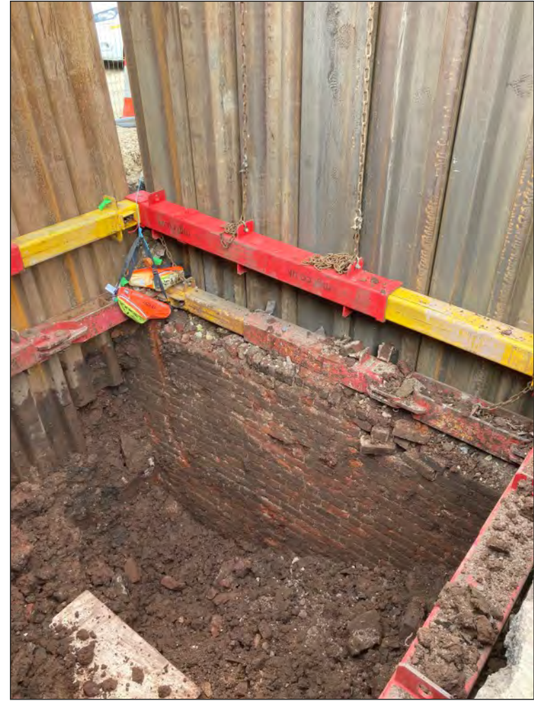
Pl. 3 General view of brick revetment wall (107). Looking southwest.
