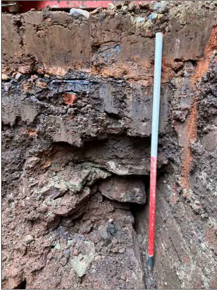
Pl. 2 Close-up of stone rubble wall foundation (108) abutting brick wall revetment (107). 1m scale. Looking southwest.
