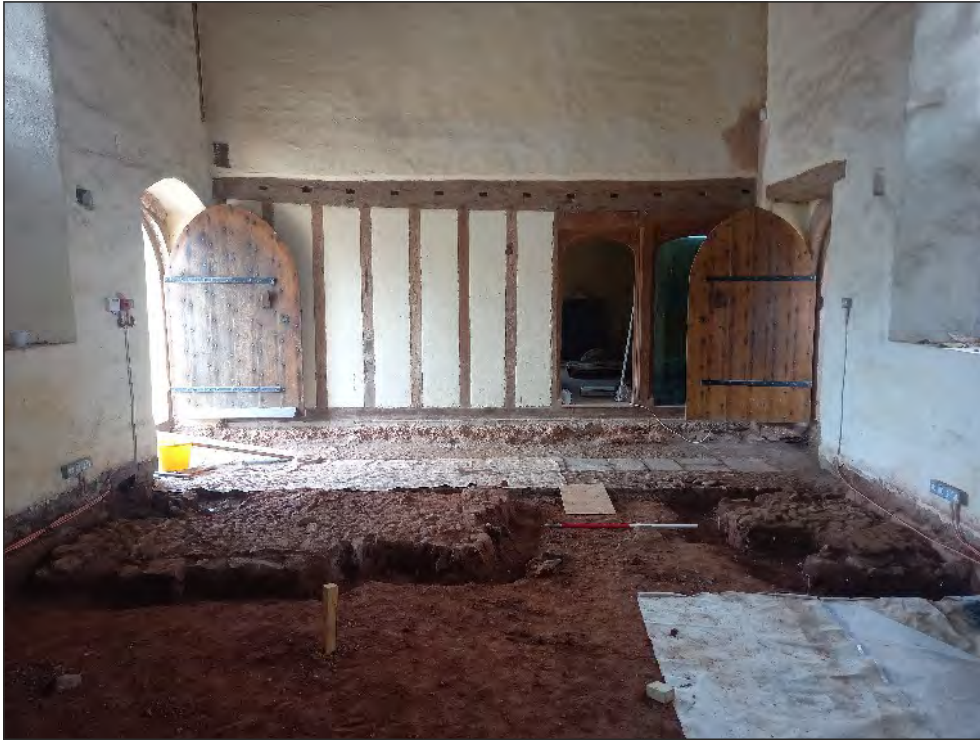
Pl. 1 General view of the cross passage showing newly exposed cobbled surface (107 - left) and the surface (2133 - right) exposed by the Department of the Environment in 1977. 1m scale. Looking southeast.
