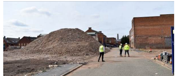
View west along Northwood St. following demolition (21.09.2021).
