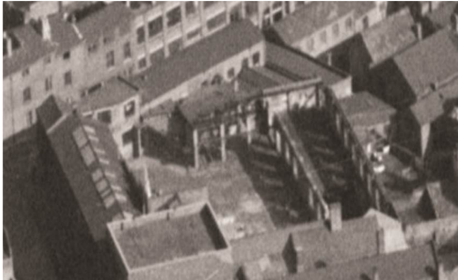
1948 aerial photograph of Buildings 10/11 looking south-east, (prior to remodelling/re-roofing of Bldg. 11b and introduction of Bldg. 11c ).
