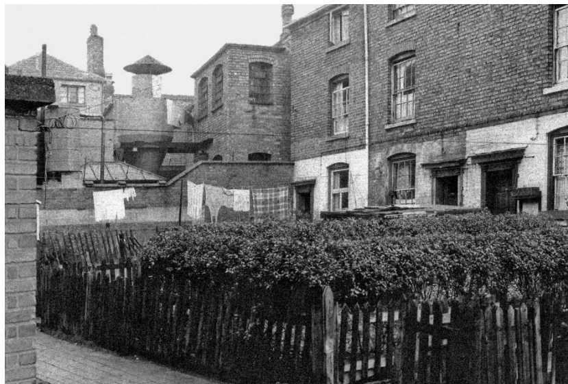
'Blind-back' housing, Court No. 2, Nos.10-12, St. Helen's Passage prior to demolition in 1955 (from Chin, nd.)
