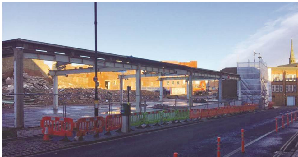
Building 14 during demolition (image: https://thehockleyflyer.info/demolition-along-graham-street ).
