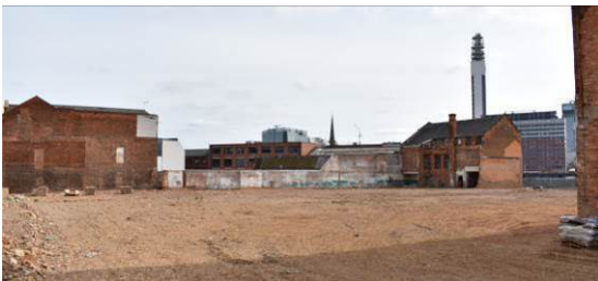
View of site east of Bldg. 7/8 following demolition (21.09.2021).
