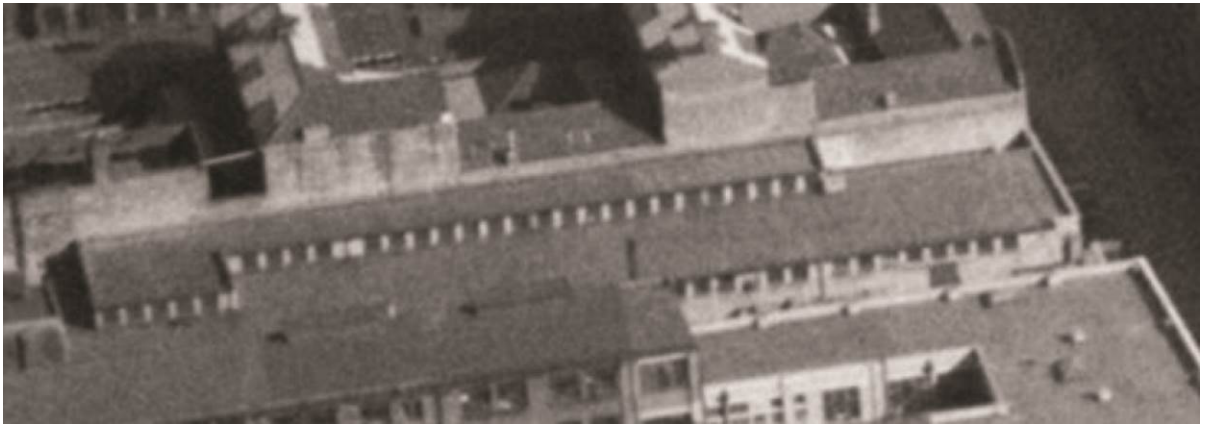
Detail of 1948 aerial photograph showing west elevation of Bldg. 6a, looking east, surviving to GF only with small, clerestory windows (as marked on 1943 plans BBP 76657; see above).
