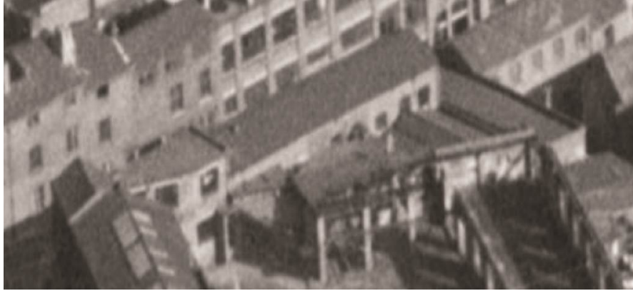
1948 aerial photograph of Building 10 looking south-east (Bldg. 11 to foreground).
