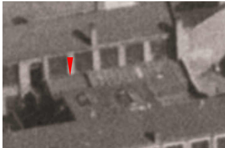
Detail from 1948 AP, looking south-east, showing form of Bldg. 13h .
