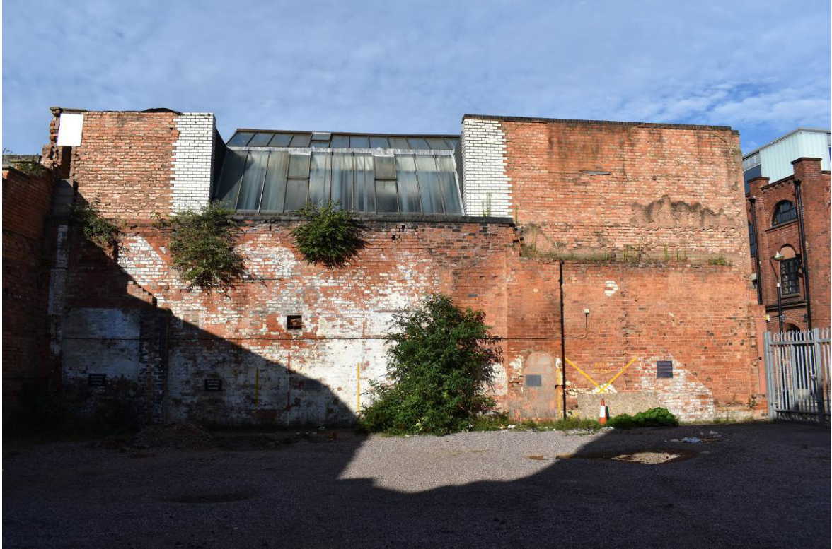
Plate 24: Building 5: east elevation to vacant plot (formerly 41-5 Regent Place); note 'ghost' of saw-tooth roof to left.
