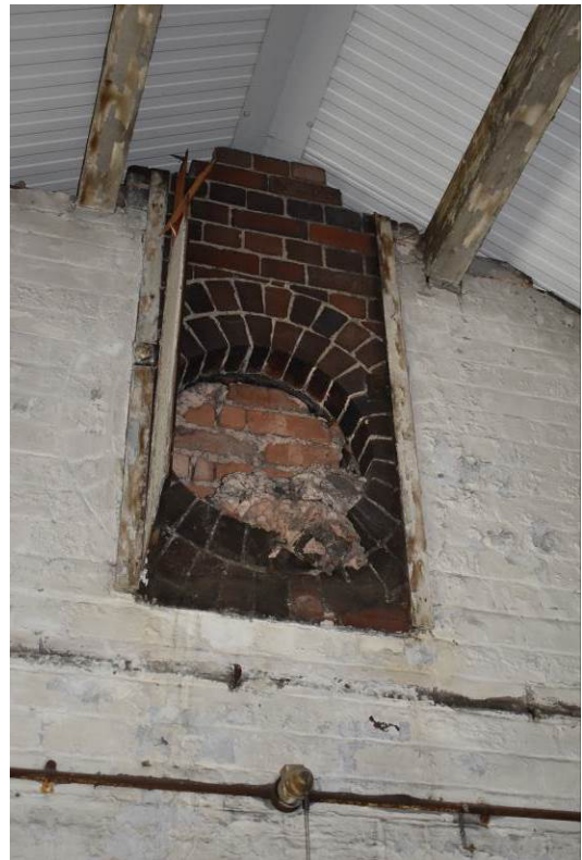
Plate 119: Circular apex vent at Bay 10/11.
