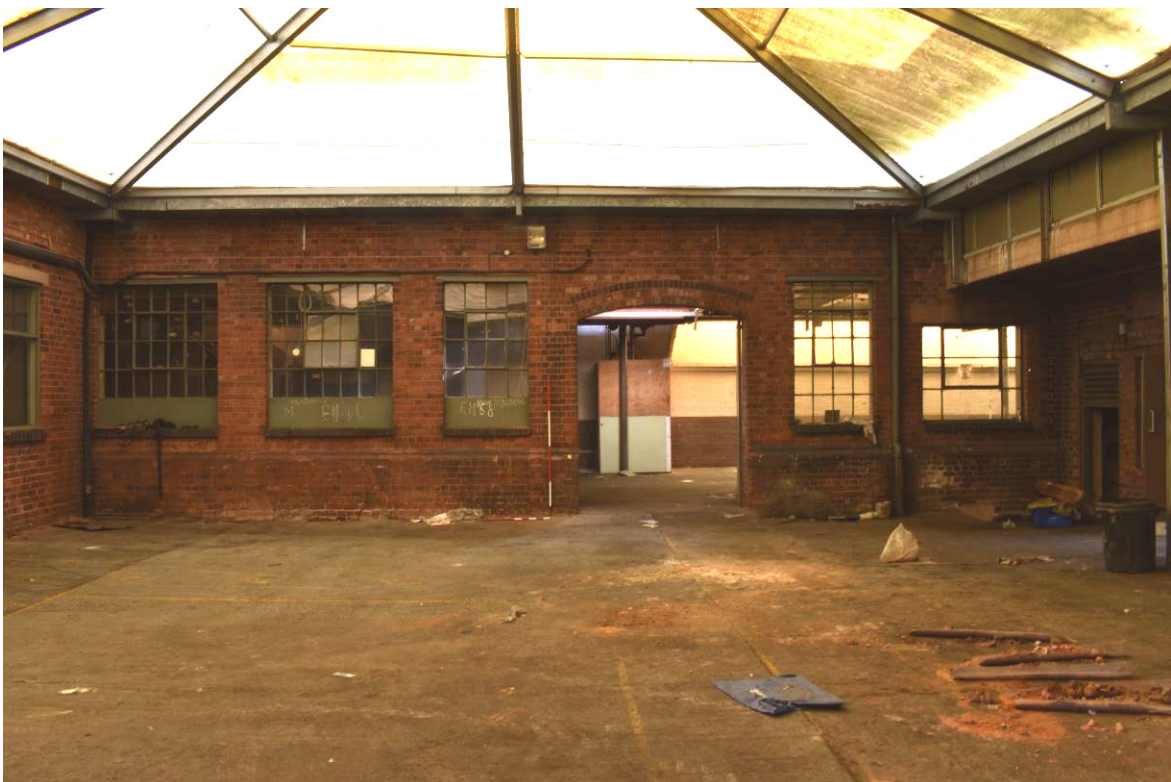
Plate 262: Bldg. 13a, west elevation (GF) as seen from covered yard 13j.
