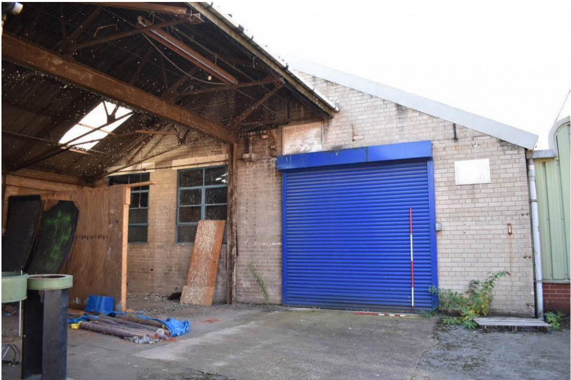
Plate 214: Building 11c: east elevation to yard.
