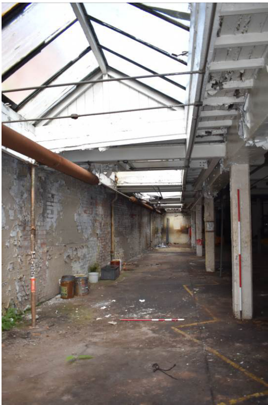
Plate 299: Building 13d, ground floor looking north beneath single-storey section.
