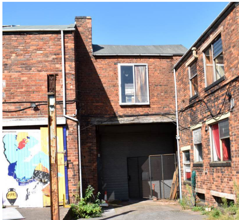
Plate 194: Building 11a; eastern section over access bay.
