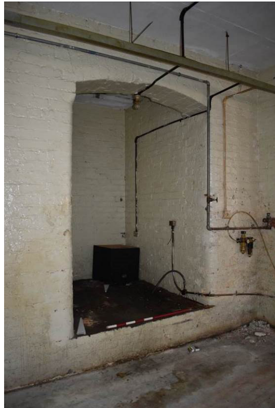
Plate 206: Building 11b; recess to north elevation: Bay 5.
