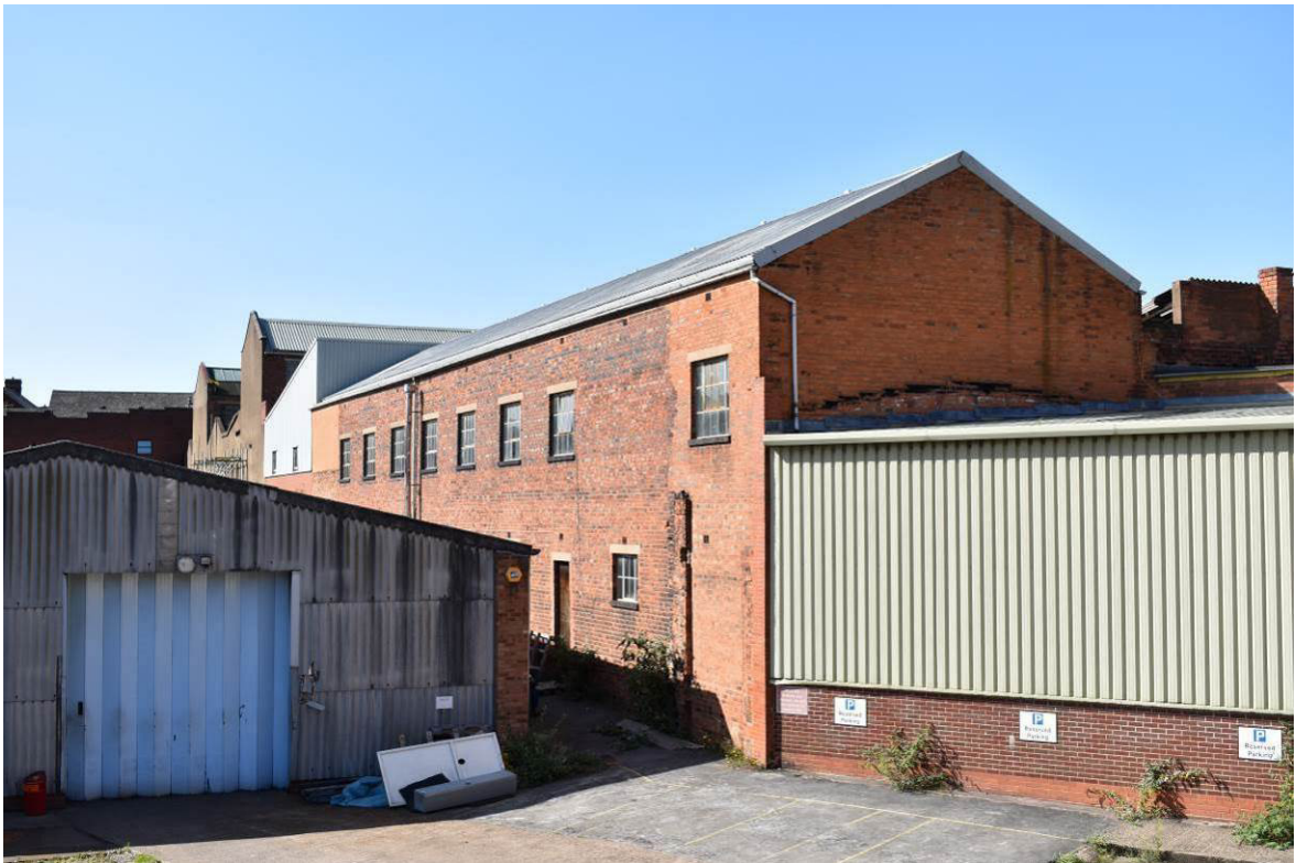
Plate 203: Building 11b; south elevation looking north-west (Bldg. 15c to left, Bldg. 10d to right); NB. rebuilt end bay.
