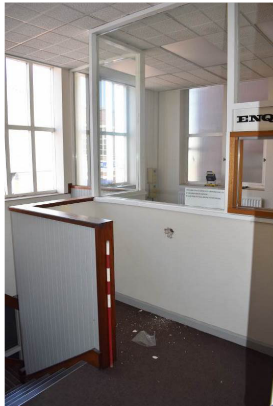
Plate 274: Building 13a; 1F landing of stair A.
