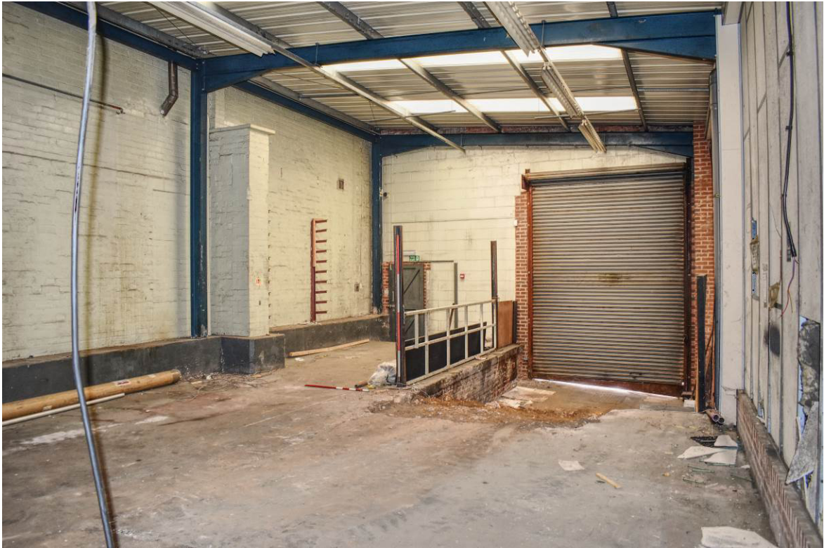
Plate 184: Building 10d, interior looking east (NB. stub wall to left).
