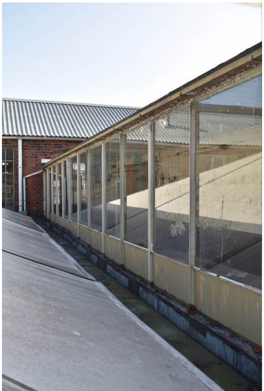
Plate 327: Raised link 13i (seen from 1F level of 13d).
