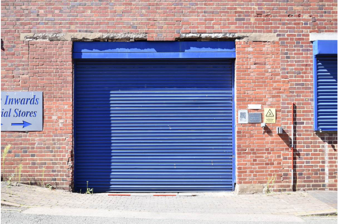
Plate 58: Building 7a; vehicular doorway [d2] inserted at Bay 5/6 of Northwood Street elevation.
