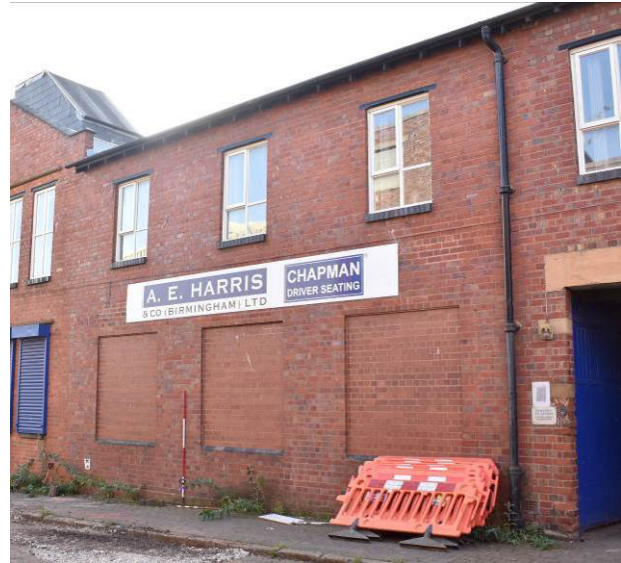
Plate 253: Bldg. 13b; north (street) elevation (1911).
