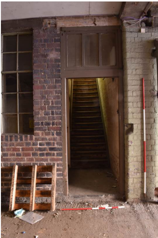
Plate 302: Building 13d: stair D rising at Bay 1.
