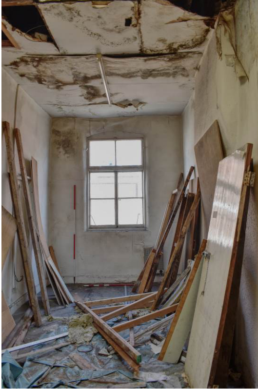
Plate 169: Room [LF1] looking east.
