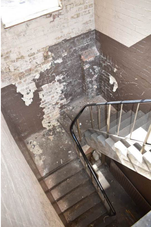
Plate 324: Stairwell F opening off south side of link 13i.
