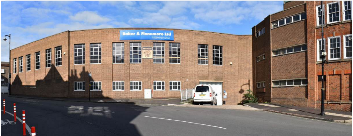
Plate 343: Building 15a/b: elevation to Graham Street.
