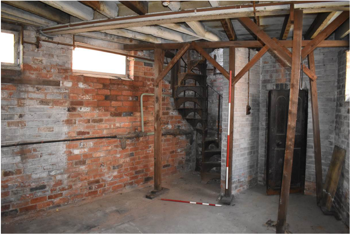
Plate 140: Building 10a basement [B1] looking north (strong room door to right).
