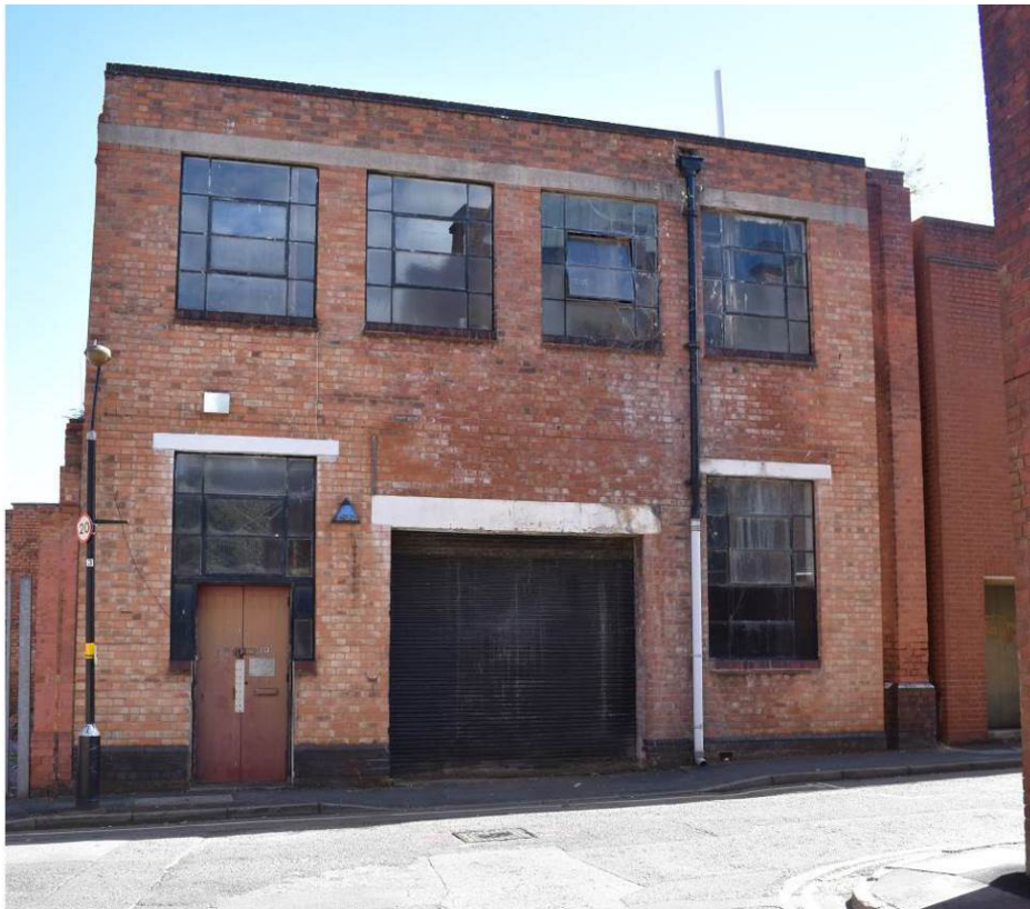
Plate 20: Building 5; north elevation to Regent Place with central roller door [d1].
