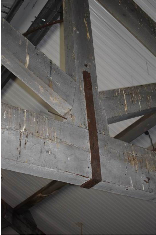
Plate 116: Strapped, joggled king-post with raking struts.
