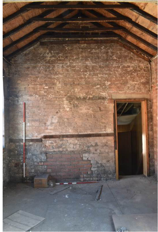
Plate 202: Building 11a: room above entrance bay, looking east.
