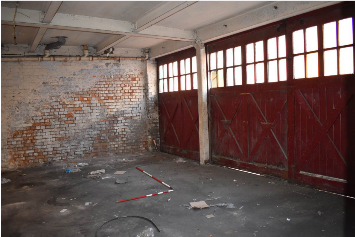
Plate 291: Building 13c; vehicular garage [G6] looking north-west.
