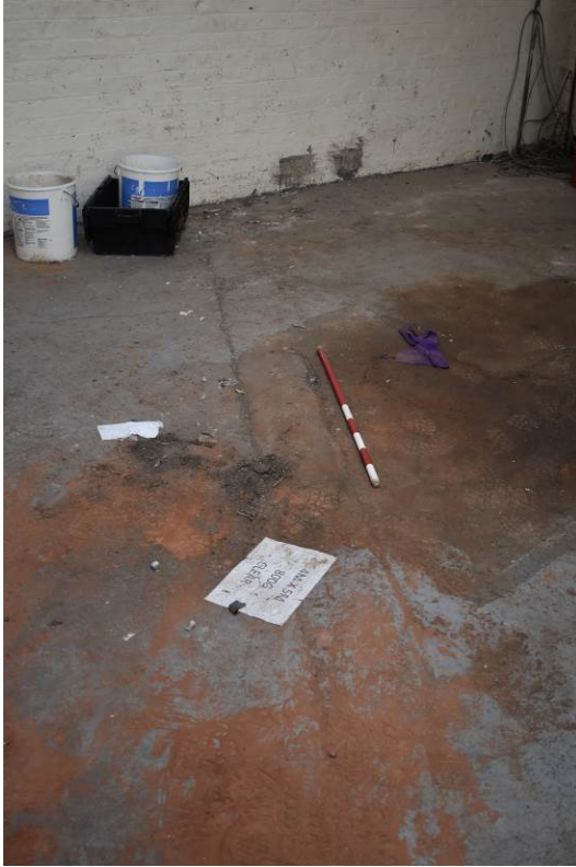
Plate 178: Scar in floor of 10c indicating eastern limit of early shopping range (removed 1927-47).
