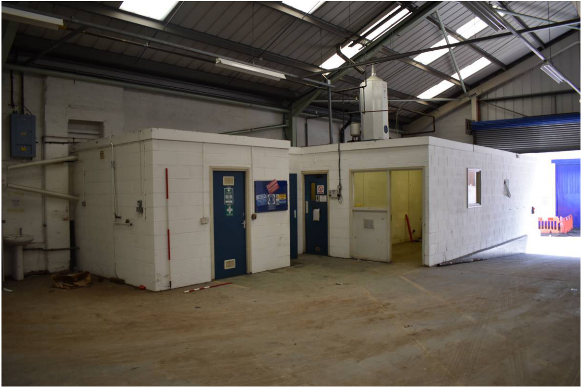
Plate 14: Building 4: inserted office / mess room / toilets at east side of Bays 2/3.
