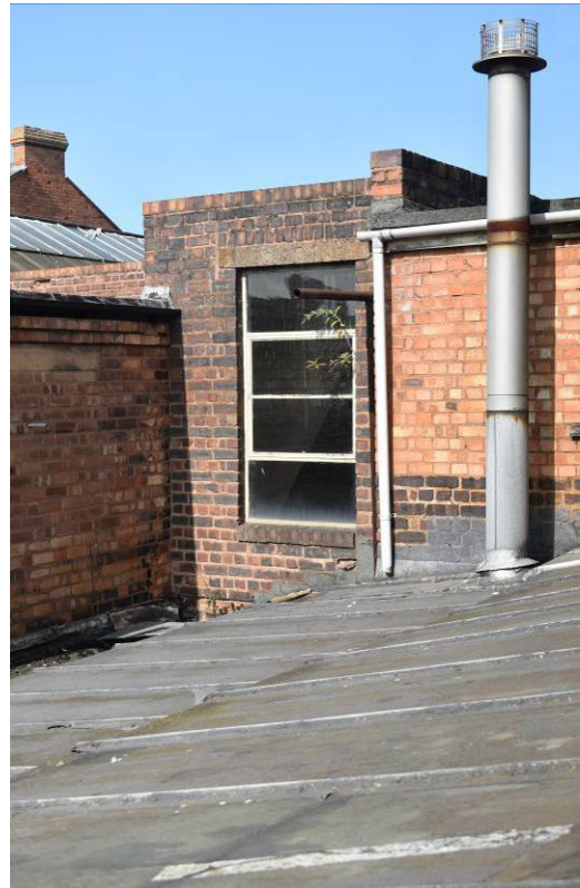
Plate 323: Boiler room 13h and stair F from 1F of 13a.
