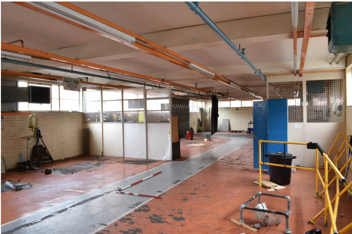
Plate 357: Building 15a; first floor looking east.
