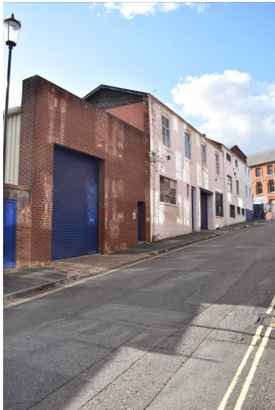
Plate 181: Bldg. 10d, streetscape looking north.
