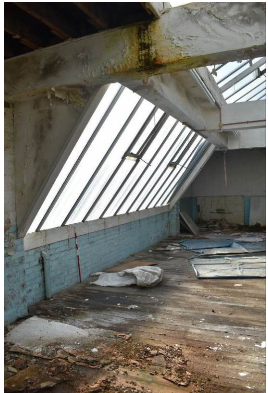
Plate 38: Building 5; 1F patent-glazed roof slope to east side of Bays 3/4.
