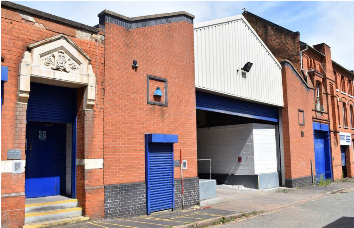
Plate 10: Building 4 (113 Northwood Street); south elevation to Northwood Street looking north-east (with Bldg. 6 top left and Bldg. 1 to right).
