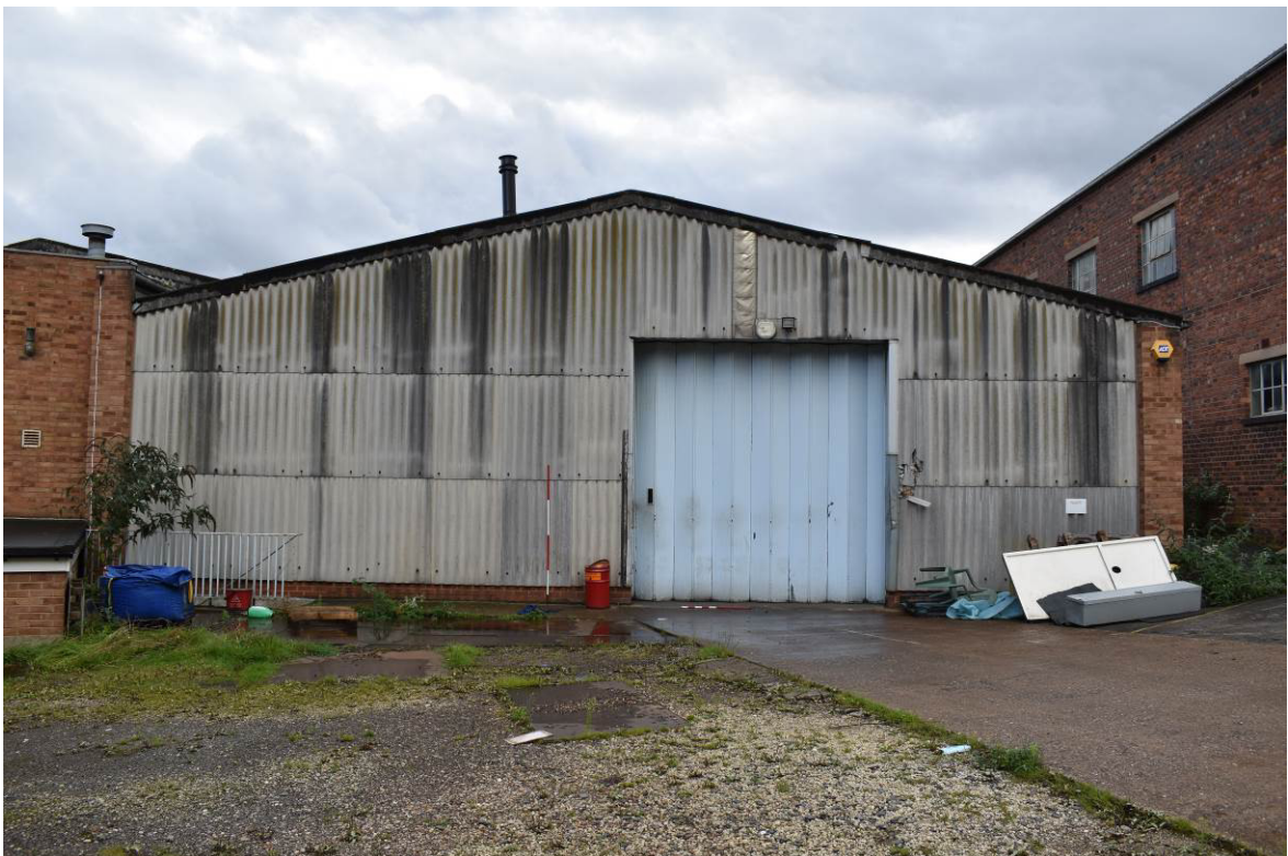
Plate 370: Building 15c; east gable end to yard.
