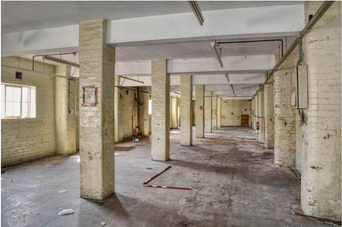
Plate 204: Building 11b; interior at basement (lower ground floor) level, looking west.
