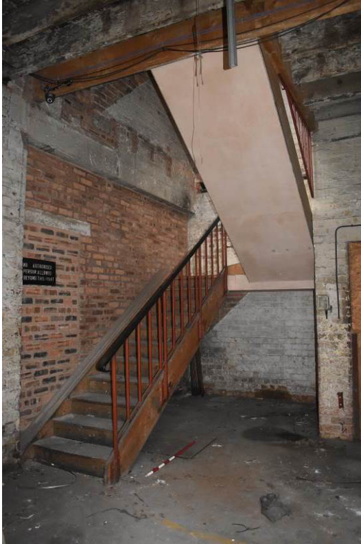
Plate 105: Stair C at GF level, Bay 14; NB. wall string cutting across blocked door in north wall.
