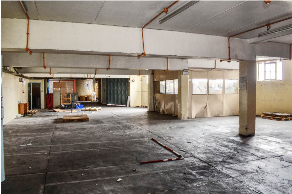
Plate 365: Building 15b; ground-floor level looking east.
