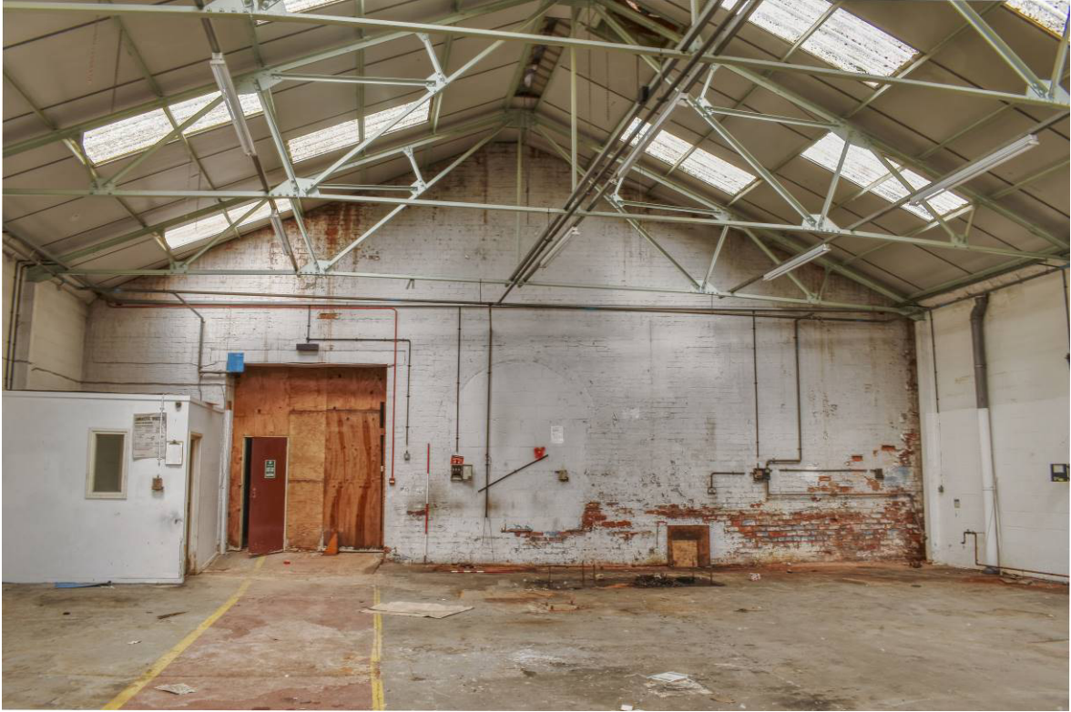
Plate 16: Building 4: north wall with inserted opening to Building 5 (left).
