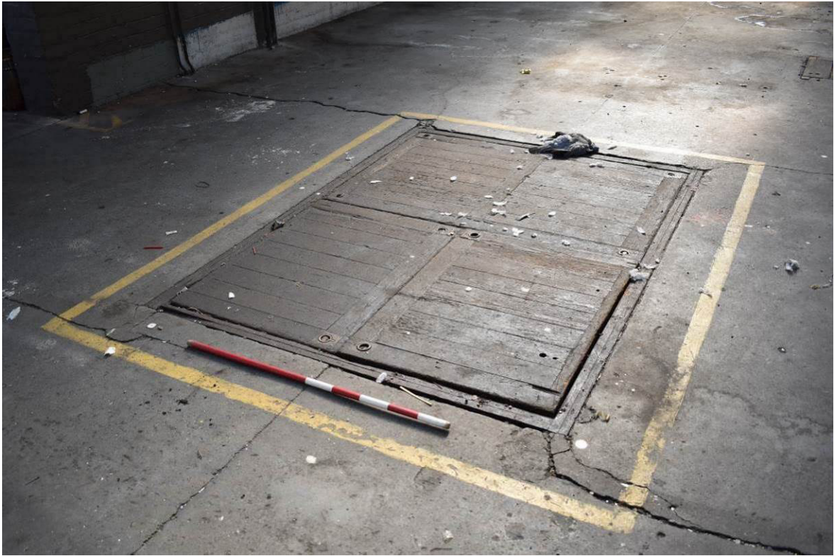
Plate 308: Shopping range 13d; first-floor floor hatch at Bay 4.
