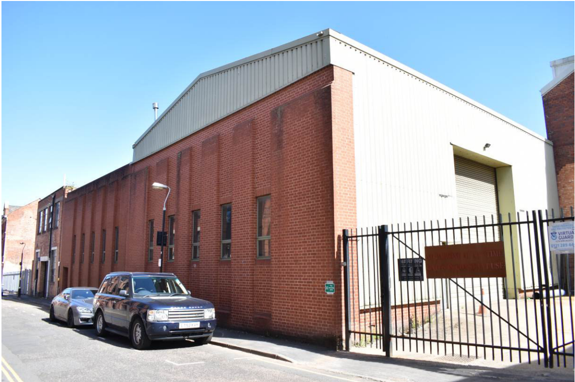
Plate 49: Building 6: north elevation to Regent Place; oblique view looking south-west.
