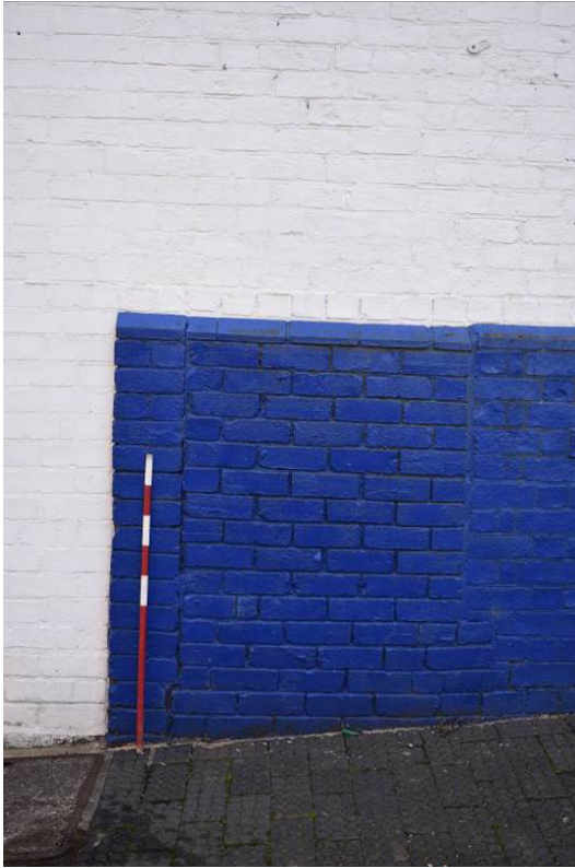
Plate 133: Building 10a; blocked opening to plinth.
