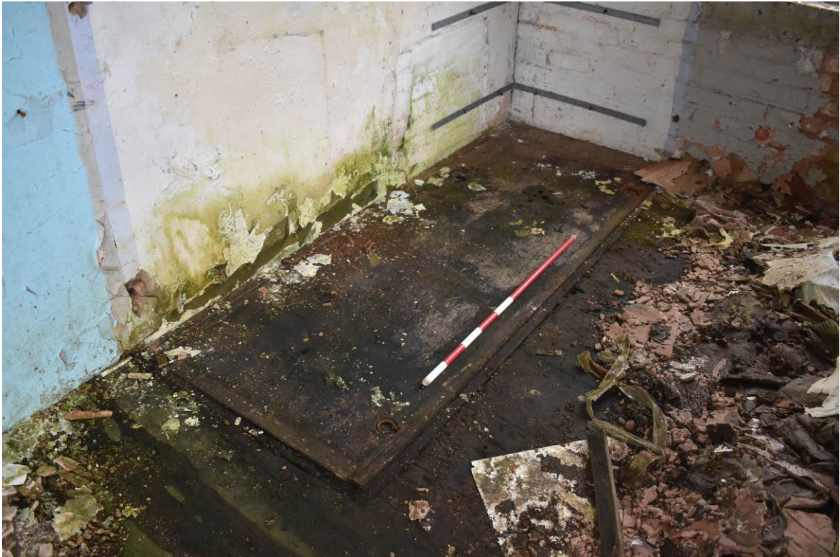
Plate 39: Building 5; hatch over hoist void at north-west angle of 1F.
