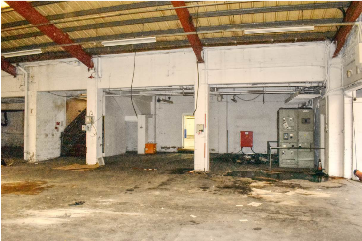
Plate 74: [G5] at Bays 4-6, looking east from covered yard 8.
