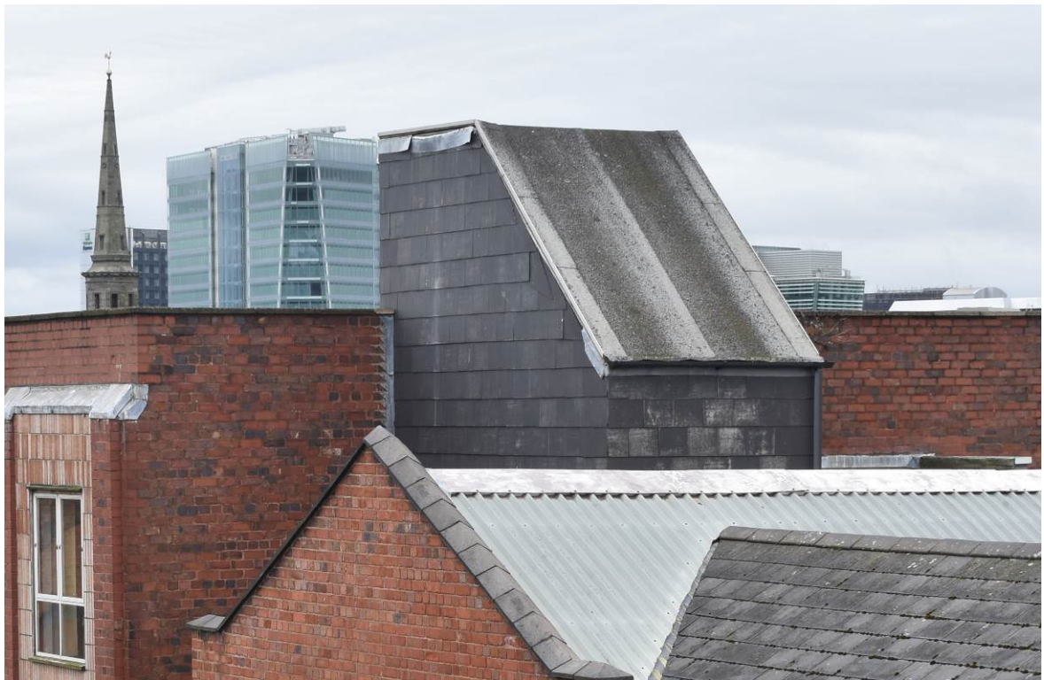
Plate 235: Secondary stair well rising from Bldg. 13 to 2F level of Bldg. 12.
