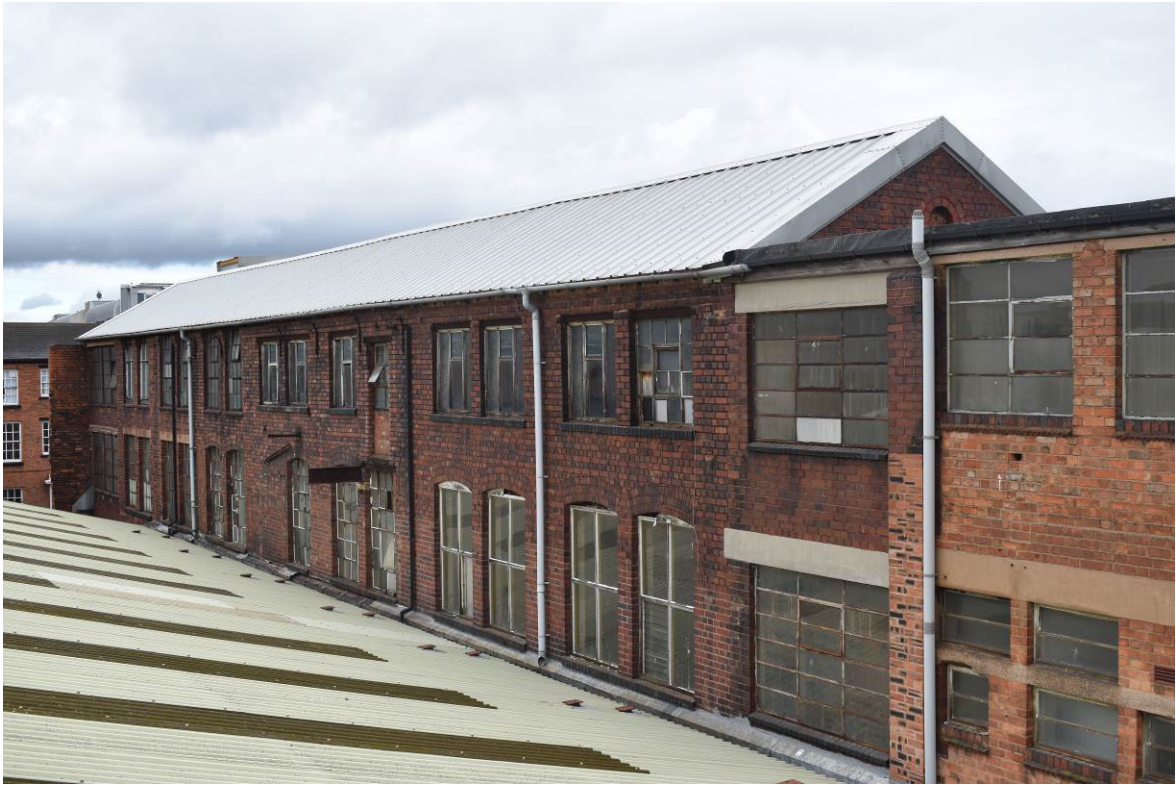
Plate 90: West elevation of Bldg. 7b seen from flat roof of 7a .
