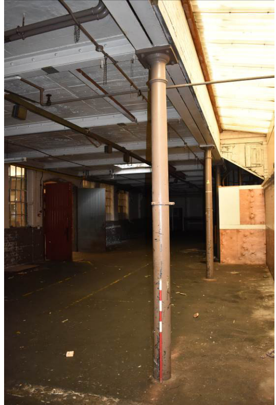
Plate 276: [G2] looking north beneath eastern sky-light with cast-iron support column.
