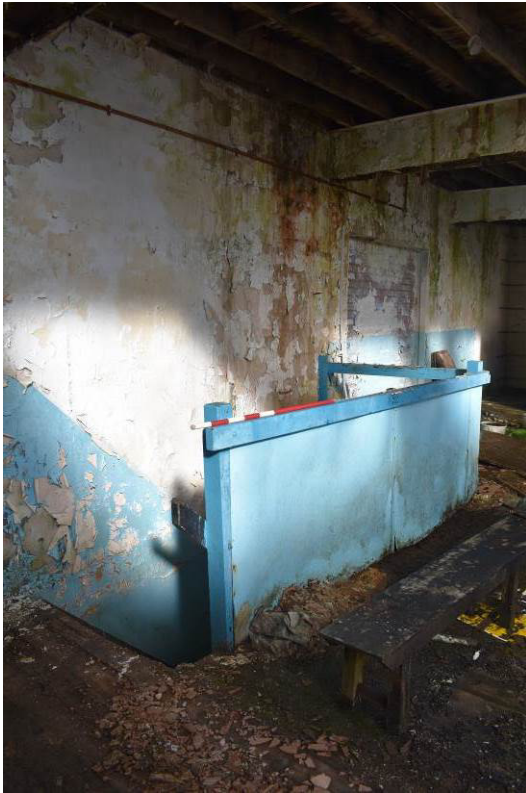
Plate 35: Building 5; head of stair A at 1F level.
