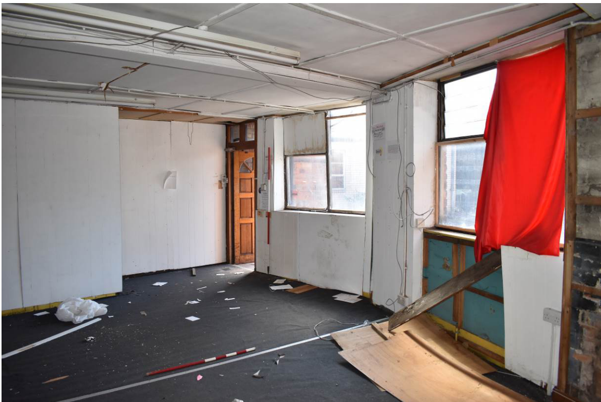
Plate 148: Room [UG1] looking south-west.
