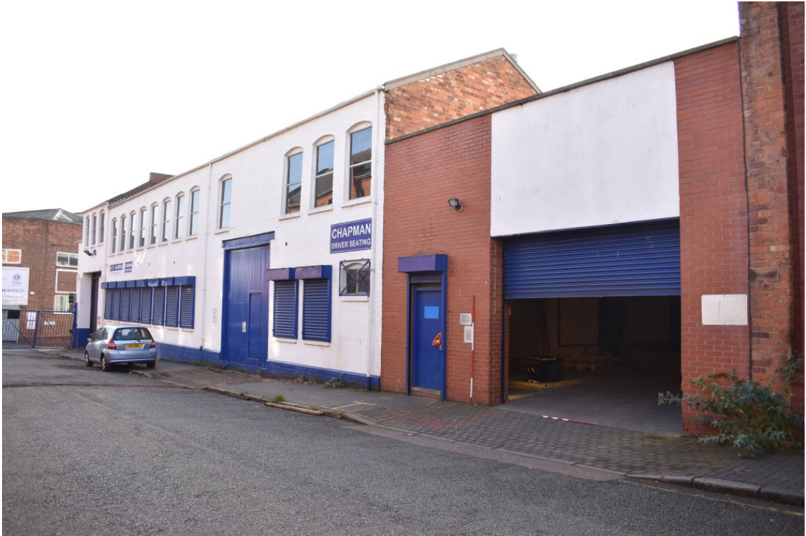
Plate 186: Building 11a; street elevation to Northwood Street (oblique) looking south-east.
