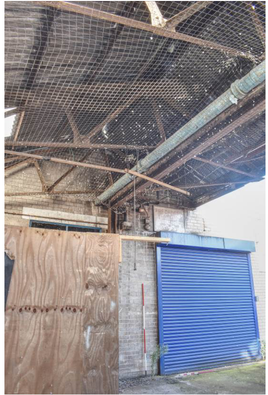
Plate 224: Covered yard 11f adjacent to Bldg. 11c.
