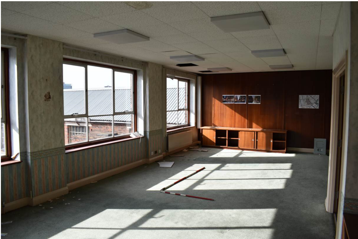
Plate 245: Bldg. 12a: second floor office [S6] looking south-west.
