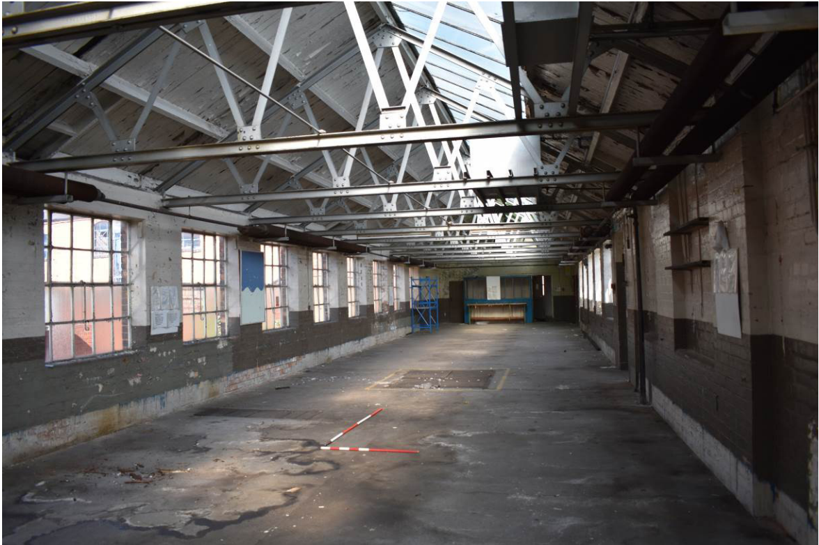
Plate 306: Shopping range 13d; first-floor level [F12], looking north.
