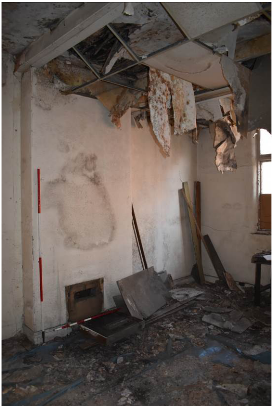
Plate 172: Chimneybreast to north wall of [LF2].
