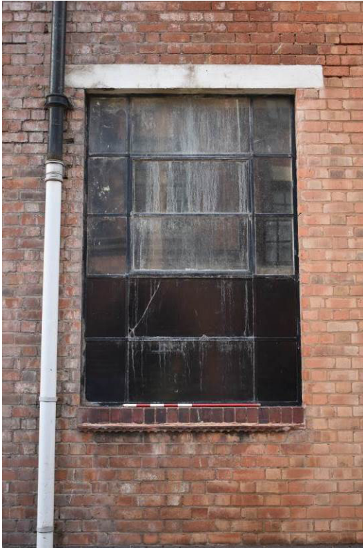
Plate 21: Crittall-type steel casement window [w1].
