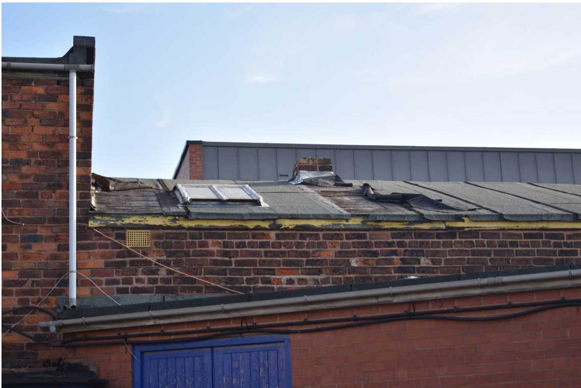
Plate 159: Bldg. 10b, upper rear (west) elevation visible from yard, above 10c.
