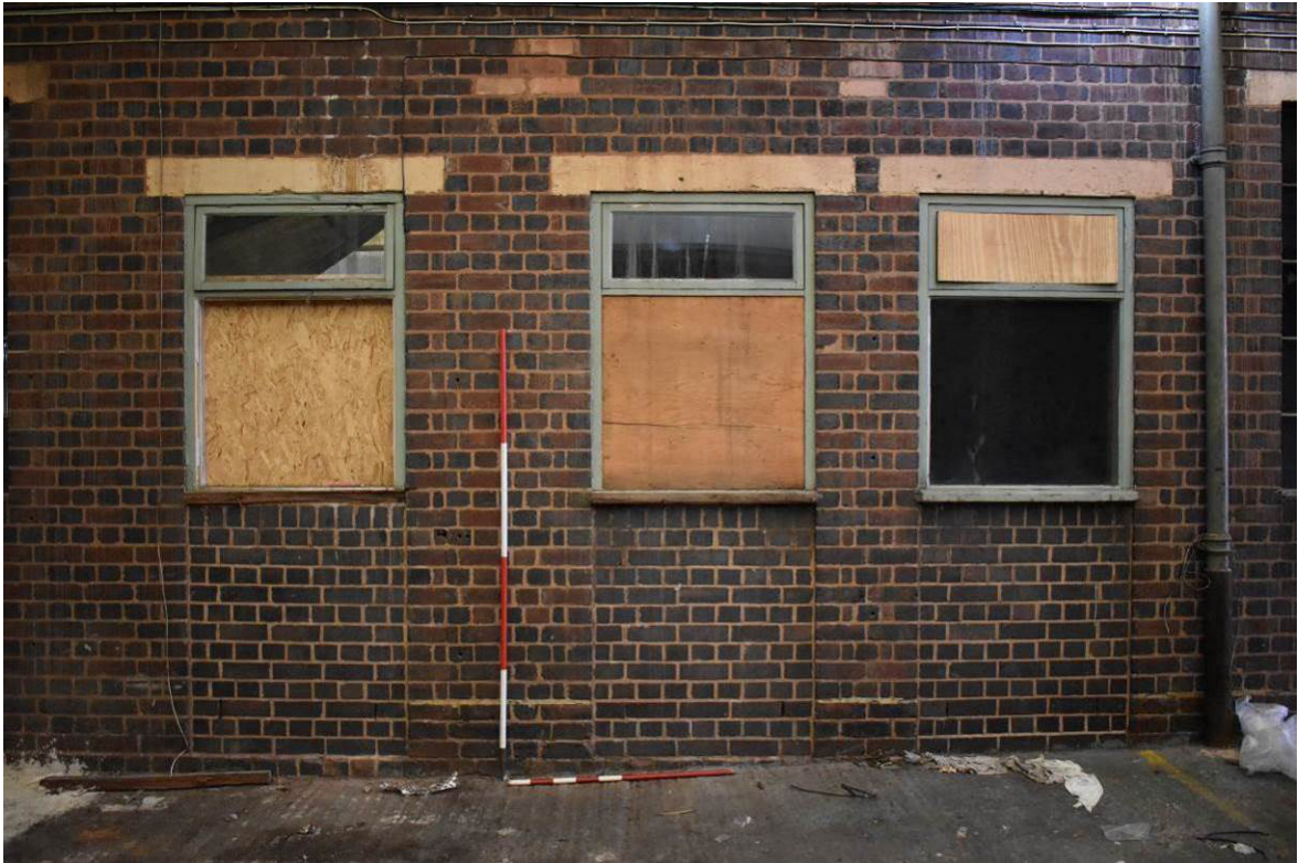
Plate 296: Partly blocked/converted doors formerly serving coal / coke / petrol stores.
