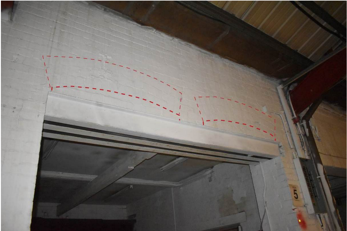
Plate 95: Building 7b; west elevation, relic triple-header brick arches at Bay 9 denoting former GF window openings.
