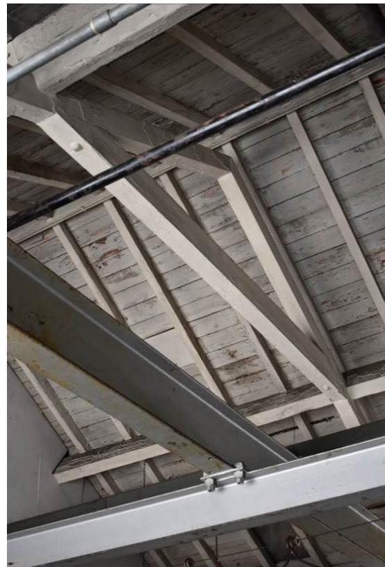
Plate 285: Roof structure over Bldg. 13a.
