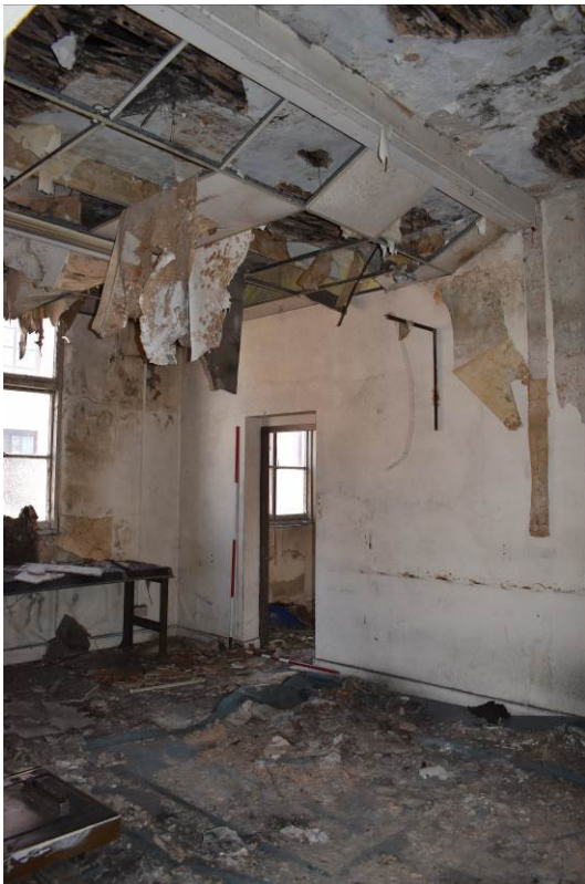
Plate 171: Room [LF2] looking south-east.
