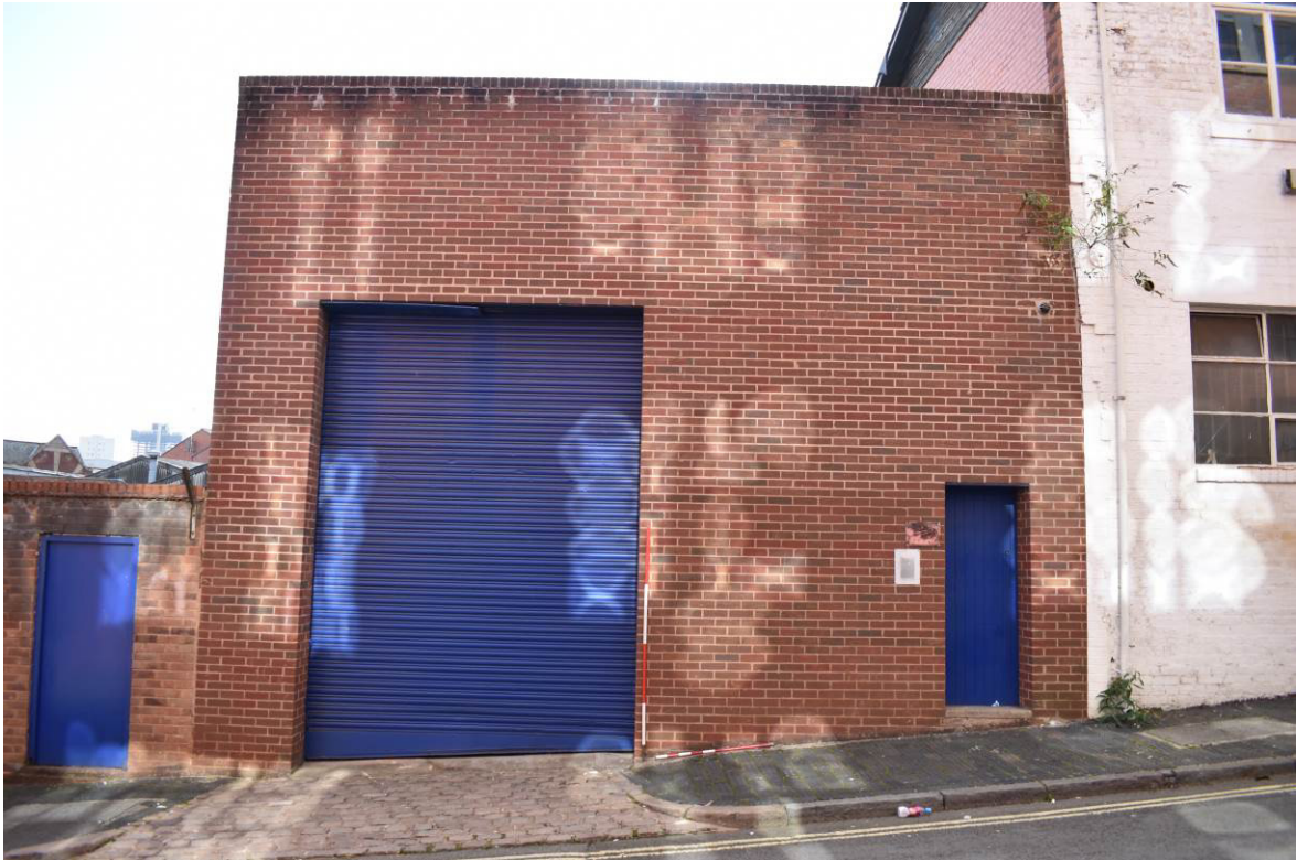
Plate 182: Bldg. 10d., east elevation to James Street.
