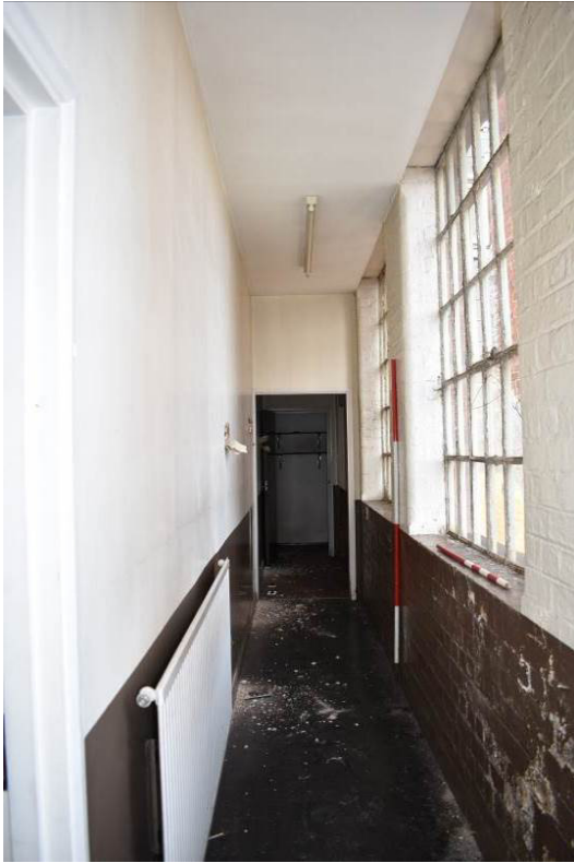
Plate 282: Corridor [F16] looking north.
