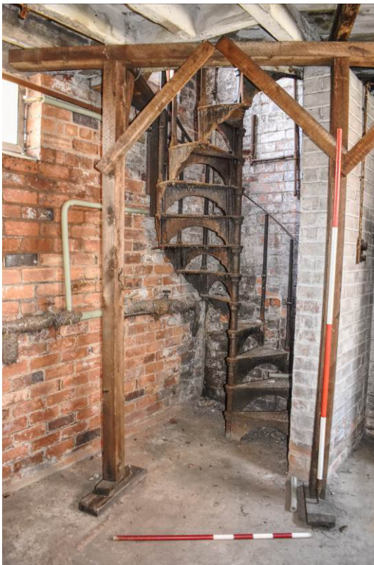
Plate 145: Spiral stair A at corner of [B1].
