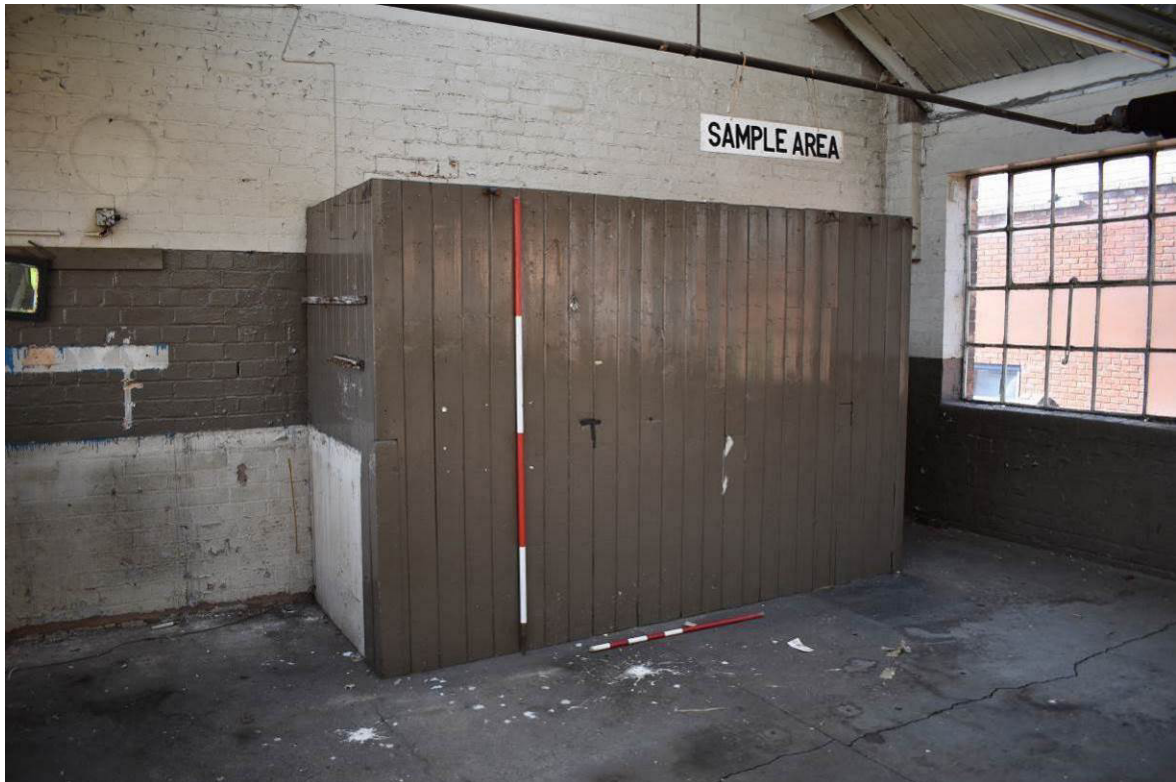
Plate 304: Building 13d: head of stair E at Bay 7.
