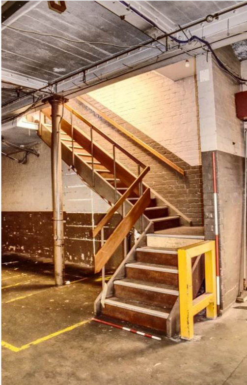
Plate 279: [G2]; inserted stair B rising at Bay 3 (E).
