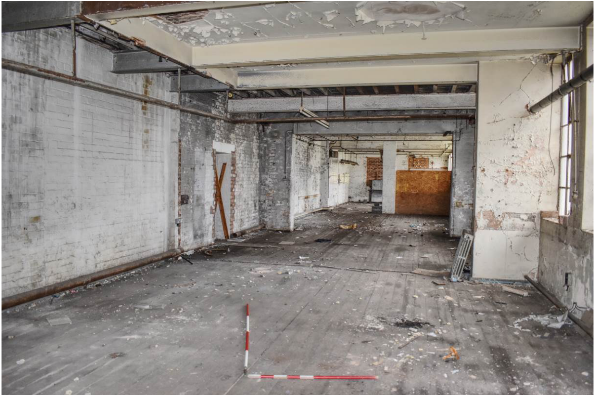
Plate 109: Building 7b; first floor looking south from Bay 13.
