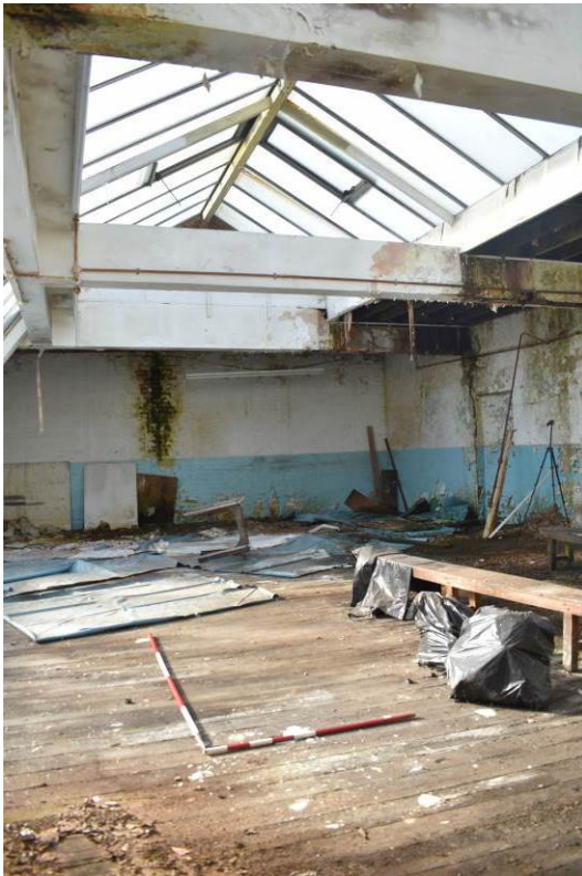
Plate 37: Building 5; 1F level looking south with pitched roof-light over.
