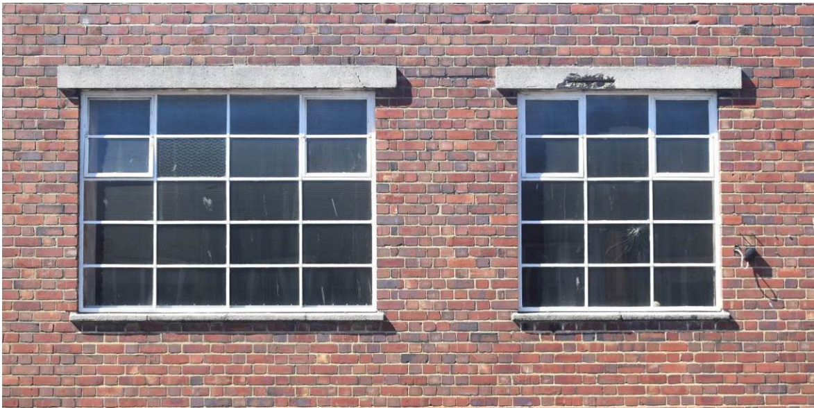
Plate 57: Building 7a; 'Crittall'-type steel casement windows.
