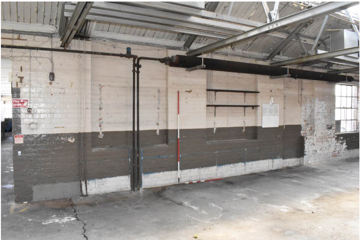
Plate 316: Blind windows and blocked door to 1F 13d (Bays 5/6), backing onto contemporary Bldg. 13e.
