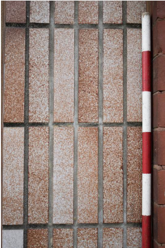
Plate 232: Building 12a; detail of tile cladding (post-1964).
