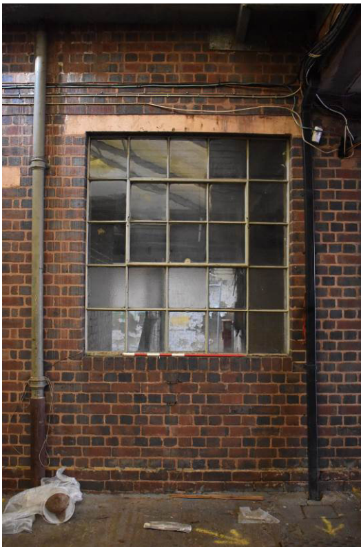
Plate 294: Building 13d : detail of GF window.
