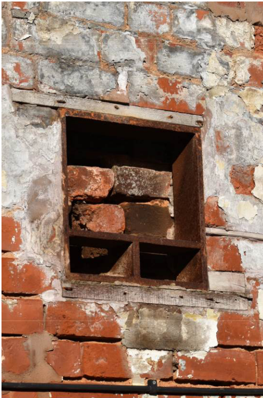
Plate 25: Remains of 'wall box' for former line-shafting.
