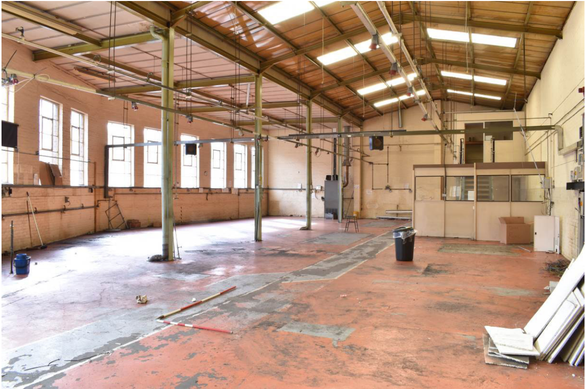
Plate 367: Building 15b; first-floor level looking west.
