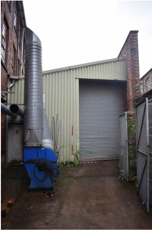
Plate 120: Building 8, north elevation.
