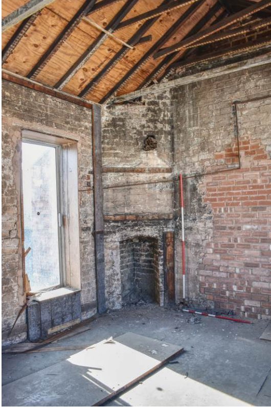
Plate 201: Building 11a: room above entrance bay.
