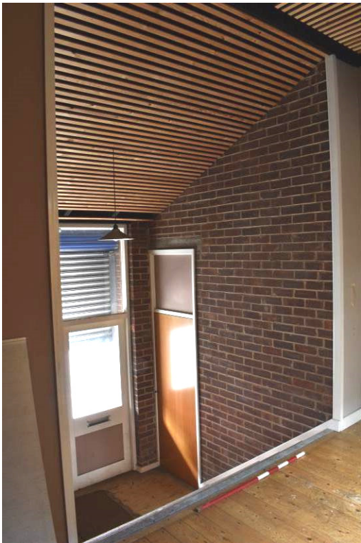
Plate 342: Detail of modernised entranceway at [G9].
