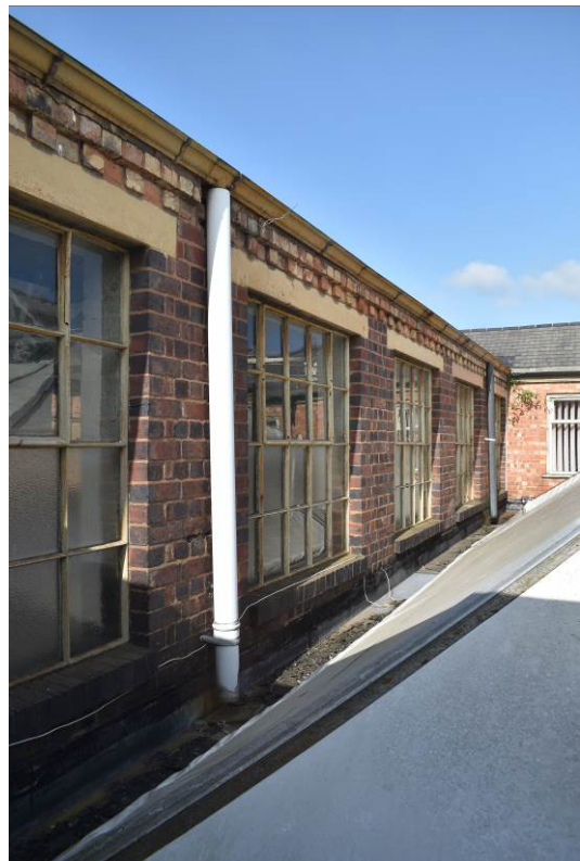
Plate 295: Building 13d : 1F (E) Bays 2/3, looking north.
