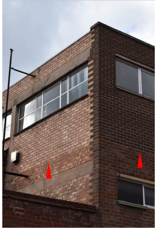
Plate 347: Detail of change in brickwork at SE angle.
