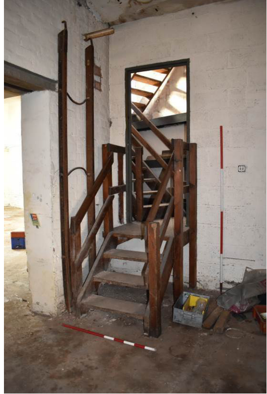
Plate 161: Inserted stair C to west side of [LG1].
