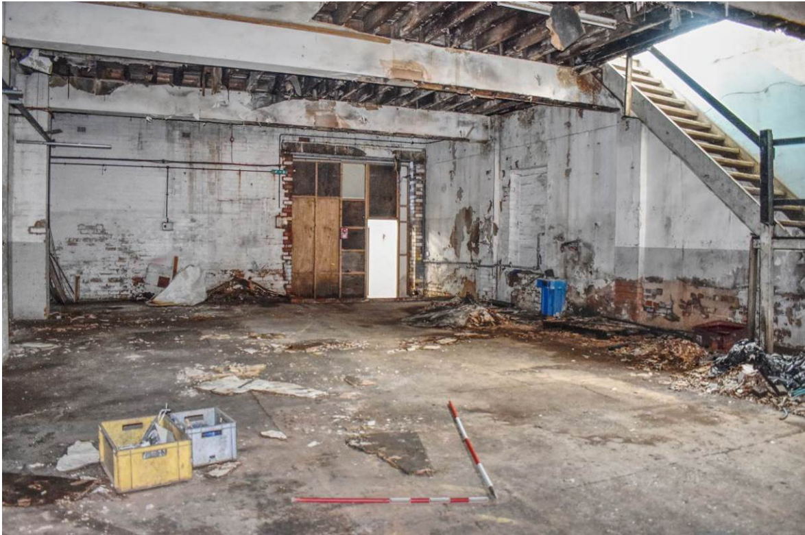
Plate 29: Building 5; ground floor [G1] looking south.
