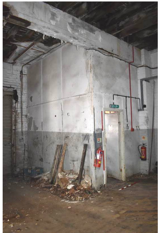
Plate 31: Building 5; enclosed stair B to NE angle .
