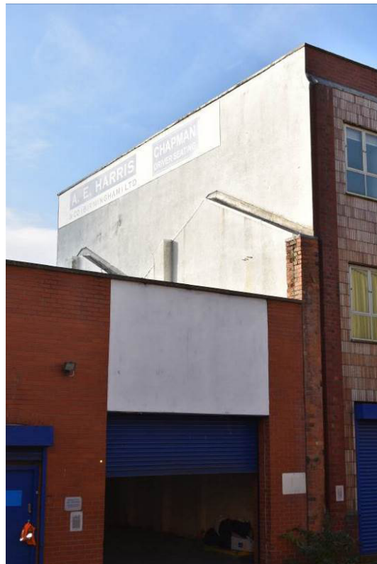
Plate 192: Building 11a: former pitched-roof profile on side elevation of Bldg. 12.
