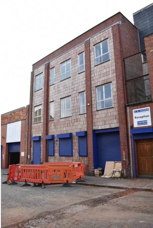
Plate 230: Building 12a; north elevation to Northwood St.
