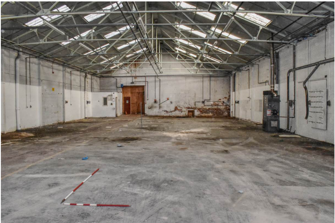
Plate 13: Building 4 (113 Northwood Street); interior looking north from Bay 5, steel-trusses Bays 4-12.
