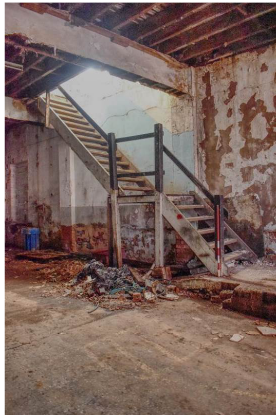
Plate 34: Building 5; stair A rising to 1F level.
