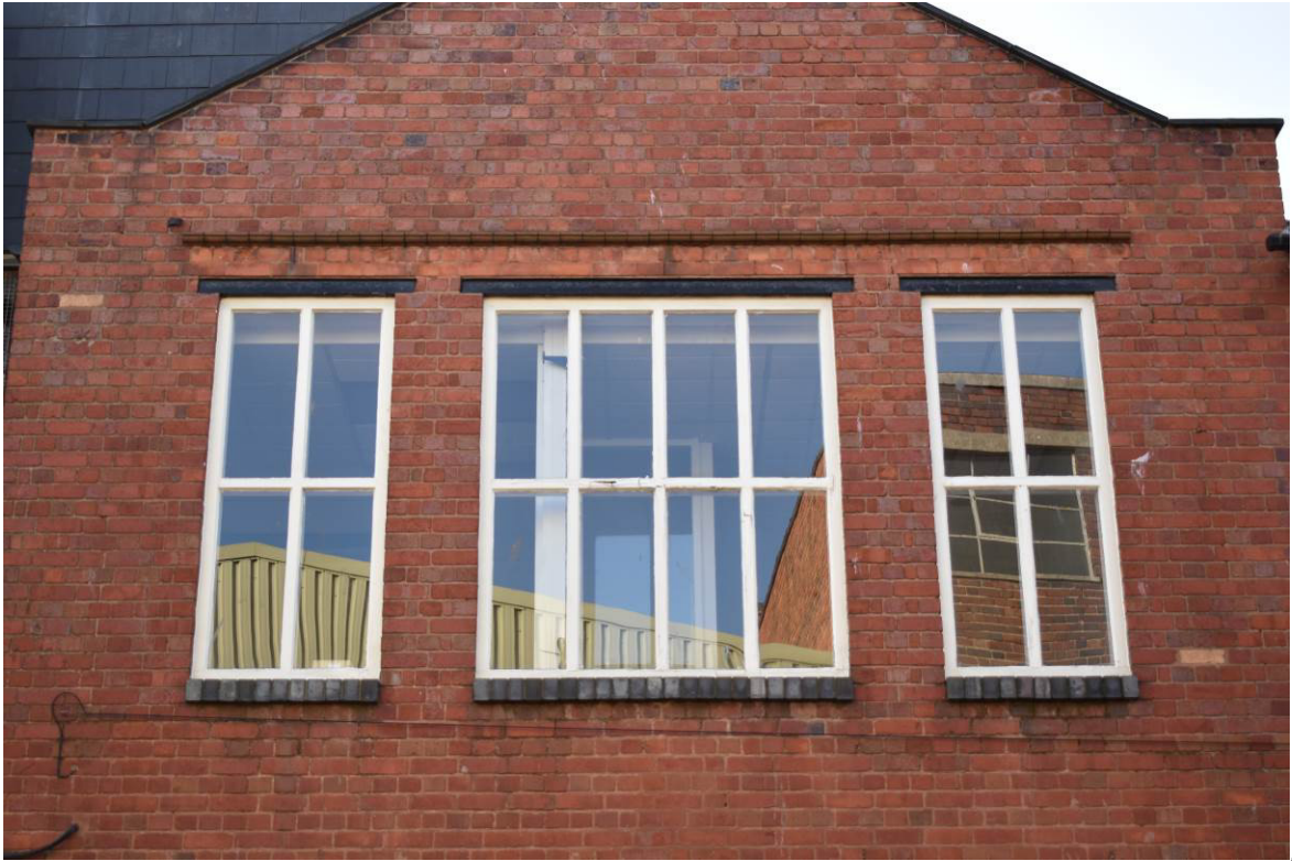
Plate 255: Building 13; first-floor fenestration details to gable end of 13a.
