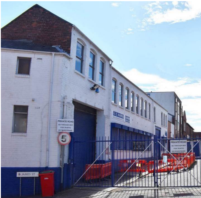
Plate 187: Building 11a; street elevation looking south-west.
