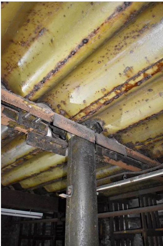
Plate 238: Bldg. 12a: [B1] ceiling structure.
