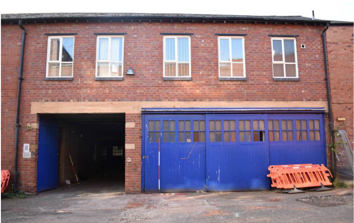
Plate 254: Building 13c; five window-bay extension of Northwood Street frontage (1920) incorporating cart entry
