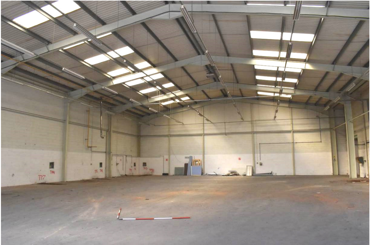
Plate 126: Building 9; interior looking north.
