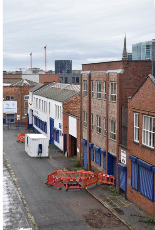
Plate 229: Building 12a within streetscape context.
