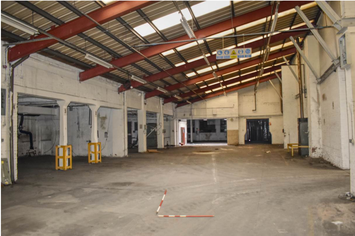
Plate 122: Covered yard 8, interior looking south with range 7b to left.
