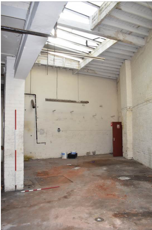
Plate 176: Covered yard 10c looking south.
