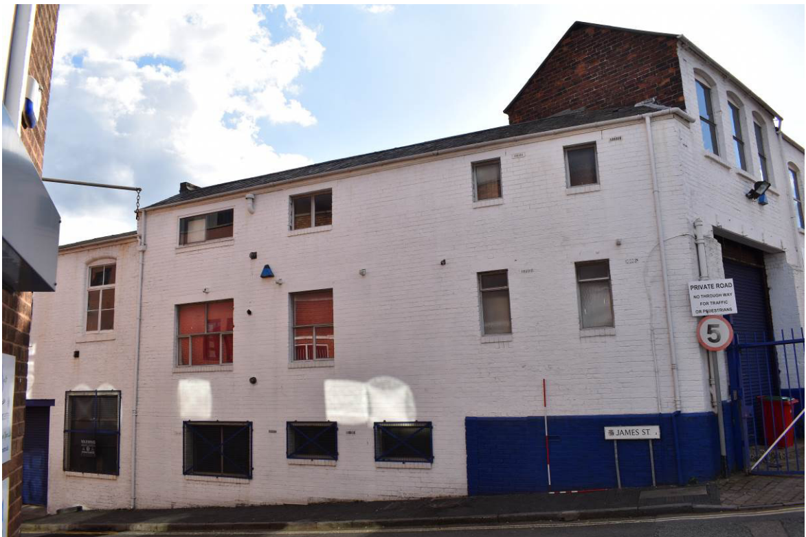
Plate 132: Building 10a (No. 10 James Street); east elevation to street. (. blue painted plinth to right may reflect former yard wall, shown on mapping on 1855 and 1870/71).
