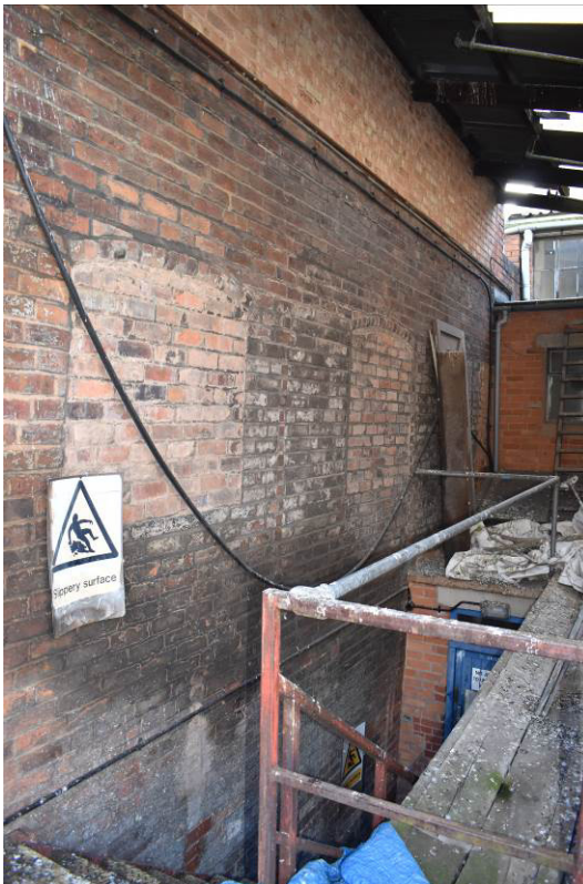
Plate 180: Blocked windows visible to west.
