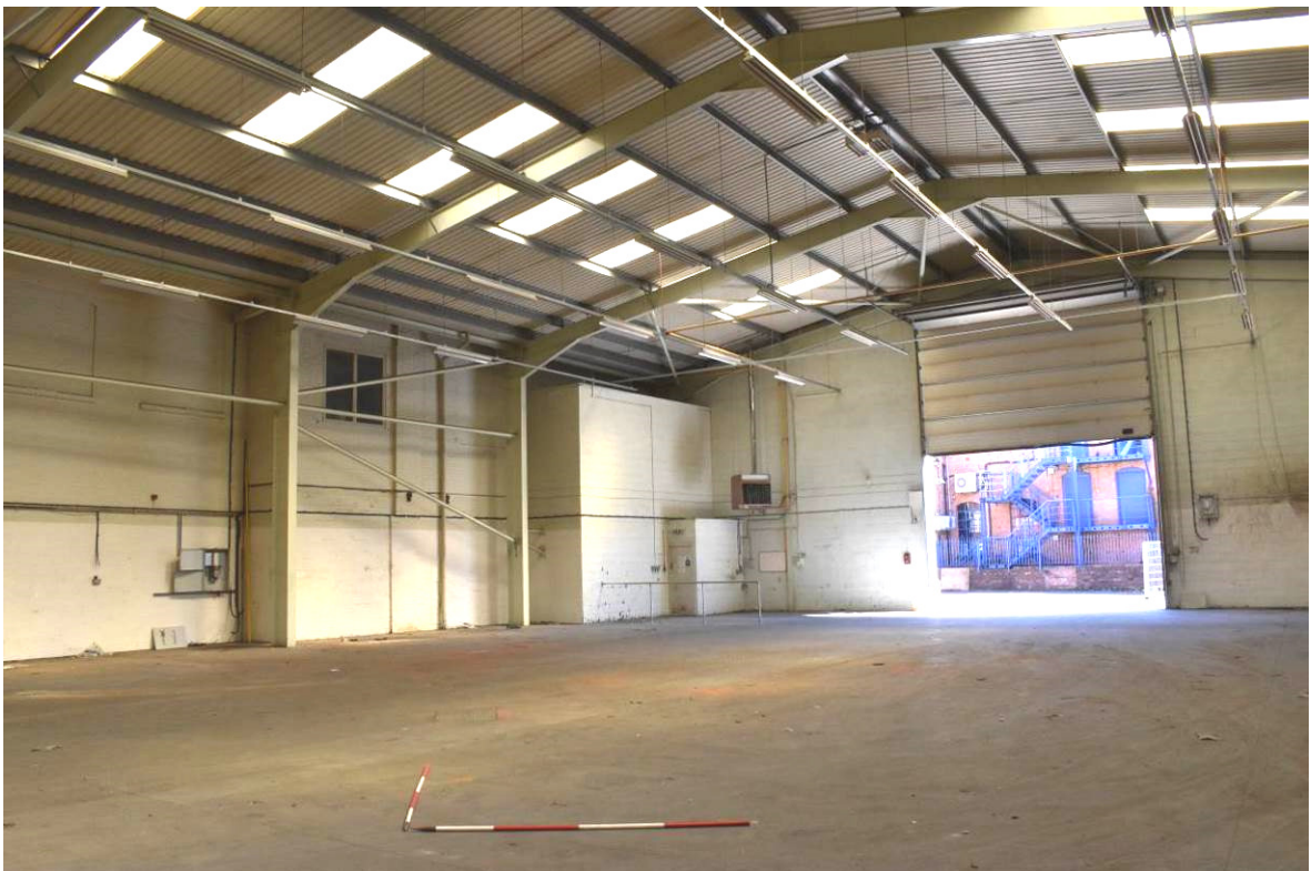
Plate 127: Building 9; interior looking south.
