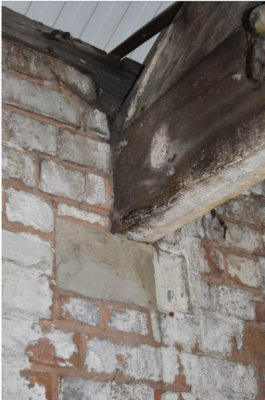
Plate 118: Tie resting on inset stone block.
