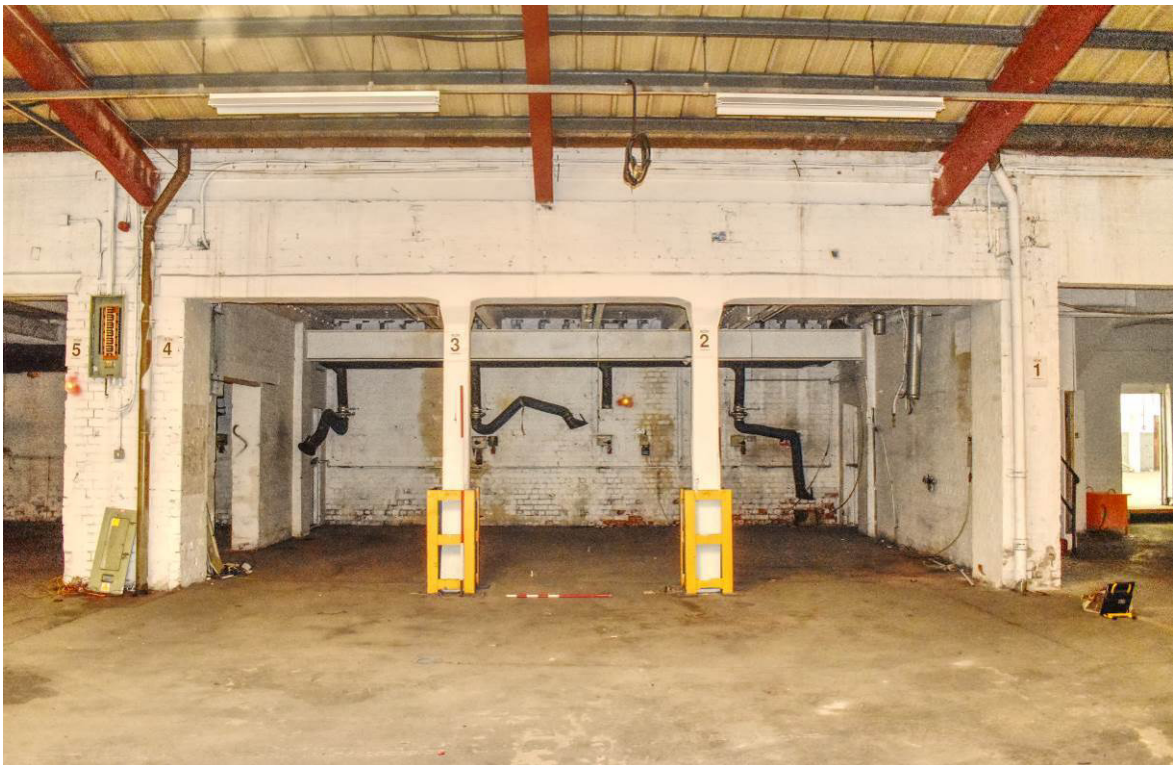
Plate 99: Building 7b; west elevation, open to yard at Bays 7/8 [G6] (original 'engine house'; formerly furnished with projecting half-glazed wall).
