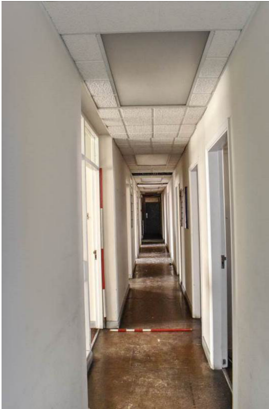
Plate 288: Building 13b: First floor corridor [F3] looking west.
