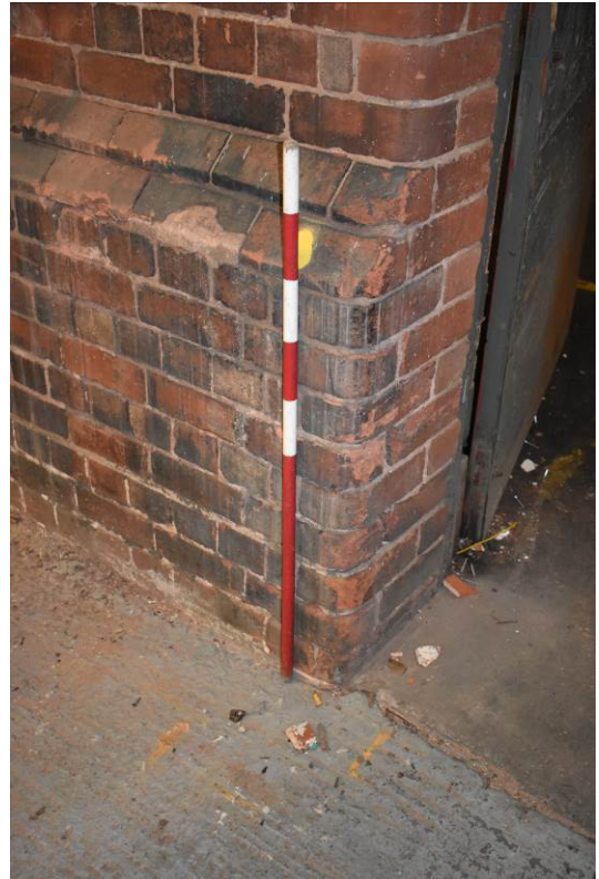
Plate 264: Bldg. 13a; chamfered plinth detail.
