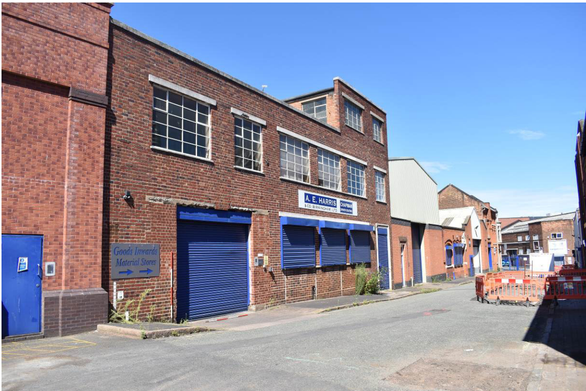
Plate 54: Building 7a; south elevation to Northwood Street looking north-east (BPP 78586, 1945).
