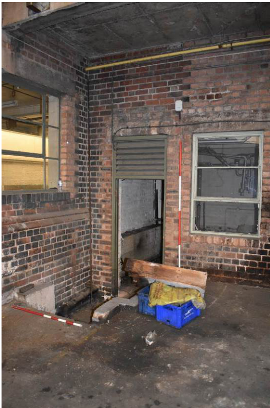
Plate 322: Boiler room 13h to SE corner of yard 13j.
