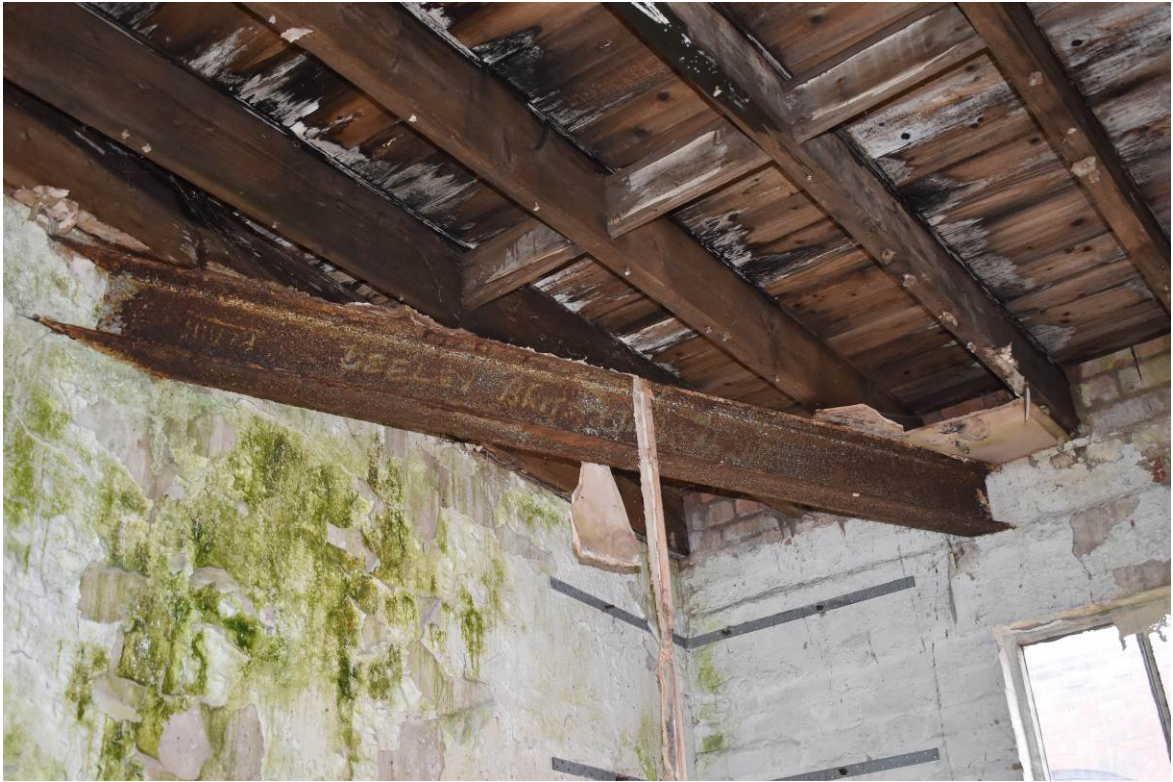
Plate 41: Building 5; angled RSJ above hoist void.
