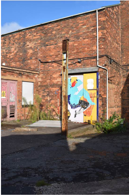
Plate 223: Free-standing steel stanchion indicating former covered loading bay serving Bldg. 11a.
