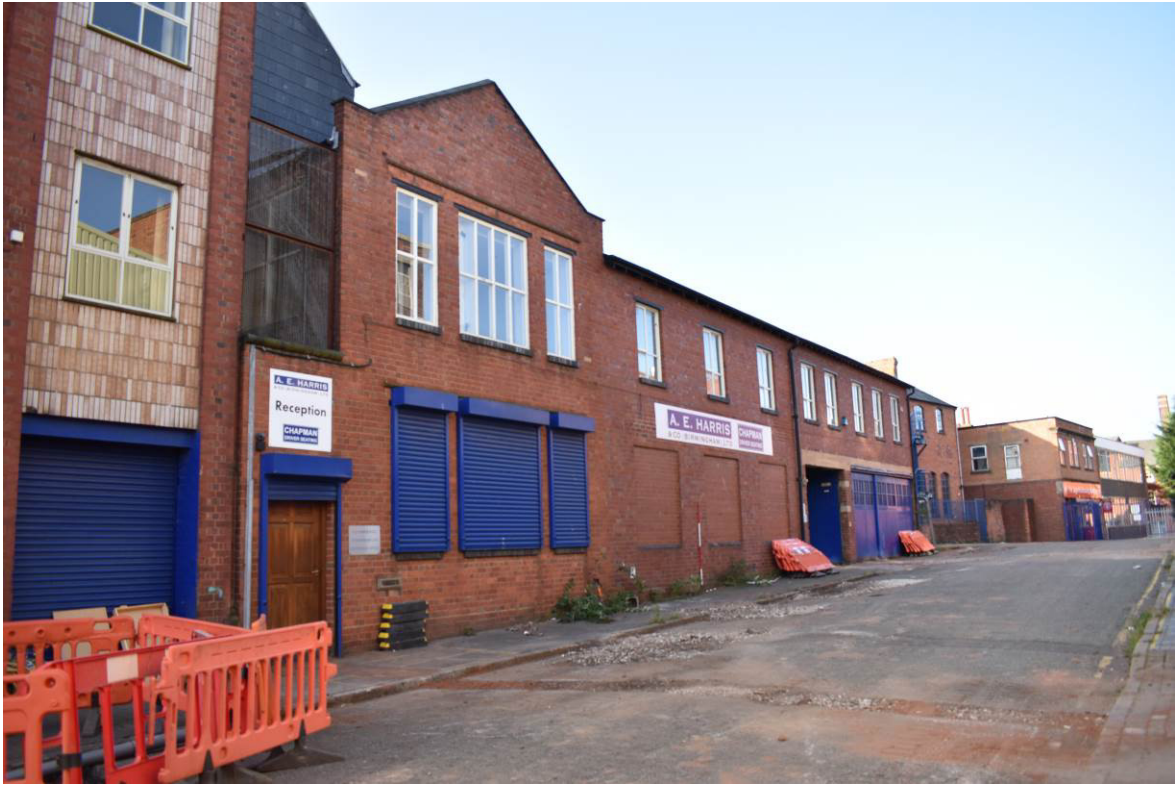
Plate 250: Building 13a-c; north elevation to Northwood Steet looking south-west (compare with image inset at §.4.10.13).
