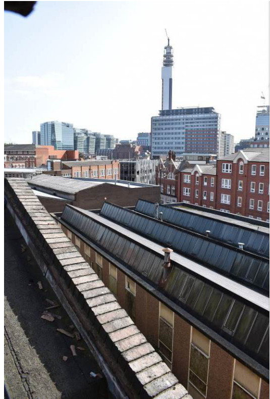
Plate 337: Building 14; view over saw-tooth roof from 2F level of Bldg. 13.
