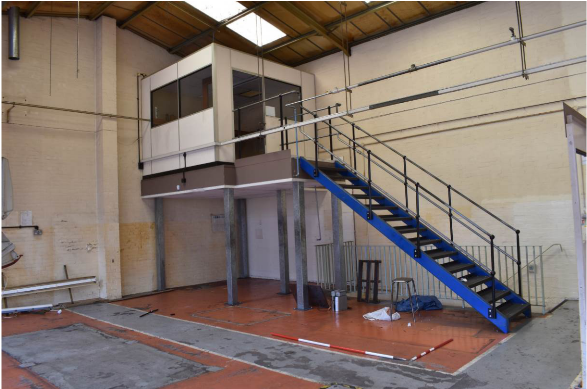
Plate 369: Building 15b; inserted, raised office to north-west corner of first floor.
