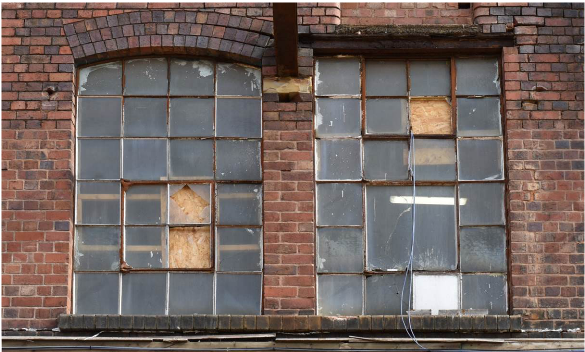
Plate 94: Building 7b: Variant window details, with multi-pane iron frames (Bay 9, 1F).
