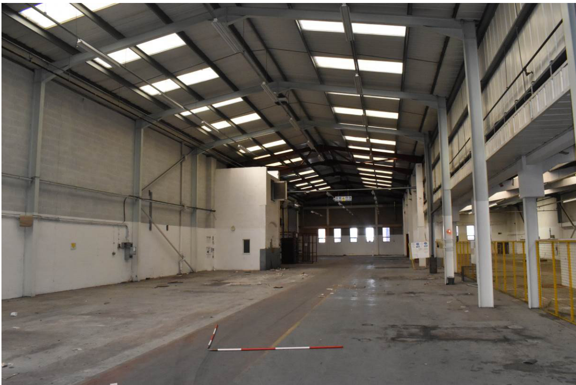
Plate 52: Building 6b: western range ([G4]; 119 Northwood Street) looking north.
