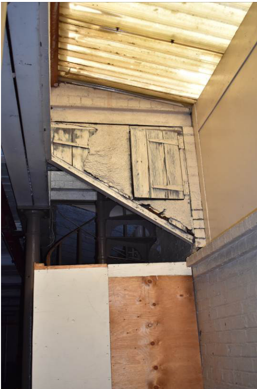
Plate 277: Original profile of eastern skylight.
