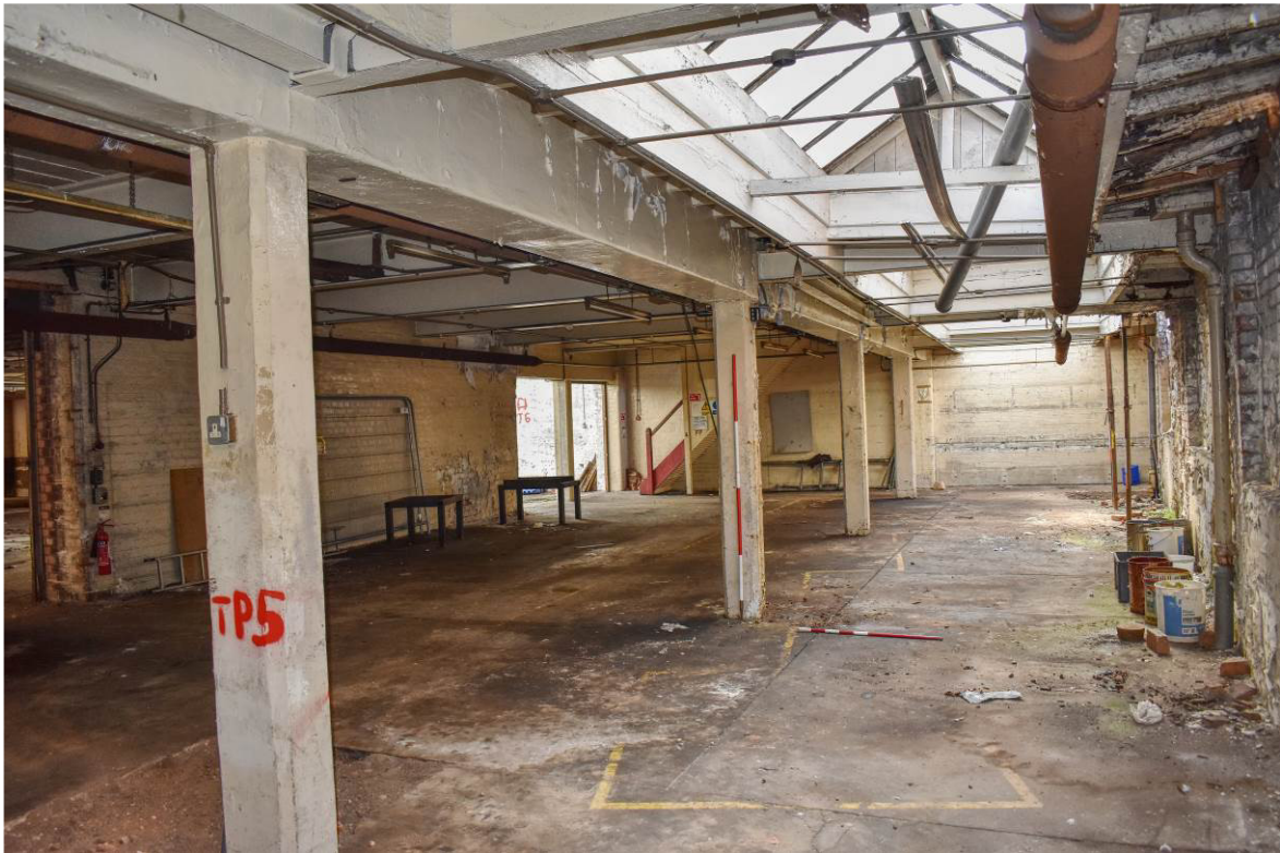
Plate 298: Building 13d, ground floor looking south.
