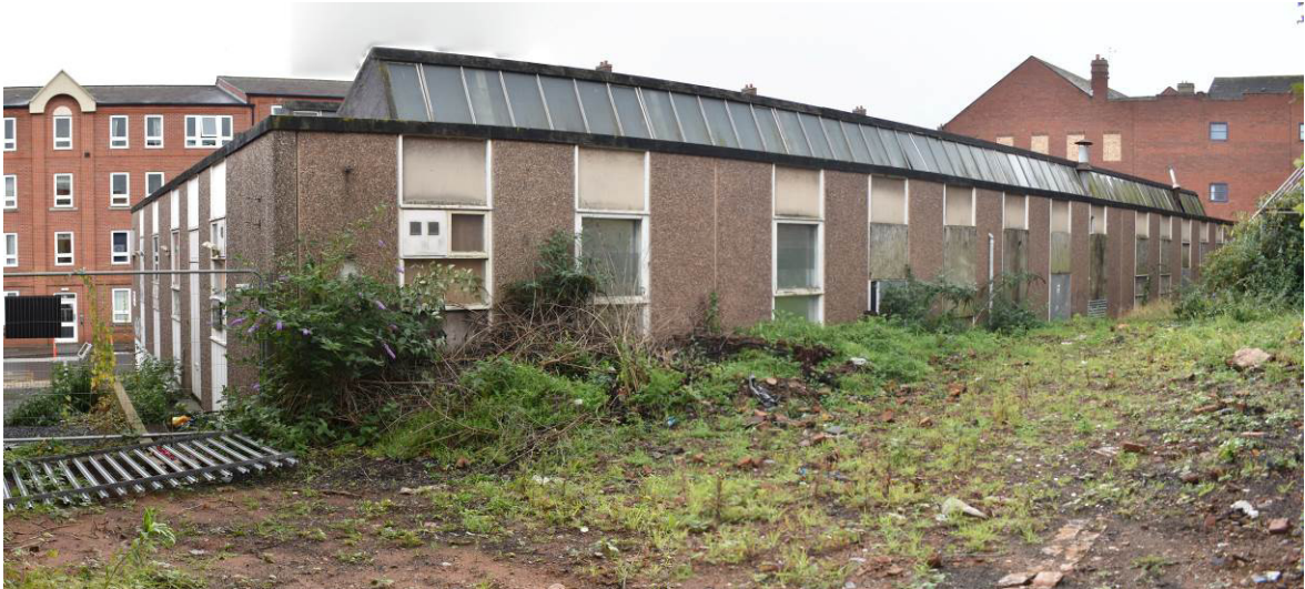
Plate 334: Building 14; rear elevation looking south-west.
