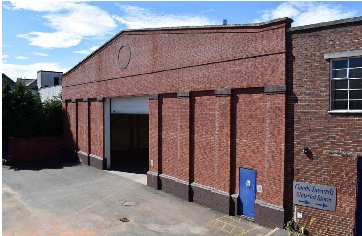
Plate 124: Building 9; south elevation to Northwood Street looking north-west, seen from 1F level of Bldg. 13.
