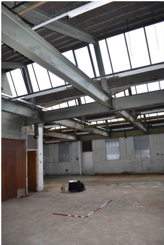
Plate 339: Bldg. 14, room [G3] looking north-west.
