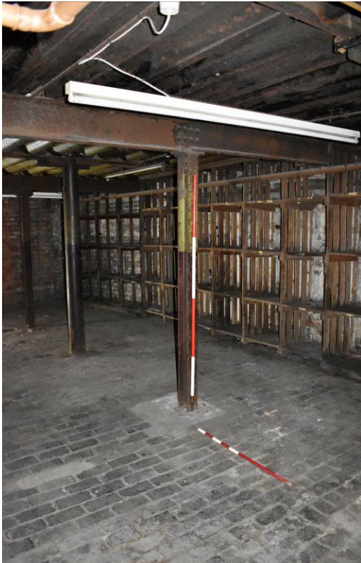
Plate 236: Bldg. 12a: basement level [B1] looking SW.
