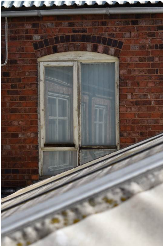
Plate 267: Bldg. 13a; original 1F door at Bay 3.
