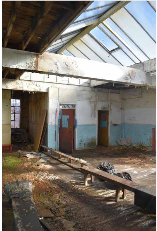
Plate 36: Building 5; 1F level looking north with pitched roof-light over.
