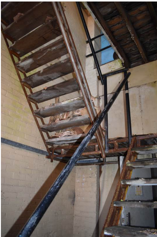
Plate 30: Building 5; secondary stair B.
