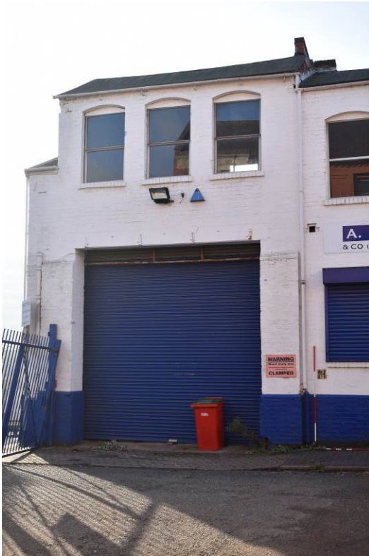
Plate 189: Building 11a: north elevation entry at Bay 1.
