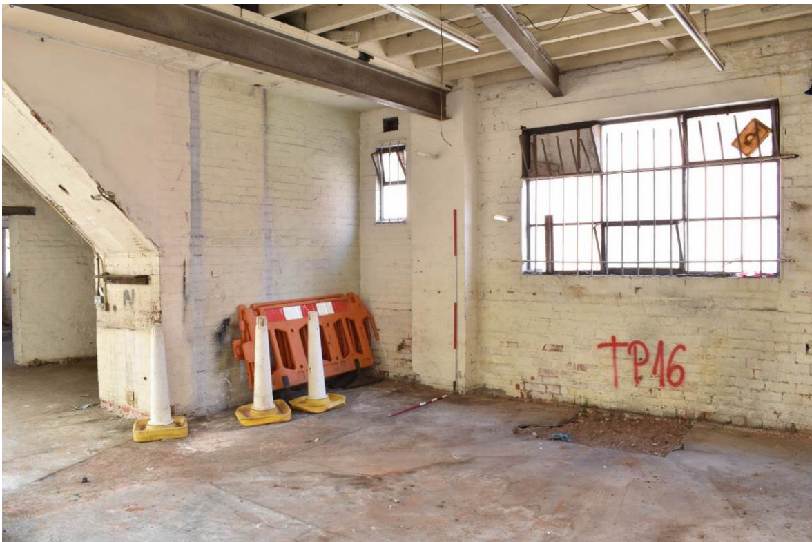
Plate 162: Building 10b; Room [LG2] looking north.
