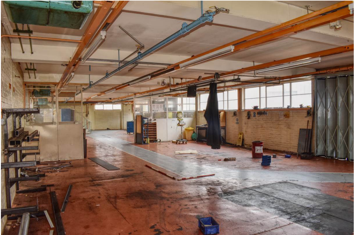
Plate 358: Building 15a; first floor looking west.
