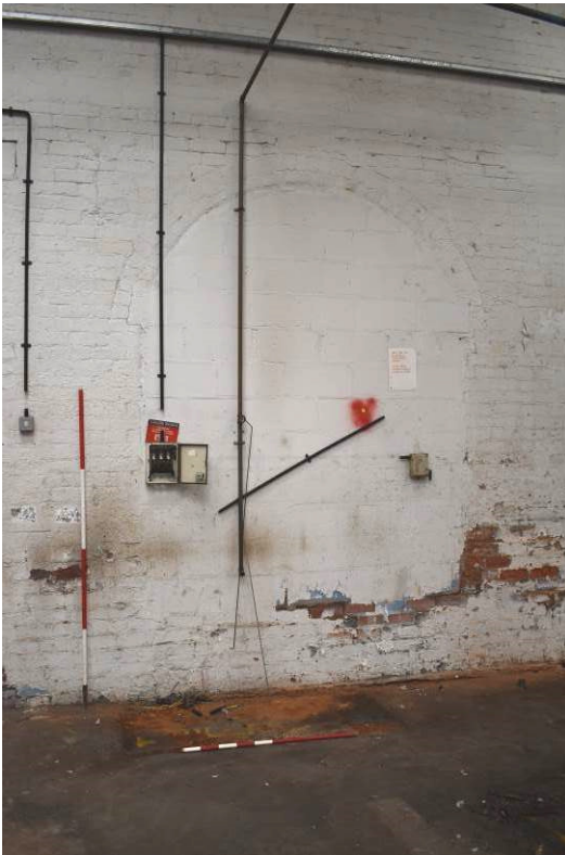
Plate 17: Blocked, arched opening to north wall.
