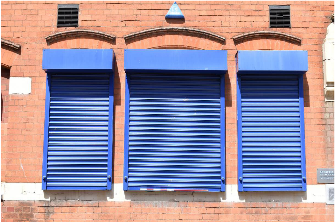
Plate 46: Building 6a; south elevation to Northwood St. – window details.
