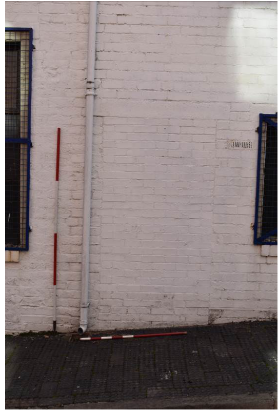
Plate 134: Building 10a; blocked door to south (see Plate 147).
