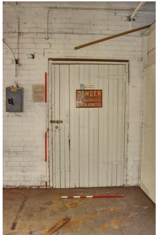
Plate 71: Door to sub-station [G3].
