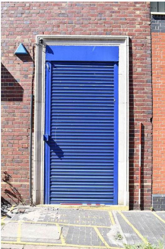
Plate 59: Building 7a; primary doorway [d1] at Bay 1.
