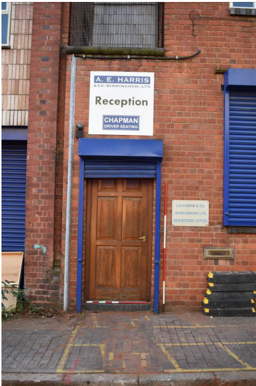
Plate 256: Bldg. 13a, pedestrian door, possibly inserted.
