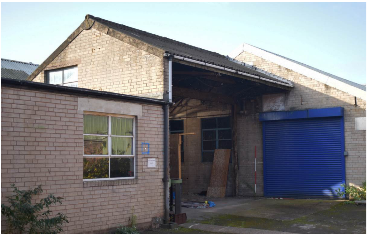
Plate 225: Covered yard 11f adjacent to Bldg. 11c; general view looking south-west.
