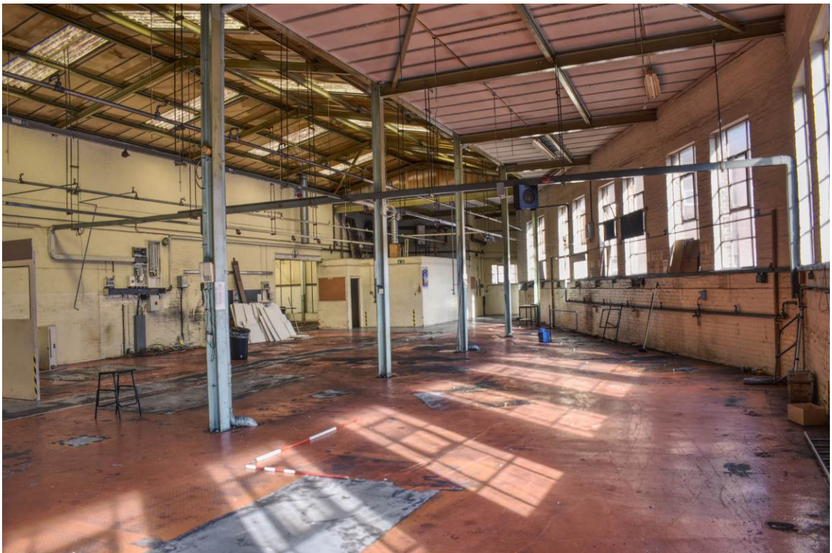
Plate 368: Building 15b; first-floor floor looking east.
