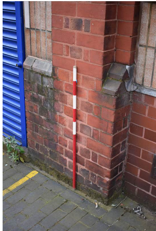
Plate 231: Building 12a; relic chamfered brick plinth
