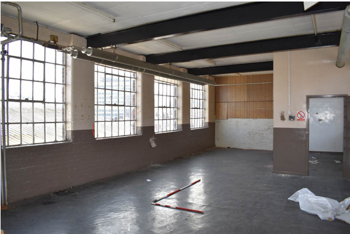
Plate 281: Bldg. 13a; canteen [F20] at Bays 5/7 looking south.
