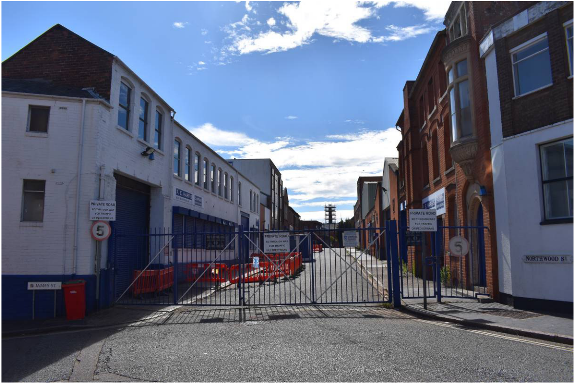
Plate 3: Northwood Street looking west from junction with James Street.
