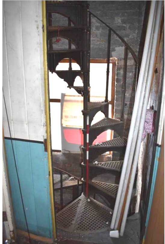
Plate 137: Spiral stair A rising from [B1].
