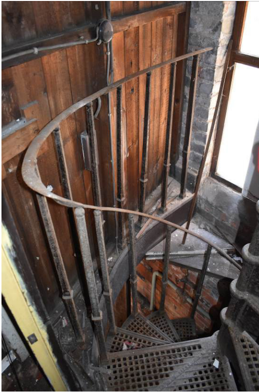
Plate 152: Head of Stair A at [UF1].
