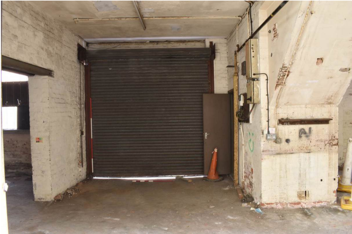
Plate 163: Building 10b; Room [LG2]; roller door to James Street.
