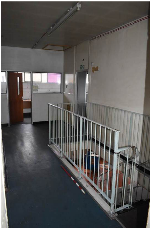
Plate 359: Building 15a; head of stair at 2F level [S1].
