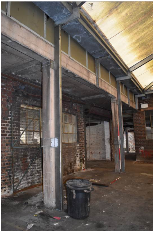
Plate 326: Concrete piers supporting raised link 13i to south side of yard 13j.
