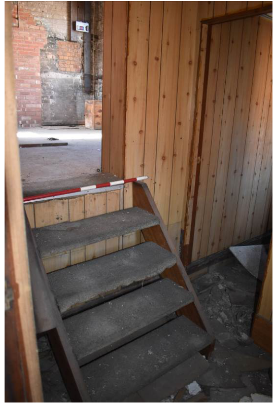
Plate 153: Door inserted in west wall of [UF2].
