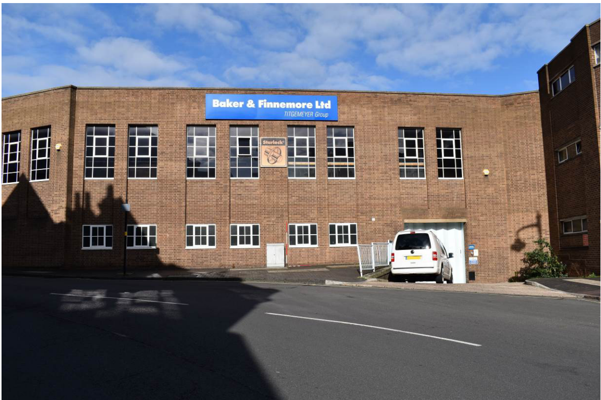
Plate 362: Building 15b; south elevation to Graham Street (east end).
