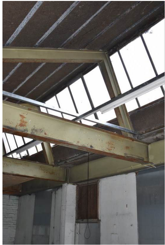
Plate 341: Detail of saw-tooth roof structure.
