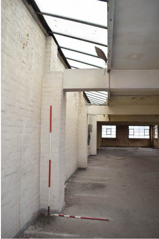
Plate 87: Lateral roof light to east side of [S2].
