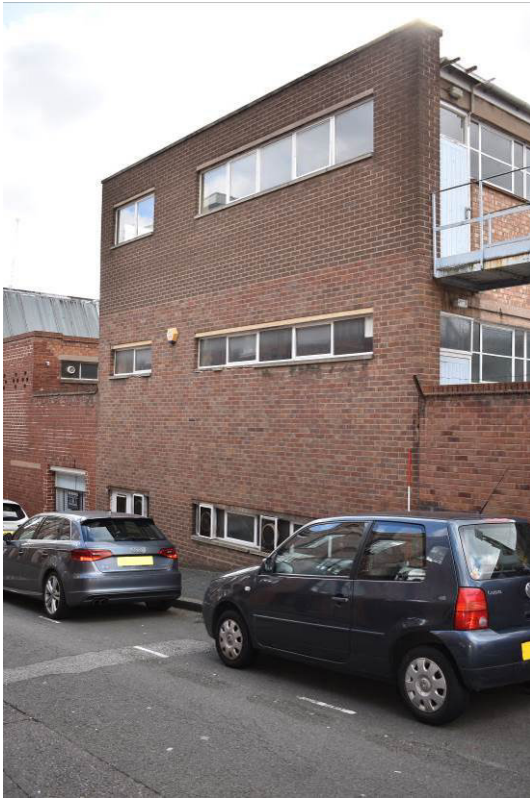
Plate 346: Building 15a; east elevation to James Street.
