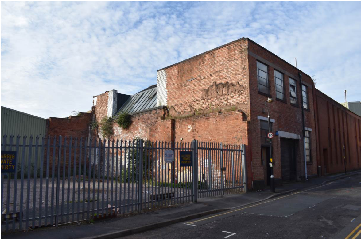
Plate 19: Building 5 in streetscape context looking south-west; vacant plot to foreground formerly Nos.41-45 Regent Place (demolished October 1999).
