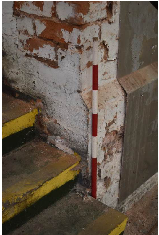
Plate 18: Detail of chamfered plinth to west wall (Bay 3).
