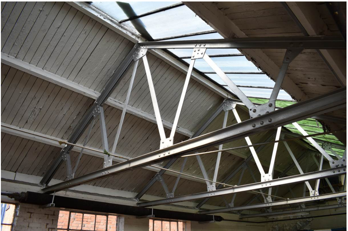
Plate 307: Detail of roof structure over shopping range 13d.
