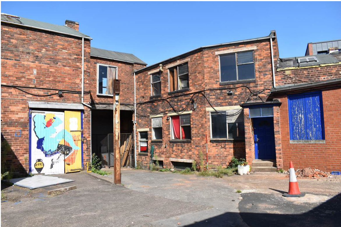
Plate 135: Building 10a; western elevation (centre) to yard of Bldg. 11.
