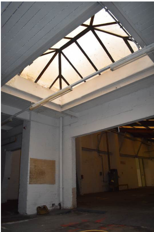
Plate 73: Pitched roof-light over rear of Bays 3/4.
