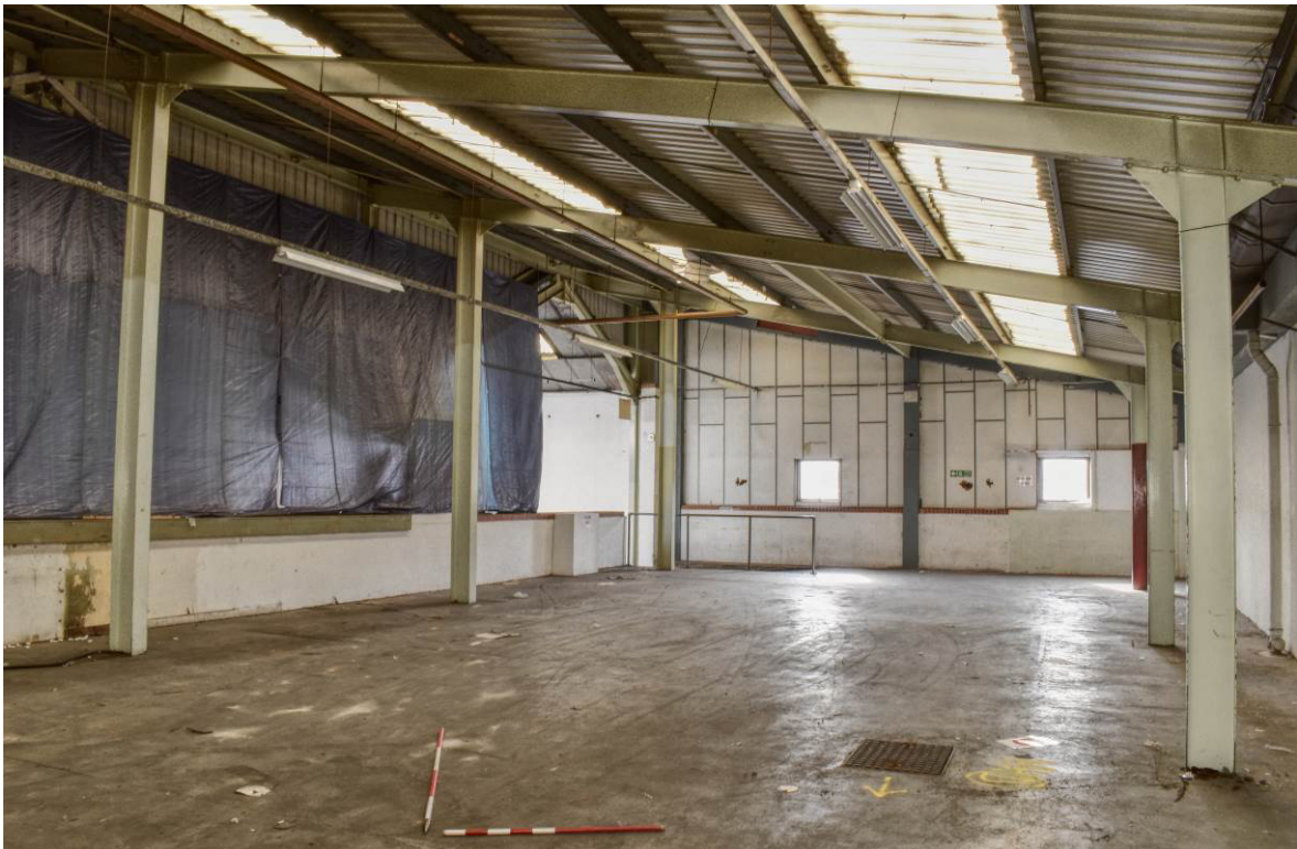
Plate 247: Building 12b; interior looking south.
