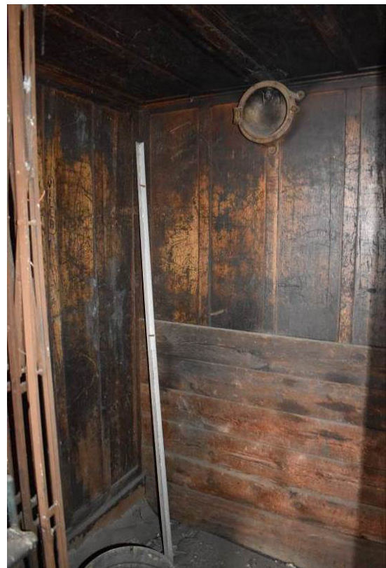
Plate 108: Timber-panel lined elevator car.
