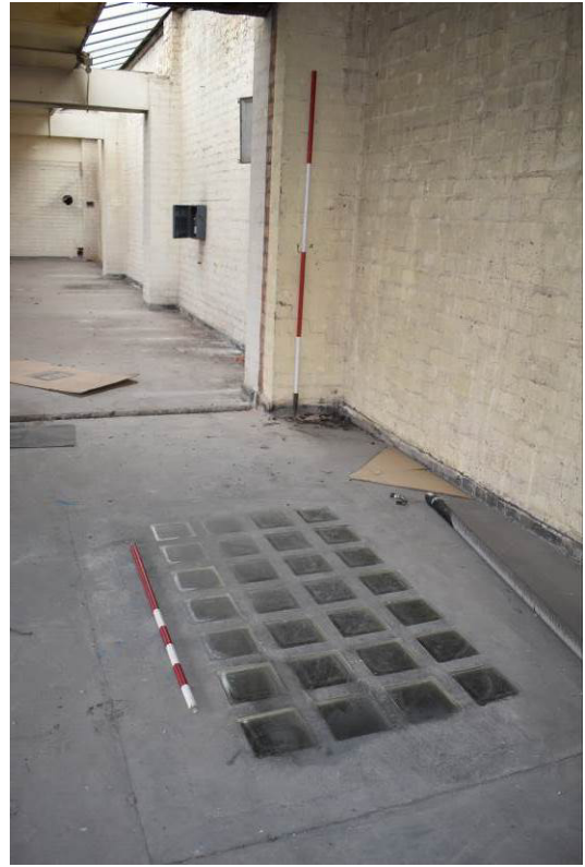
Plate 88: Glass-block panel in floor of [S2], formerly lighting stair A.
