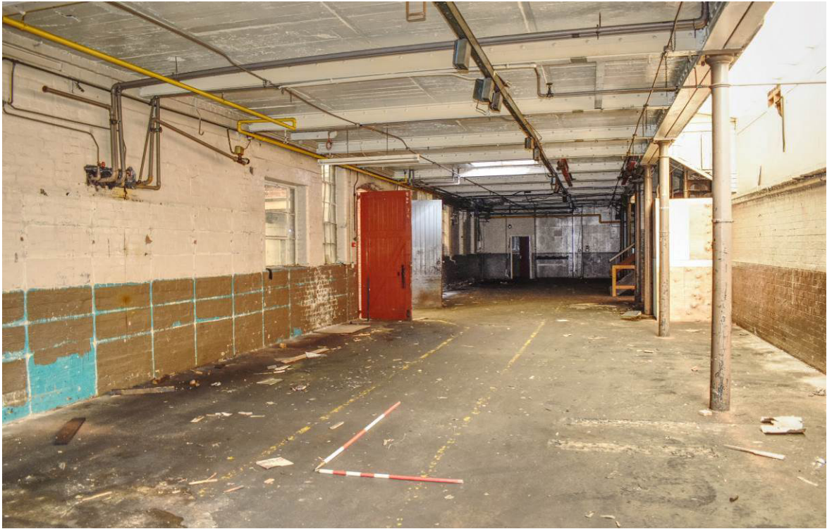
Plate 272: Building 13a, interior; ground floor [G2] looking north.
