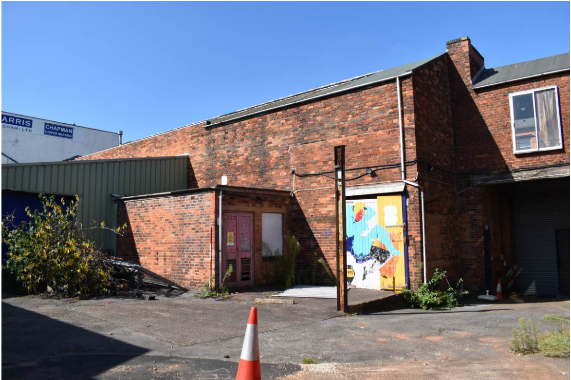
Plate 193: Building 11a; blind rear (south) elevation to yard (with Bldgs. 11d and 11e to foreground left and centre).
