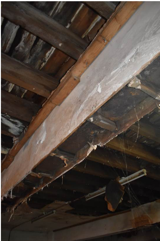
Plate 33: Building 5; first floor structure
