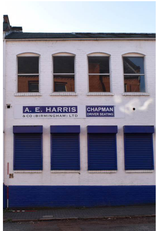
Plate 190: Building 11a: north elevation representative detail of fenestration (Bays 2/3).
