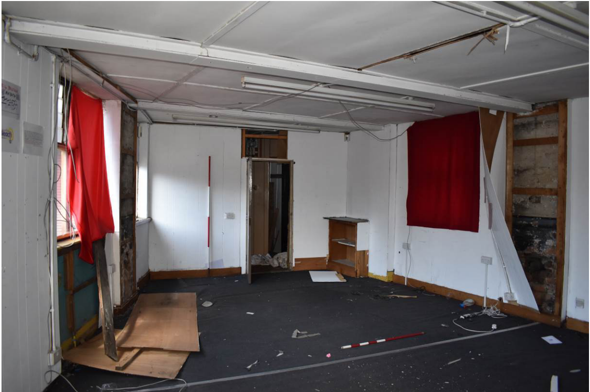
Plate 149: Room [UG1] looking north.
