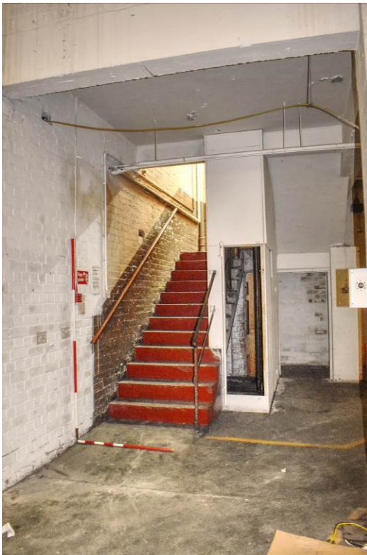
Plate 75: Stair B rising at Bay 6 Plate to 1F level.
