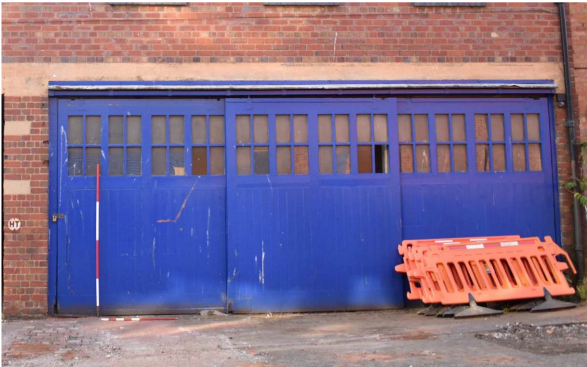
Plate 260: Bldg. 13c, sliding doors to three-bay vehicular garage.
