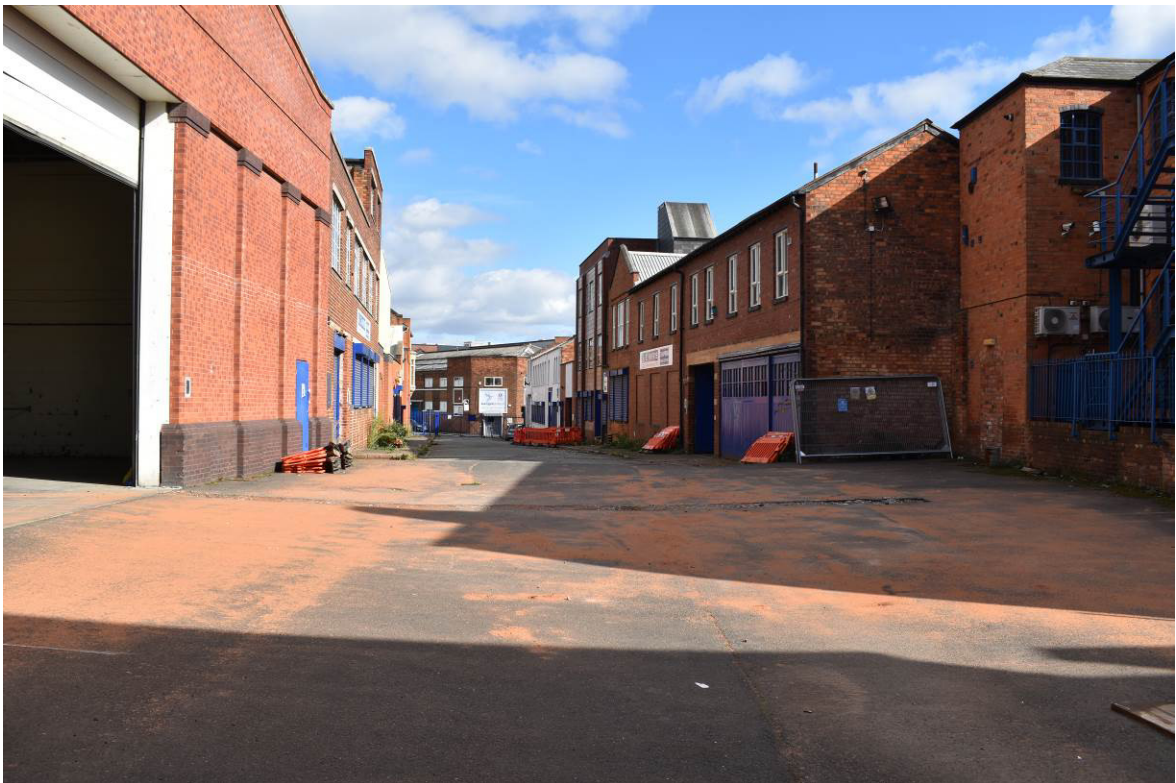
Plate 4: Northwood Street looking east (from Bldg. 9).
