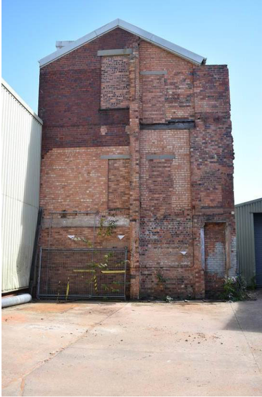
Plate 97: Building 7b; north gable end.
