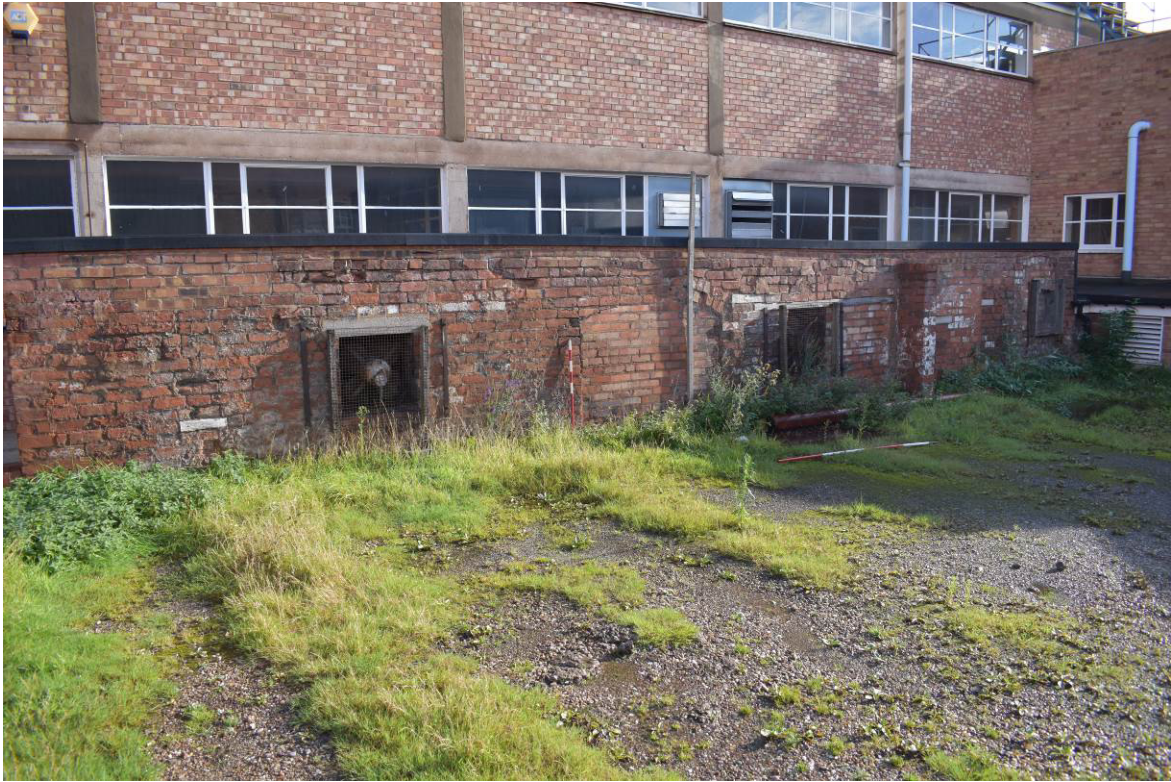
Plate 354: Building 15a; relic wall enclosing north side of raised office/plant room.
