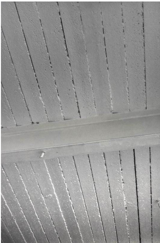
Plate 70: Concrete beam ceiling over [G2].
