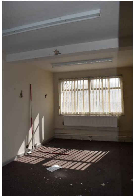
Plate 289: Building 13b: Office [F12] looking south.
