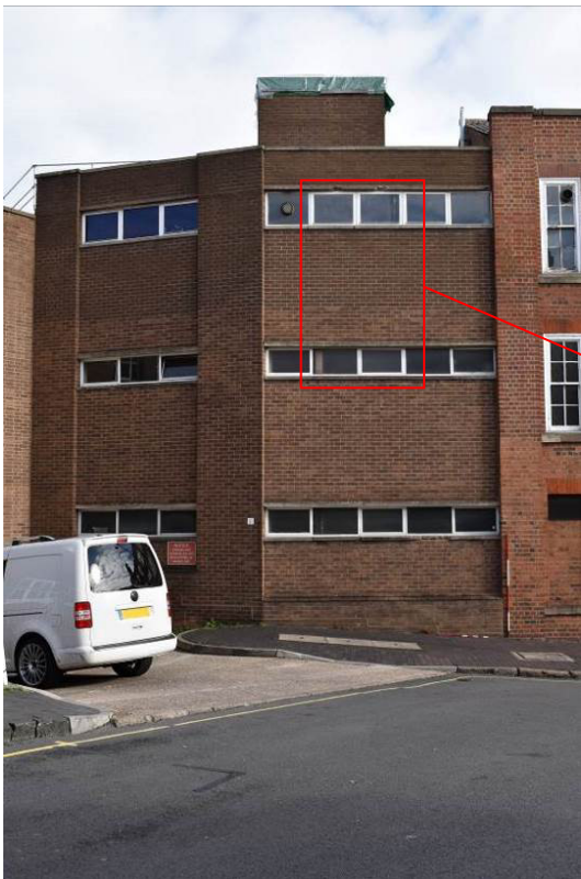
Plate 348: Building 15a; west elevation to Newhall St.
