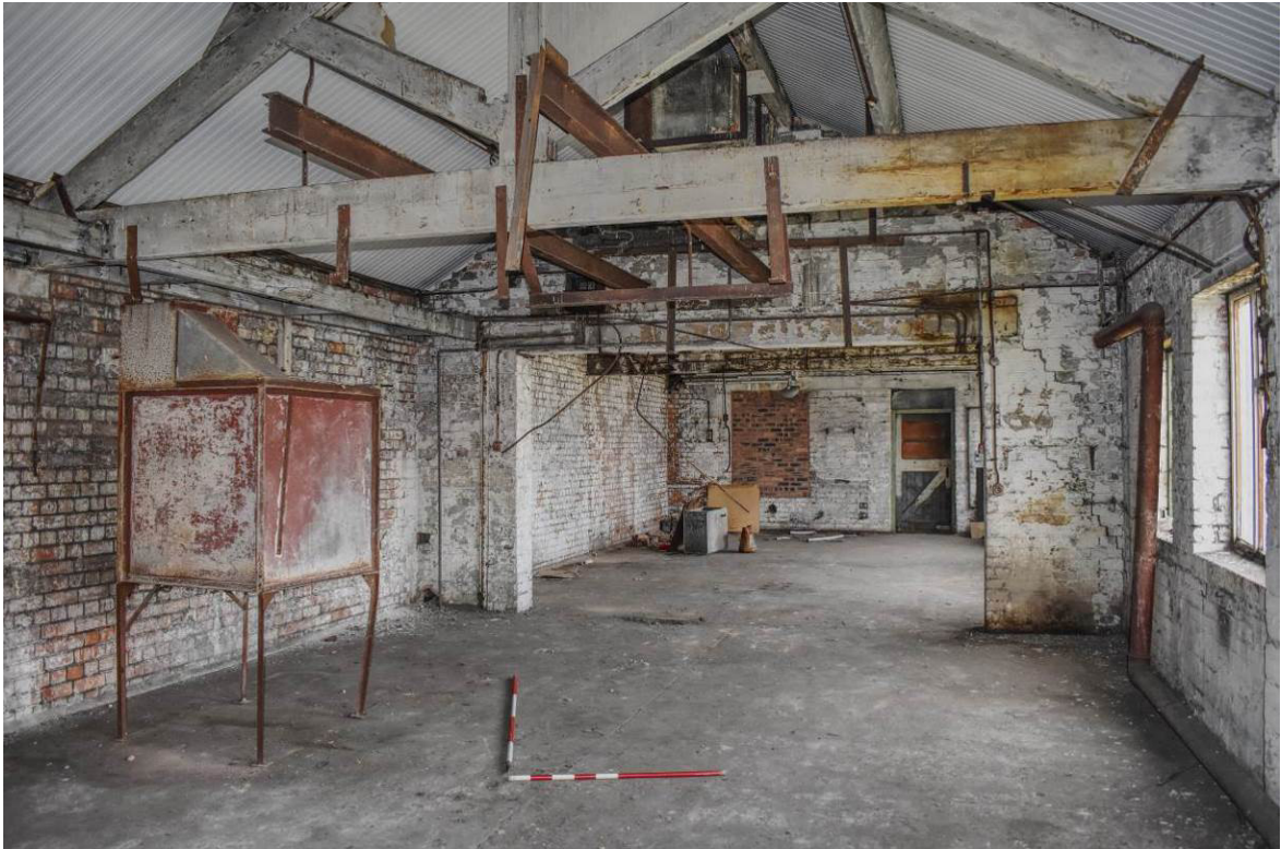
Plate 114: Building 7b; 2F looking south from Bay 9 towards Bays 7/8.
