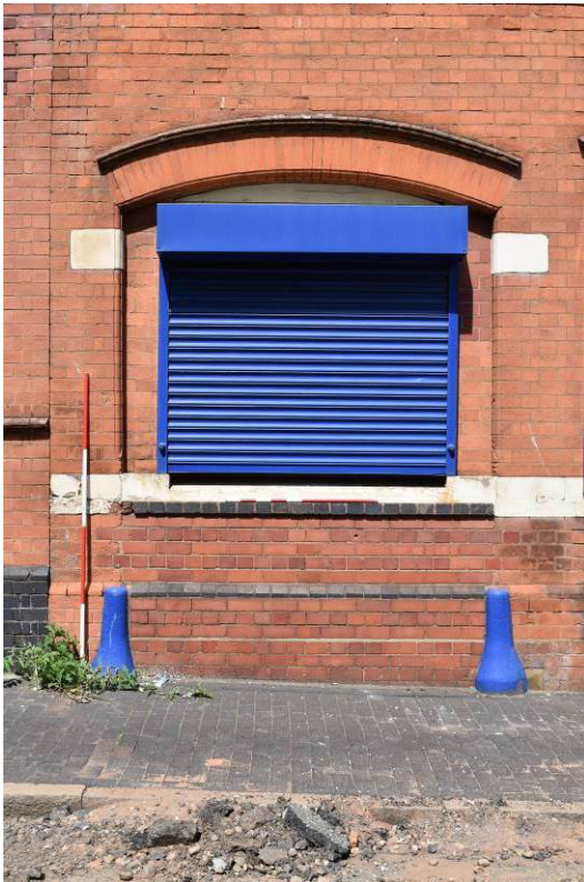
Plate 47: Building 6a; south elevation to Northwood St. blocked cart entry.
