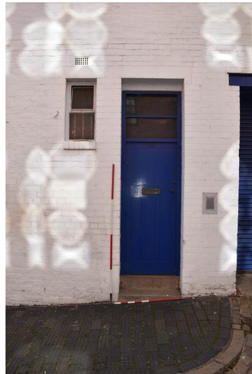
Plate 157: Doorway at Bay 3 from N.
