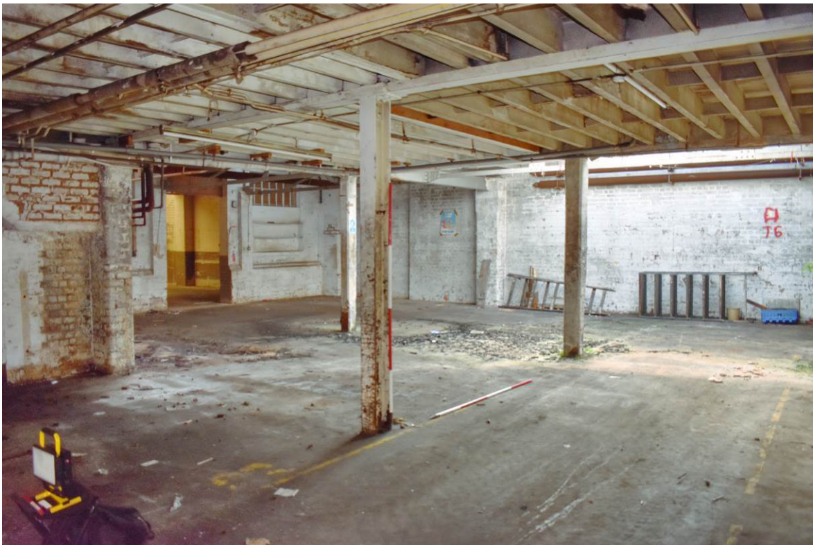
Plate 314: Building 13e; looking south-east at ground floor level, open to covered yards 13f/g.
