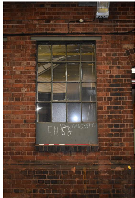
Plate 266: Bldg. 13a; window detail to west elevation.
