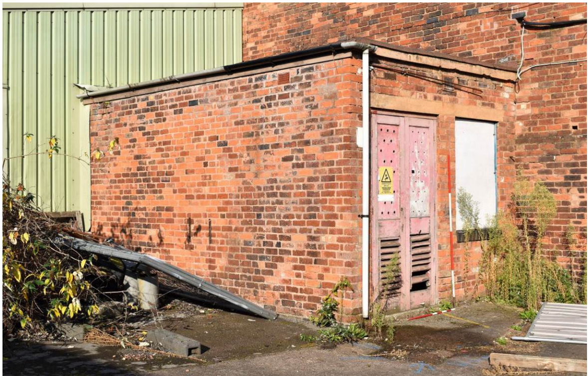
Plate 222: Building 11e (sub-station); general, oblique view looking north-west.
