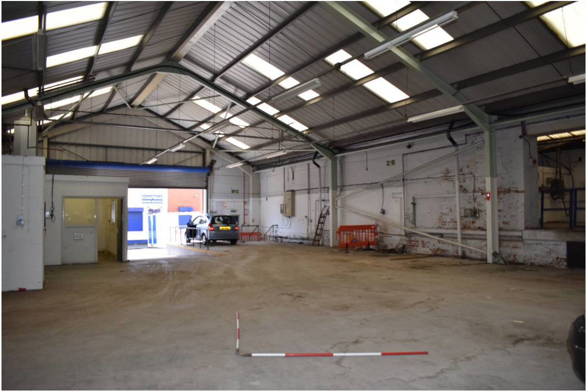
Plate 12: Building 4 (113 Northwood Street); interior looking south, portal-framed Bays 1-3.
