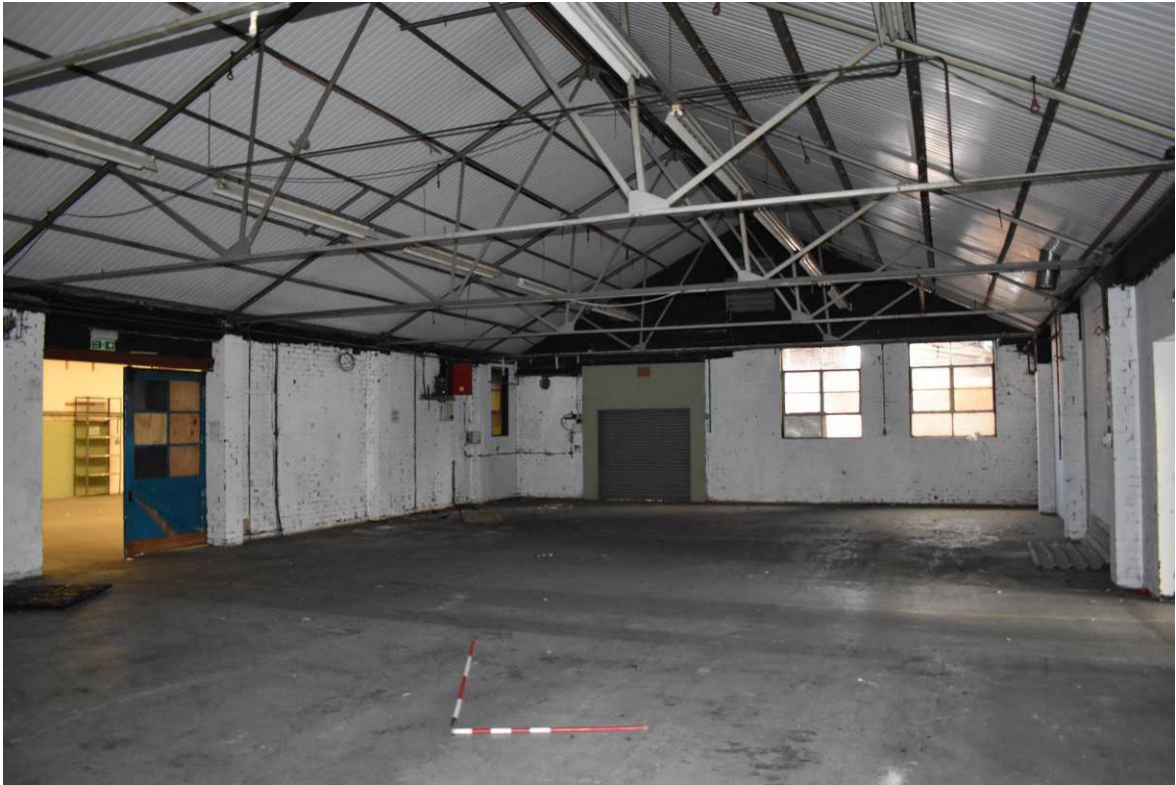
Plate 215: Building 11c: interior looking east, doorway to left opens onto range 11d.
