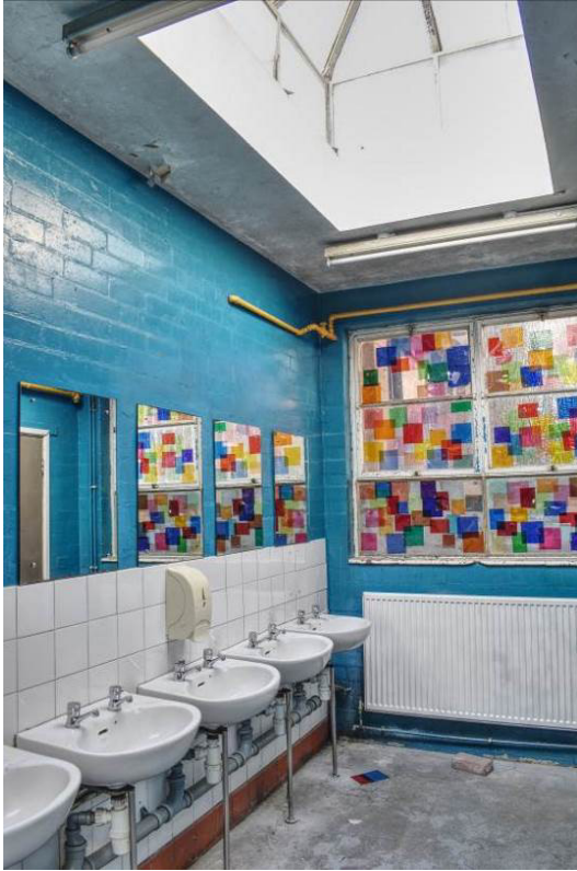
Plate 228: Building 11g; interior of wash-room with pitched, glazed ceiling-light.
