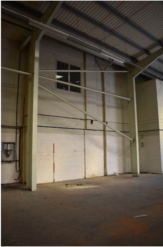
Plate 128: Building 9 looking south-east, relic features of former shopping range assoc. Bldg. 7.
