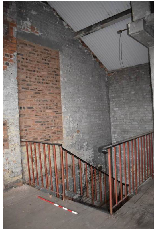
Plate 113: Building 7b, 2F; head of Stair C at Bay 14.
