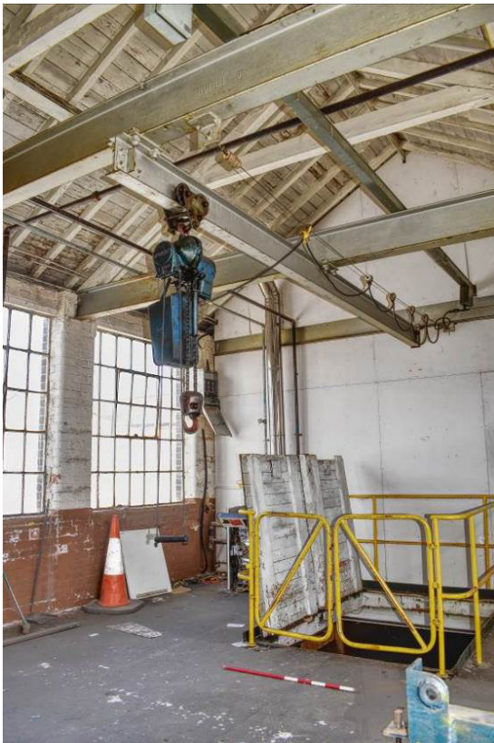
Plate 284: Bldg. 13a; 1F hoist at Bay 4 [F19].
