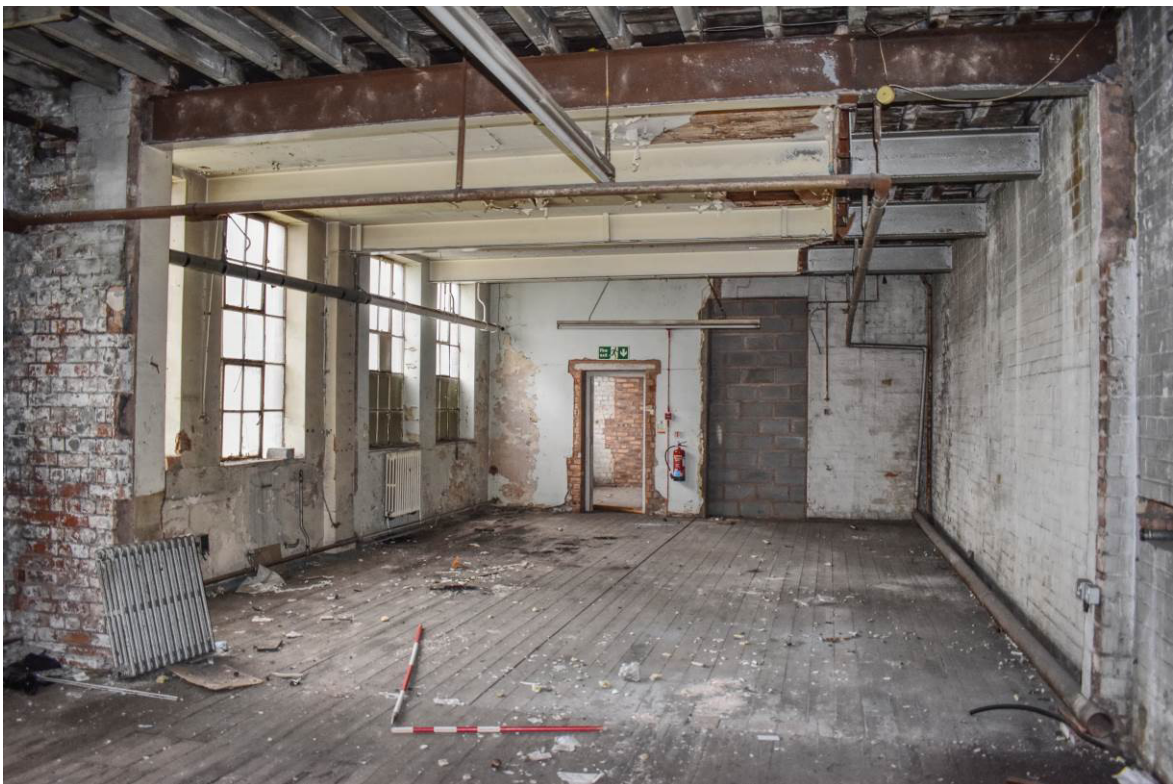
Plate 110: Building 7b; first floor looking north from Bay 11.
