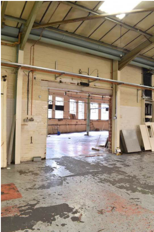
Plate 374: Building 15c: opening onto 15b.
