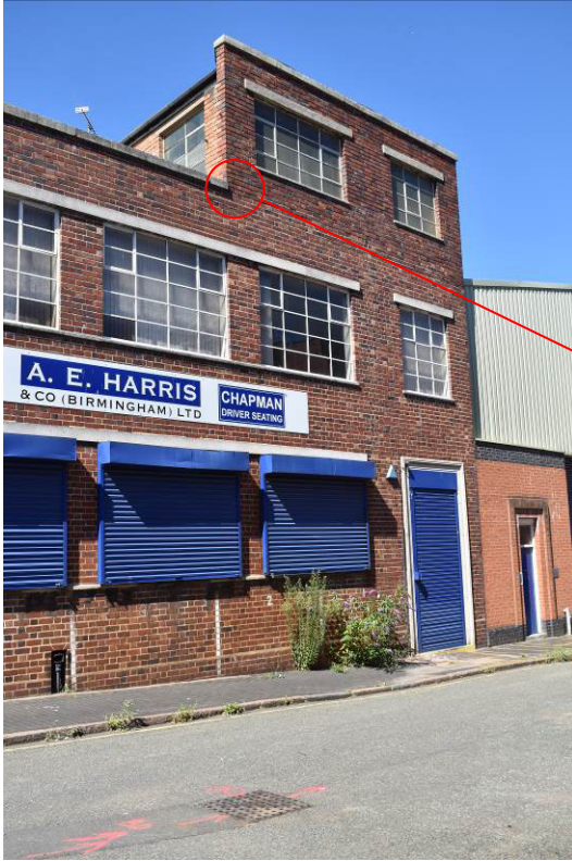
Plate 55: Raised elevation at Bays 1/2.
