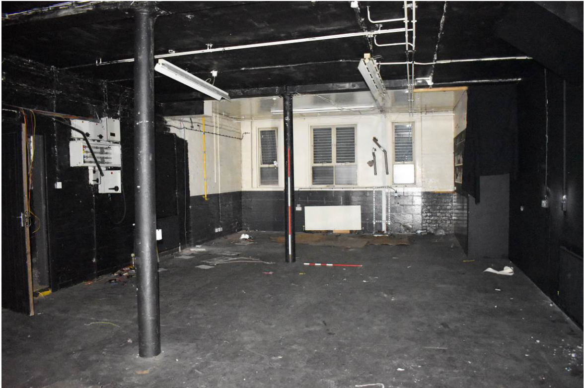
Plate 240: Bldg. 12a: ground floor [G2] looking north.
