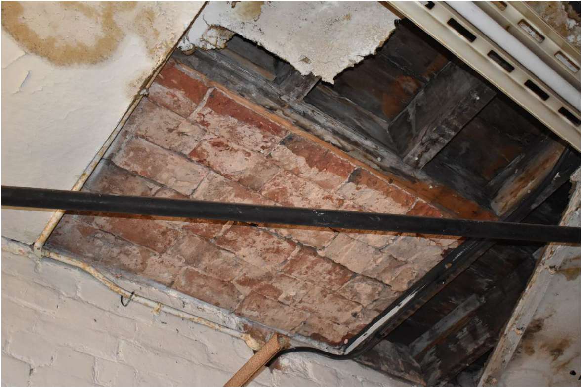
Plate 173: Trimmed, brick hearth slab exposed in ceiling of [LG1].
