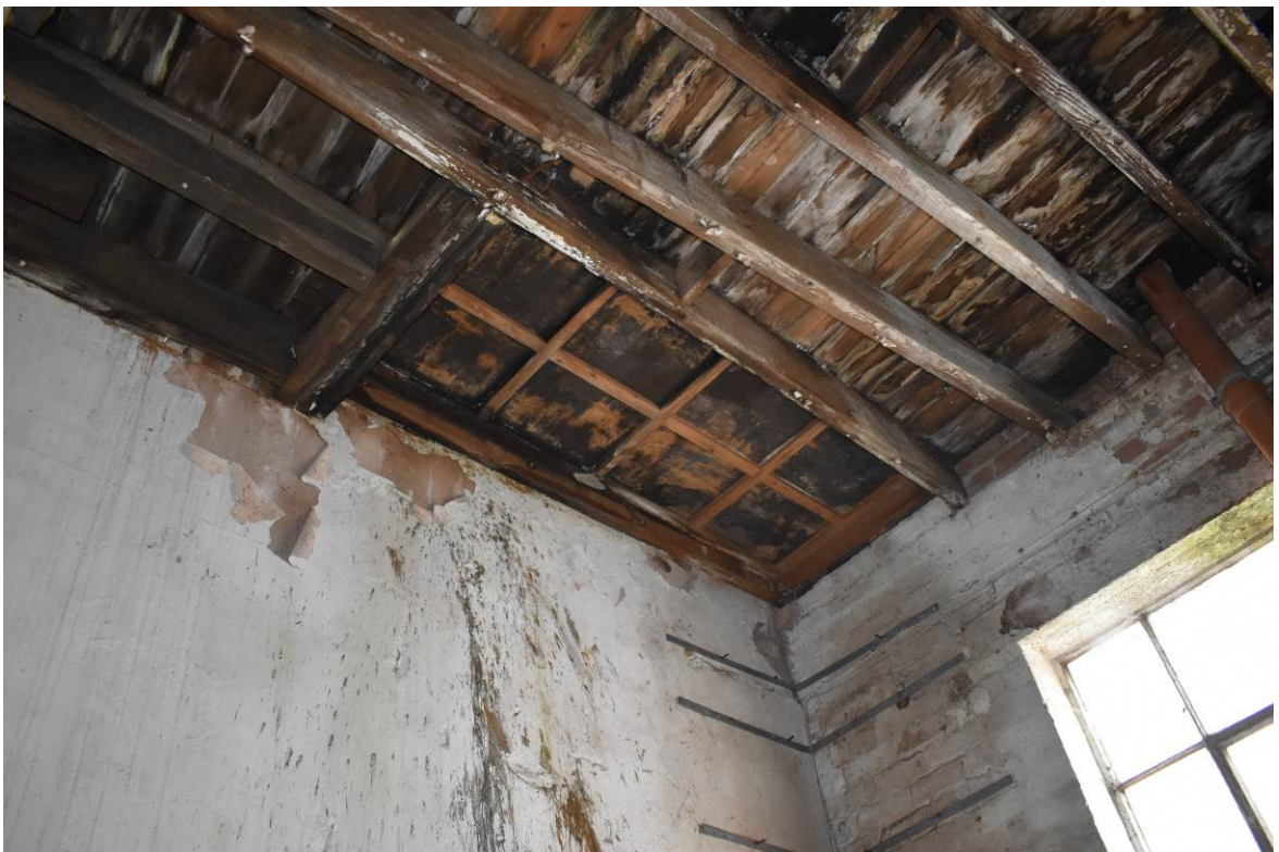
Plate 40: Building 5; infilled hoist void as visible at GF level.
