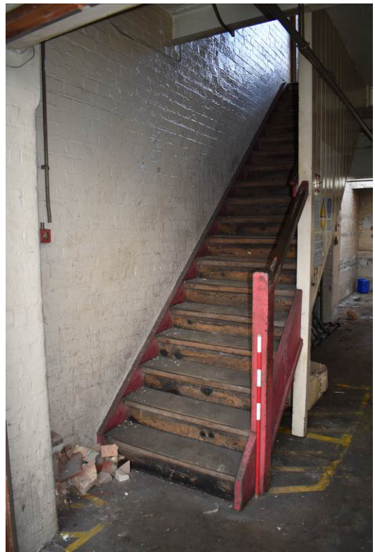
Plate 303: Building 13d: stair E rising at Bay 7.
