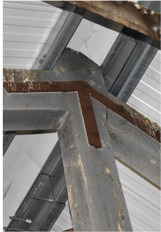
Plate 117: Strapped apex.
