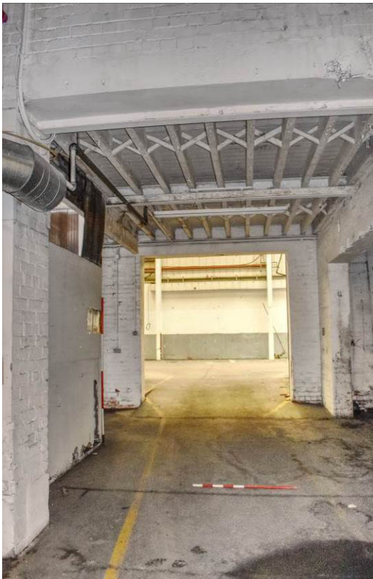
Plate 103: Building 7b; transverse access at Bay 12.
