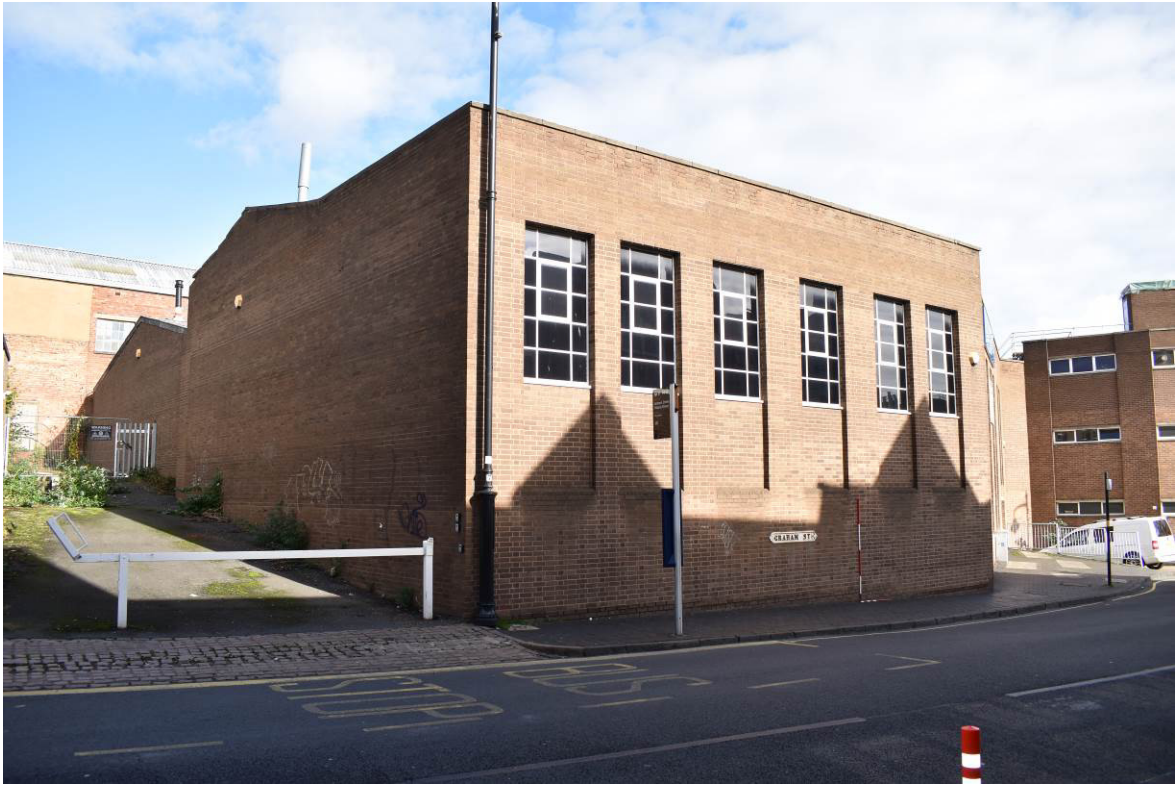
Plate 363: Building 15b; south elevation to Graham Street (west end) and blind, north-western façade (left).
