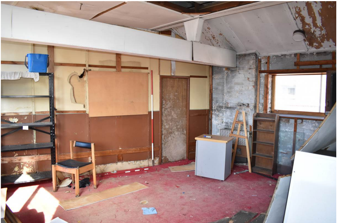
Plate 154: Room [UF1] looking north-east.
