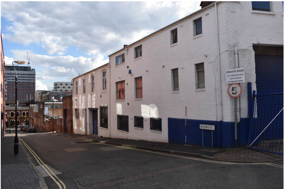
Plate 130: Building 10; east elevation, looking south down James Street (10a to right; 10b to centre; 10d to left).
