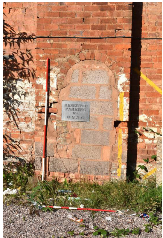
Plate 26: Blocked archway in projecting chimneybreast.
