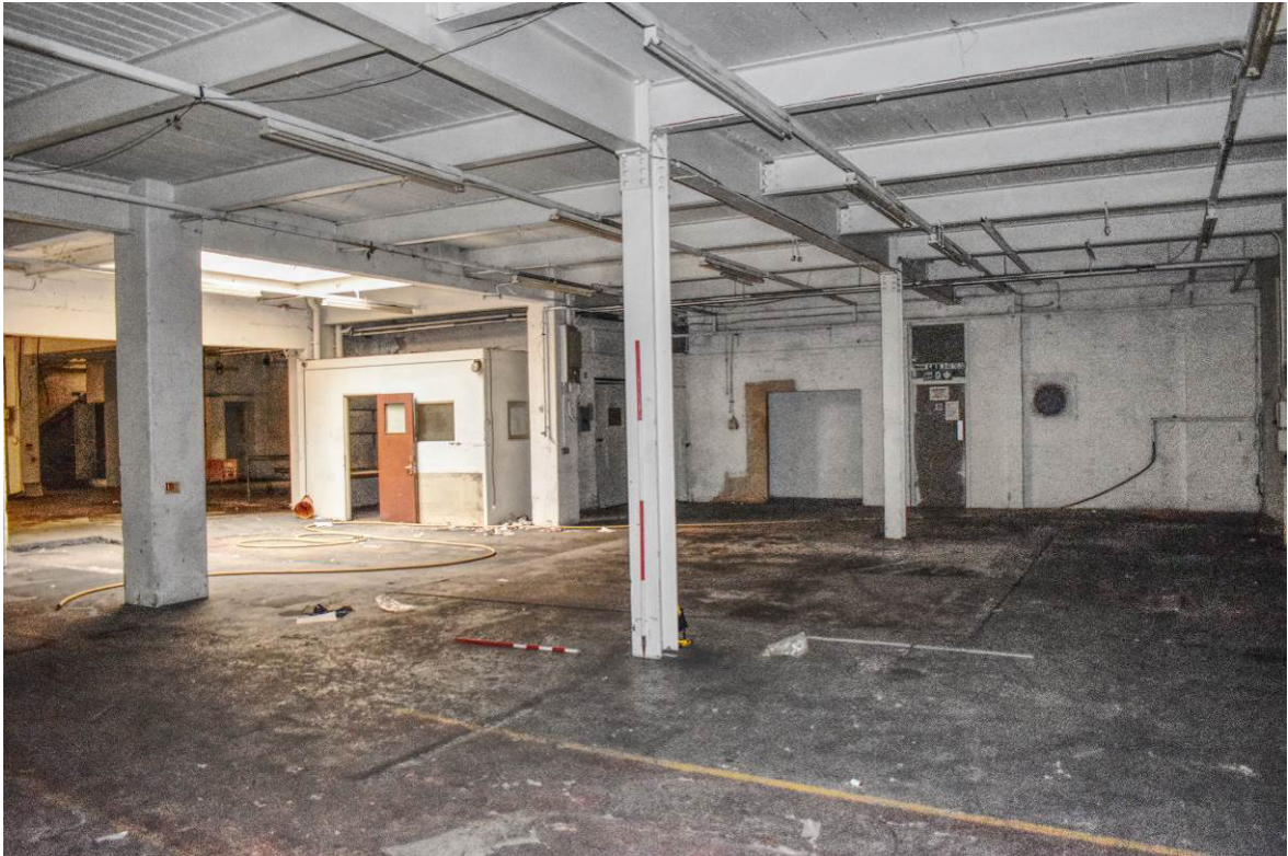
Plate 69: Ground floor interior of street frontage range 7a, [G2] looking north-east.
