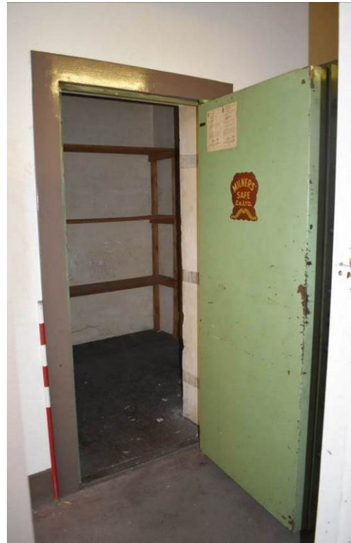
Plate 83: Steel door to strong room [F8].
