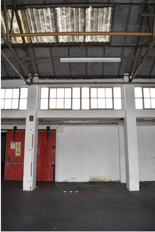
Plate 212: Bldg. 11b: modified north wall with upper clerestory lighting.
