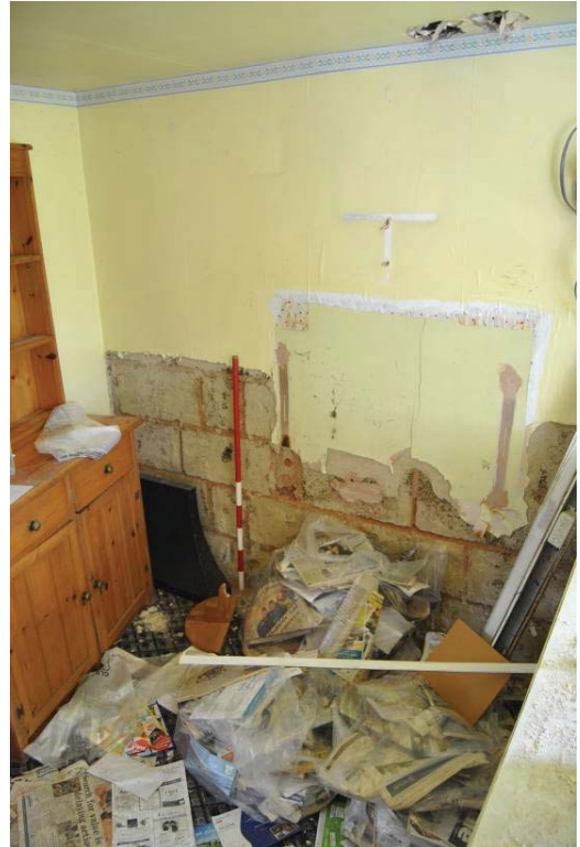
Plate 19: Kitchen [G.02]; note blockwork infill of FP.
