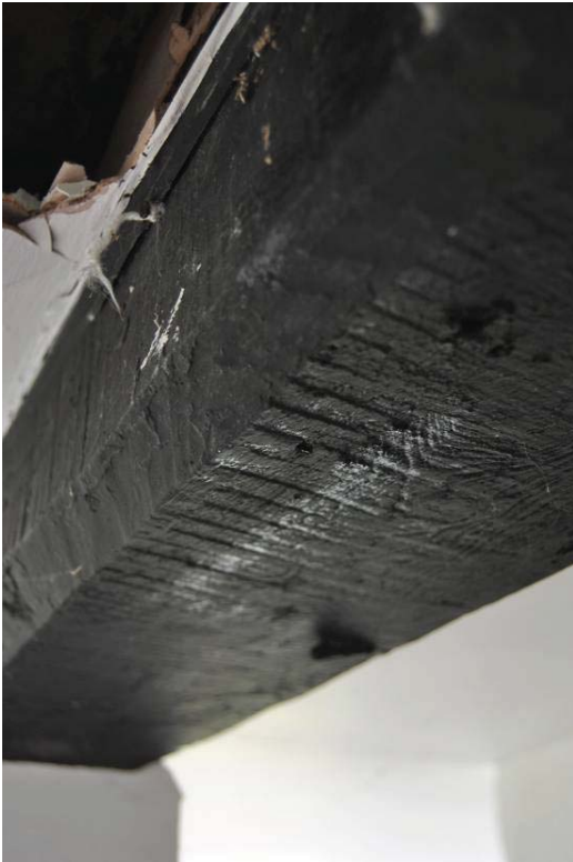
Plate 35: Marks of machine sawing to soffit of transverse beam.
