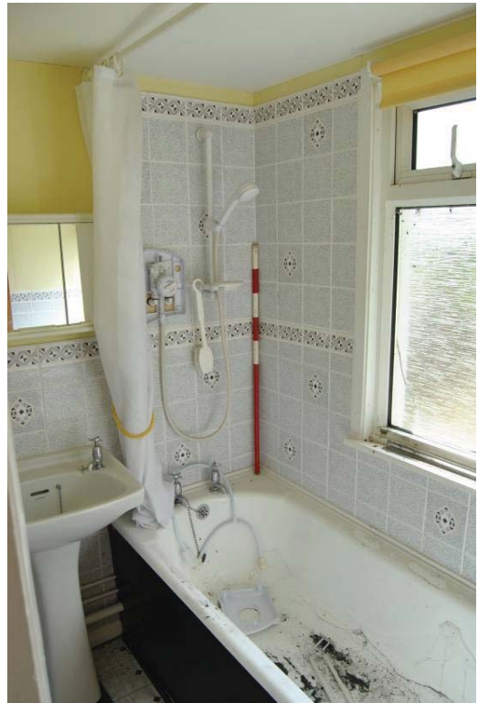
Plate 28: Bathroom [F.04] within flat-roofed extension.
