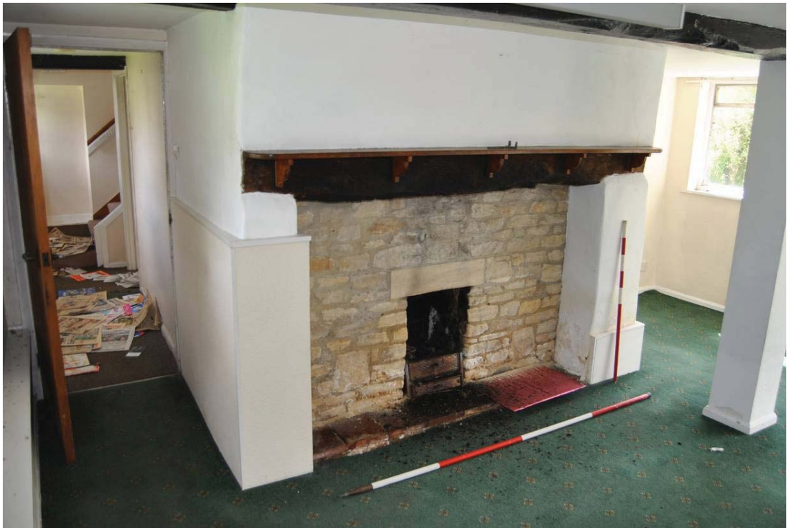
Plate 31: Fireplace dominating living room [G.06].
