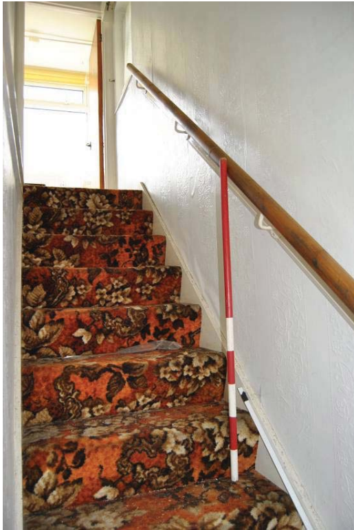
Plate 22: Stair A from [G.01] to [F.01].
