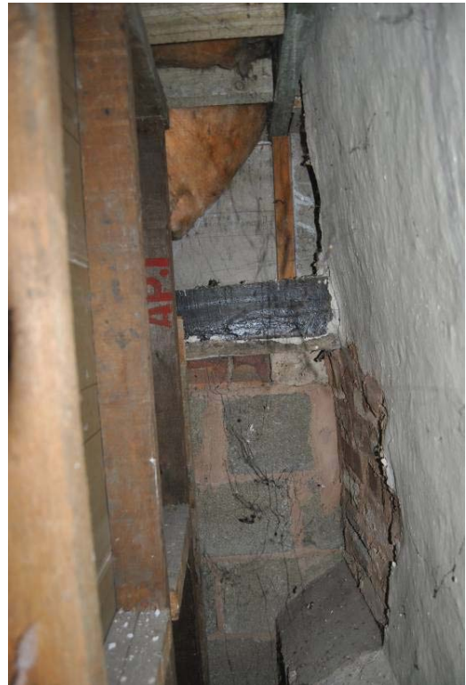
Plate 44: Tie of truss T3 embedded into masonry of eastern stack.
