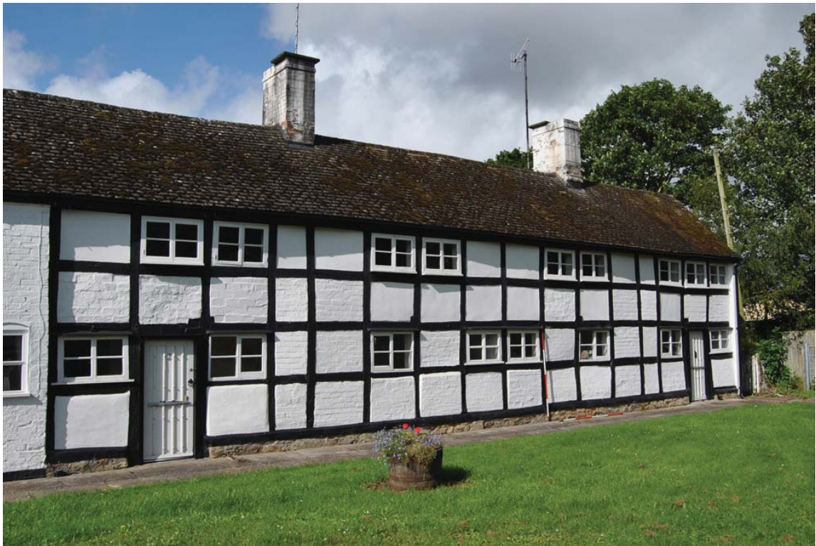
Plate 2: Nos. 1 and 2 Black and White Cottages, north elevation.
