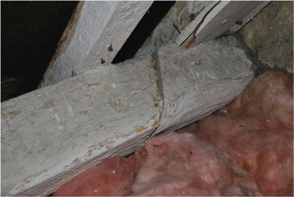
Plate 51: Detail of splayed purlin scarf.
