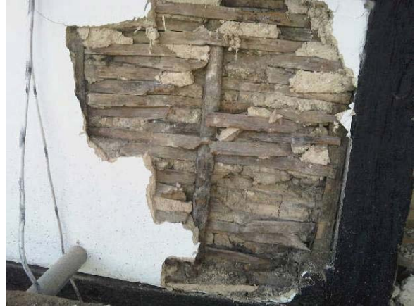
Plate 4: Wattle and daub infill exposed during building works (Photo: Russell Sumner)
