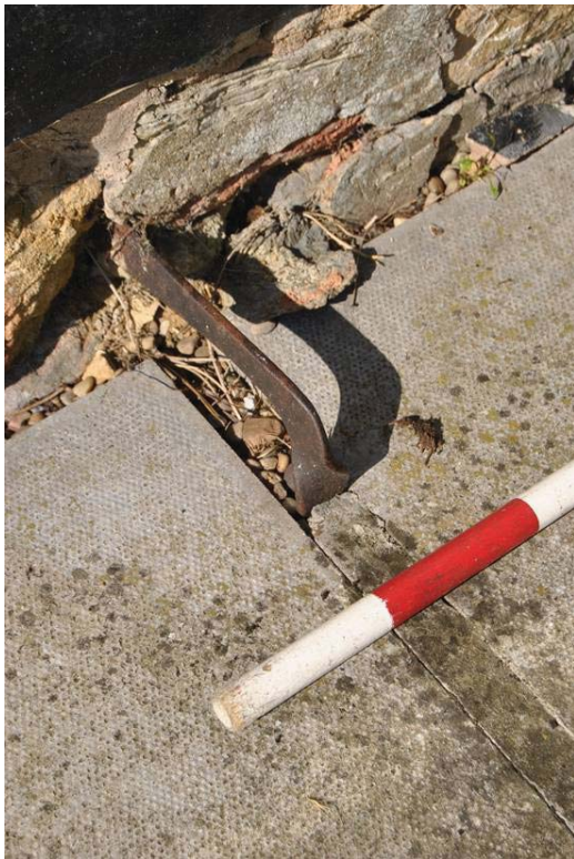
Plate 6: Iron boot-scraper adjacent to blocked door.
