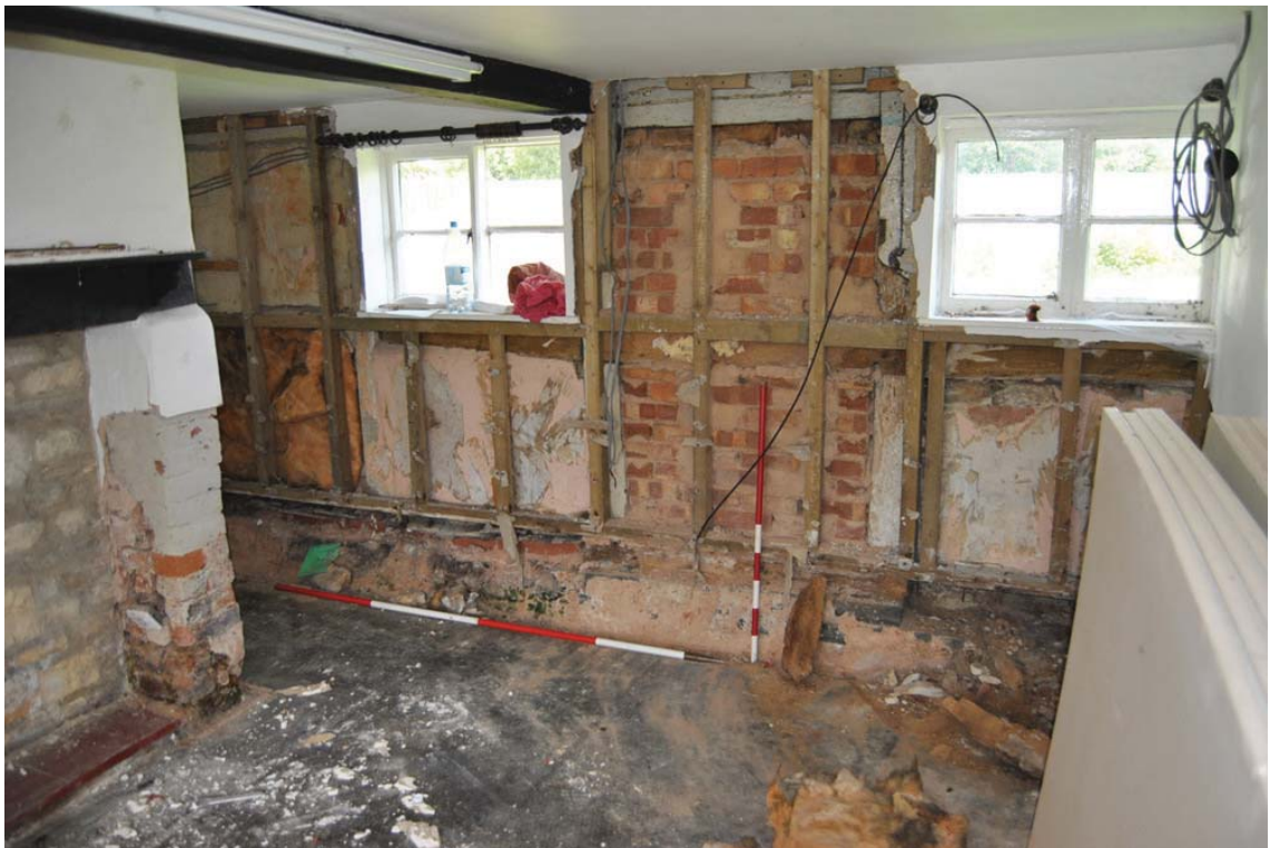
Plate 13: Timber-framed front elevation with studwork lining; NB: blocked door behind vertical scale (see Plate 13).
