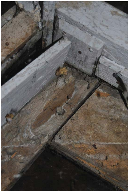
Plate 50: Double-pegged principals at apex.
