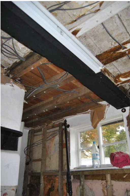
Plate 20: Renewed ceiling to N of stack [G.03]: location of primary stair.
