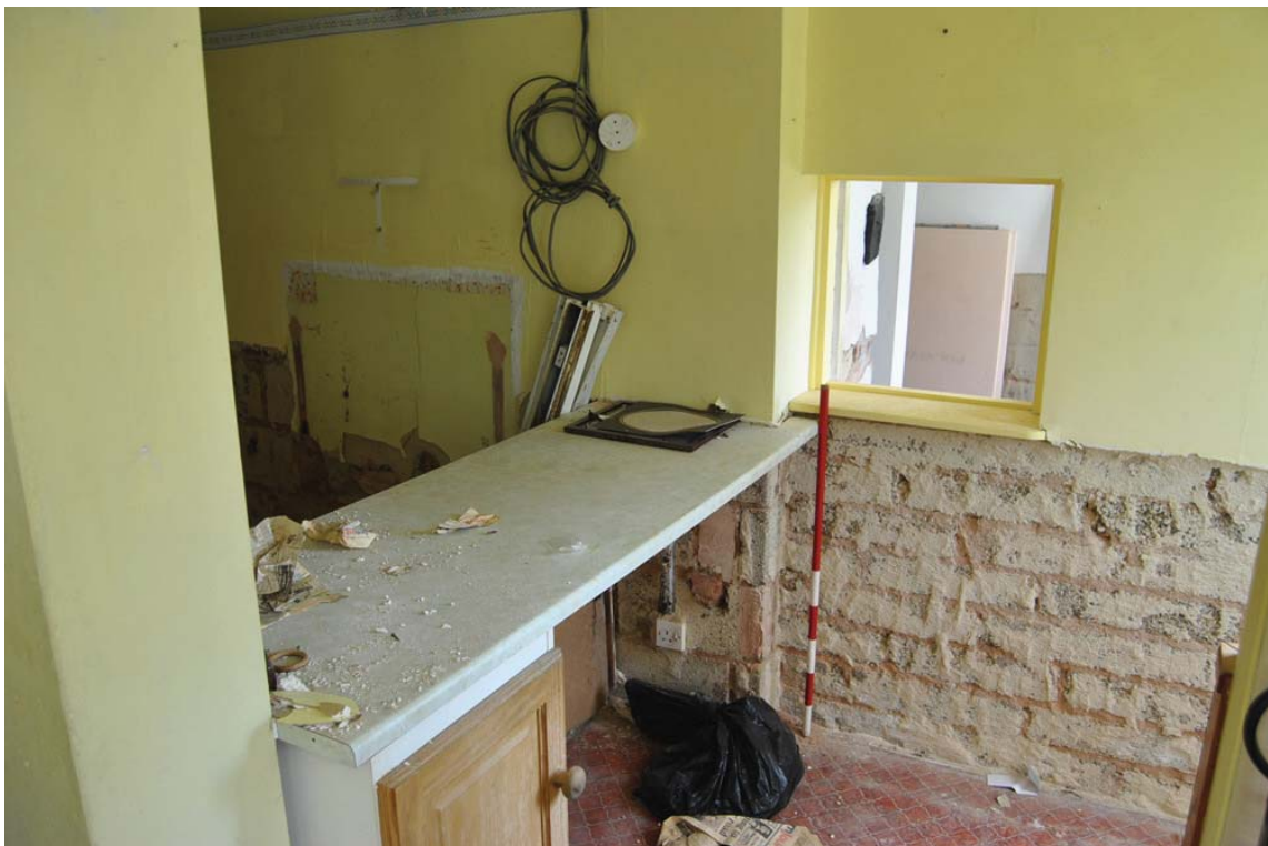
Plate 17: Kitchen [G.02] looking north-east, note blockwork partition.
