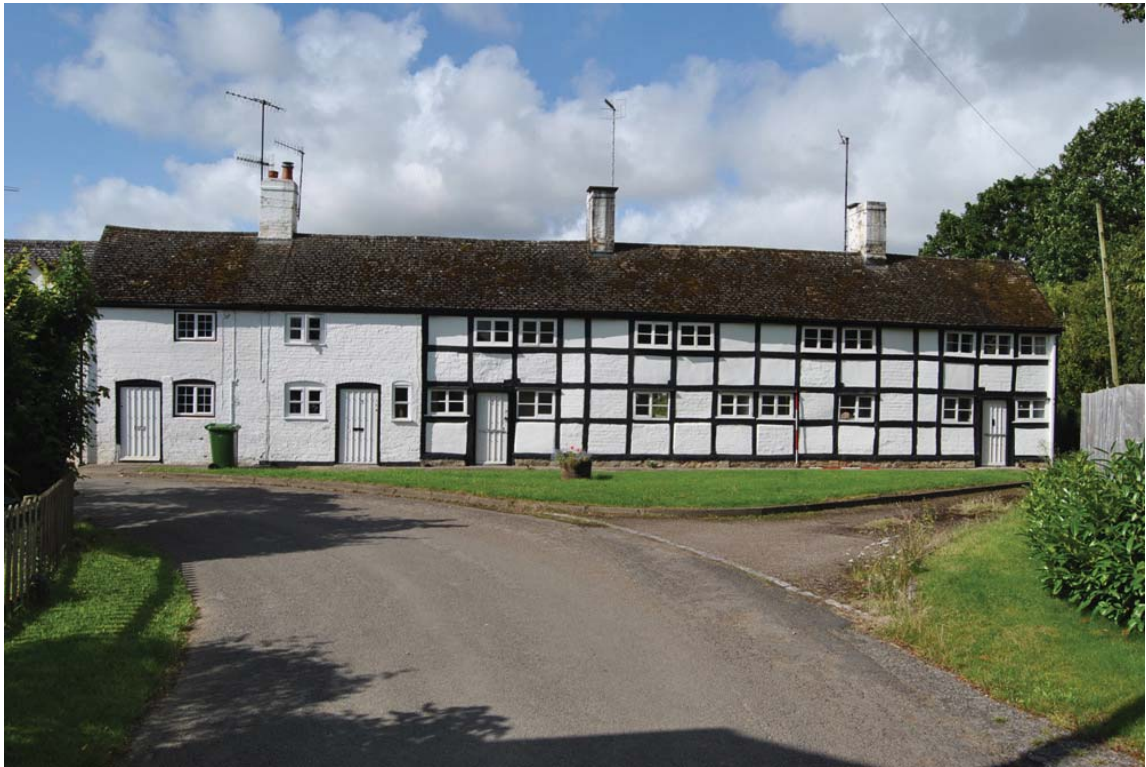
Plate 1: General view of Black and White Cottages from the north, Nos. 1 & 2 being framed units to right.
