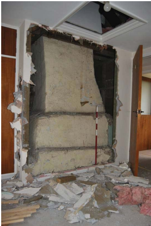
Plate 43: Stack revealed behind modern partition [F.10].
