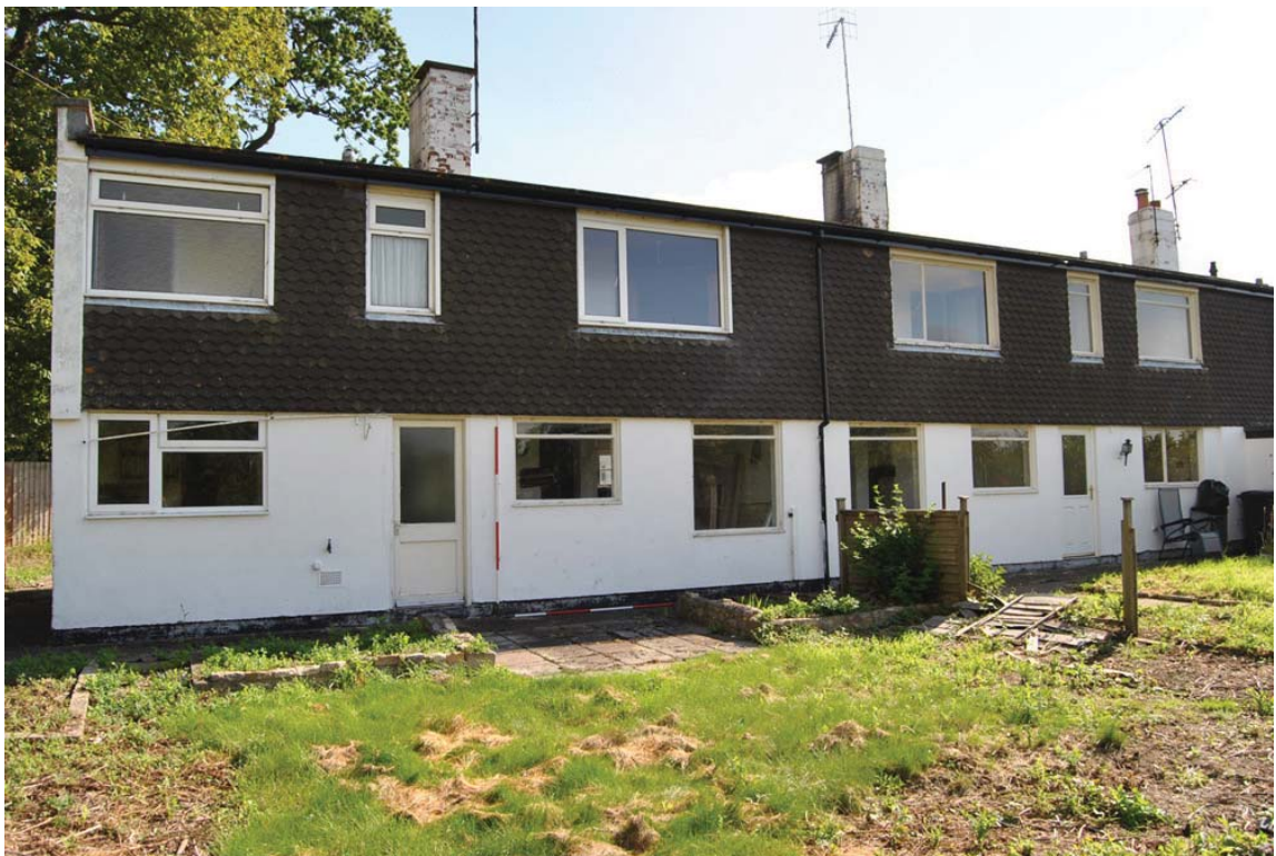
Plate 8: Nos 1 and 2 Black and White Cottages; extended elevation to rear (south).
