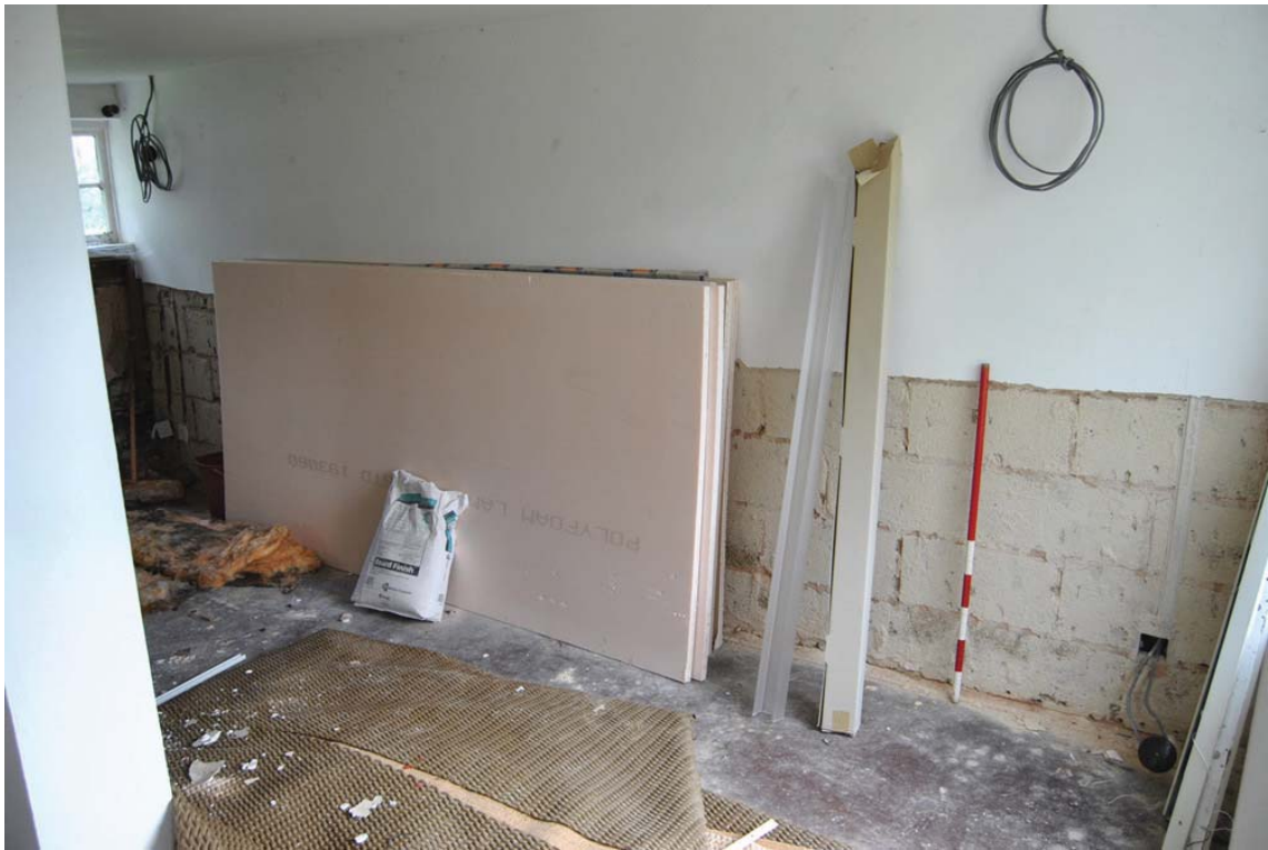
Plate 16: Inserted blockwork east wall of [G.03].
