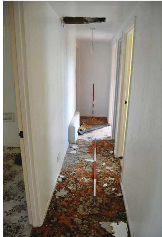
Plate 23: Corridor [F.01] looking east.
