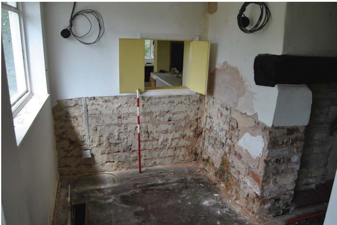
Plate 15: Blockwork wall south of stack, [G.03].
