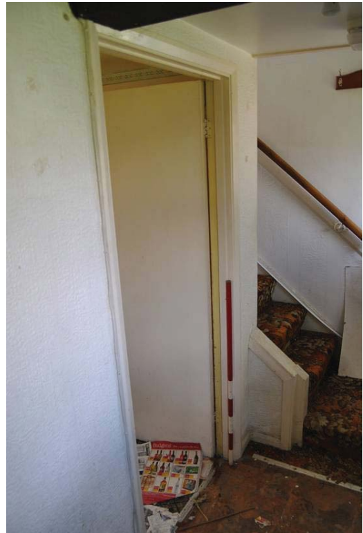
Plate 10: Hallway [G.01] looking west.
