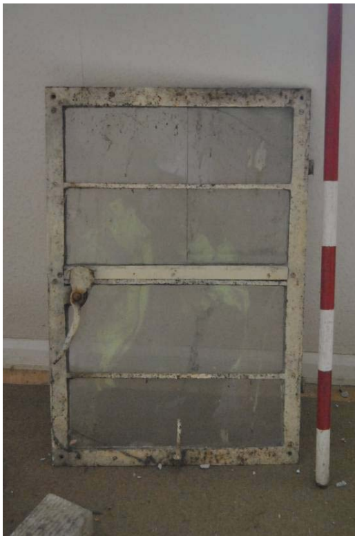
Plate 45: Early iron casement retrieved from behind plasterboard in [F.10].
