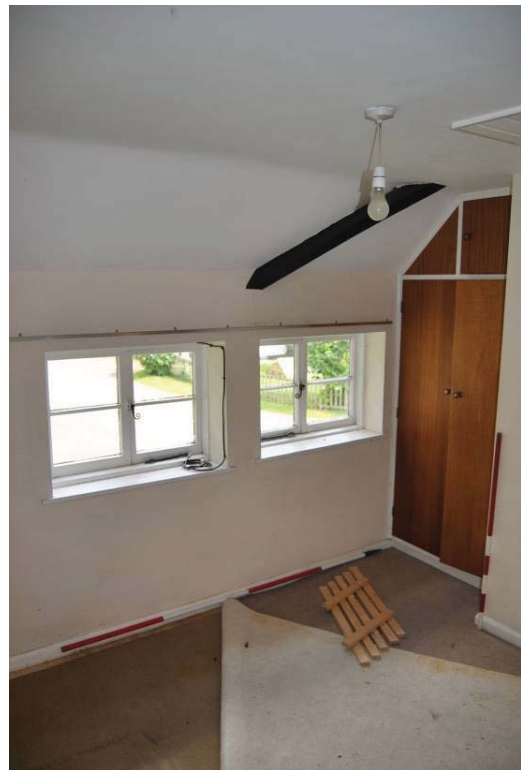
Plate 42: Bedroom [F.10] looking north-east; NB: angled brace.
