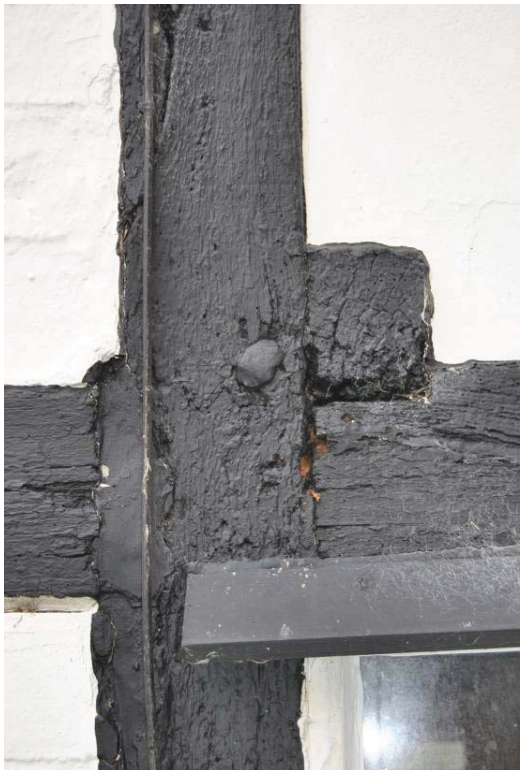
Plate 21: Transverse beam (bolted) visible to front elevation.
