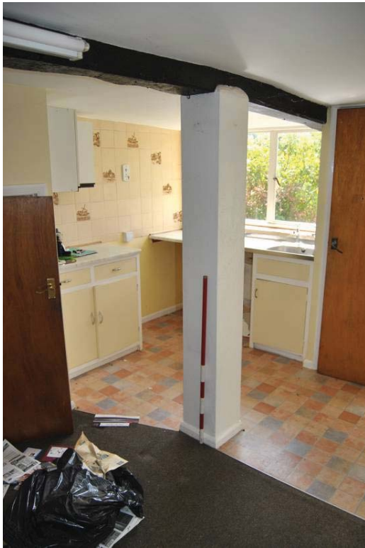
Plate 37: Kitchen [G.05] looking south; NB: transverse beam supported by brick pier.
