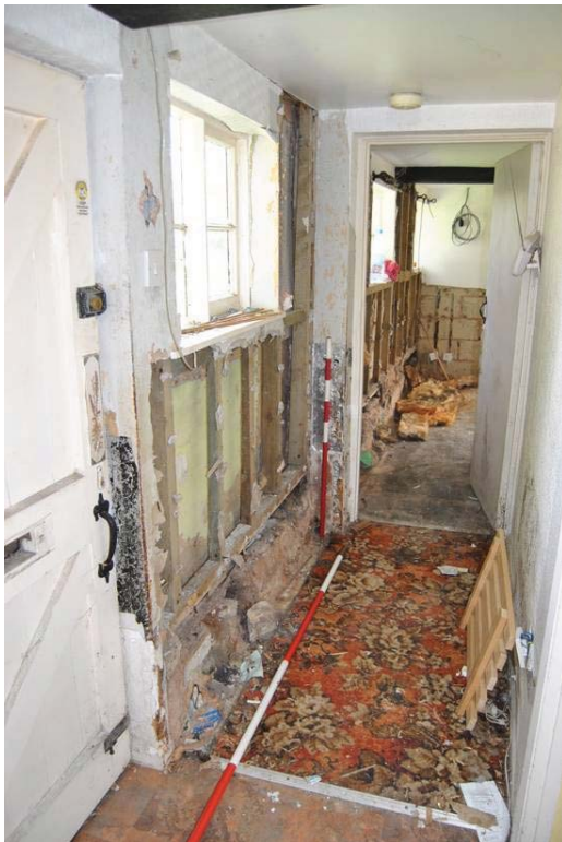
Plate 9: Hallway [G.01] looking east.
