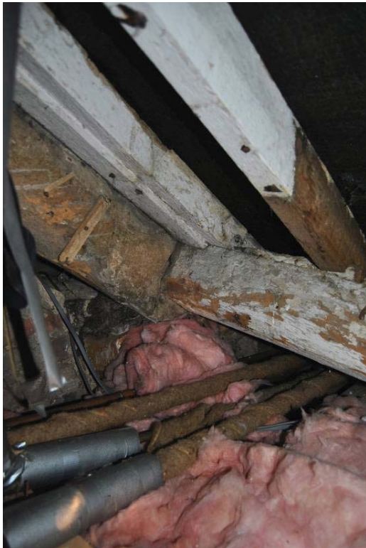
Plate 48: Detail of through purlin lodged over principal.
