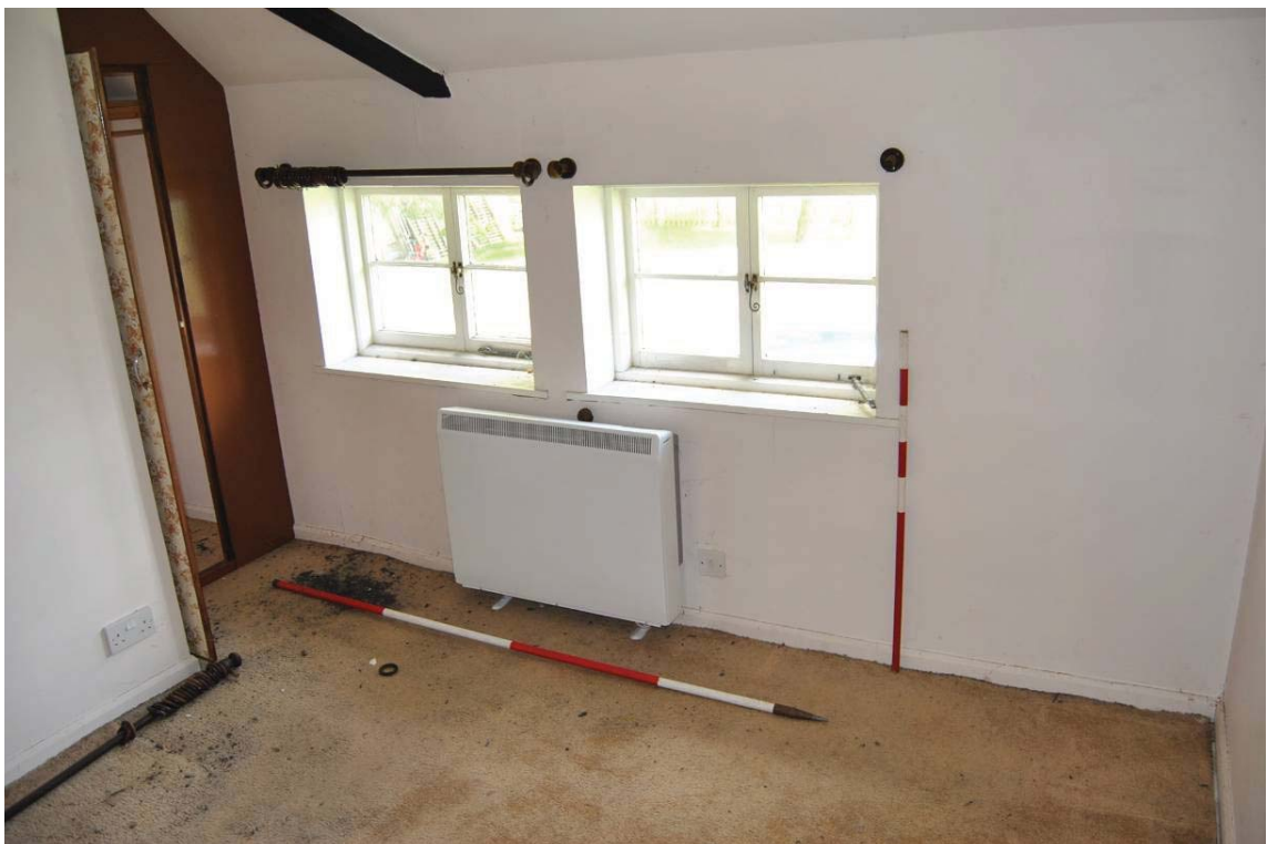
Plate 26: Bedroom [F.03] within early, front part of range (cupboard to left flanks stack); NB: angled brace (see Plate 48).
