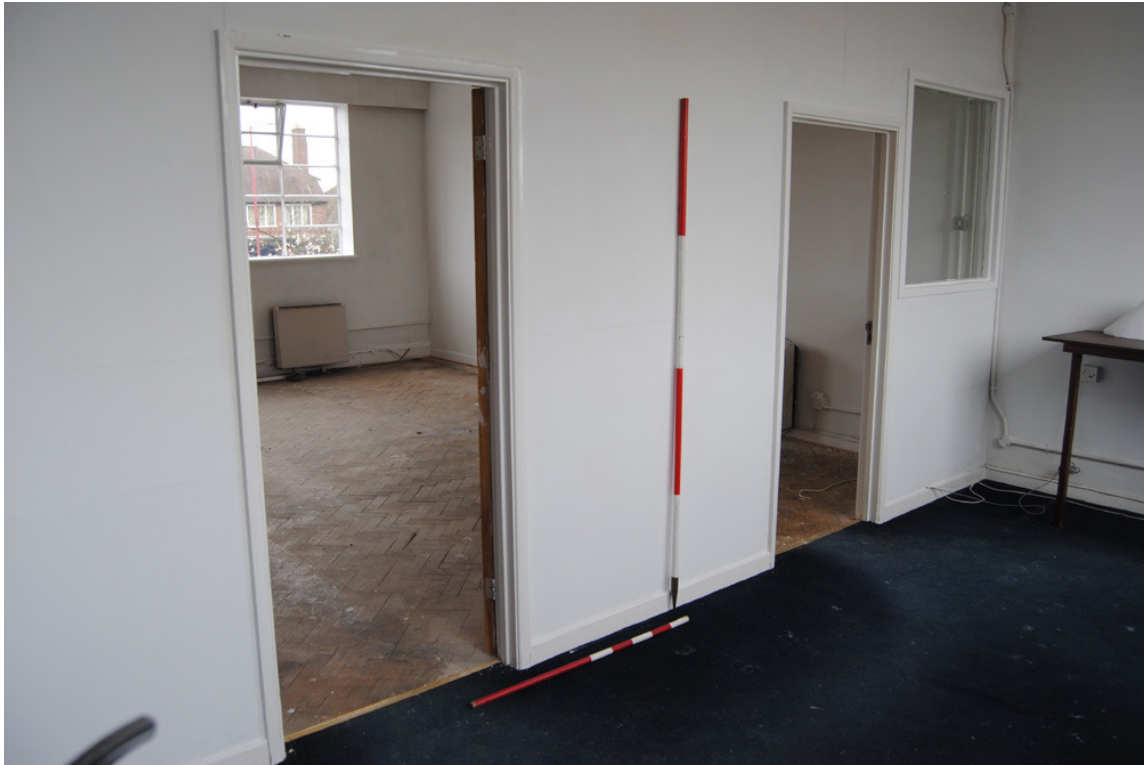
Plate 23: Crown Buildings; inserted partitions at [1F10/11].
