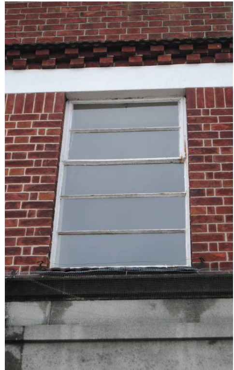
Plate 4: Crown Buildings; 1F single-light window lighting internal stair (north).
