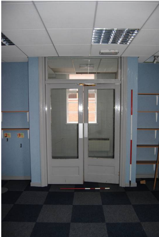
Plate 18: Crown Buildings; original double doors at head of Stair A.
