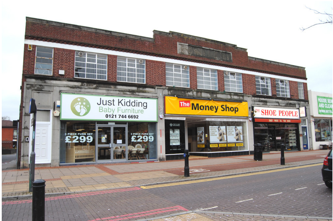
Plate 2: Nos.180-184 Stratford Road ('Crown Buildings'), general view looking west.
