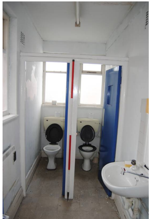
Plate 25: Primary lavatory partitions at [1F09].
