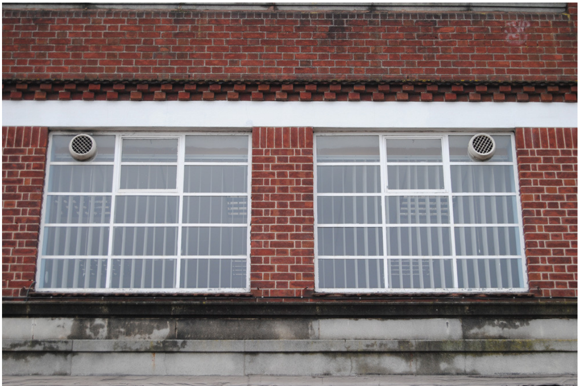
Plate 5: Crown Buildings; detail of first floor fenestration and dentillated string course.
