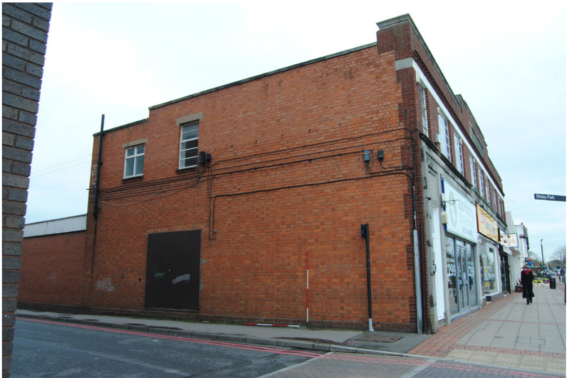
Plate 7: Crown Buildings; southern return elevation.
