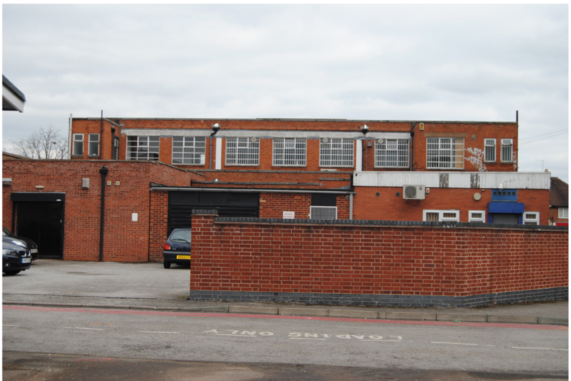
Plate 9: Crown Buildings; rear (western) elevation.
