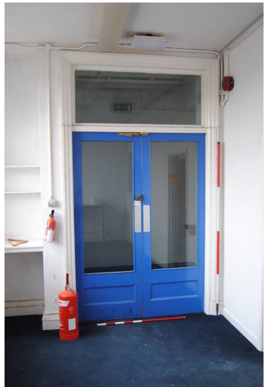
Plate 19: Crown Buildings; original double doors at head of stair B.
