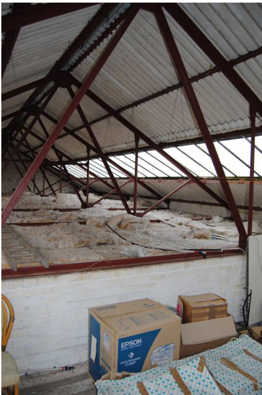
Plate 36: Warehouse roof looking south-west.
