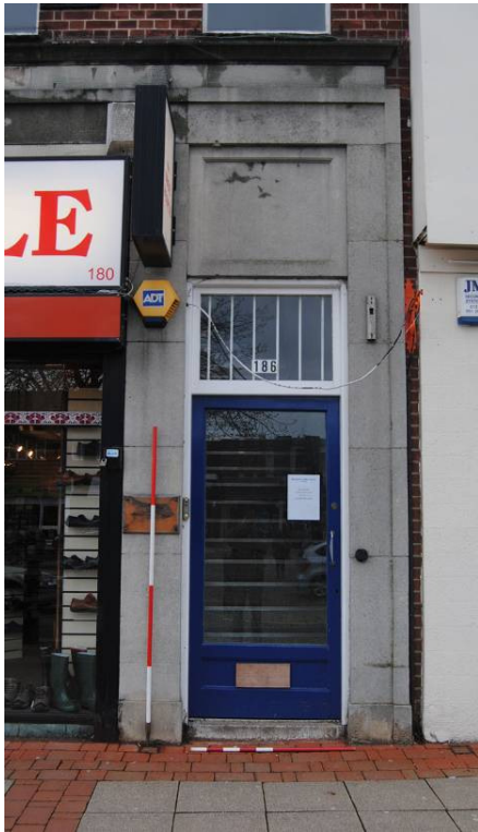
Plate 3: Crown Buildings; northern doorway.
