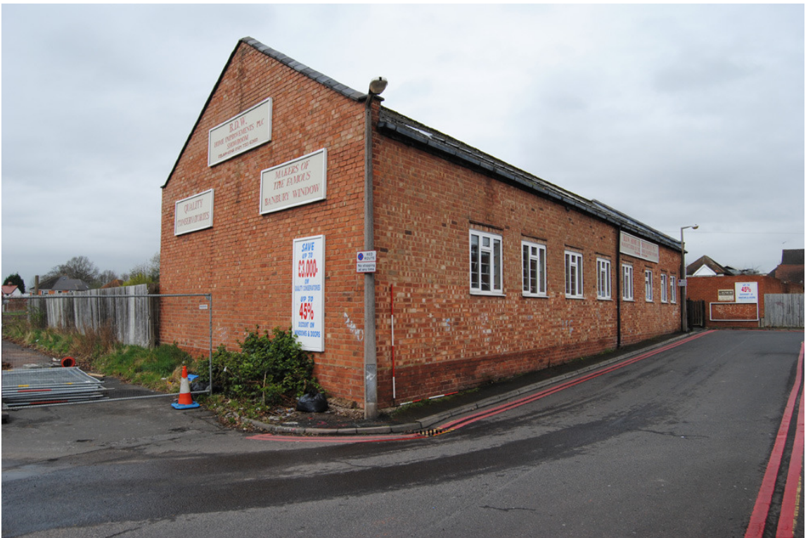
Plate 32: Warehouse; general view looking north-west.
