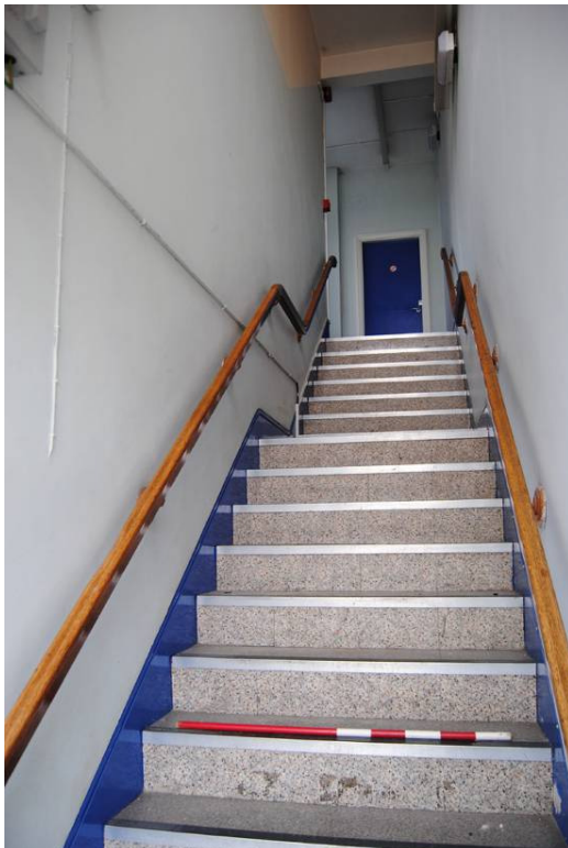
Plate 16: Crown Buildings; northern stair B.
