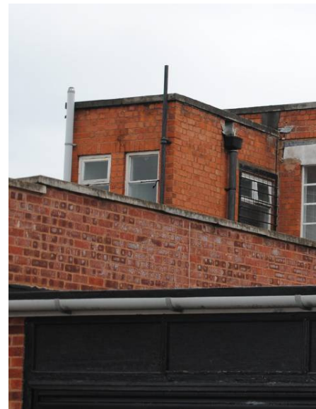
Plate 12: Crown Buildings; northern 1F projection.
