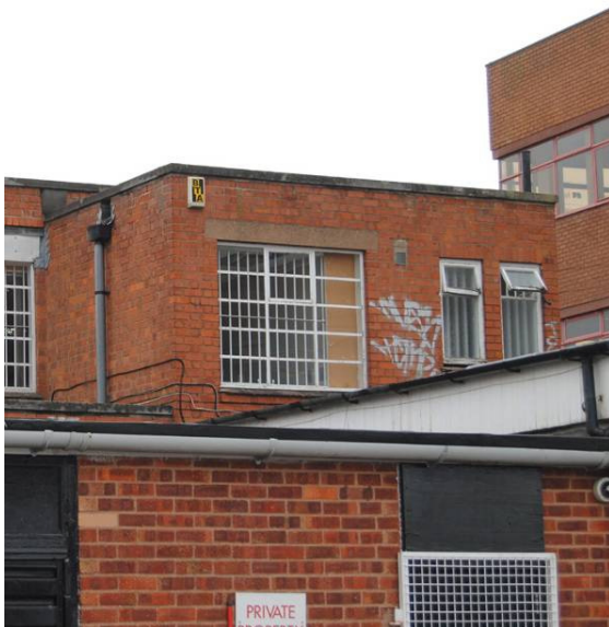
Plate 11: Crown Buildings; southern 1F projection.
