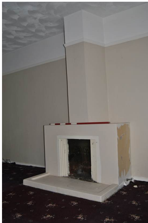
Plate 12: Original FP, flue and hearth (No.52).
