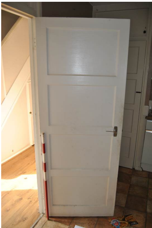
Plate 21: Detail of original four-panel door (kitchen, No.30).
