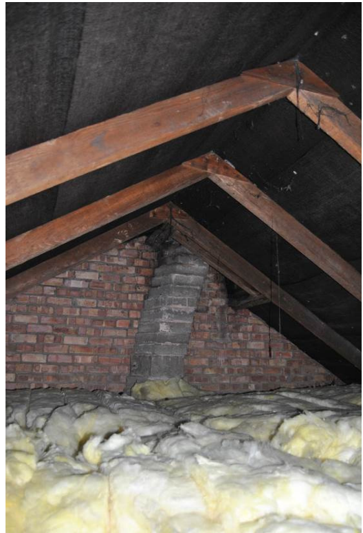
Plate 20: Roof structure over No.30 looking west, NB: concrete block stack angled to rear roof slope.
