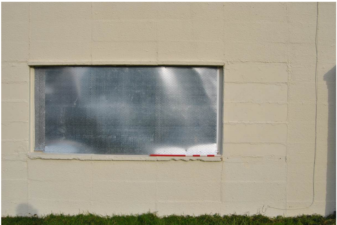
Plate 7: Detail of window opening fitted within bay system of PRC frame (No.50).
