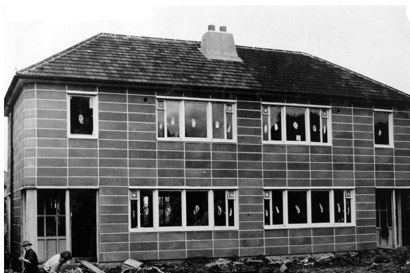
A 'Unity' house under construction (variant fenestration etc.) illustrating system of PRC columns and block infill walls.
