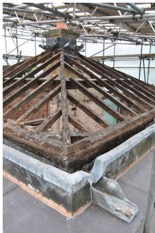
Plate 35: Lead-lined gully with outlet and overflow channel to north side of lodge.
