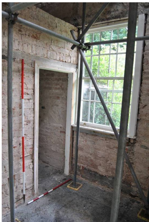
Plate 21: Detail of partition wall abutting south jamb of window [w1].
