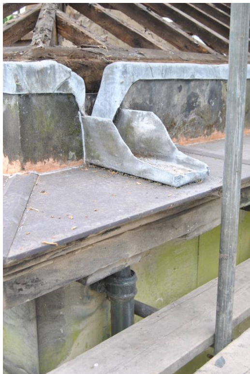
Plate 36: Detail of gutter outflow and downpipe beneath cornice.
