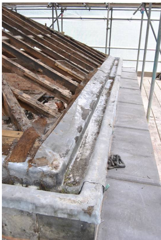
Plate 34: Lead-lined drainage gully, south side of lodge.
