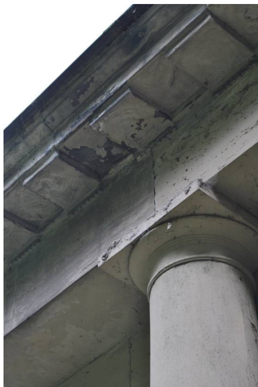
Plate 15: Projecting stone cornice with plain, flat mutules and guttae.
