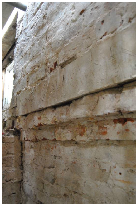
Plate 26: Offset in brickwork of south wall at 1F level.
