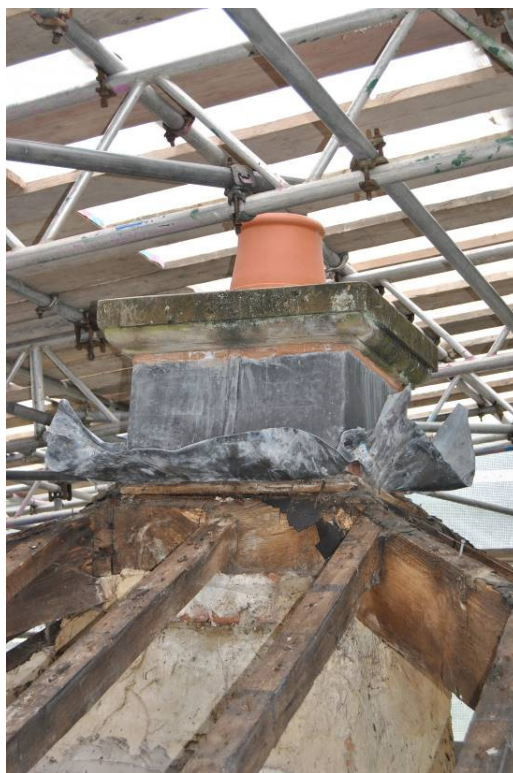
Plate 33: Central stack to apex of roof with trimmed-frame supporting head of hip rafters.
