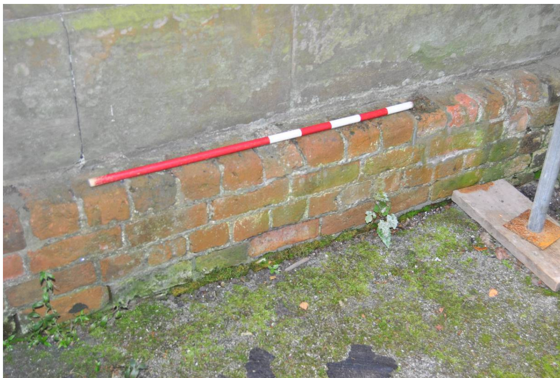
Plate 18: Brick footing to base of north elevation.
