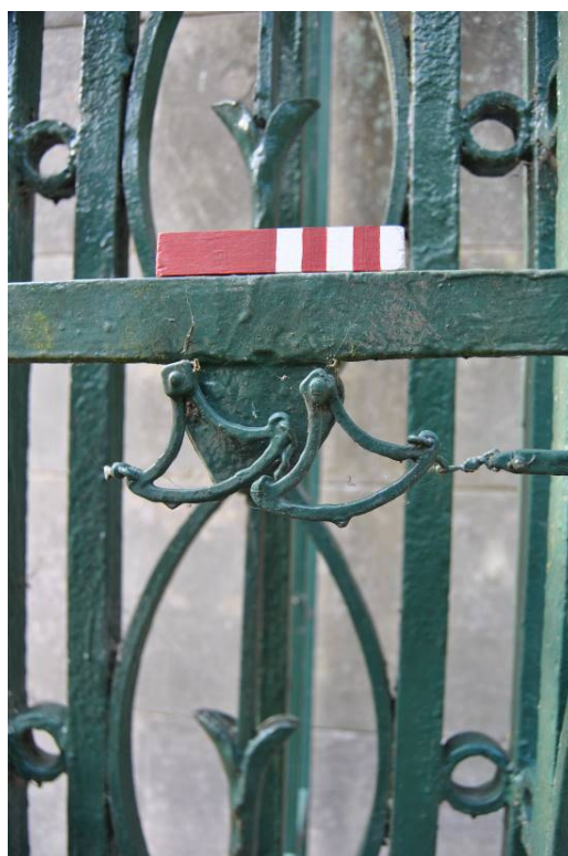
Plate 7: Detail of bell pull mechanism.
