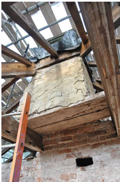
Plate 37: Detail of 'offset' section of upper stack supported on timber planks between ceiling beams.
