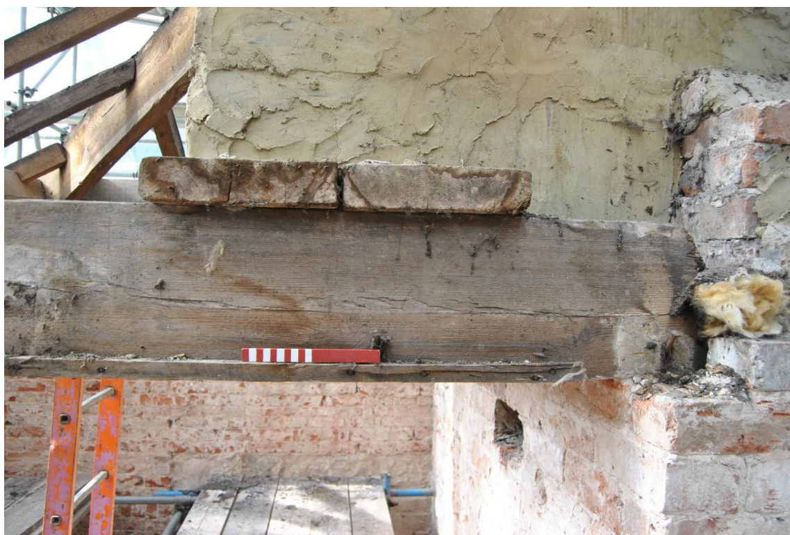
Plate 38: Detail of upper chimney supported on timber planks laid across top of ceiling beams.
