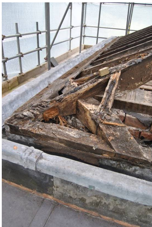
Plate 32: Angle-tie to north-west corner of roof.
