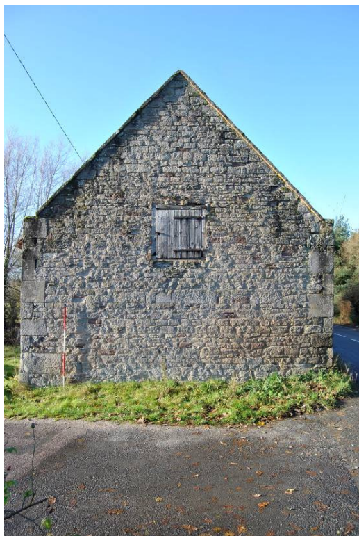
Plate 9: East gable end (?upper section rebuilt).
