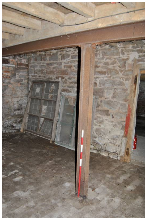
Plate 66: Secondary RSC support to 1F.
