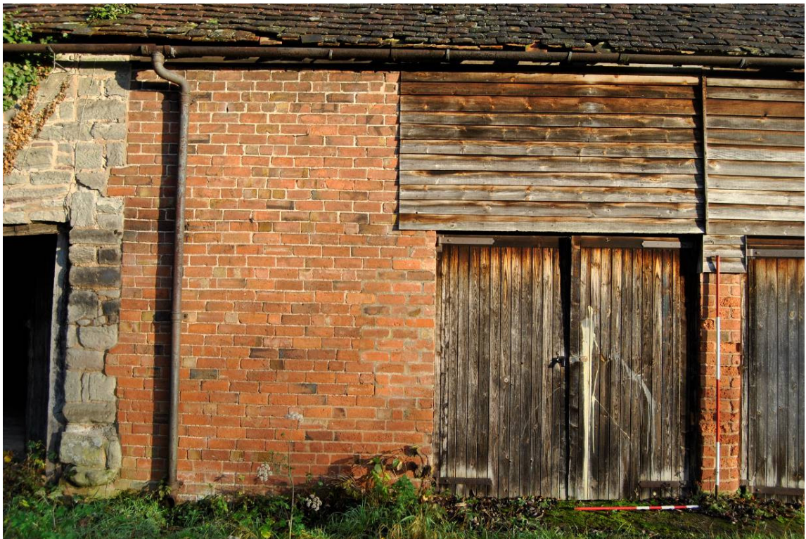
Plate 35: Block [B] (west); doors [d3] with brick patching to western jamb.
