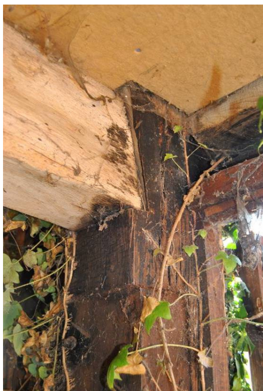
Plate 43: Transverse beam supported at wall post (S).
