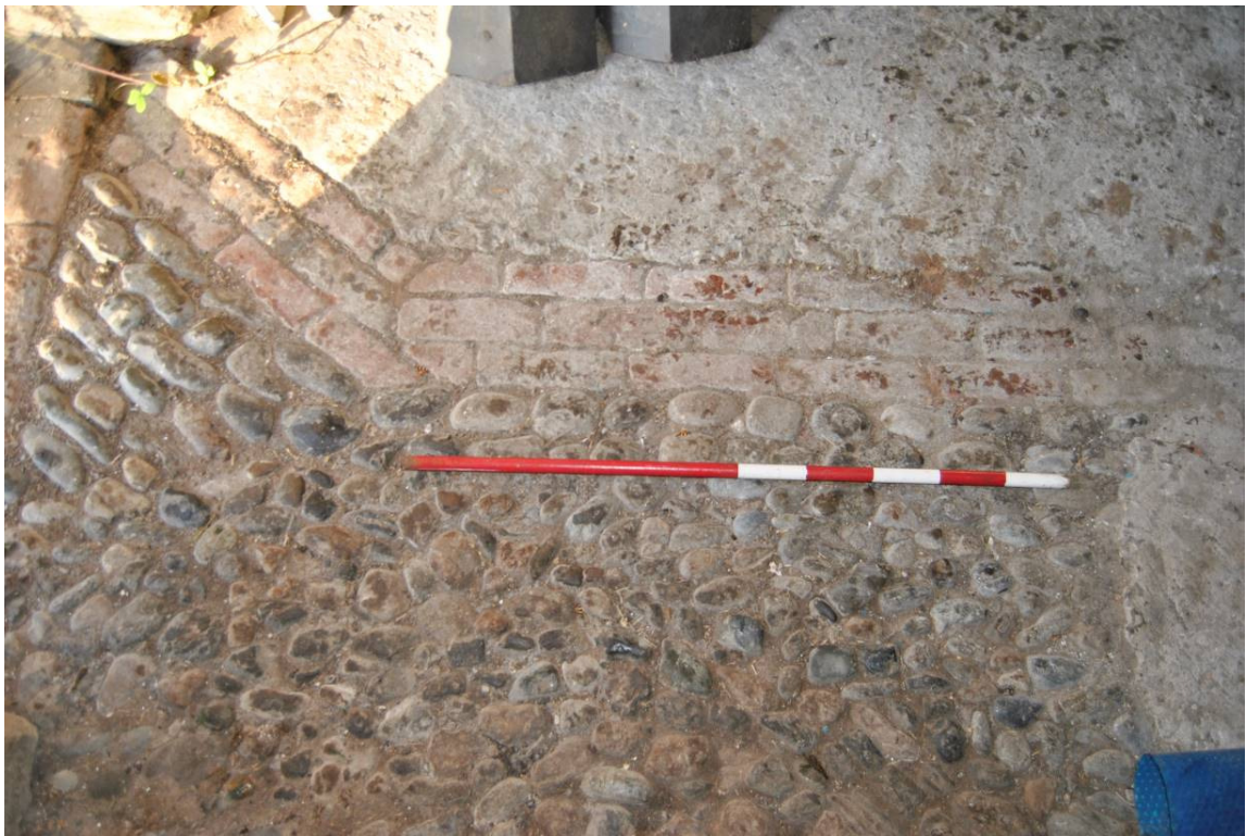
Plate 19: Detail of surviving cobbled floor with brick-lined drainage channel.
