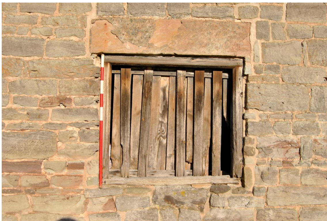
Plate 6: 'Hit and Miss' ventilator [w1].
