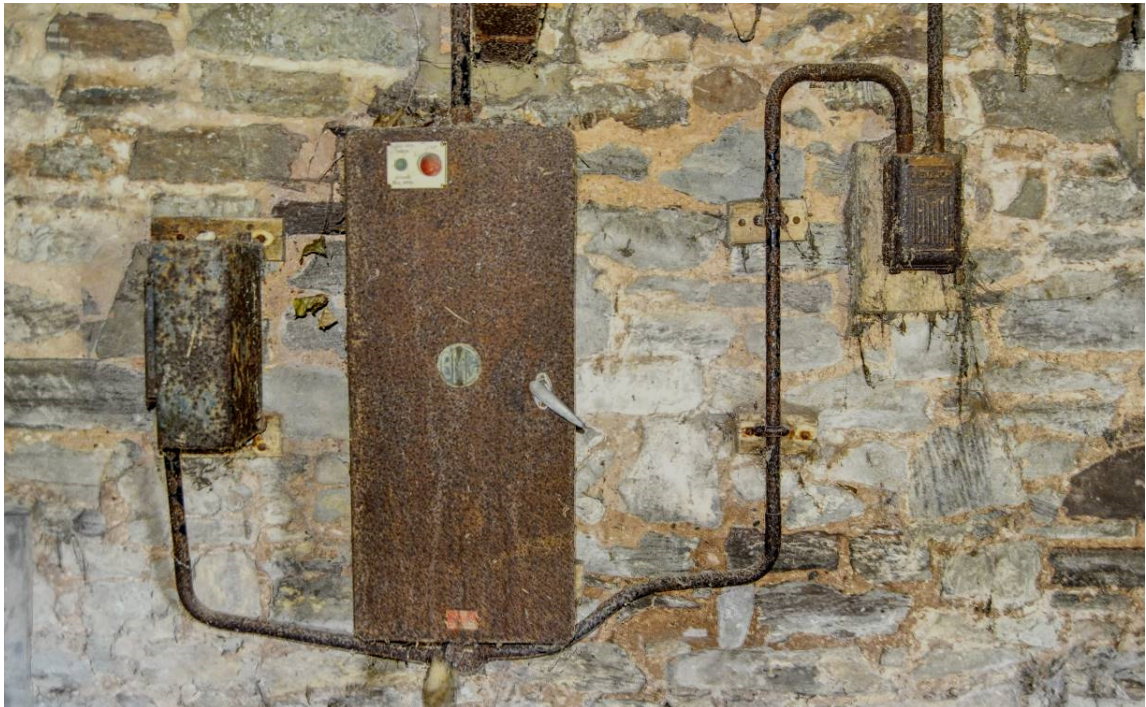
Plate 74: Electrical switch-gear by Brook Motors Ltd of Huddersfield, north wall [G4].
