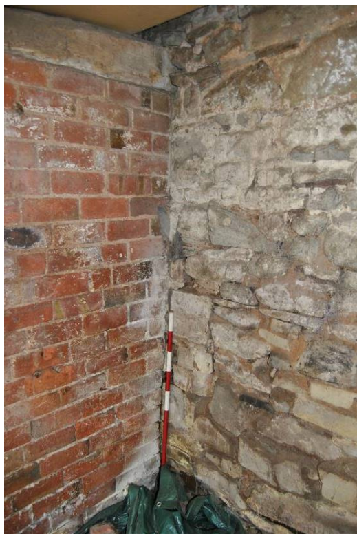
Plate 41: Brickwork partition abuts north wall.
