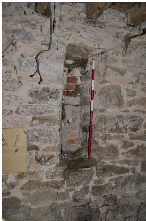
Plate 71: Splayed ventilation slot to west wall, blocked externally in brick.
