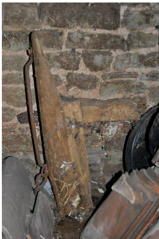
Plate 23: Feed-trough support with tethering bar.
