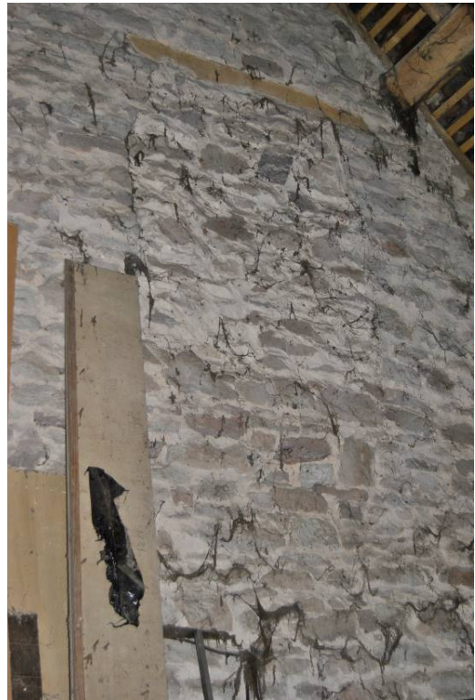
Plate 53: Blocked pitching door [w11] to west wall.
