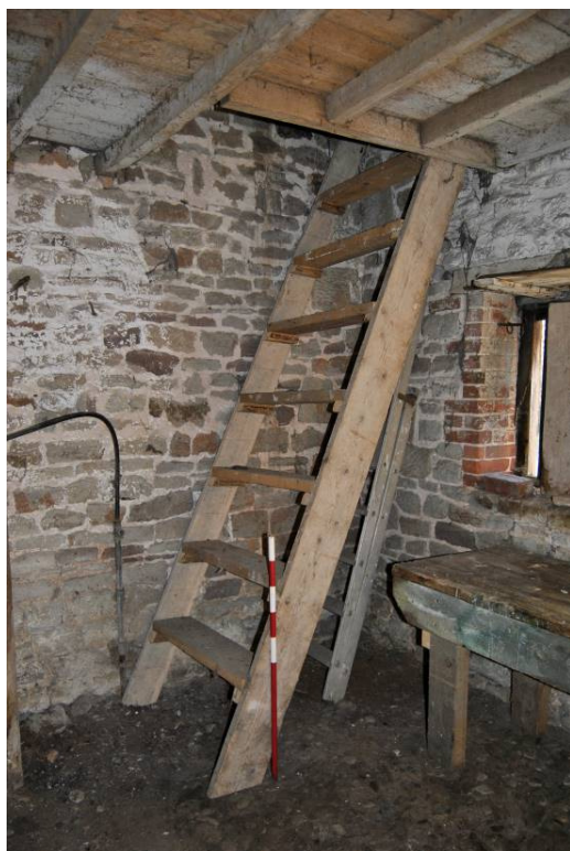
Plate 26: Inserted timber stair at SE angle.
