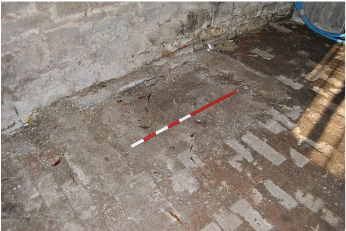
Plate 73: Concrete pad against west wall for former article of plant (?a.c. motor).
