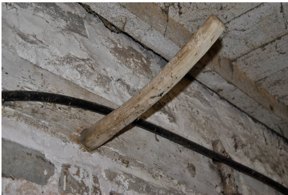
Plate 25: Detail of timber harness hook, north wall.
