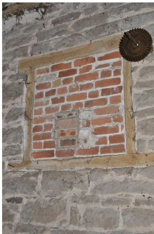
Plate 86: Blocked pitching door [w11] to east wall.
