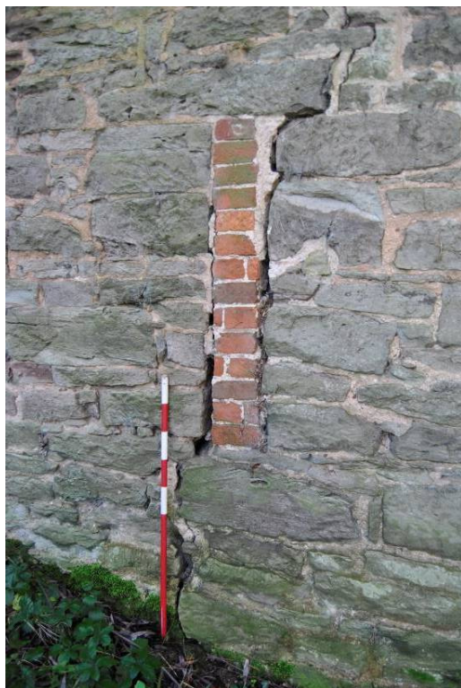
Plate 63: Blocked ventilation slot.
