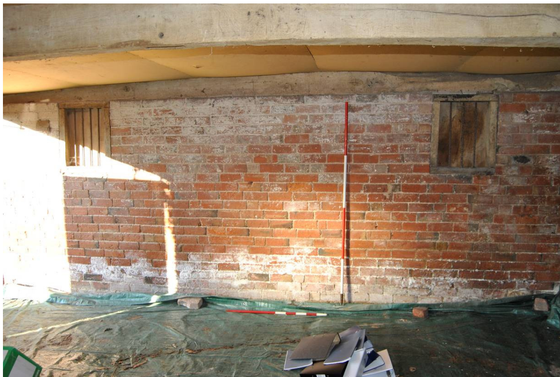
Plate 40: Inserted, transverse partition to west side of [G2].
