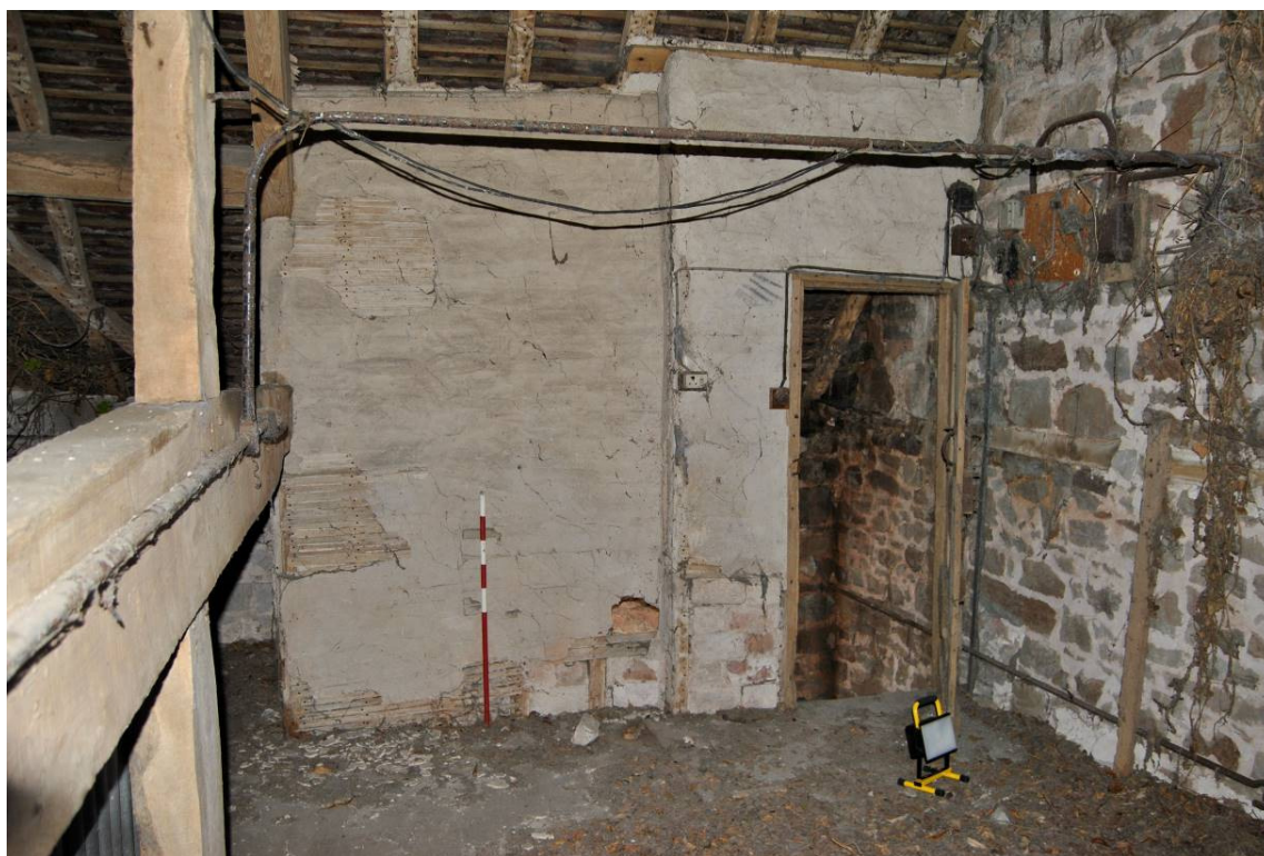
Plate 79: Detail of head of enclosed stairwell looking south. NB. ducted cable runs and switch-gear to west wall (right).
