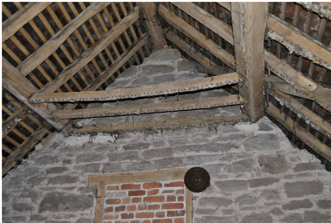
Plate 84: Ceiling joists extending between upper purlins with evidence for former L&P render.
