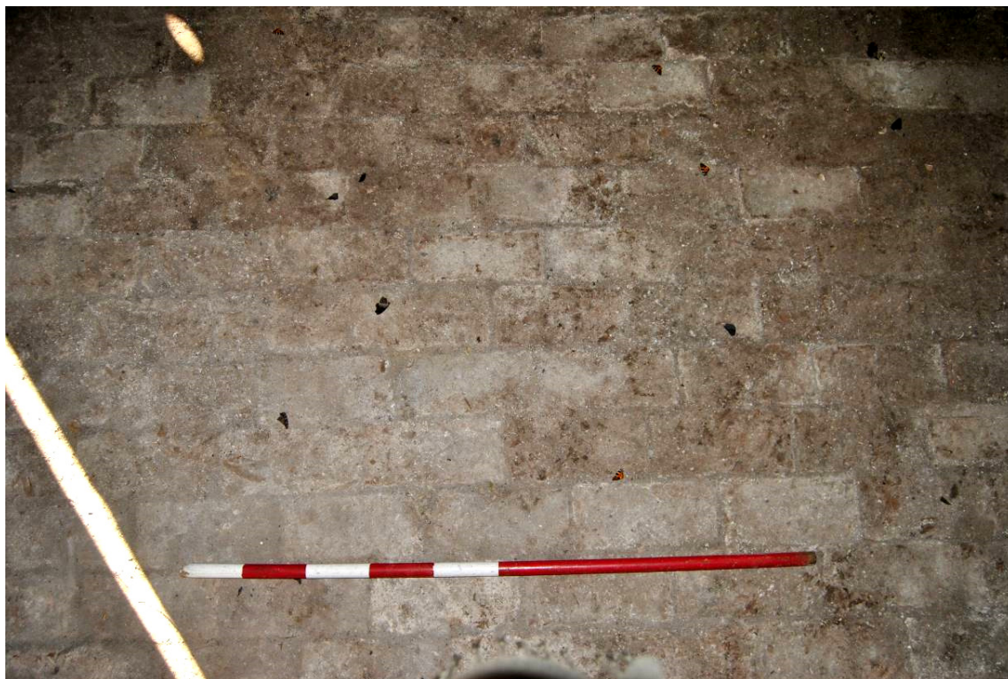
Plate 69: Face-laid brick paviour floor.
