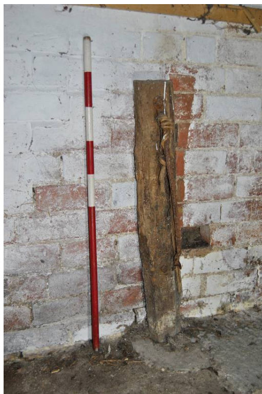
Plate 47: Timber post with tethering bar to south wall.
