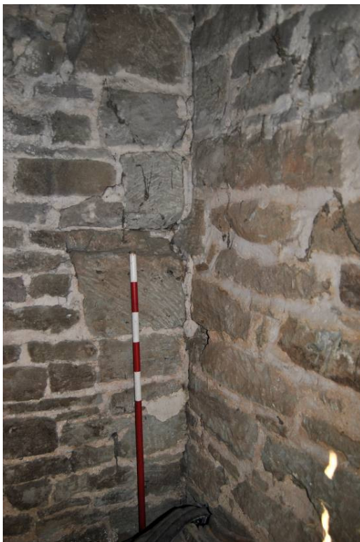
Plate 20: South wall (left) abuts west wall (right).
