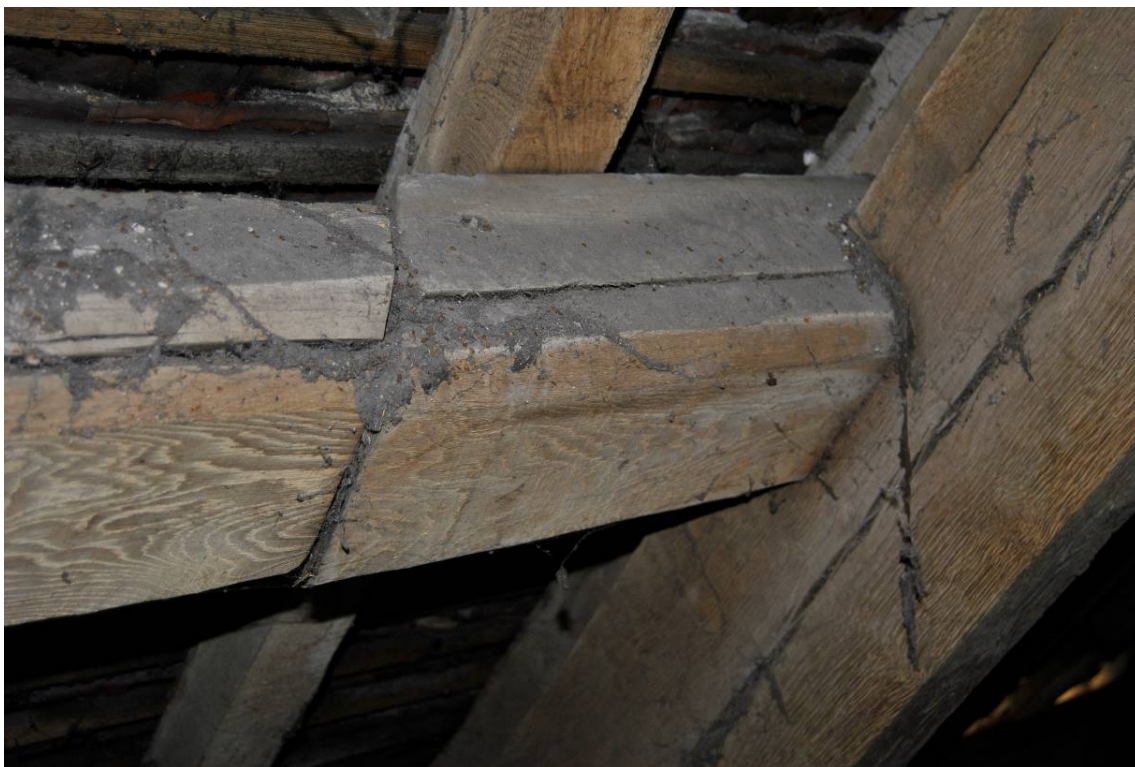
Plate 32: Detail of lower purlin (S); scarf joint to east of T1.
