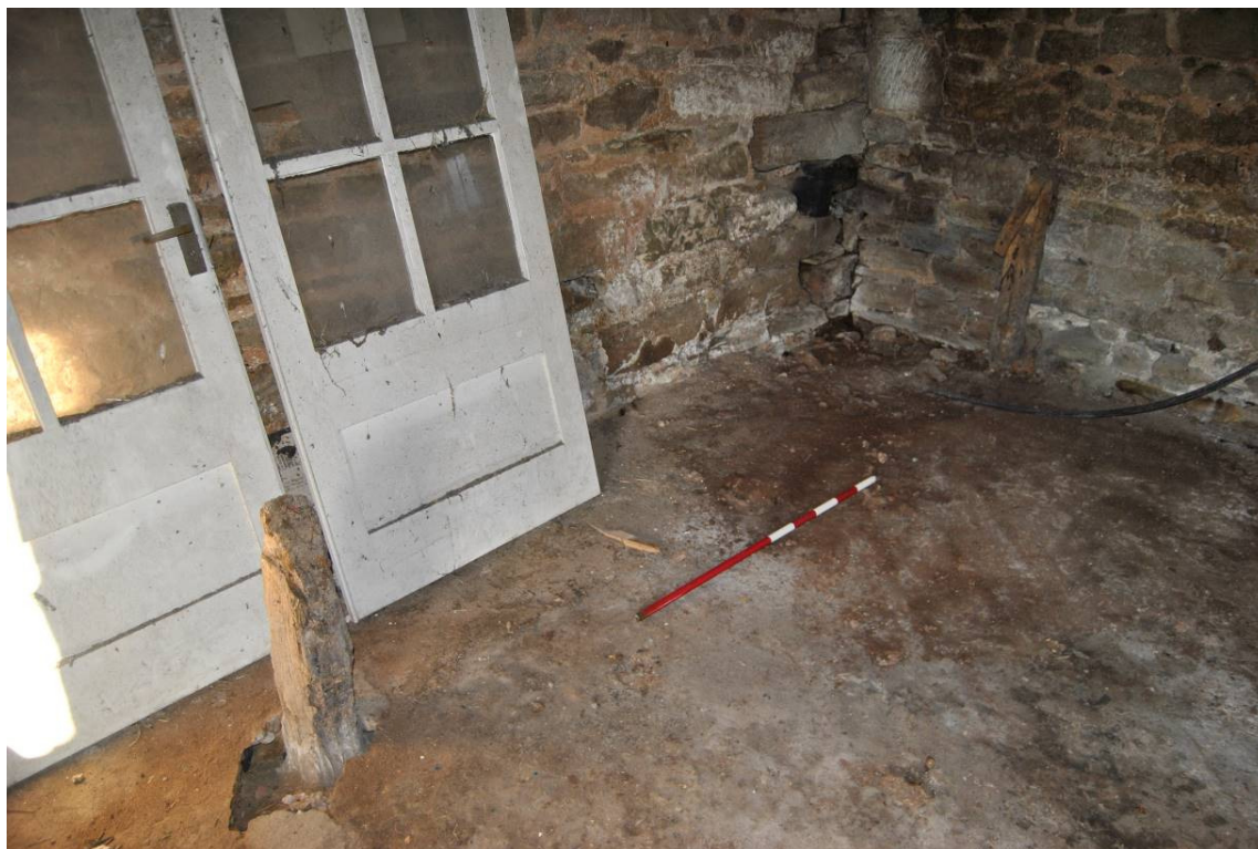
Plate 22: Feed trough supports to west side of [G1].
