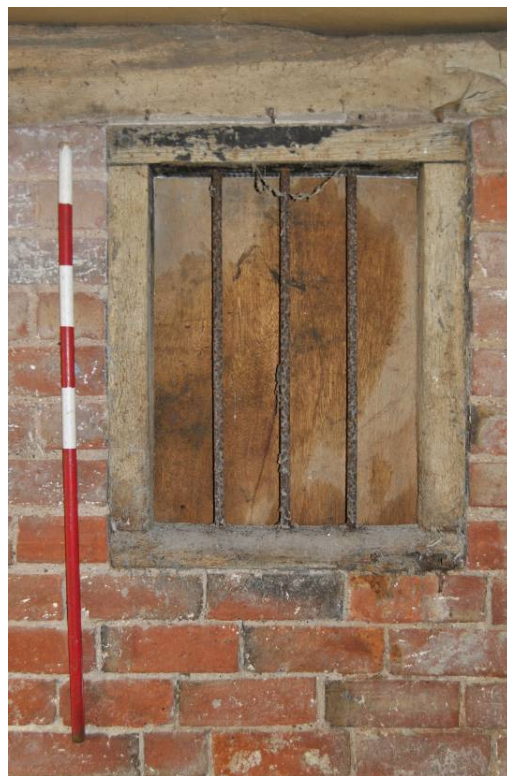
Plate 42: Detail of window in partition wall.
