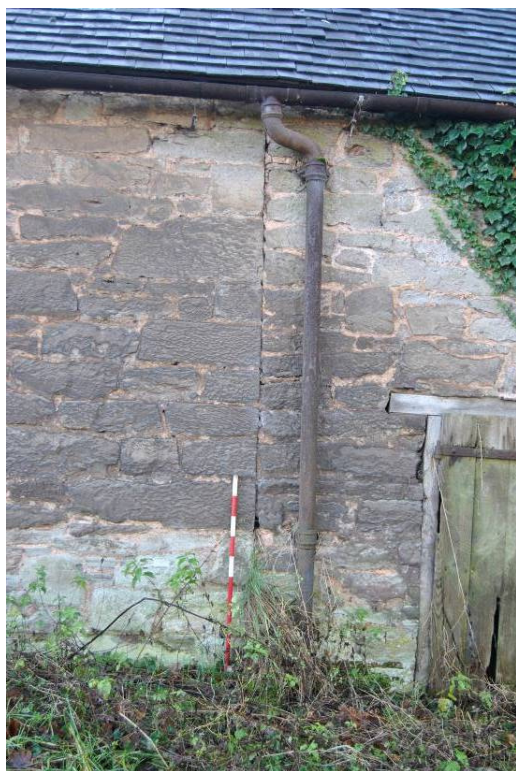
Plate 61: SJ at junction of [B] (left) and [C] (right).
