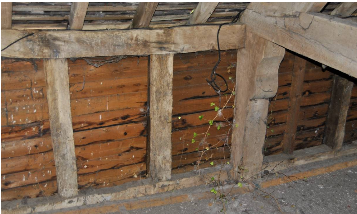
Plate 54: Studs extending between rail and wall plate at Bay 3 (S), pegged top and bottom.
