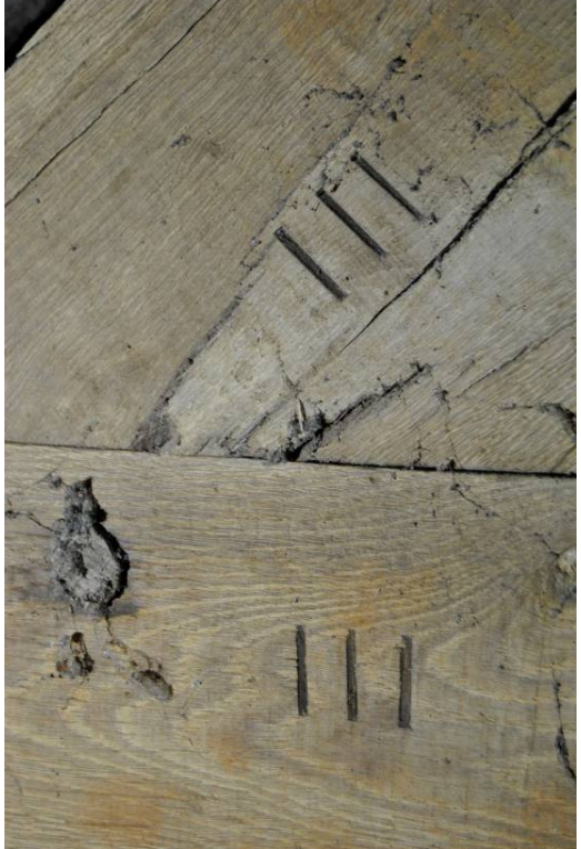
Plate 31: Detail of chiselled carpenter's marks (T1).
