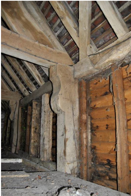
Plate 52: Ogee-moulded wall post to truss T3 (S).
