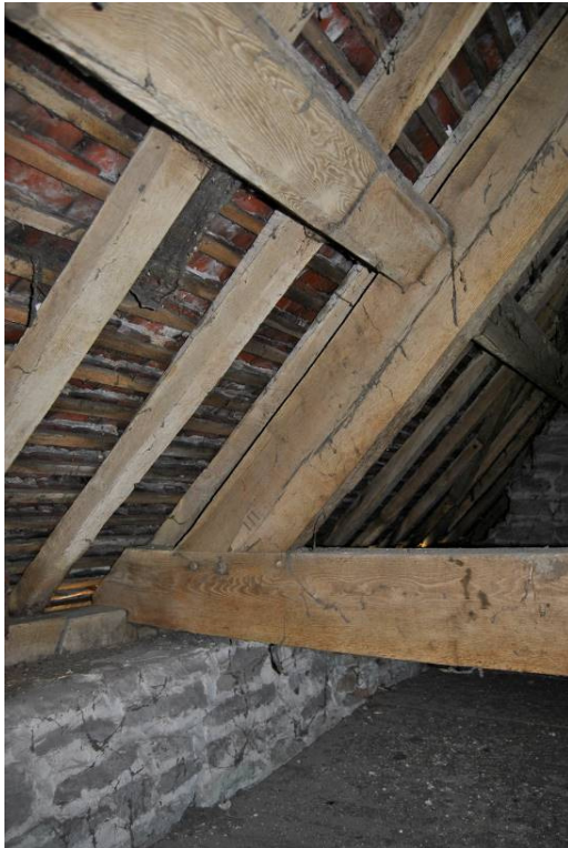
Plate 30: Detail of truss T1; tie / principal (S).
