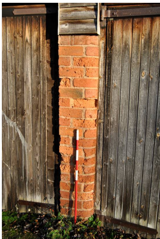
Plate 36: Brick pier between [d2/3]; NB. bull-nosed to east, plain to west.
