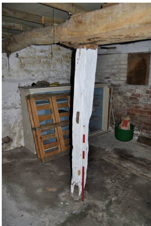
Plate 46: Timber post beneath transverse beam.
