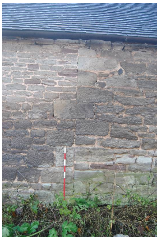
Plate 13: Detail of SJ/quoins at junction of [A] (left) and [B] (right).
