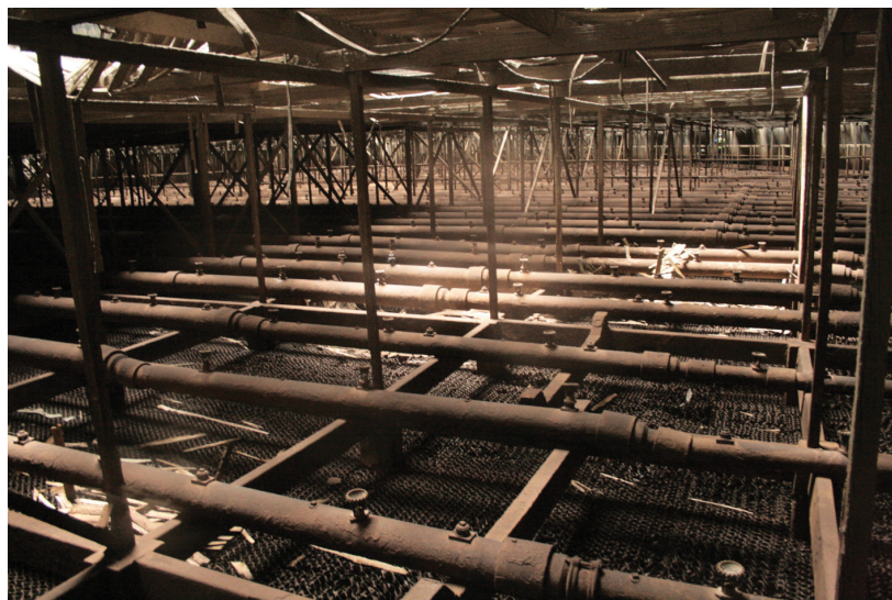
(c) original distributor pipework prior to removal (NB. sprays to top of pipes)
