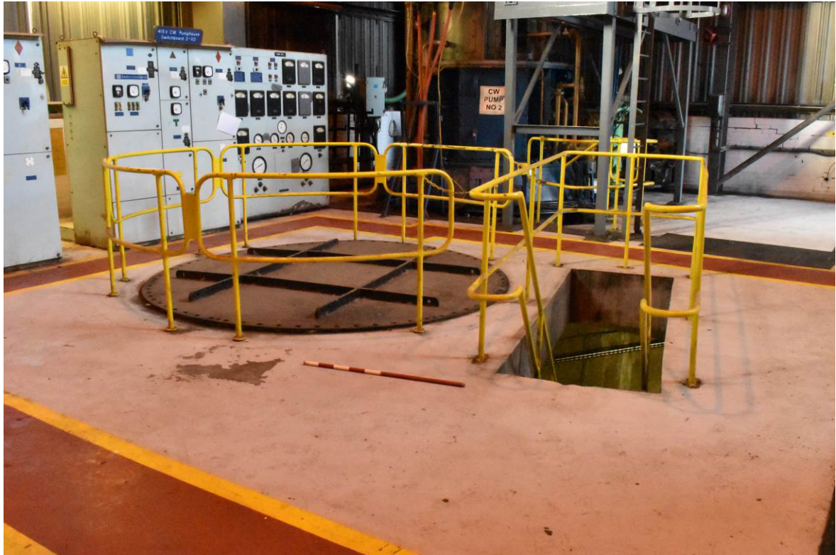
Plate 48: Dismantling pit and associated access stair adjacent to CW pump 2.
