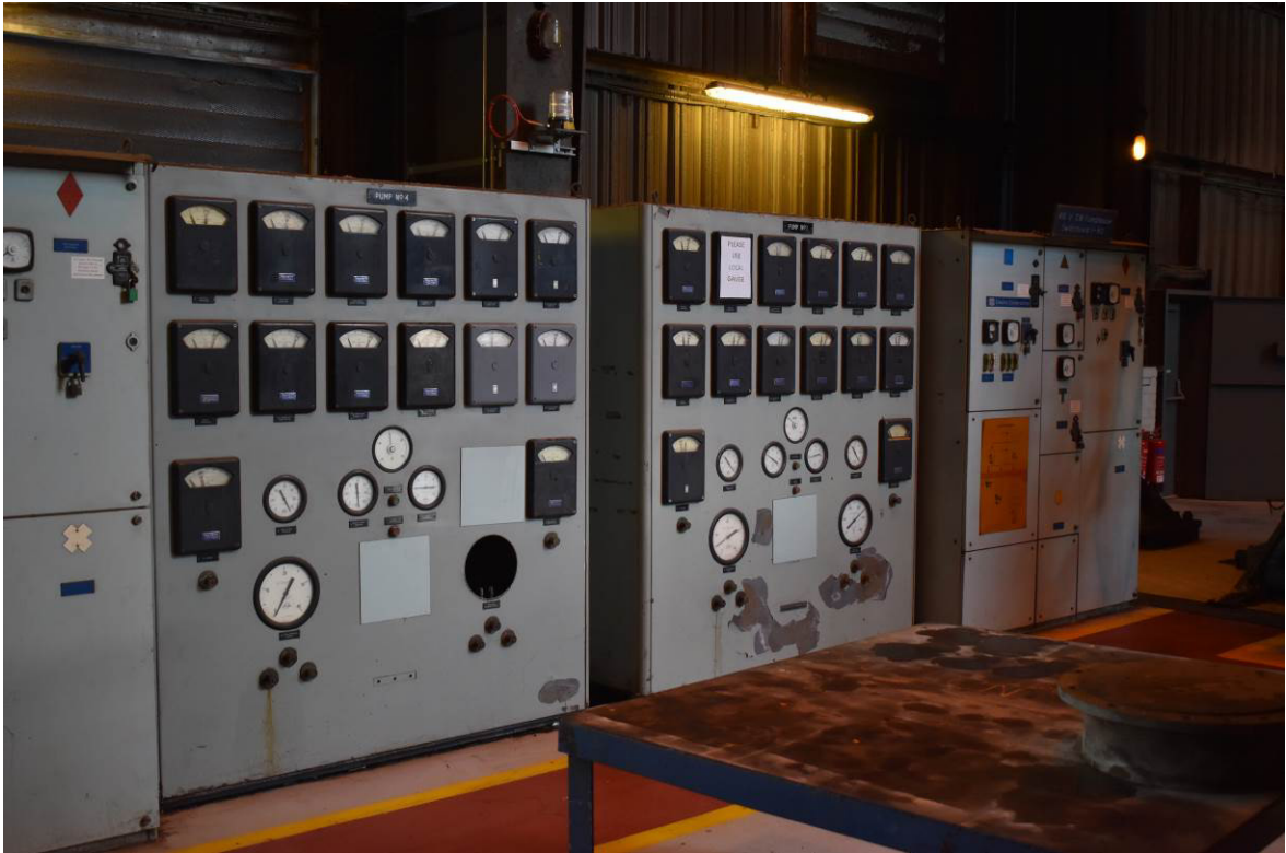
Plate 46: Pump 1 and 4 control panels to east side of CW pump house.
