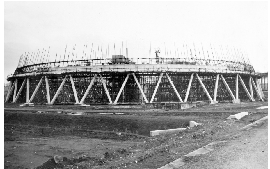
(b) Cooling tower 2a early in construction, CEGB photo ref. RAT.243, dated 15.04.1965.
