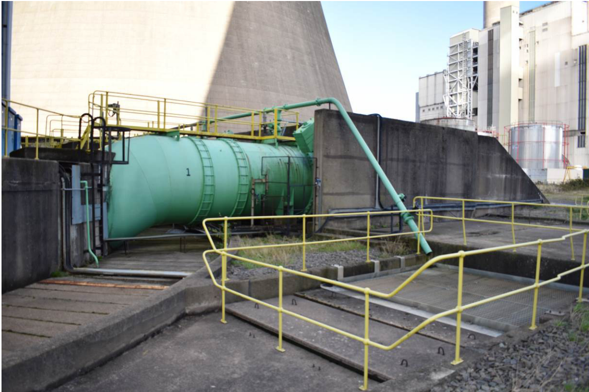
Plate 39: CW pumphouse discharge pipework with CT3a return channel to foreground.
