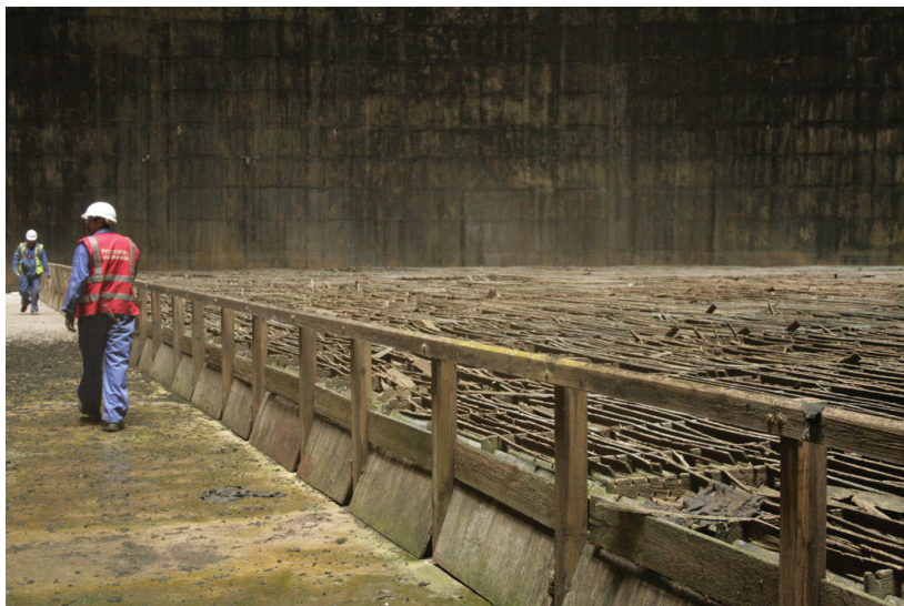
(a) timber drift eliminator prior to removal
