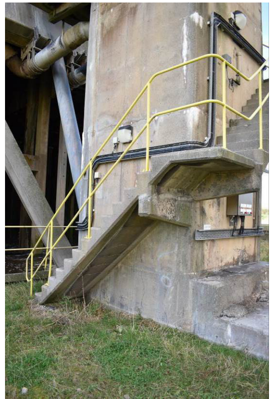
Plate 18: Detail of cantilevered concrete stair
