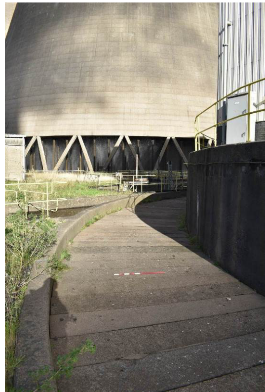
Plate 38: Detail of covered annular moat.
