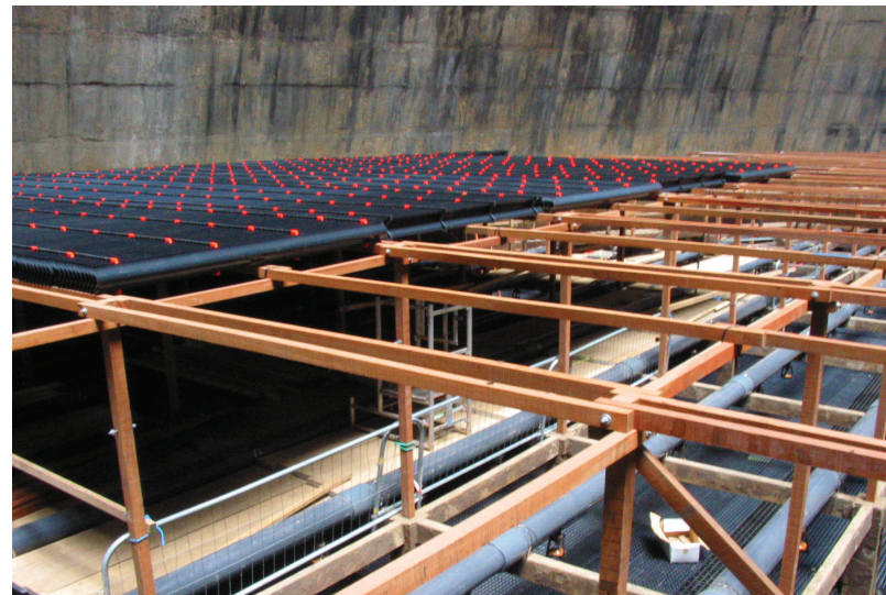
(b) new drift eliminator during installation
