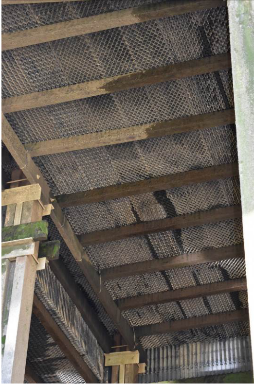
Plate 26: Soffit of (replacement) plastic packing units.
