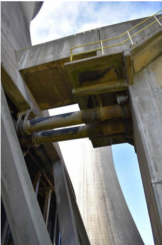
Plate 15: Detail of de-icer pipework feeding off main culvert upriser.
