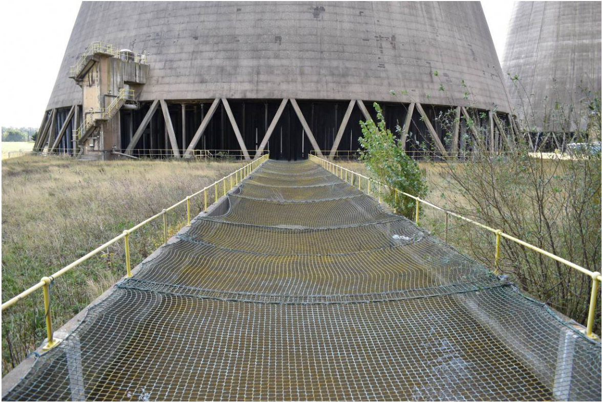
Plate 32: Circulating water return channel (netted) between CT3a and CT4a, looking south.
