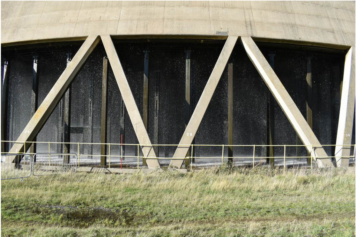
Plate 7: Primary V-strutting supports to air intake at base of cooling tower 4a.
