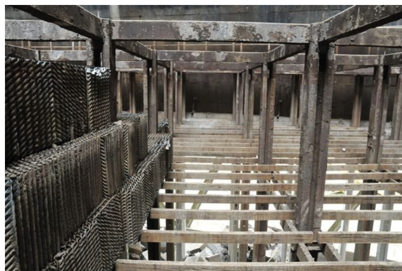
(d) previous (secondary) packing units during removal
