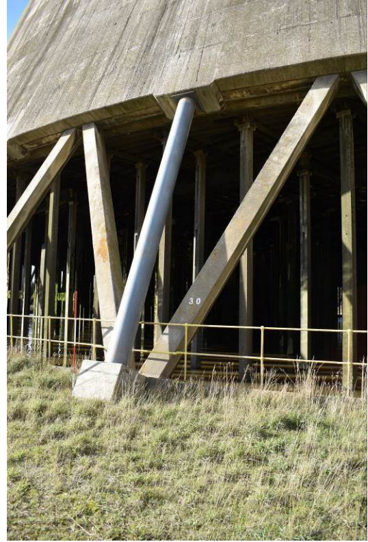
Plate 9: Detail of V-strutting with added prop, CT2a.
