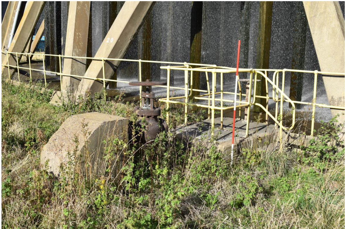
Plate 34: Redundant silt sump to pond perimeter of CT4a.
