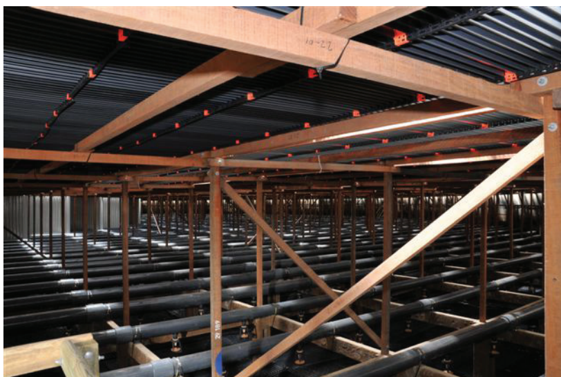
(c) new distributor pipework and drift eliminator in-situ
