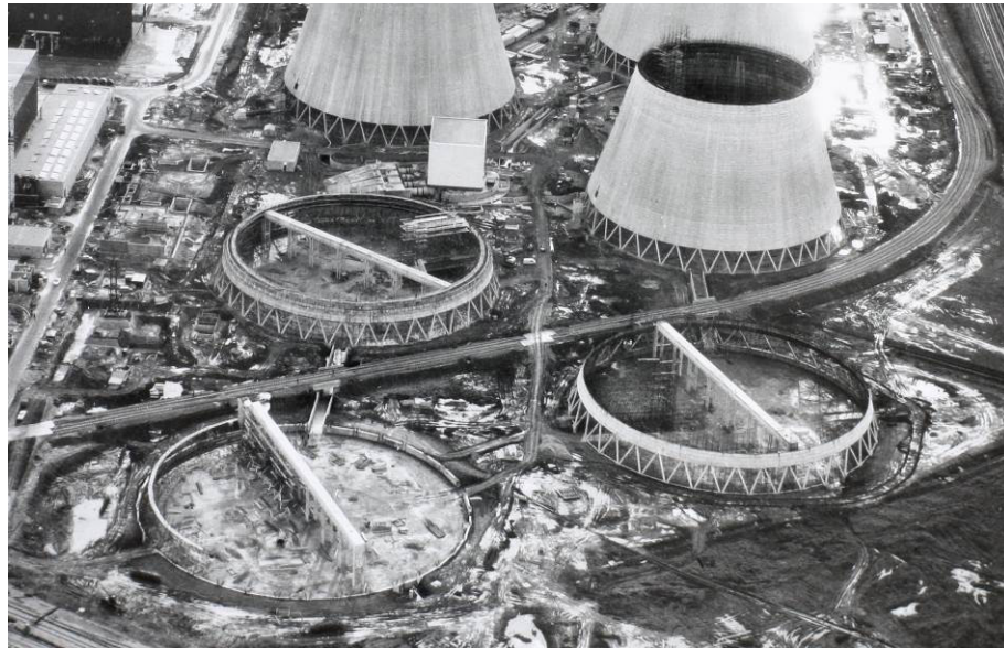
Aerial photograph of 'B' towers during construction, looking south, showing stages of progression (CEGB photo ref. A1168183, dated 14.11.1966; Uniper Archive, IMG_0383.jpg)
