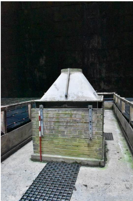
Plate 24: Vent to outer end of main distributor culvert.
