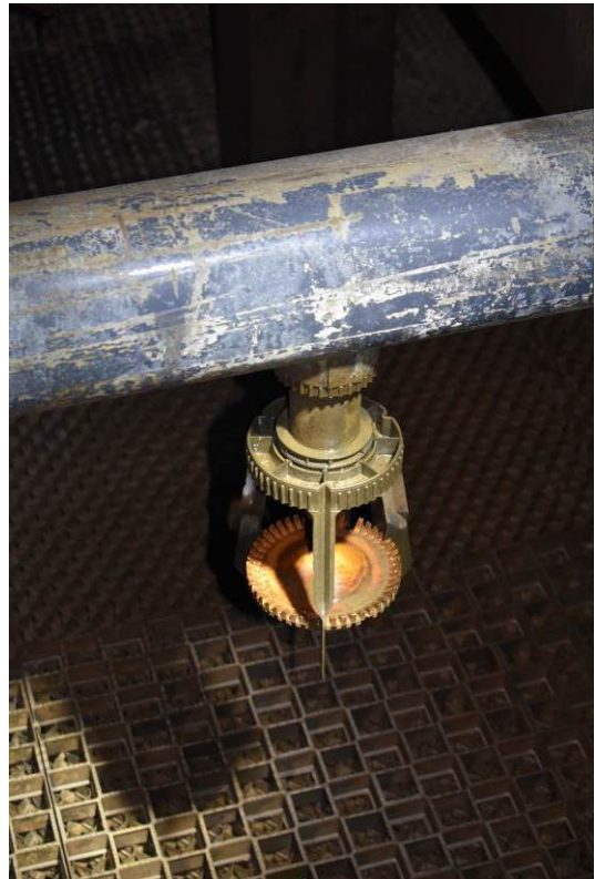
Plate 30: Detail of (renewed) pendant spray head.
