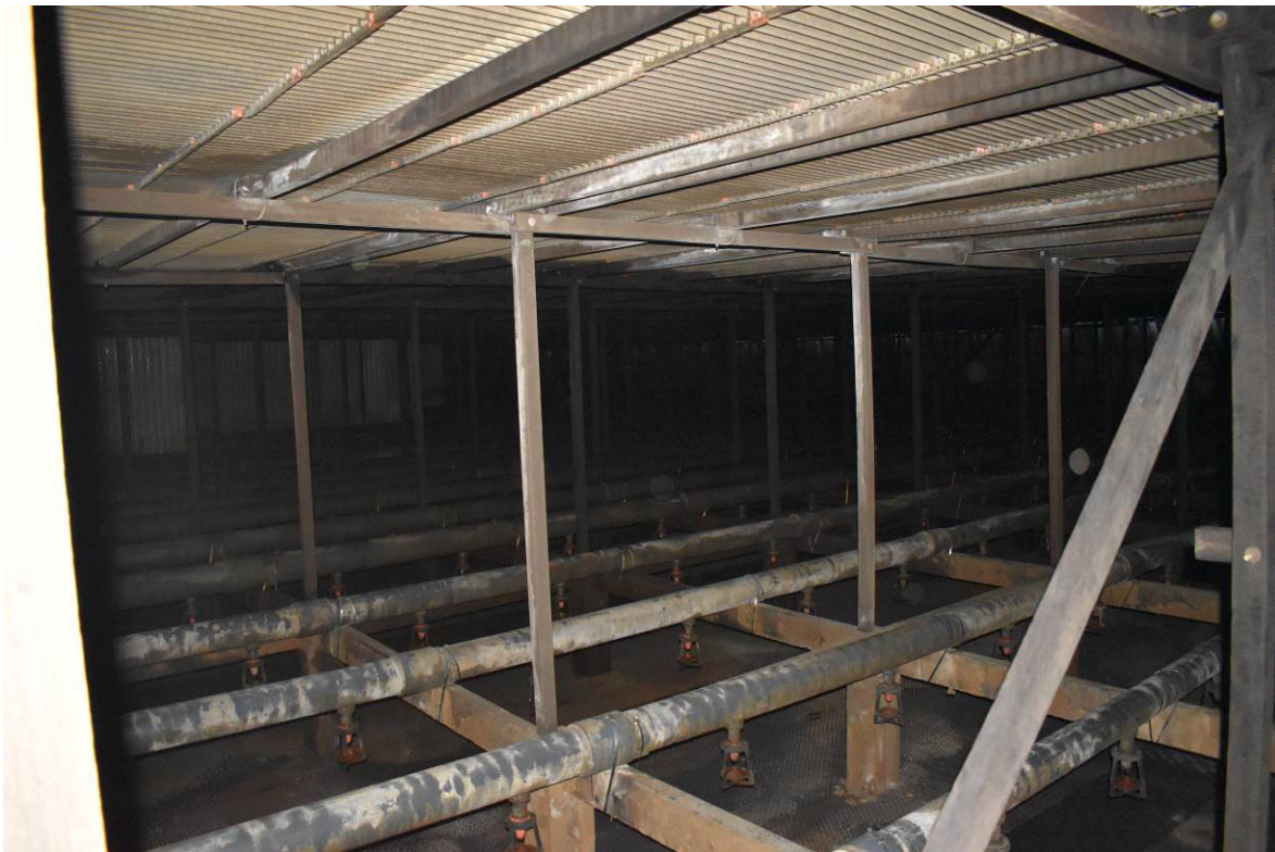
Plate 28: Distributor pipes supported on concrete beams above packing and below drift eliminator.
