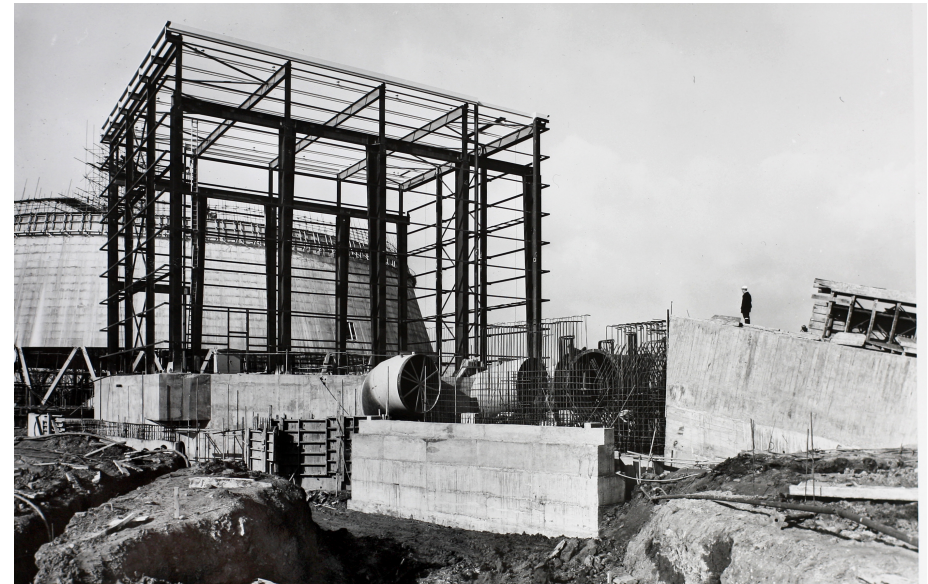
(b) CW pump house frame complete; CEGB photo ref. RAT.397, dated 15.10.1965.
