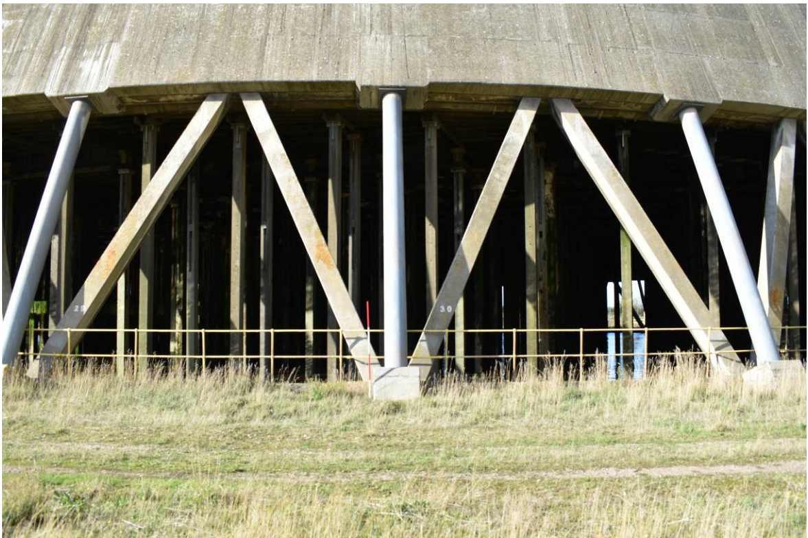
Plate 10: Primary V-strutting with secondary prop (1990) to air intake at base of cooling tower 2a.
