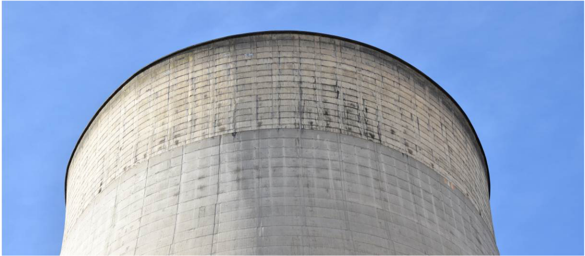
Plate 14: Head of cooling tower 2a with additional mantle (1990) to throat level.
