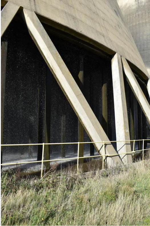
Plate 8: Detail of V-strutting to CT4a.
