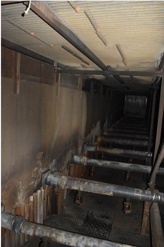
Plate 29: Distributor pipes opening off main culvert.
