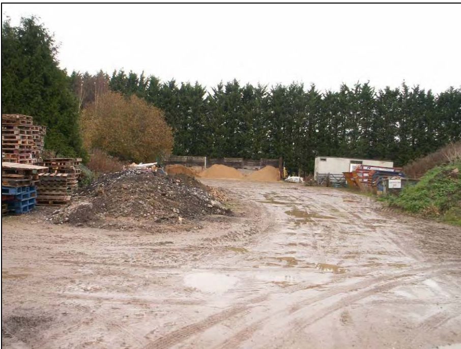
Photograph 4: Storage area for building materials, facing north.
