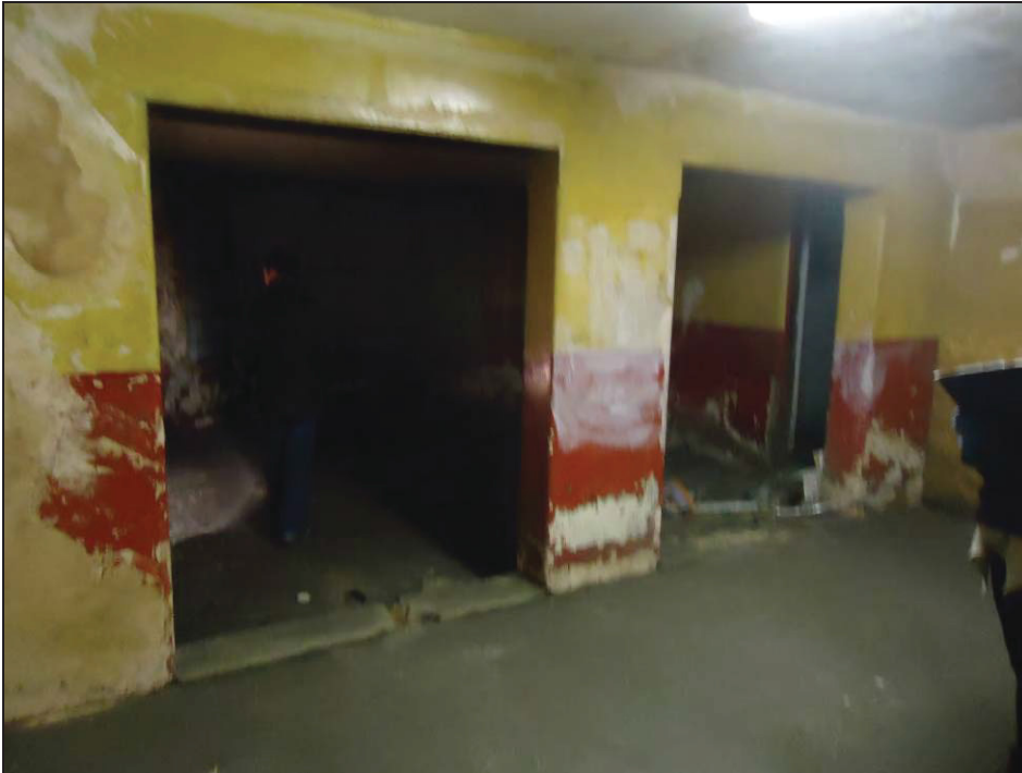
Photograph 5: Basement internally facing front of building (C. Mitchell, April 2013).
