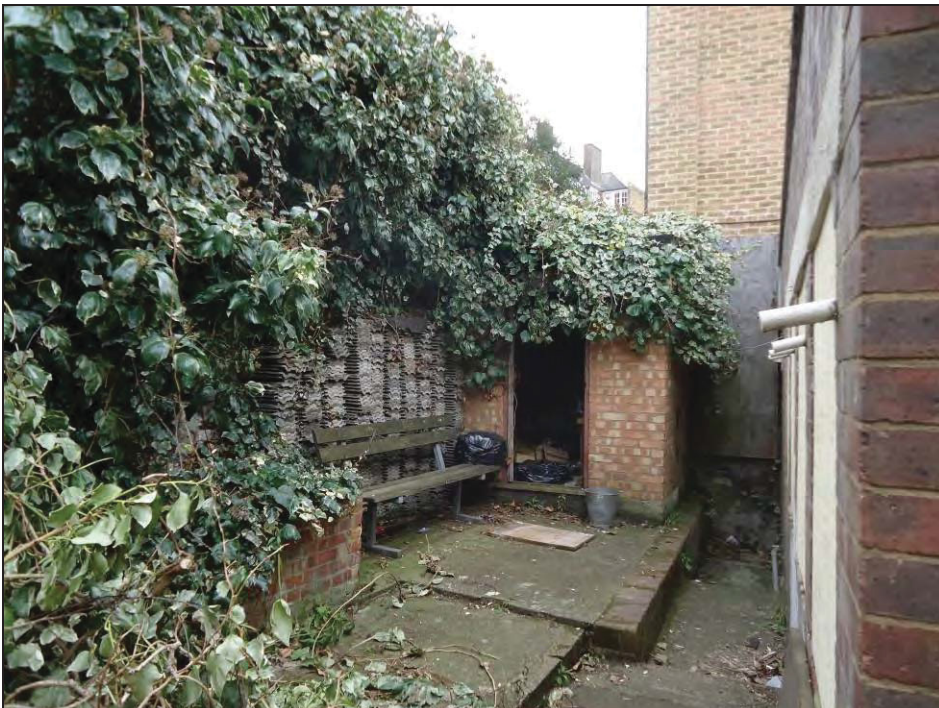
Photograph 2: Rear of property behind the toilet block (to be demolished) (C. Mitchell, April 2013).
