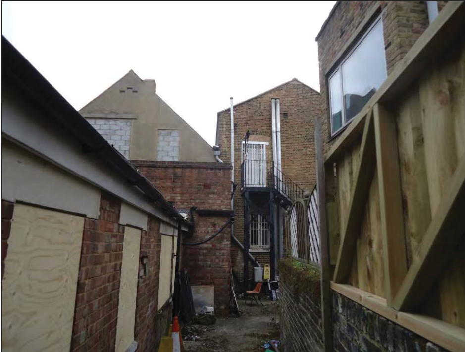
Photograph 3: Rear of property showing brick toilet block and concrete dance hall (to be demolished) (C. Mitchell, April 2013).
