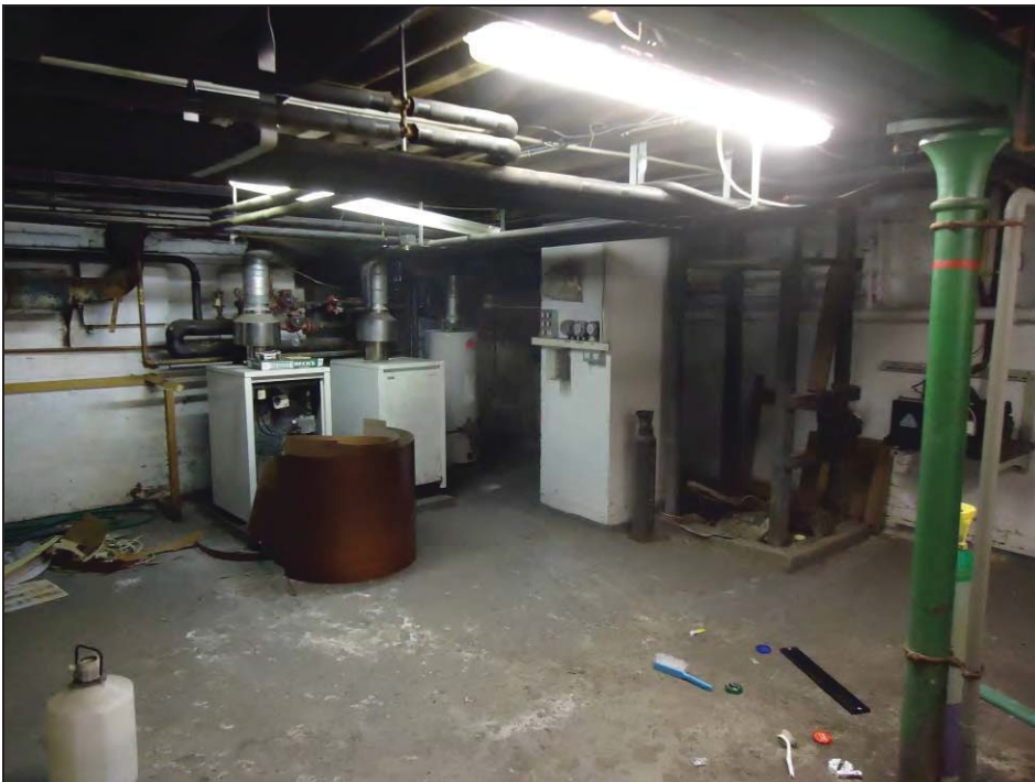
Photograph 6: Basement internally facing rear of building (C. Mitchell, April 2013).
