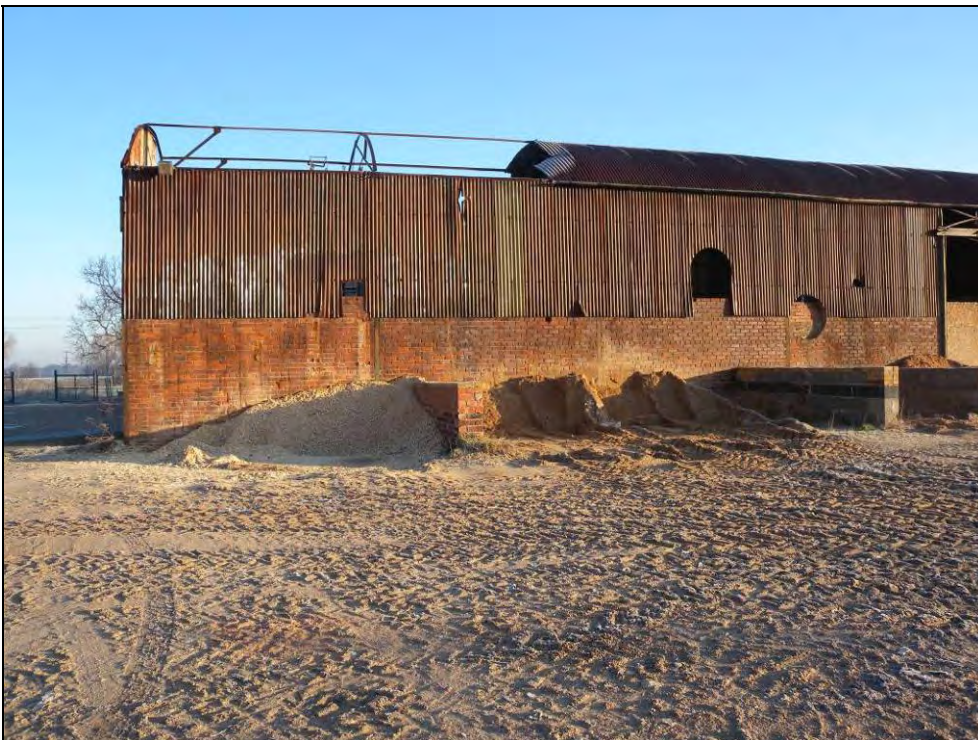
Photograph 7: Southern barn to the south-west of Grange Farm.
