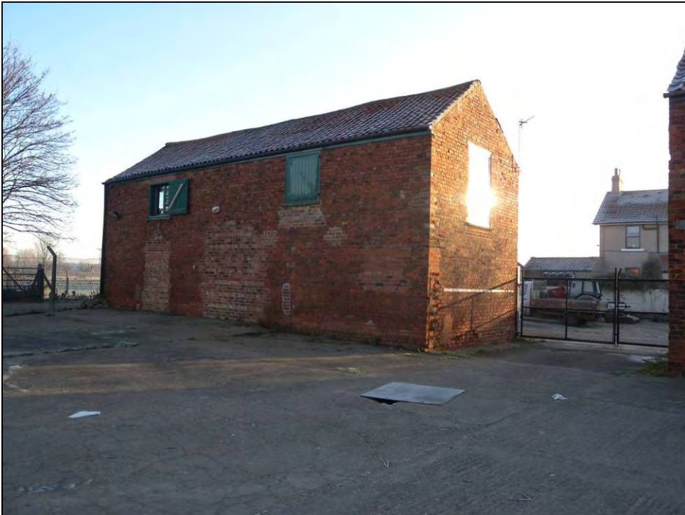
Photograph 5: Northern barn to the rear of Grange Farm.
