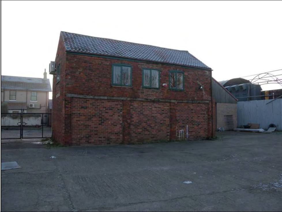
Photograph 6: Central barn to the rear of Grange Farm.
