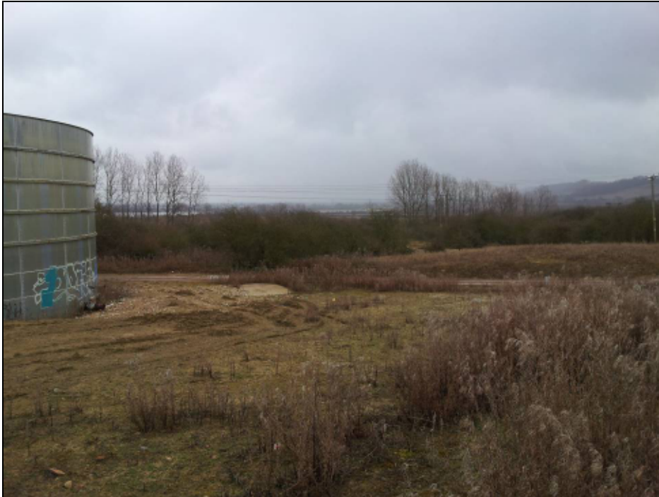
Photograph 1: Looking east with the existing tank on the left (Paul Russell, Cemex UK).
