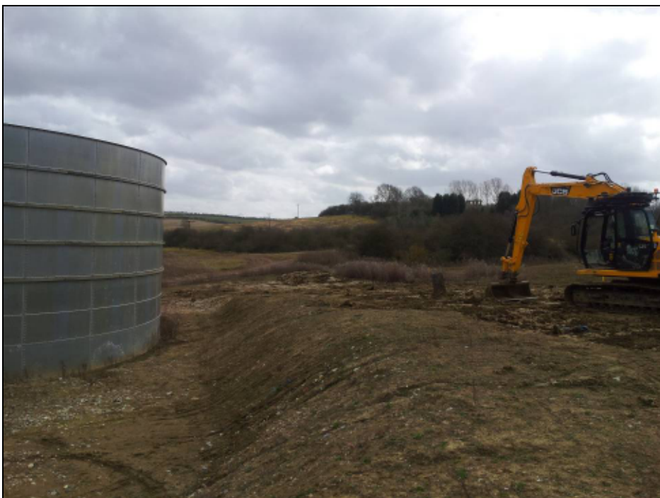
Photograph 2: Facing south with the derelict upper storeys of the Round House, Listed Building, visible on the horizon between the trees (Paul Russell, Cemex UK).
