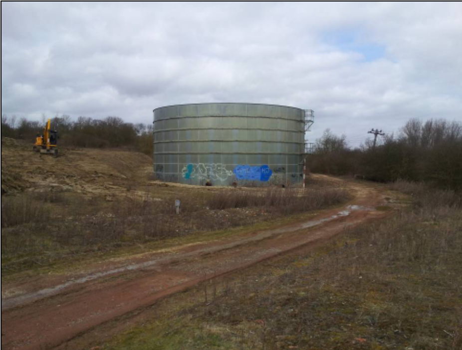
Photograph 3: Facing north with a view of the access track to the right of the tank (Paul Russell, Cemex UK).
