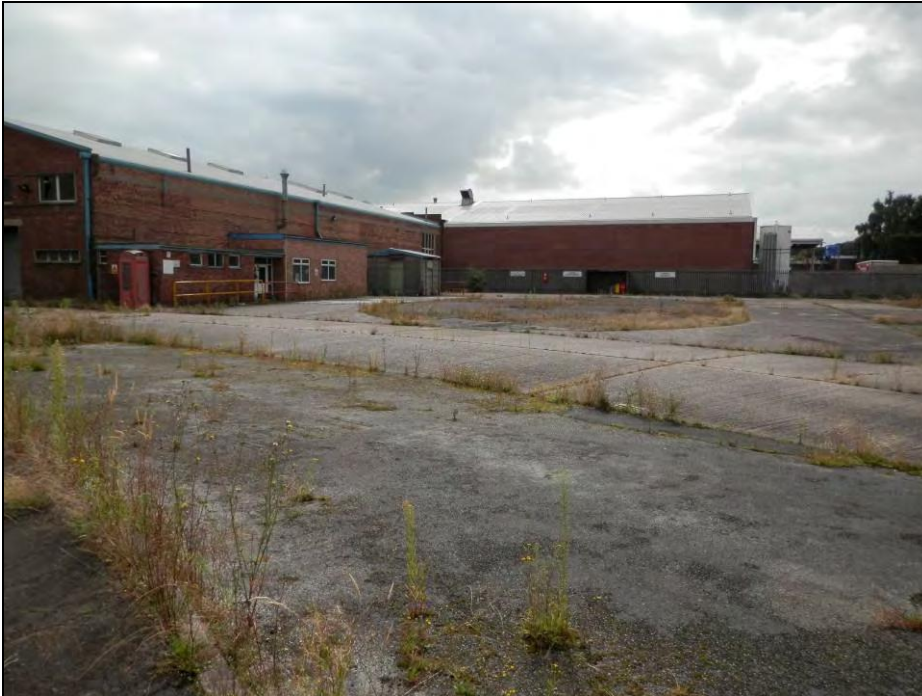
Photograph 1: Open yard area in west of site (southern half) facing south.
