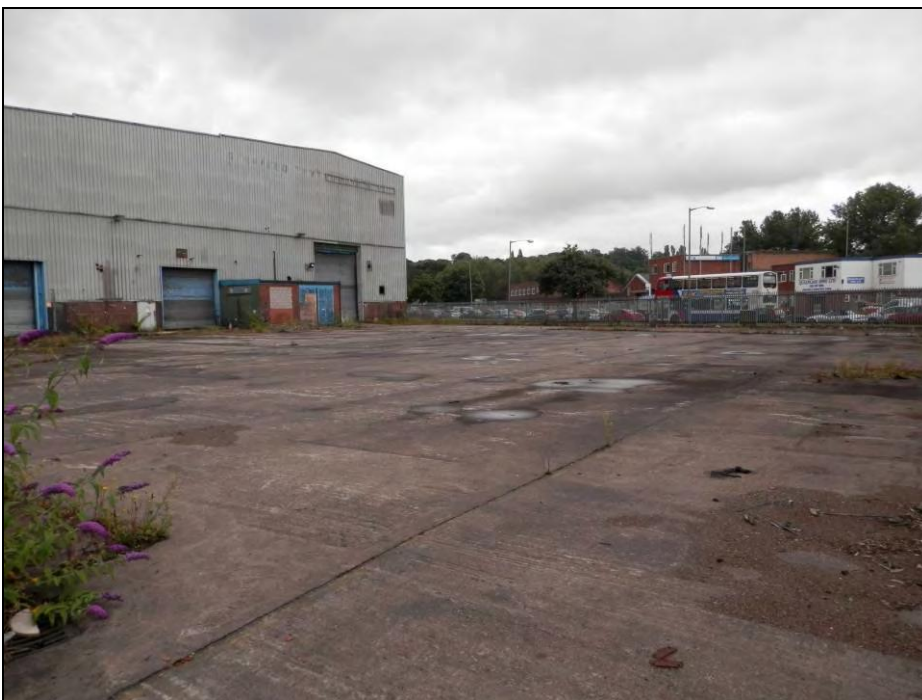
Photograph 2: Open yard area in west of site (northern half) facing west.
