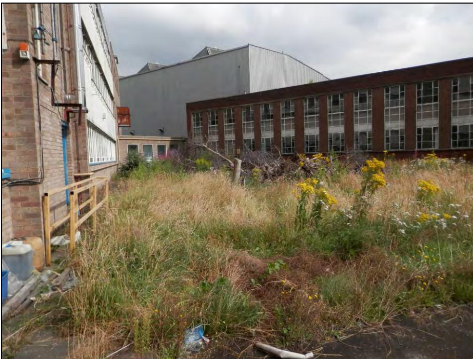
Photograph 10: Exterior of the office buildings and workshops with canteen and offices, facing north.
