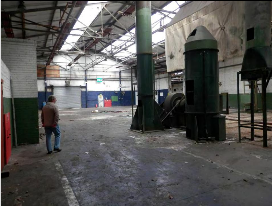
Photograph 5: Workshop with small furnaces, ovens and chimney still present.
