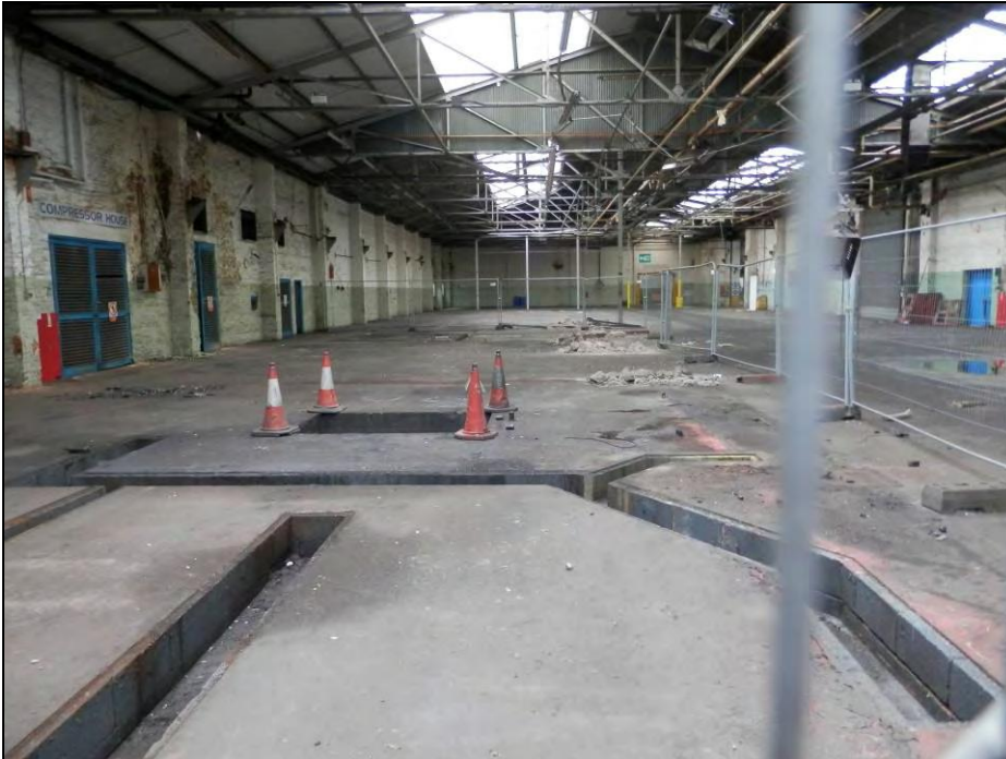
Photograph 7: Examples of small channels and pits within workshops.
