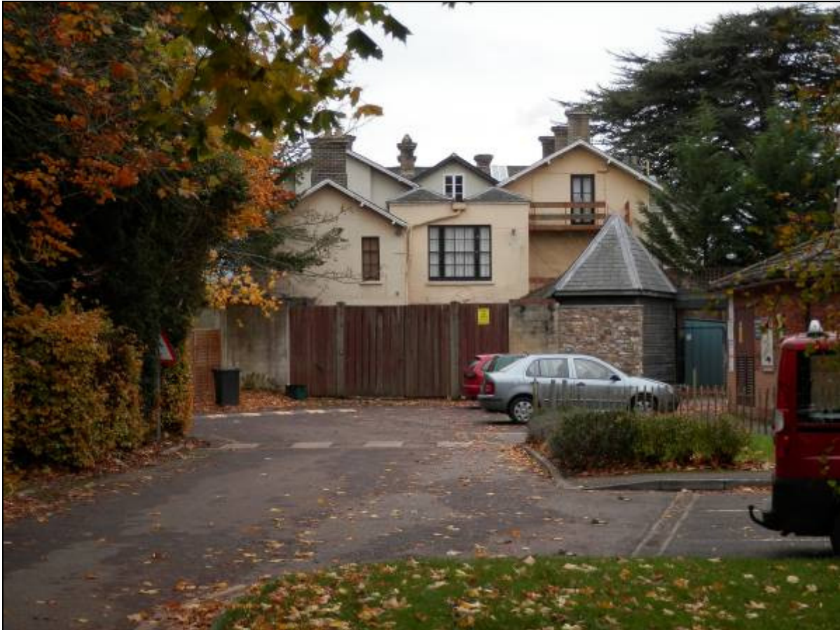
Photograph 9: View looking south showing access at rear of Canonsgrove House by the current entrance to the campus.
