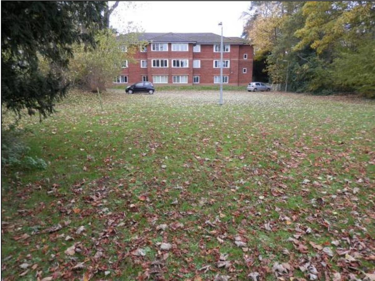
Photograph 7: View East across the car park from the western boundary of the site.
