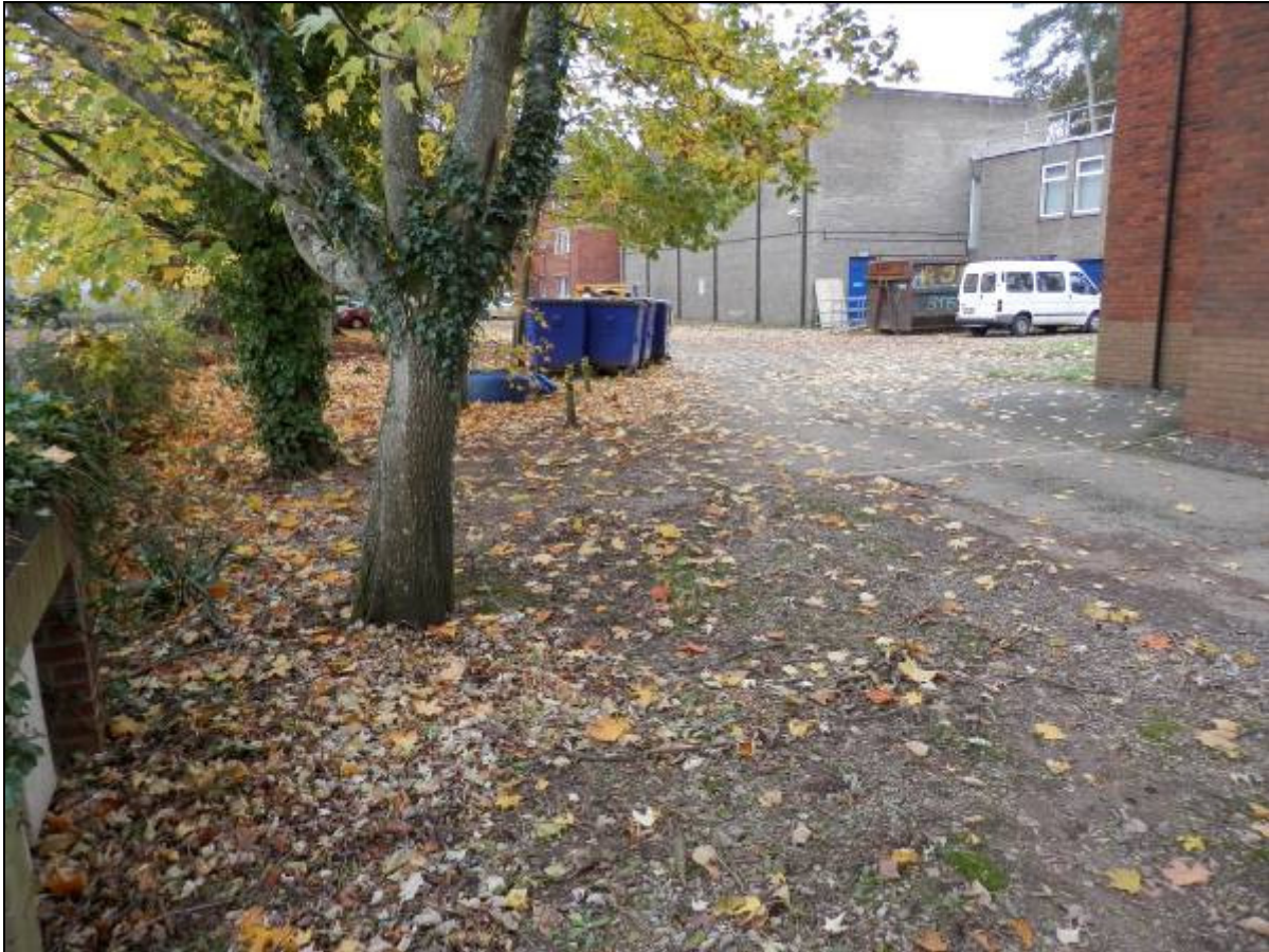
Photograph 8: View across the northern part of site showing buildings, infrastructure and planting.
