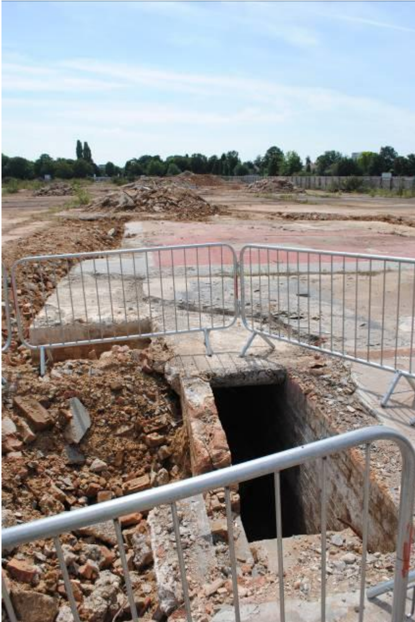
Photograph 13: View south showing eastern access stairs to Shelter 2.
