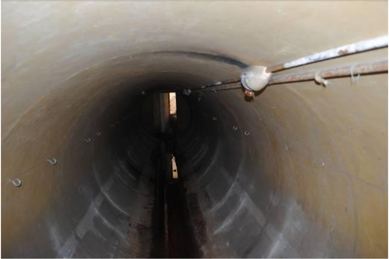
Photograph 4: South Gallery of Shelter 1.
