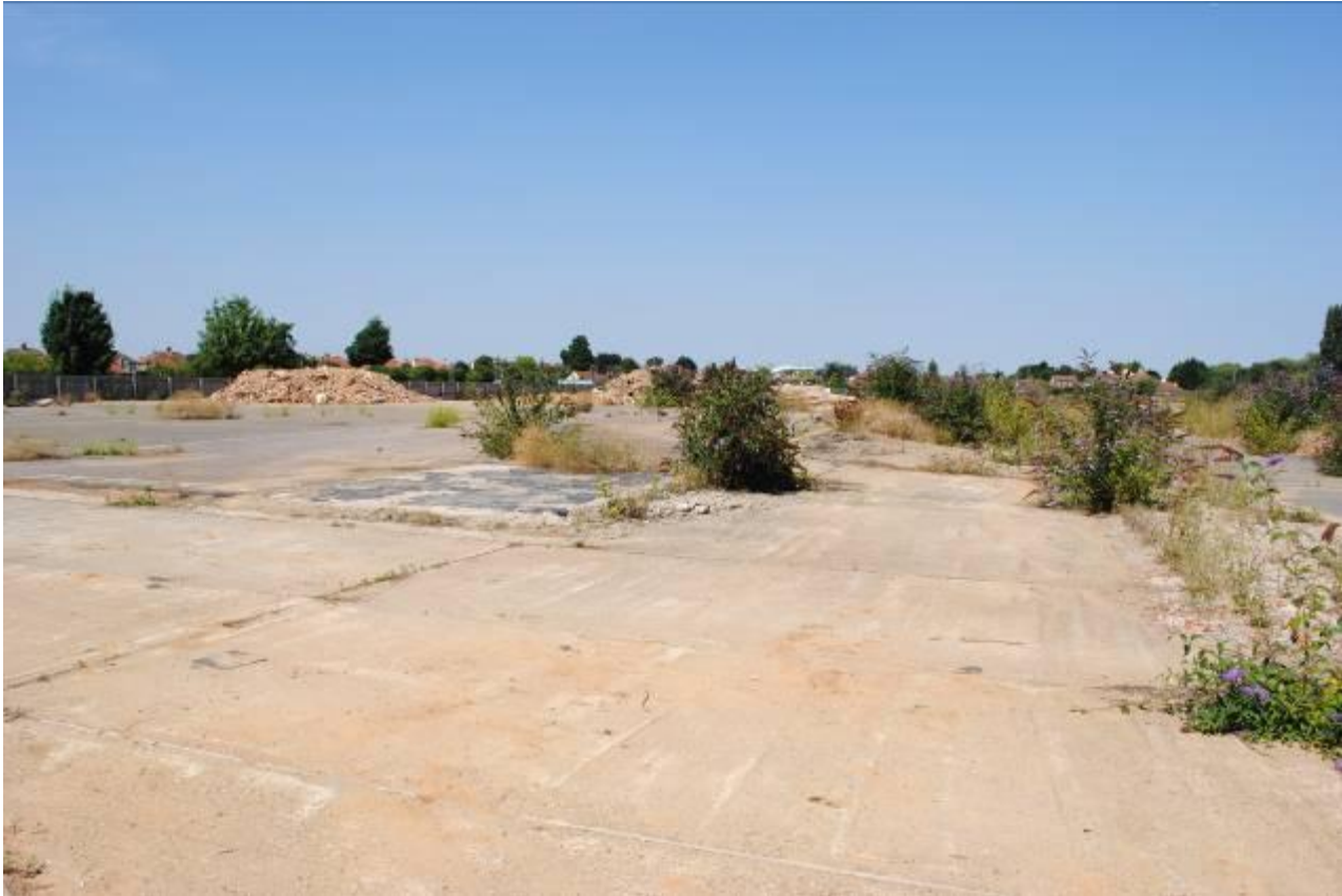
Photograph 2: General View North across the site, showing demolition of all buildings on the former Ekco Factory site.
