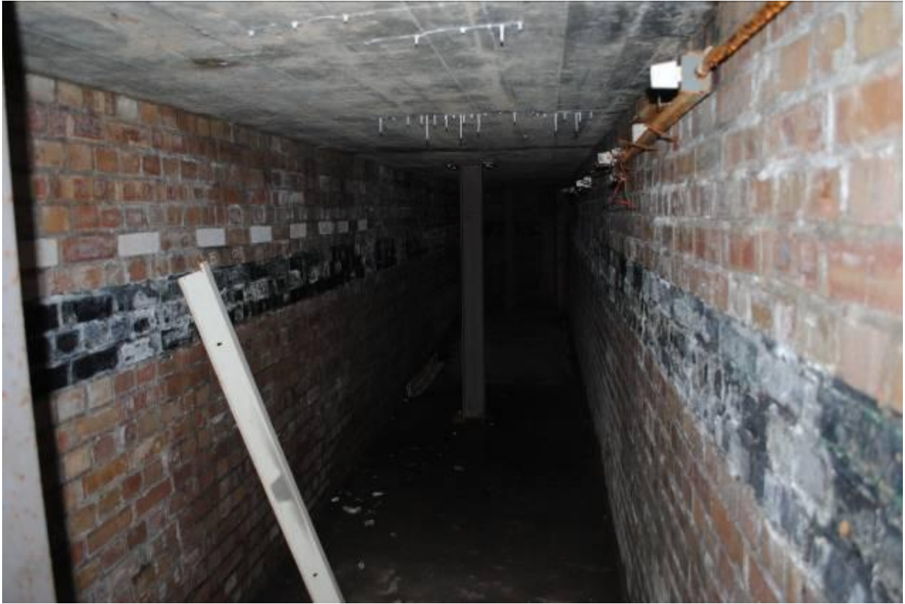
Photograph 14: Interior, east gallery of Shelter 2.
