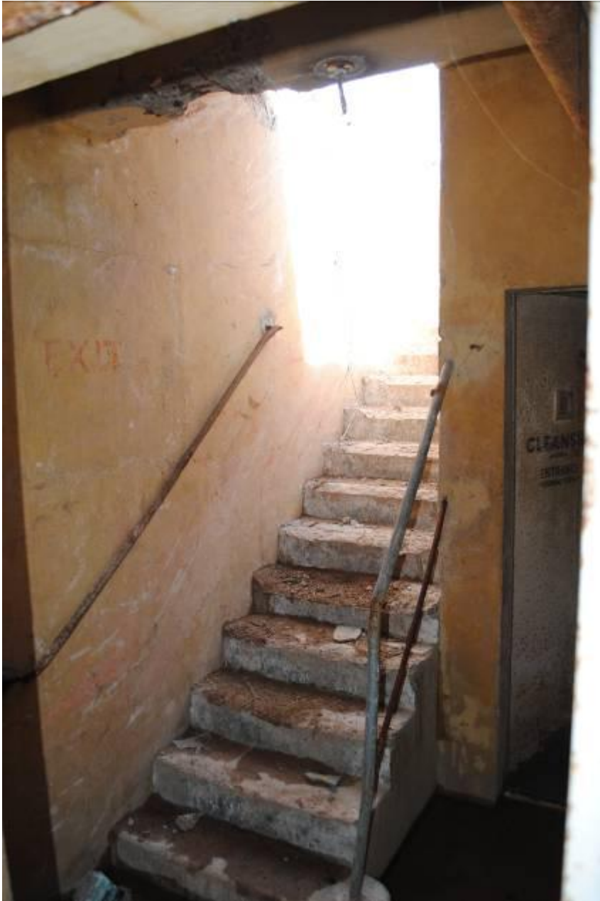
Photograph 11: North access to surface showing stencilled signage. The indicative cartoon hand remains visible to the right of the EXIT sign.
