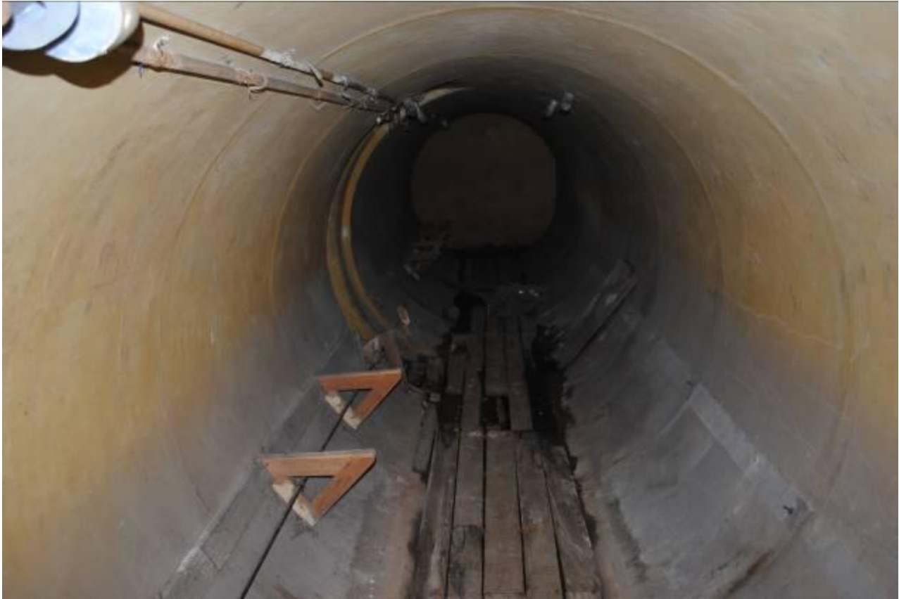
Photograph 6: View north along the Centre Gallery of Shelter 1 showing original Bakelite light fitting (top right), cable ducting, remnants of air filtration system (top centre), plank flooring and fitments for benches.
