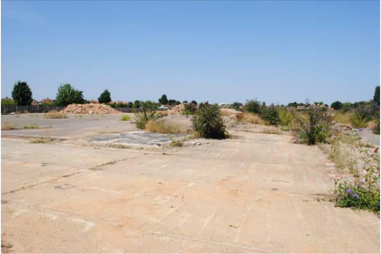
Photograph 2: General View North across the site, showing demolition of all buildings on the former Ekco Factory site.
