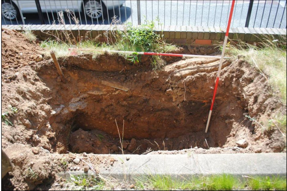
Picture 2: View of the works from the north during excavation.
