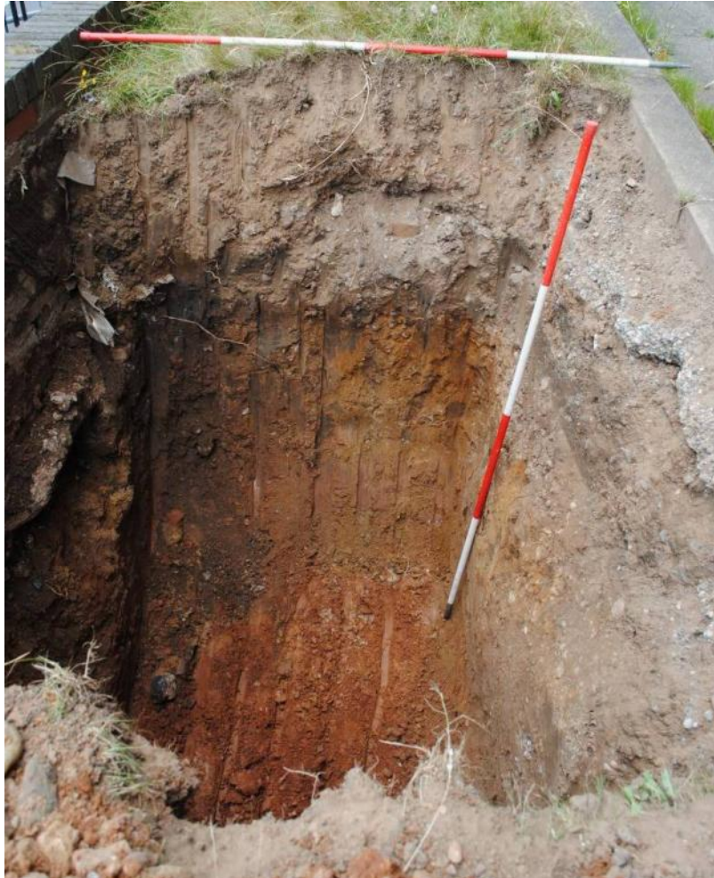
Picture 5: East-facing section showing the sequence of layers identified as well as structures of the paved pathway (004) and the boundary and retaining wall (005).
