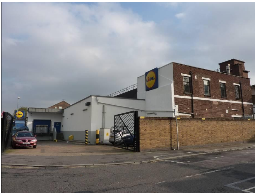
Photograph 6: 43-49 High Street, Walthamstow: view of side and rear from junction of Carisbrooke Road and Mission Grove.
