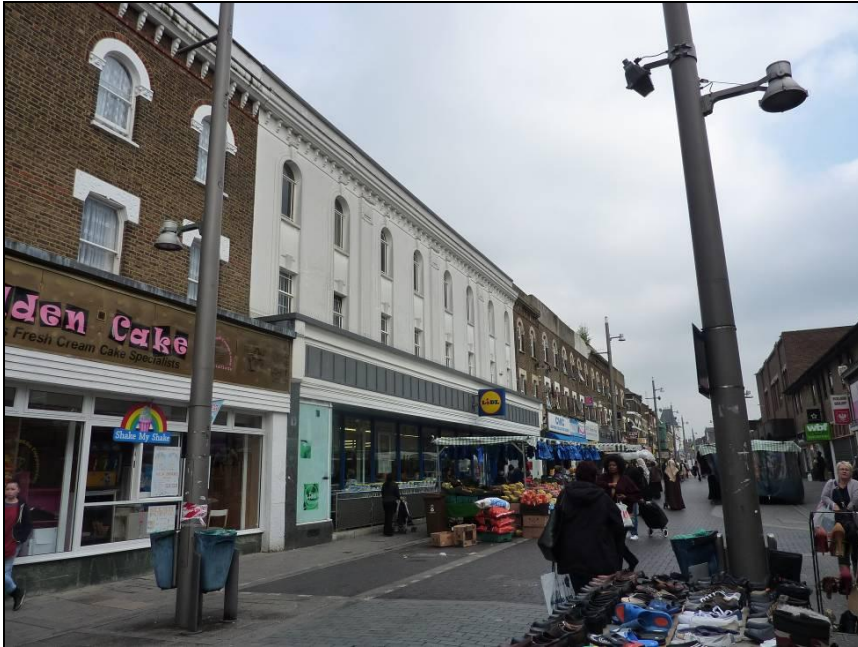
Photograph 1: 43-49 High Street, Walthamstow: view east towards Walthamstow Central from south side of High Street.
