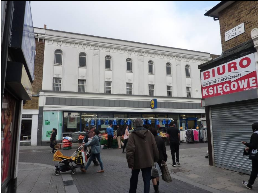
Photograph 3: 43-49 High Street, Walthamstow: view from northern end of Courtenay Place.
