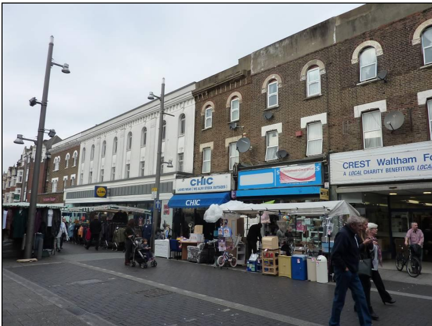
Photograph 2: 43-49 High Street, Walthamstow: view west towards St James Street from south side of High Street.
