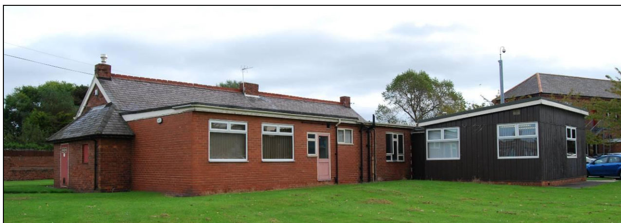
Plate 4: view from the northwest of the building facing southeast and showing detail of the exterior of the original WC and sink room with more modern plant room extension to the left, and two phases of modern office extension to the rear at the centre and right. The redbrick extension is of post-WWII date (1954), while the timber clad extension is of 1970s date.
