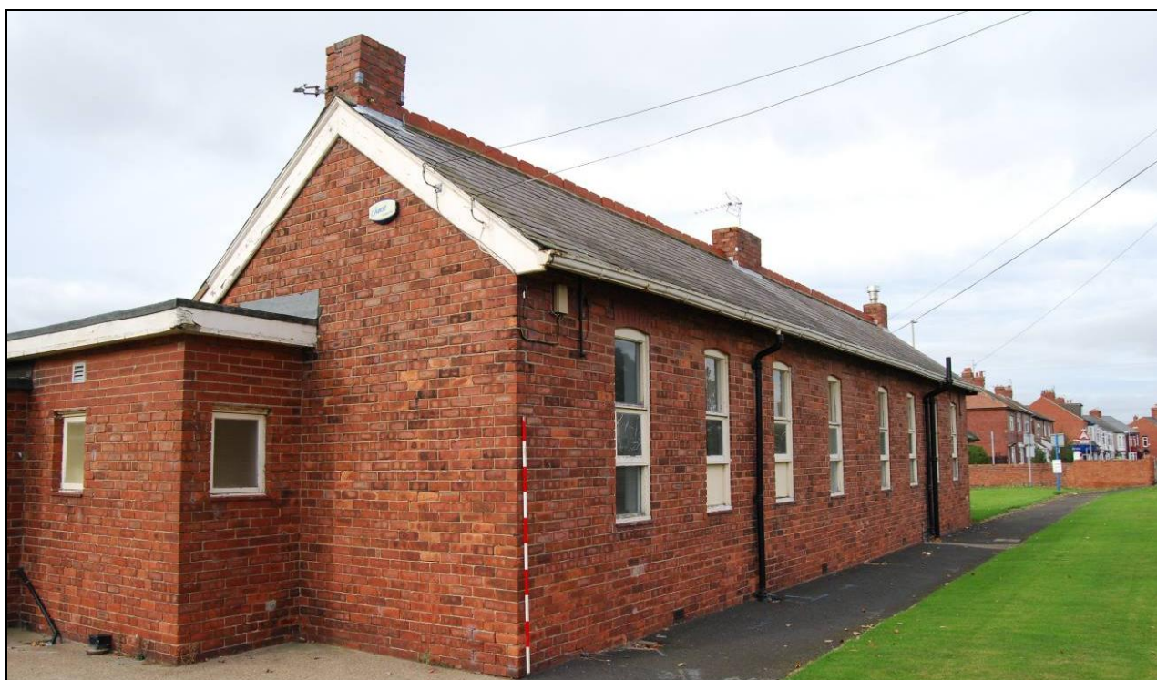
Plate 1: View from the southeast of the building, showing the northeast and southeast elevations, with original windows along the northeast facing wall, and original coal shed along the southeast facing gable (the windows are a later addition and the roof has been replaced in the past). The chimney stacks, main roof and ridge tiles are also original.
