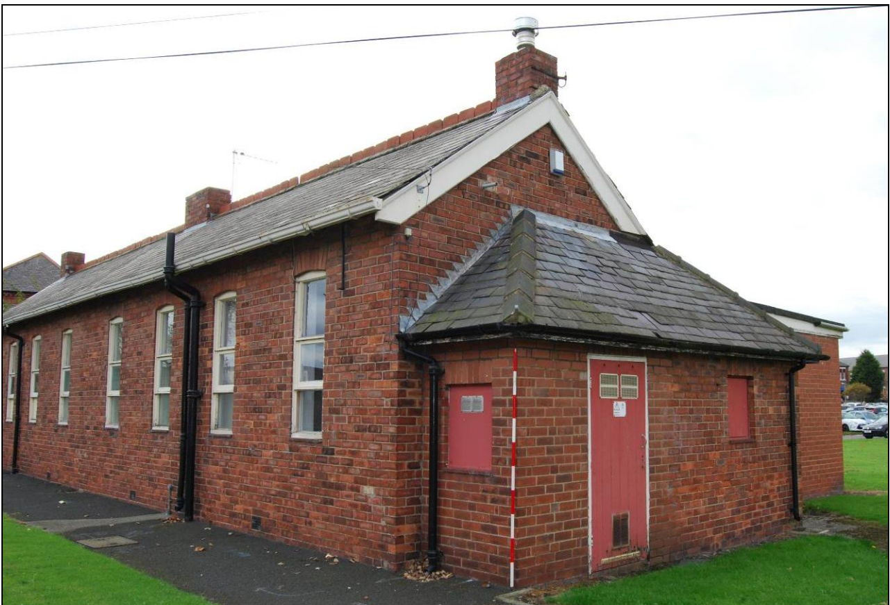
Plate 3: view from the northeast of the building facing southwest and showing detail of the exterior of the original WC and sink room with more modern plant room extension in the foreground and modern office extension to the rear. The original windows along the northeast elevation are visible. The junction between the original WC room and porch is apparent in the change in fabric.
