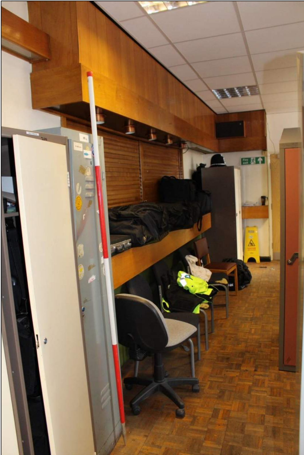
Photograph 42 – Interior of locker area Room S3.
