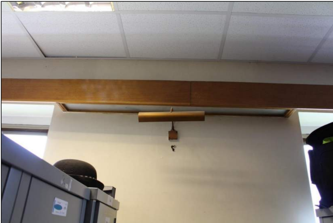
Photograph 41 – Detail shot of light fitting in locker area Room S3.
