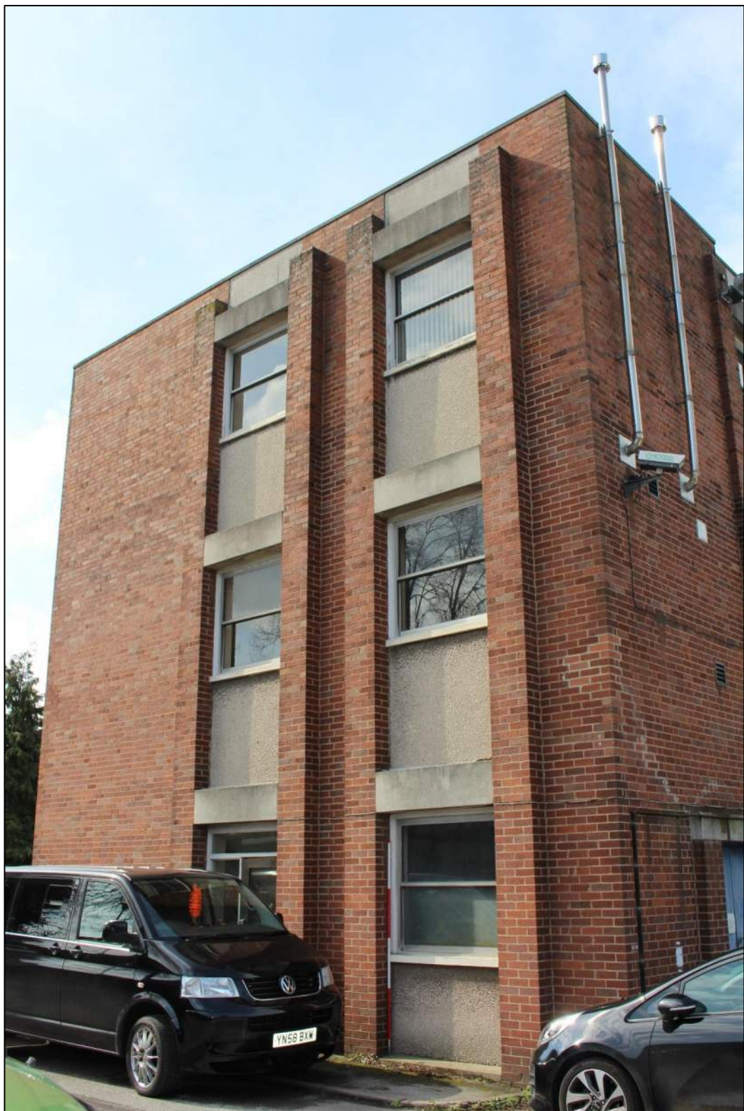
Photograph 11 – South-east short elevation of Lichfield Police Station.
