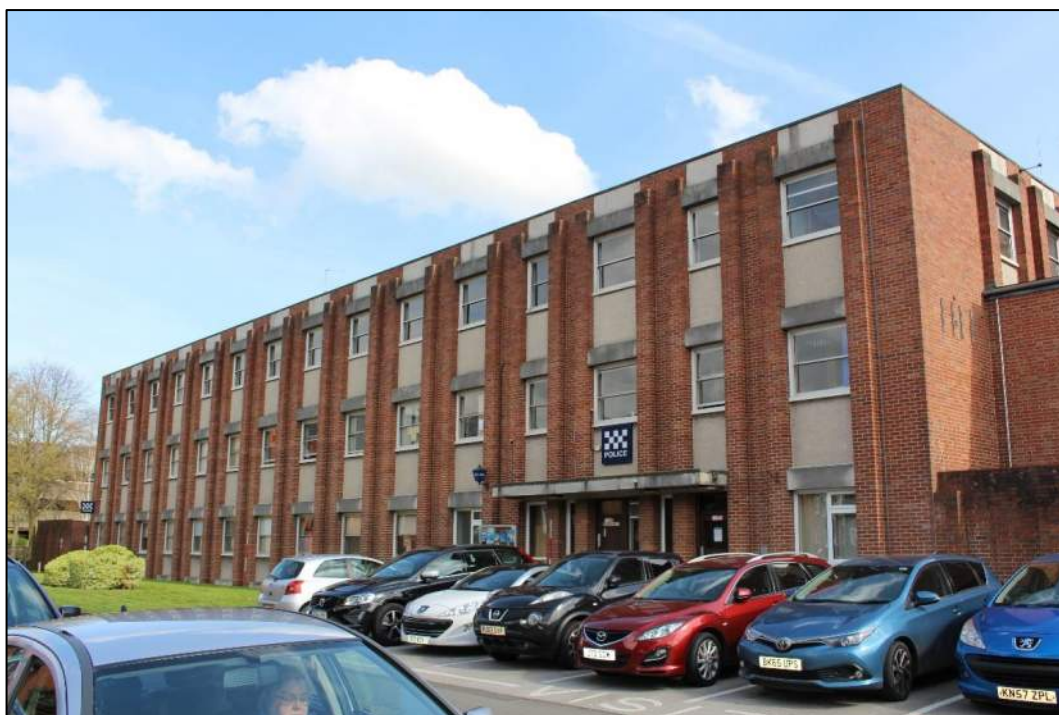
Photograph 2 – North-west elevation of Lichfield Police Station.
