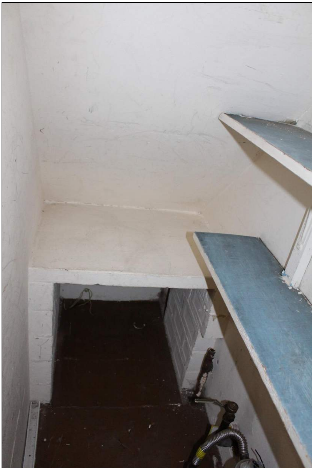
Photograph 56 – Under-stair larder for No. 20 Frog Lane.
