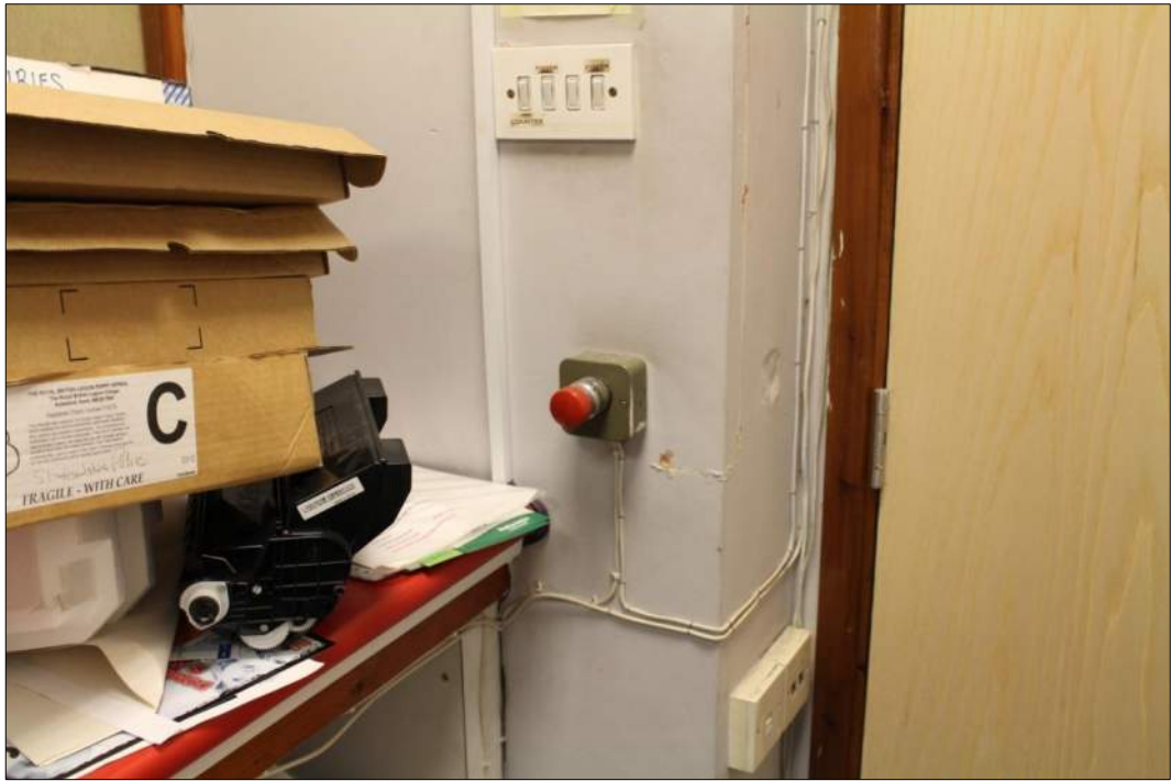
Photograph 20 – Room G3 detail of panic button next to the door in the north-east wall.
