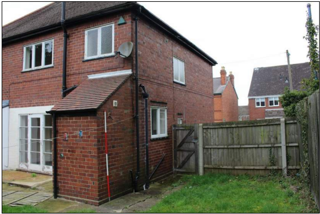
Photograph 51 – North-east elevation of No. 20 Frog Lane.
