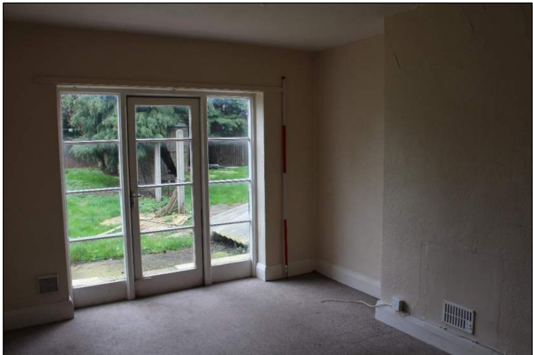
Photograph 54 – Ground floor back room of No. 20 Frog Lane, facing south.
