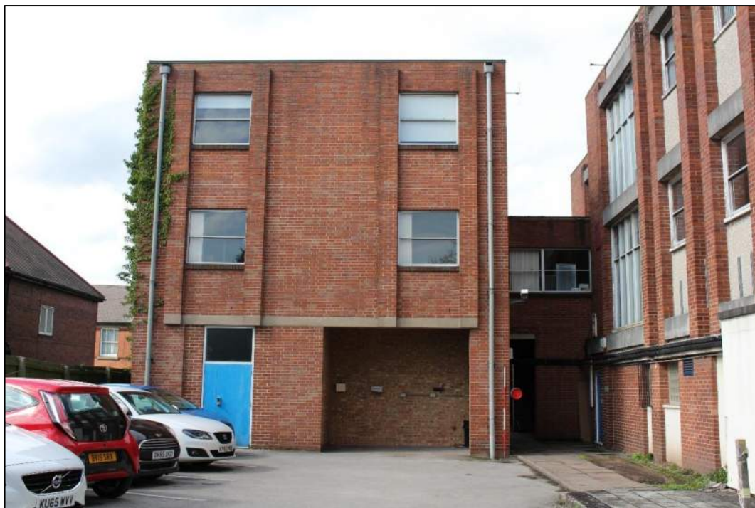
Photograph 16 – South-east elevation of Lichfield Police Station ancillary block.
