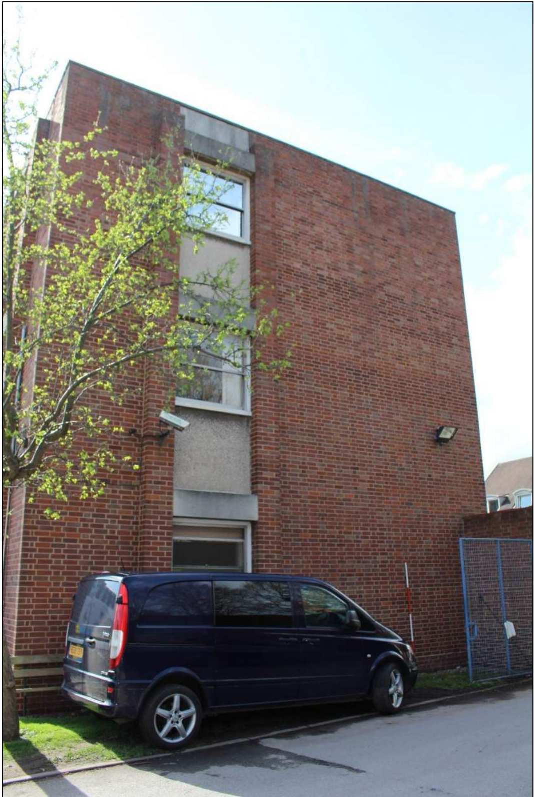
Photograph 8 – North-west short elevation of Lichfield Police Station.
