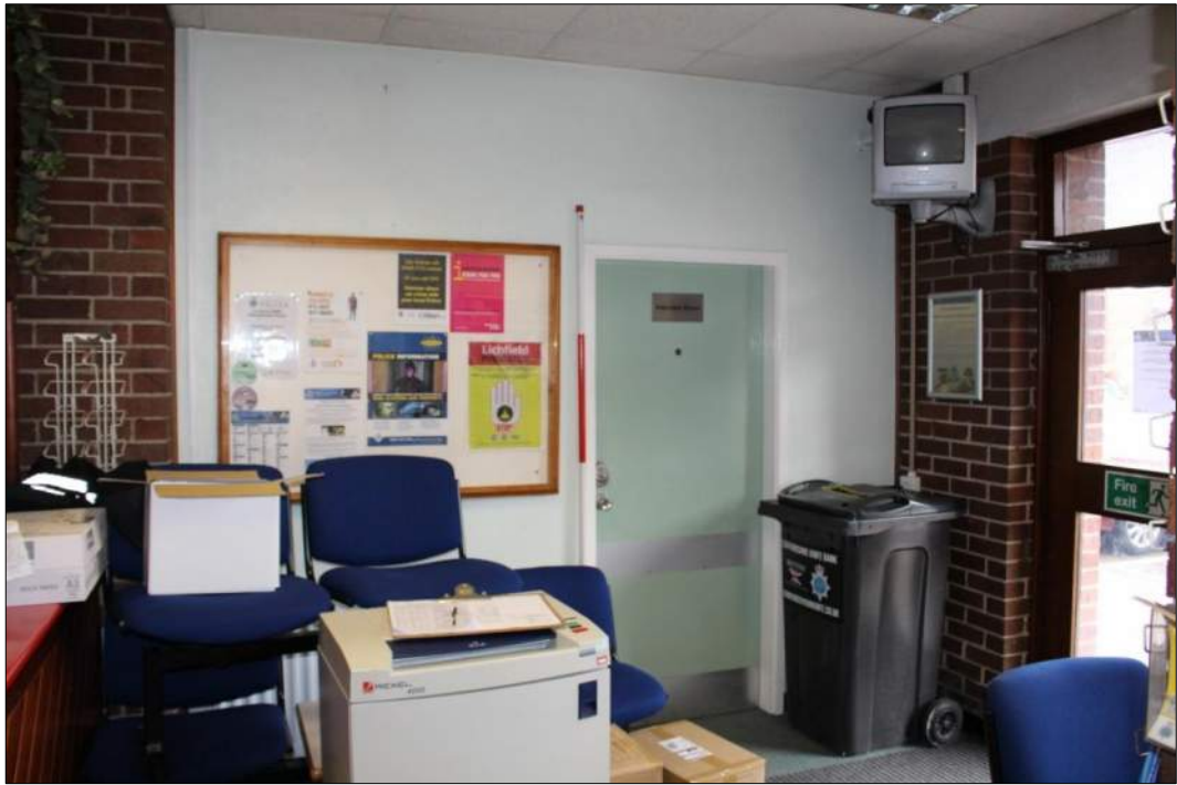
Photograph 18 – South-west wall of Room G1 showing door to the interview room.
