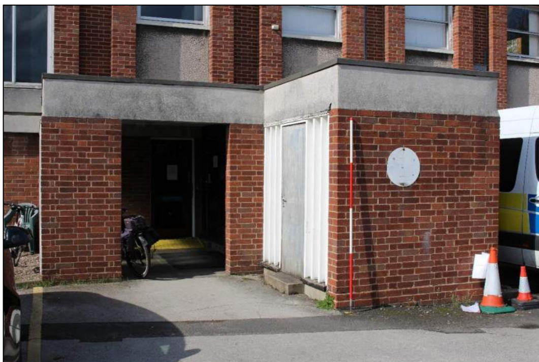
Photograph 13 – Ancillary structure abutting the south-east long elevation of Lichfield Police Station.
