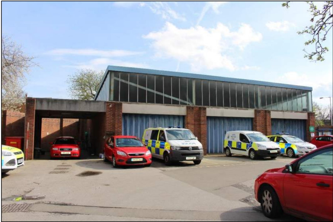
Photograph 4 – North-west elevation of Lichfield Police Station garage block.
