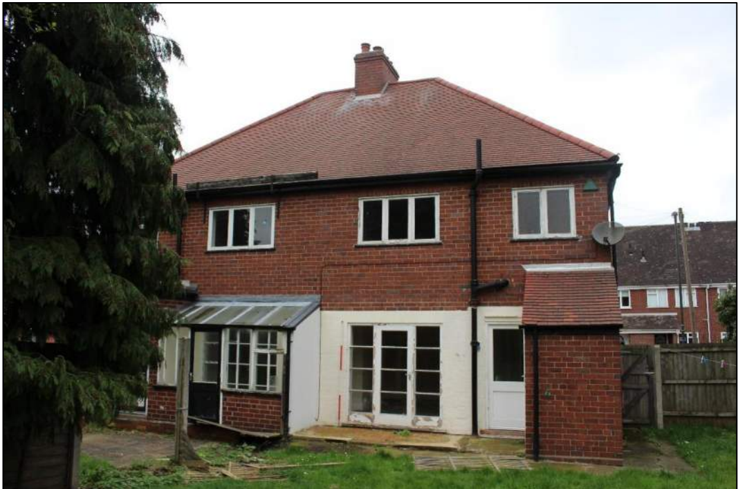
Photograph 48 – South-east elevation of Nos. 18 and 20 Frog Lane.
