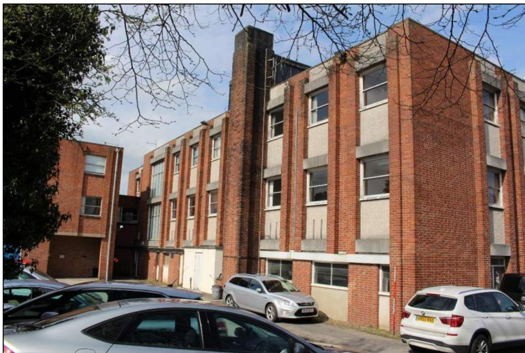
Photograph 14 – South-west elevation of Lichfield Police Station.
