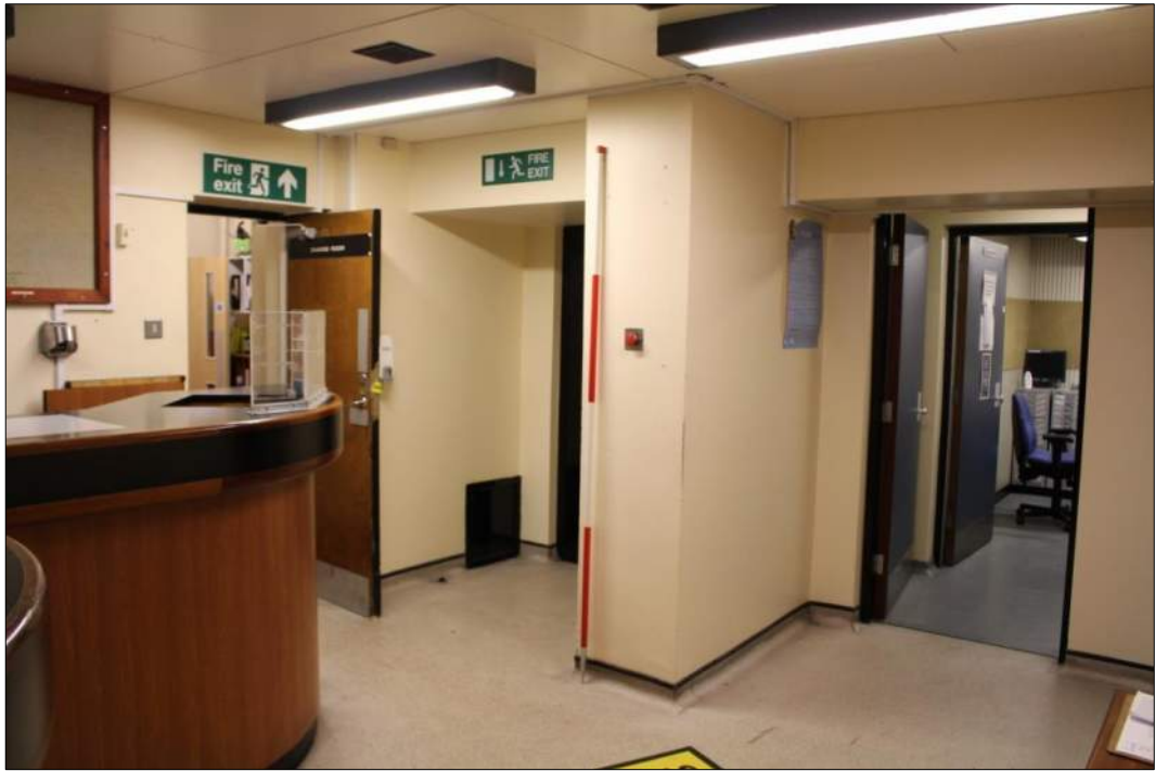
Photograph 22 – View north within Room G4. NB the panic button on the wall.
