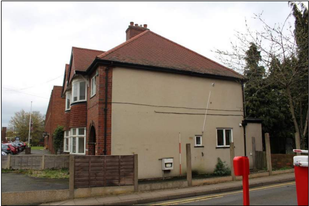
Photograph 47 – South-west elevation of No. 18 Frog Lane.
