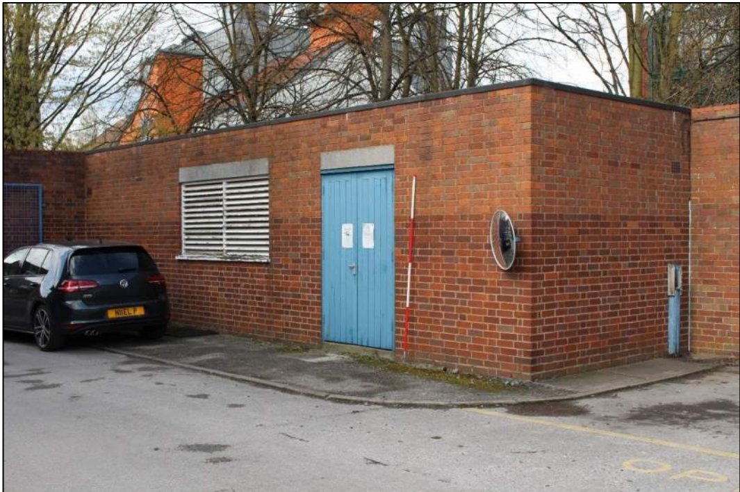
Photograph 5 – South-west elevation of Lichfield Police Station kennels.
