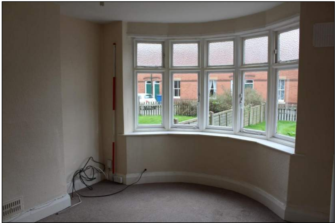
Photograph 53 – Ground floor front room of No. 20 Frog Lane, facing west.
