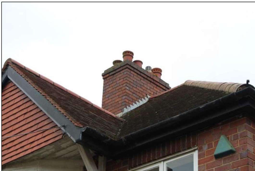
Photograph 44 – Detail shot of chimney stack of Nos. 18 and 20 Frog Lane.
