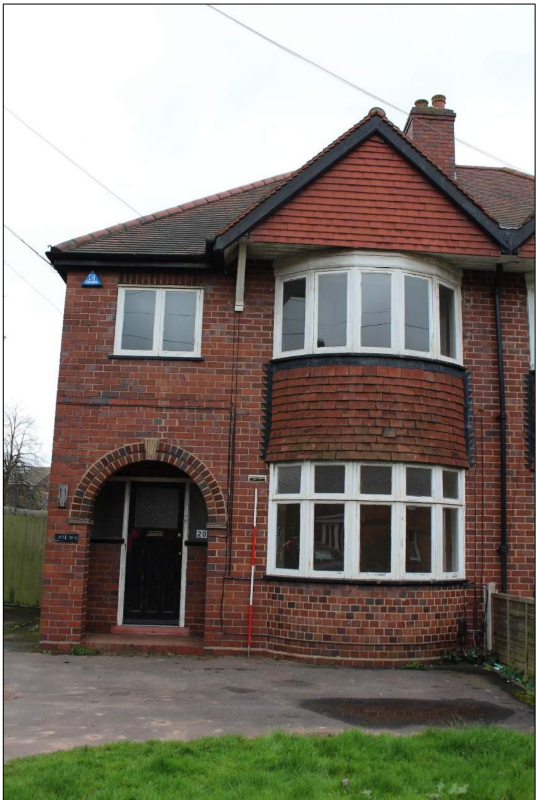
Photograph 46 – North-west elevation of No. 20 Frog Lane.
