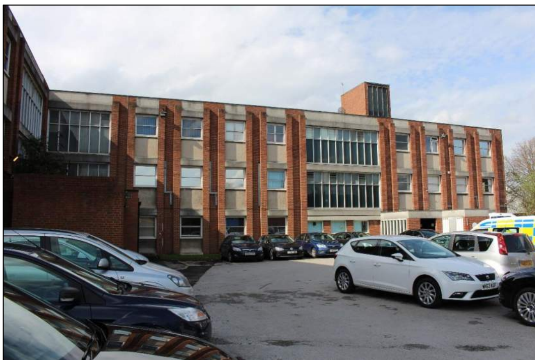
Photograph 12 – South-east long elevation of Lichfield Police Station
