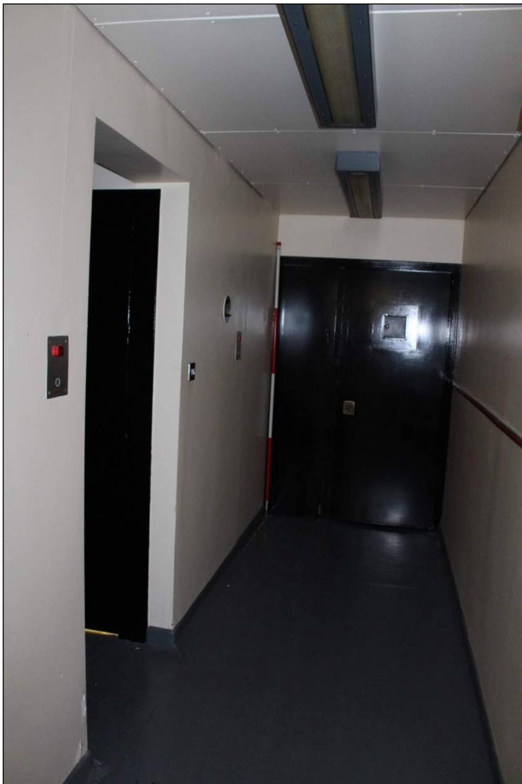
Photograph 27 – Cell block corridor (Room G6), Lichfield Police Station ground floor.
