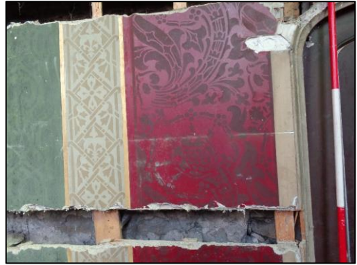
Plate 25. Various views of the chapel taken in 2014 after removal of the 20 th C squash court showing the revealed mid-19 th century decoration and the extent of the damage caused by the squash court. (bottom left), two views of a heater within a niche on the east wall and still in-situ. (below) a view in 2020 showing how the damaged decoration was conserved behind a new ventilated plasterboard wall.
