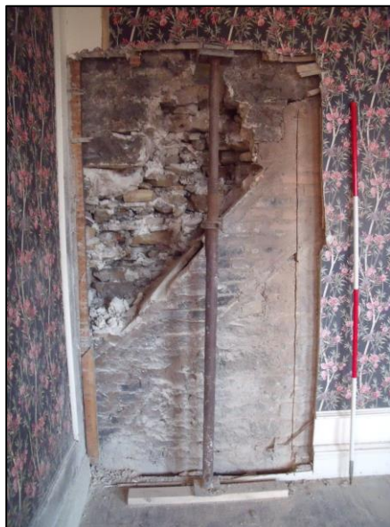
Plate 29. West wall of principal bedroom F6A showing revealed quoins of pre 18 th century hall east wall (shown on insert of Buck drawing of 1720, and later inserted flue for ground floor room G6a)
