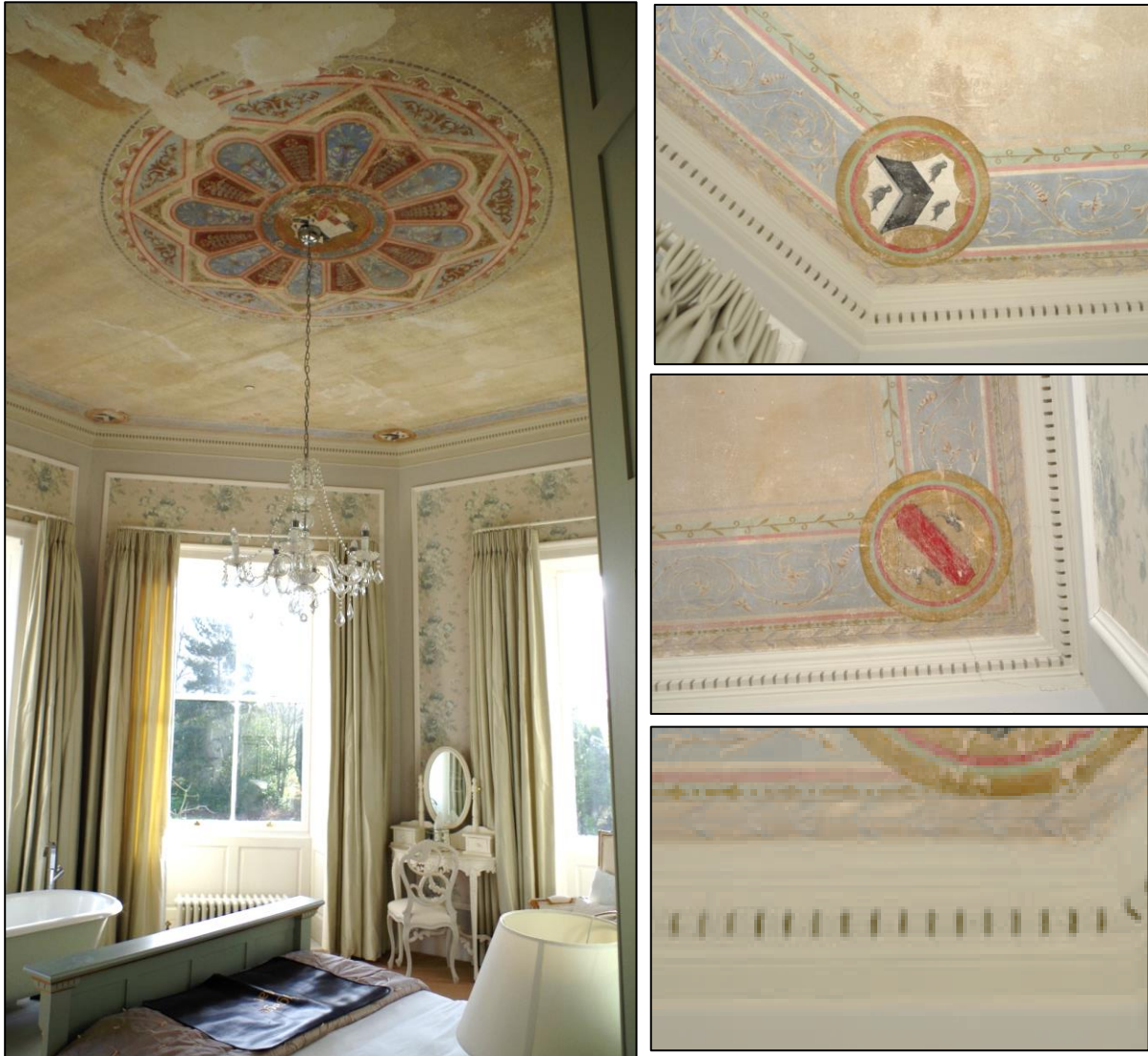
Plate 30. Room F6a looking south east (above left), showing the mid-19 th century painted ceiling revealed during restoration works. The scheme is likely to be of c.1859-63 during improvements by Msgr Witham and includes heraldic shields of related Catholic families who had previously owned the Hall. Prior to the building works this was covered by an early 20 th century wood chip wall paper.
