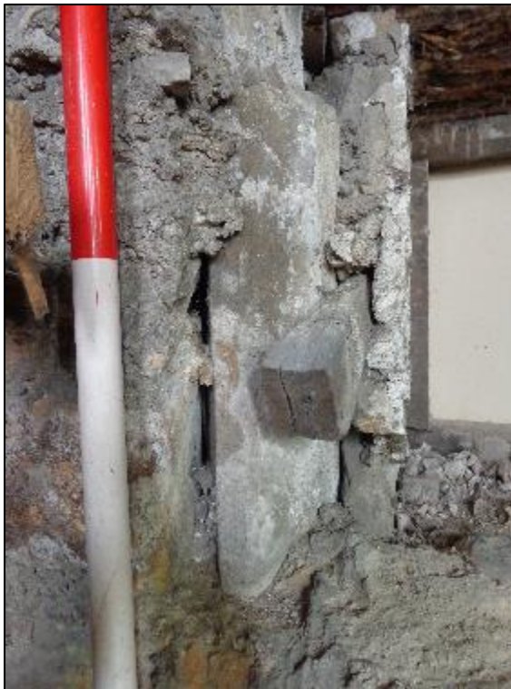
Plate 34. (above) 17 th C mullion & transom window on the entrance tower previously concealed by the sundial dated 1641 (top left). The central transom is identical in form to that exposed in the east wall of the Chapel, the former west wall of the Hall (left)
