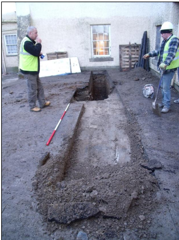
Plate 11. Trench 2, (above), looking south towards north wall of the Hall; and (right) showing the insubstantial depth and size of the foundation of the Hall's north wall.
