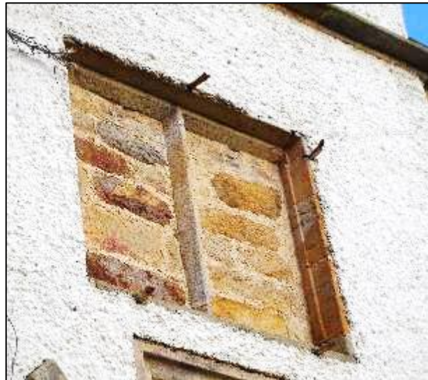
Plate 34. (above) 17 th C mullion & transom window on the entrance tower previously concealed by the sundial dated 1641 (top left). The central transom is identical in form to that exposed in the east wall of the Chapel, the former west wall of the Hall (left)
