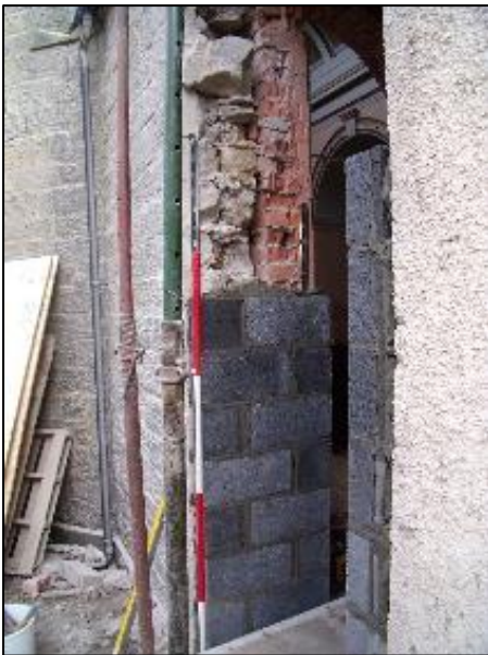
Plate 4 (4a above left), Looking north-east at the outside west wall of the Grand Corridor constructed in 1861-3 showing new opening to access the new toilet block. (4b above right), Opening up works for the new entrance seen from the inside and (5c far left), outside wall at the same point showing brick internal construction with outside facing in sandstone.
