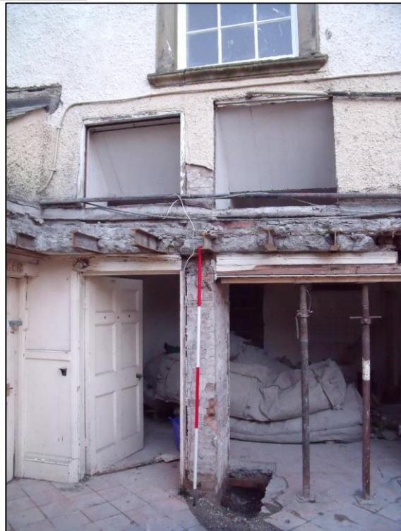
Plate 7 a, b (above). Demolition of mid-19 th century and later single storey buildings looking south east and south. While the rear of the structure used steel joists to support a concrete roof and appears 20 th century (above right), the mostly northerly elements (see above left) were of stone rubble and lime mortar construction beneath a modern render. The Grand Corridor of 1861/3 had been built around the east end of the north wall of this building and so must post date it. It therefore seems likely this small part of the structure was a part of the early post-1800 service buildings and kitchen range.
