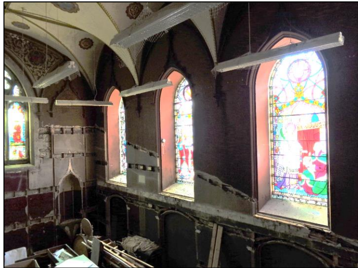
Plate 26. 19 th century stained glass revealed by the removal of the squash court structure in the chapels west wall (above from south to north) and above the altar at the south end (left). The angled scar left by the squash court can be seen in the view looking SW from the balcony (below)
