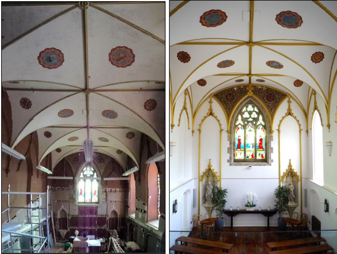
Plate 27. The Chapel room G8, looking south from the balcony at the north end. (above left) in 2014 following removal of the late 20 th century squash court; (above right) after building and conservation work in 2020.
