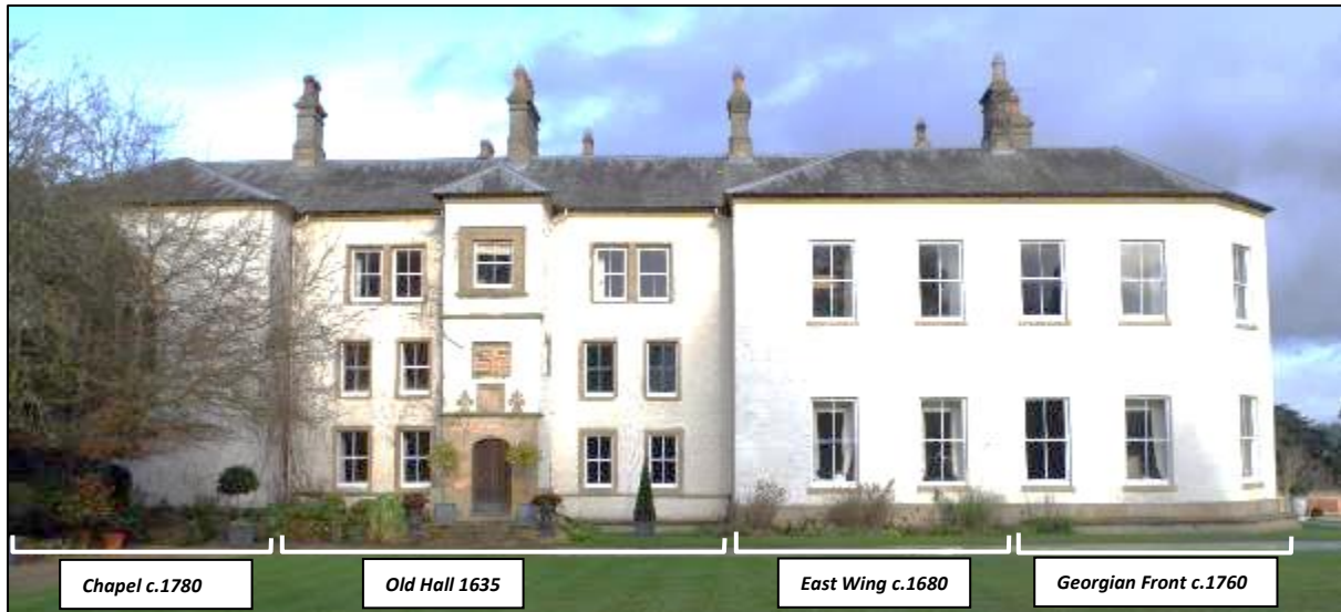
Plate 36. The South elevation of Lartington Hall in 2020 at the completion of works showing phases of construction and extension. Comparison with the Samuel Buck drawing of 1720 (below) also shows how as well as the extensions, the roofline of the Hall has also been altered to a shallower pitch without dormers the whole being unified by a moulded sandstone course running around the whole of south and east elevations. This seems likely to have been part of the significant Georgian work of c.1760 which altered the principal elevation of the Hall from the south to the east to look over the newly laid out landscape parkland.
