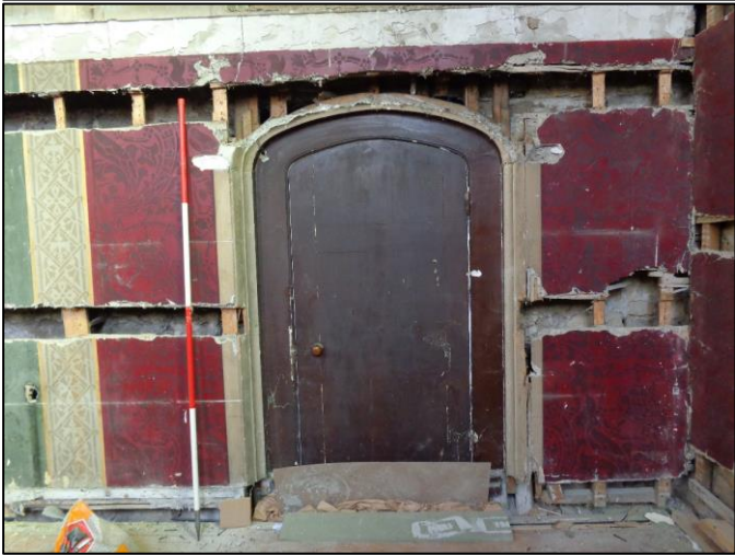
Plate 25. Various views of the chapel taken in 2014 after removal of the 20 th C squash court showing the revealed mid-19 th century decoration and the extent of the damage caused by the squash court. (bottom left), two views of a heater within a niche on the east wall and still in-situ. (below) a view in 2020 showing how the damaged decoration was conserved behind a new ventilated plasterboard wall.
