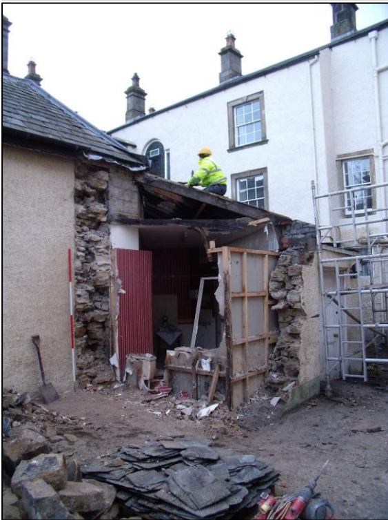
Plate 7 a, b (above). Demolition of mid-19 th century and later single storey buildings looking south east and south. While the rear of the structure used steel joists to support a concrete roof and appears 20 th century (above right), the mostly northerly elements (see above left) were of stone rubble and lime mortar construction beneath a modern render. The Grand Corridor of 1861/3 had been built around the east end of the north wall of this building and so must post date it. It therefore seems likely this small part of the structure was a part of the early post-1800 service buildings and kitchen range.
