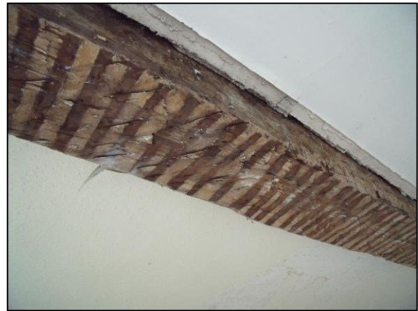
Plate 28 Room G9, formerly a principal room of the 17 th C Hall. (Clockwise from top left) looking SE showing floor scar left by removal of the later N-S partition wall, with 19 th C encaustic tile floor to the east. (Above right), detail of the encaustic tile floor. (Right) scars from earlier lathe and plaster to the central supporting beam. (below right) view of room in 2012 prior to building works looking SW showing 18 th C fireplace and steps to the chapel (Below left) view of the room in 2020 after building works.
