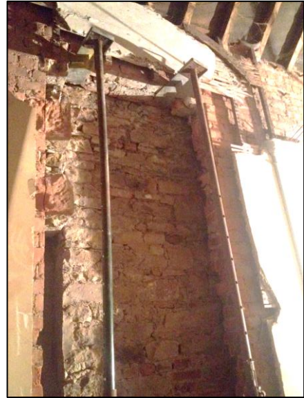
Plate 4 (4a above left), Looking north-east at the outside west wall of the Grand Corridor constructed in 1861-3 showing new opening to access the new toilet block. (4b above right), Opening up works for the new entrance seen from the inside and (5c far left), outside wall at the same point showing brick internal construction with outside facing in sandstone.
