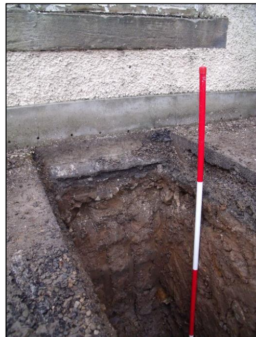
Plate 11. Trench 2, (above), looking south towards north wall of the Hall; and (right) showing the insubstantial depth and size of the foundation of the Hall's north wall.
