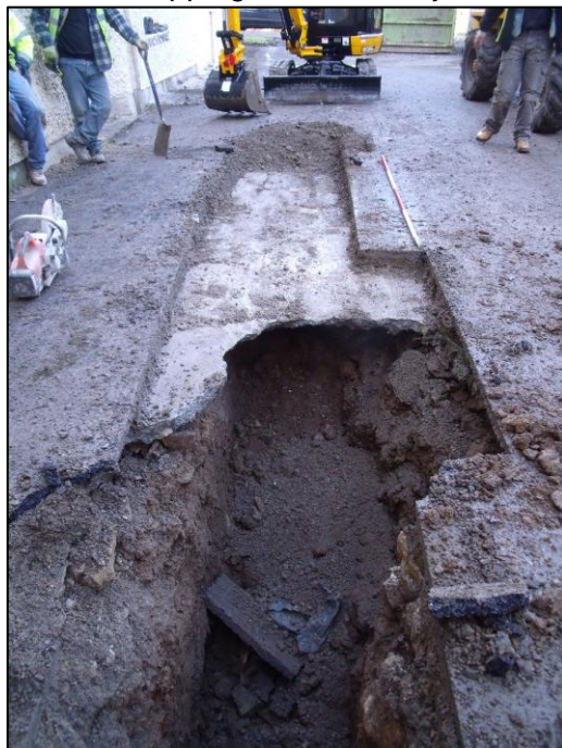
Plate 9. Trench 2, looking north with surface partially removed showing the loose and unstable material beneath the tarmac and concrete courtyard surface.
