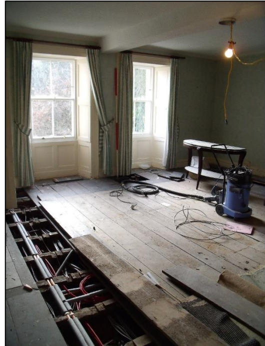
Plate 33. (above right) room F9 during building works in 2012 looking SW and showing how modern wiring and services were accommodated. (above left) the same room and view following conservation works in 2020.
