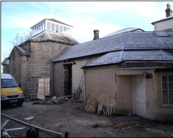
Plate 4 (4a above left), Looking north-east at the outside west wall of the Grand Corridor constructed in 1861-3 showing new opening to access the new toilet block. (4b above right), Opening up works for the new entrance seen from the inside and (5c far left), outside wall at the same point showing brick internal construction with outside facing in sandstone.
