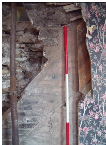
Plate 29. West wall of principal bedroom F6A showing revealed quoins of pre 18 th century hall east wall (shown on insert of Buck drawing of 1720, and later inserted flue for ground floor room G6a)
