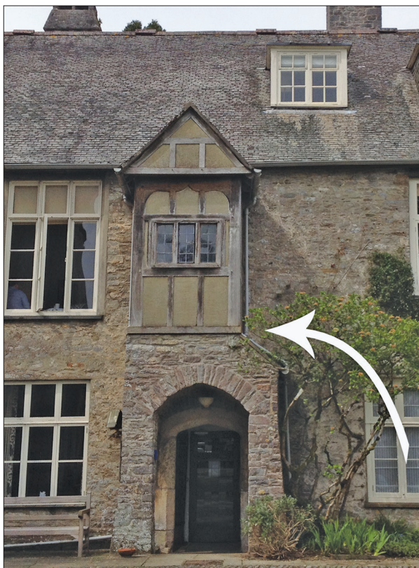
Figure 4a The image shows the direction of the staircase, now removed, which gave access to the first-floor room. This is different to the other staircases on the range, and this would have been distinctive to the medieval audience.
