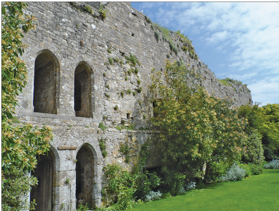
Figure 2 Paired garderobe doors at Amberley Castle, contribute to the uniform elevation. Paired features are a main characteristic of lodging ranges, present in nearly all examples.
