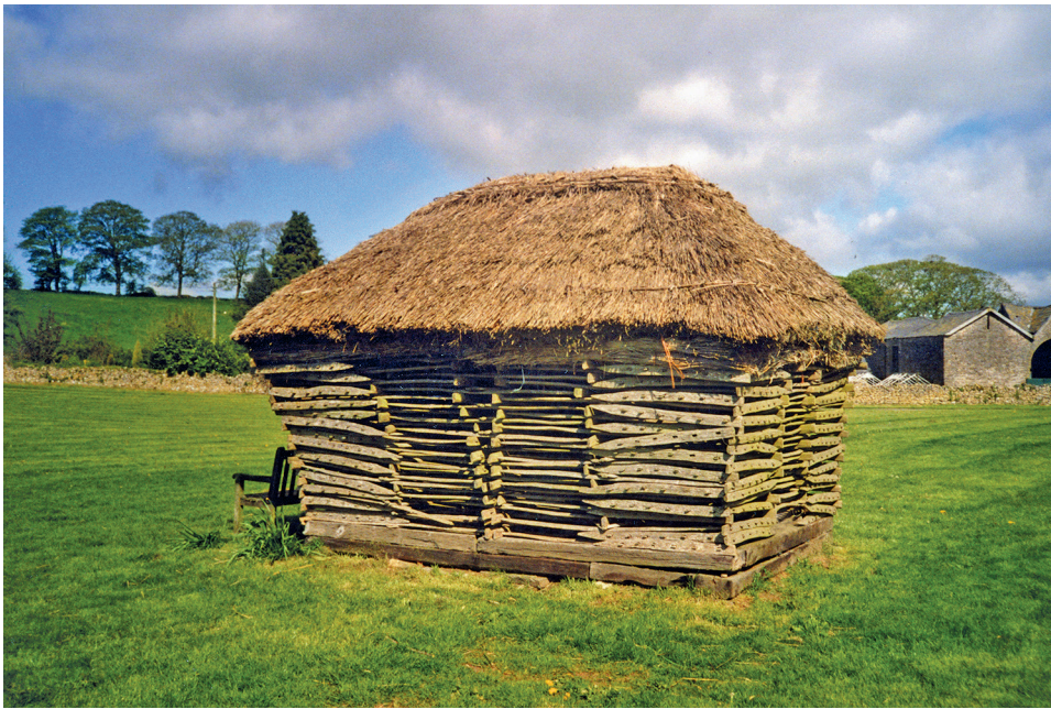
Figure 7 The Priddy hurdle stack; note the arrangement of beams supporting the base of the stack. Photographer Graham E. Cook.
