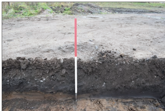
Plate 1: Overburden deposits in Trench 1A.
