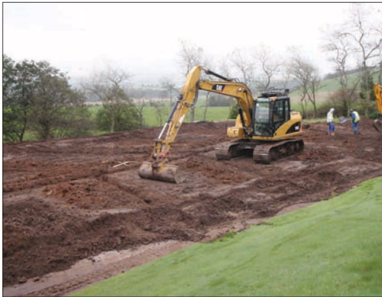
Plate 1: 13th Green from south, after drainage features were excavated
