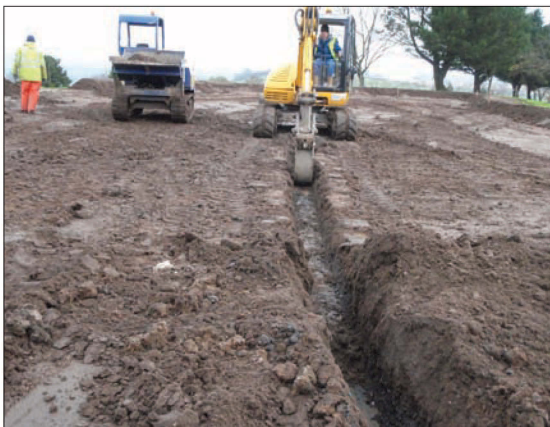
Plate 3: Working shot, excavation of central drainage channel, 15th green from east
