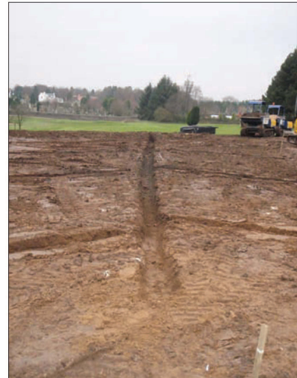
Plate 2: 15th Green from west after drainage features were excavated
