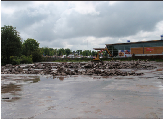
Plate 1: Concrete removal using machine with breaker.
