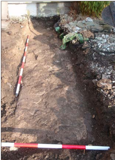
Plate 1: Foundation wall of previous house demolished in the 1960's.
