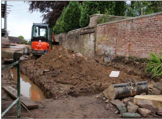
Plate 3: Garage trench location.
