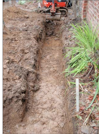
Plate 4: Excavation of garage foundation trench at garden boundary wall.
