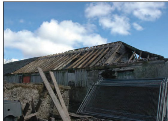
Plate 14: Roof timbers visible at south of Building 3.
