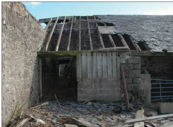
Plate 13: Roof timbers visible at north of Building 3.
