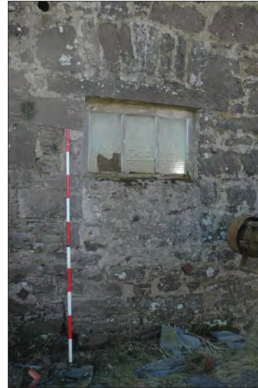
Plate 8: Partially blocked window on Building 2, north elevation.
