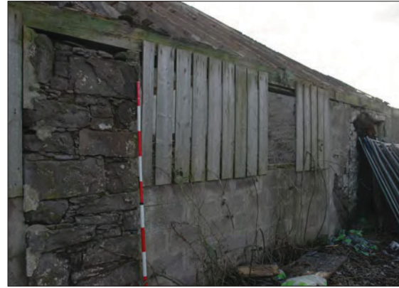
Plate 12: Breeze-block and timber slat wall.
