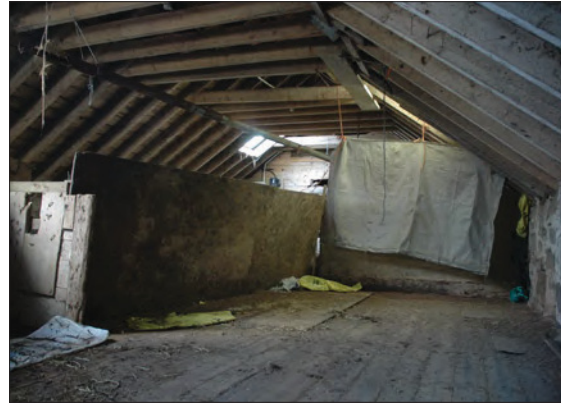
Plate 16: Upper storage space in Building 1.
