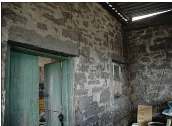
Plate 19: Door and window on original exterior wall of Building 1.
