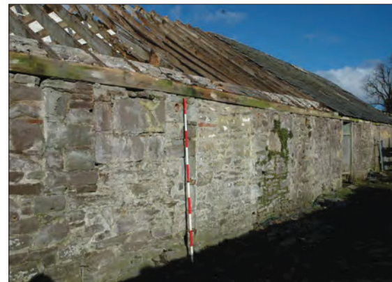
Plate 10: Block-up doors and window on Building 3.
