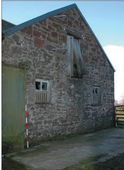
Plate 7: Arrangement of windows on Building 2, north gable end.
