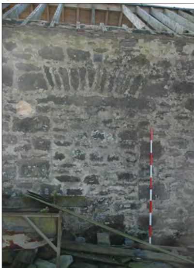
Plate 5: Blocked entrance with splayed stone headwork. Building 2, north elevation.
