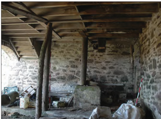
Plate 17: Wooden support posts in Building 1.
