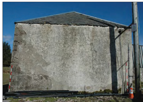
Plate 2: Harling and exposed stones on south facing elevation of Building 1.
