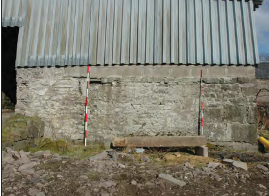
Plate 3: Blocked-up window in lean-to component of Building 1.
