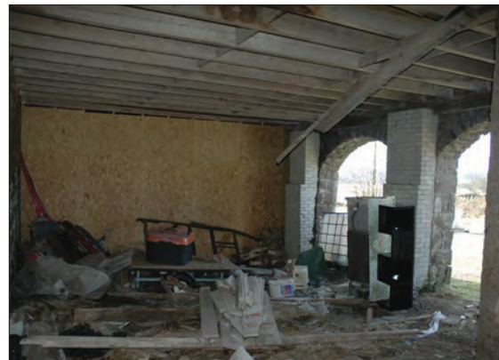
Plate 18: Breeze-block support columns in Building 1.
