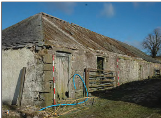
Plate 9: View of east side of Building 3.
