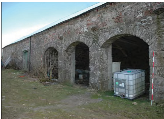
Plate 1: West facing elevation of Building 1.
