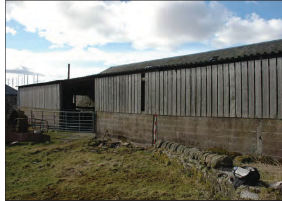
Plate 4: East facing elevation of Building 1.
