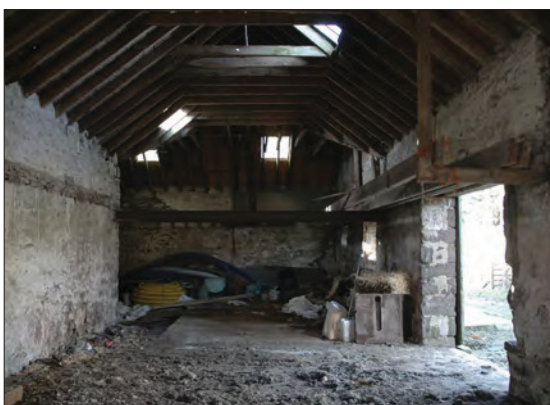
Plate 21: East end of Building 2.
