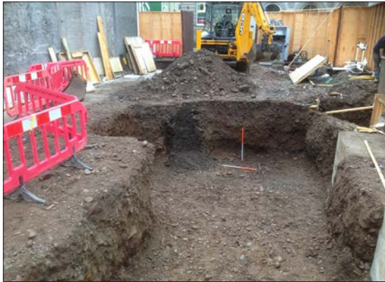
Plate 1: Surviving part of well on the south-eastern edge of foundation trench.
