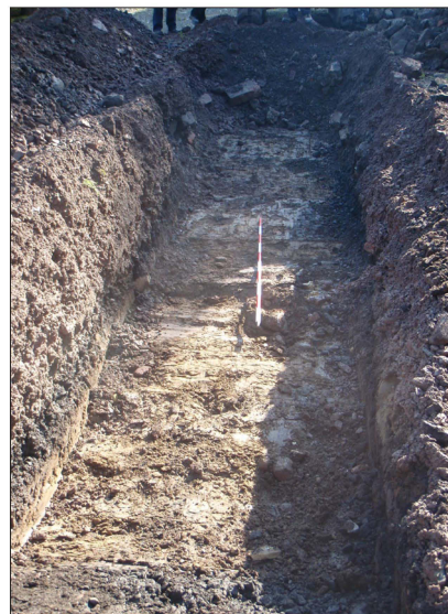
Plate 3: Post-excavation of trench.
