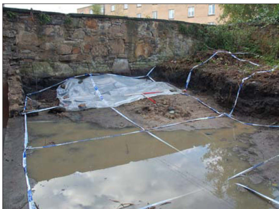
Plate 1: Pre-excavation of site.
