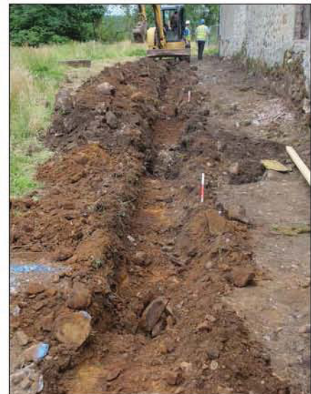
Plate 2: Linear foundation trench to east of steading.
