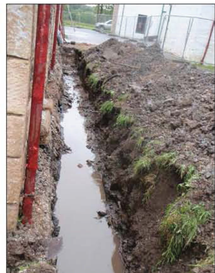
Plate 4: Drainage trench to west of steading.
