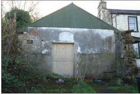
Plate 4: Eastern outbuilding north elevation.
