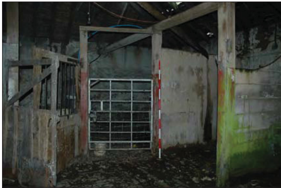
Plate 11: Room 1 interior stalls.
