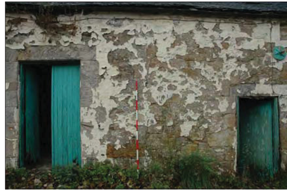
Plate 9: Visible join in stonework at extended section.
