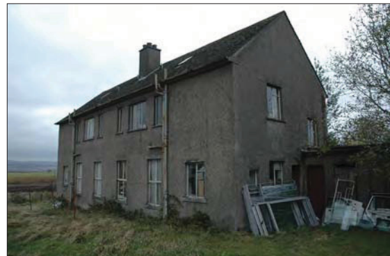
Plate 18: Auchinleck cottages south and west elevations.
