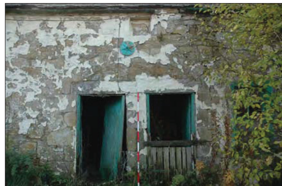
Plate 10: Blocked cart arch in Stables east elevation.
