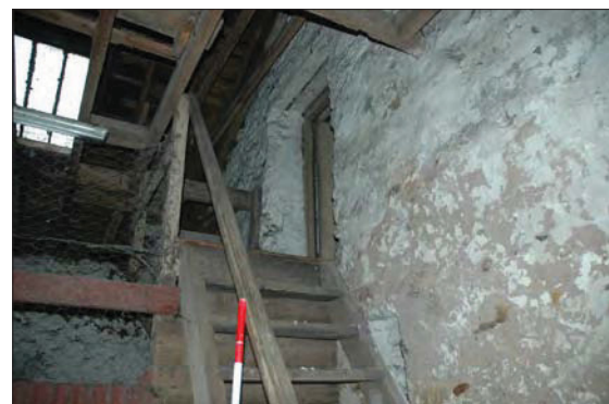
Plate 14: Room 2 staircase to upper level.
