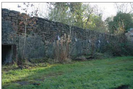
Plate 6: West elevation of extension wall remains.
