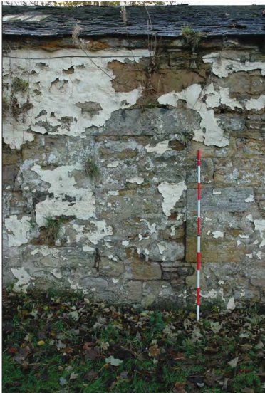
Plate 8: Blocked entrance in Stables east elevation.
