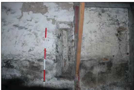
Plate 13: Detail of blocked window slit.
