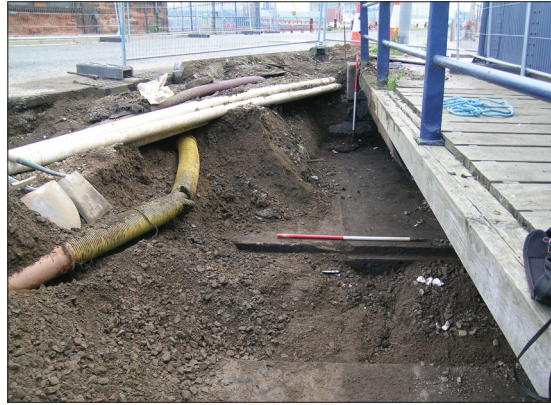
Plate 5: Old pier stanchion at Victoria Swing Bridge
