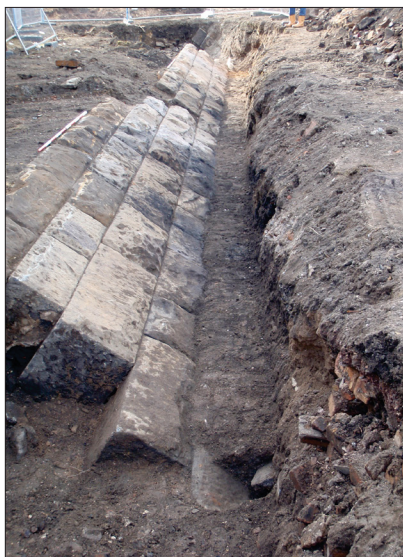
Plate 1: View of Old Sea Wall from the east
