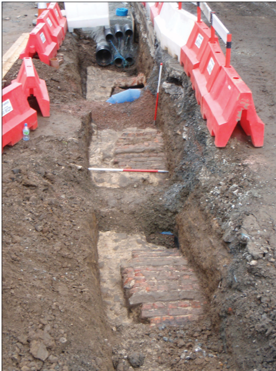
Plate 20: Pre-excavation view of three chambers
