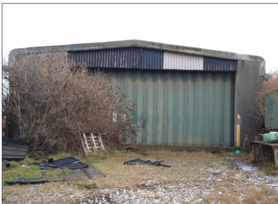
Plate 8: West exterior of depot building
