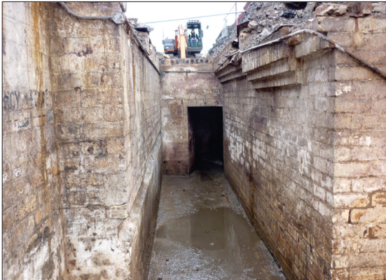
Plate 35: Main shelter after removal of debris and water
