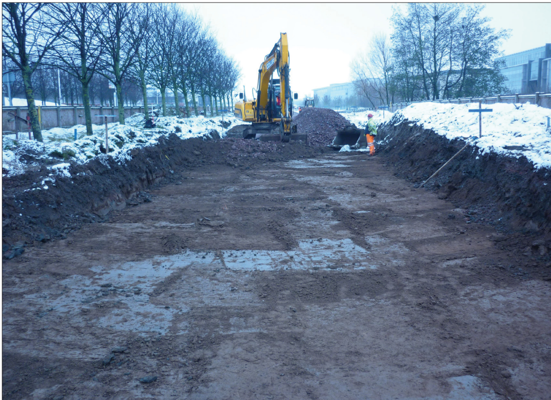
Plate 39: Excavating in the snow
