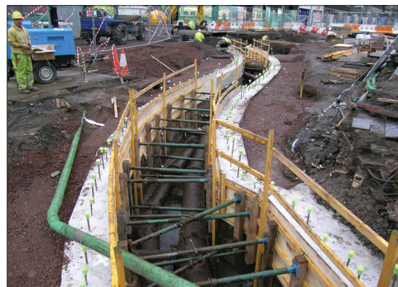
Plate 14 : Crawley Tunnel with roof removed and water pipes exposed
