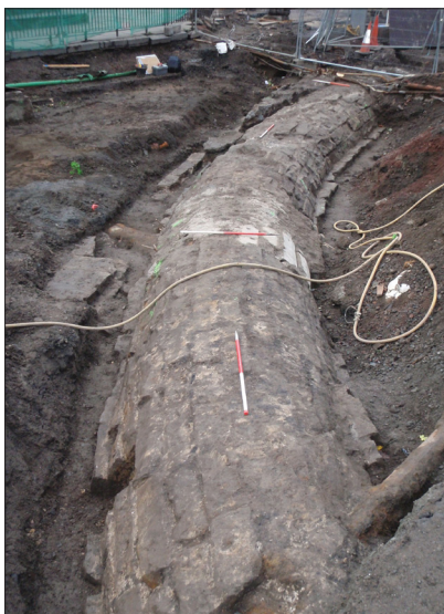
Plate 13: Crawley Tunnel exposed with arched roof
