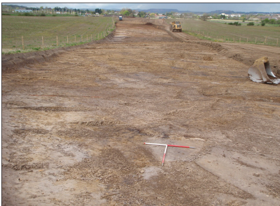
Plate 40: General view of construction corridor
