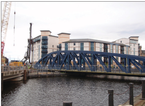
Plate 3: General view of Victoria Swing Bridge
