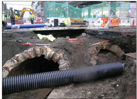
Plate 19: Both Tunnels converging at foot of Hannover St
