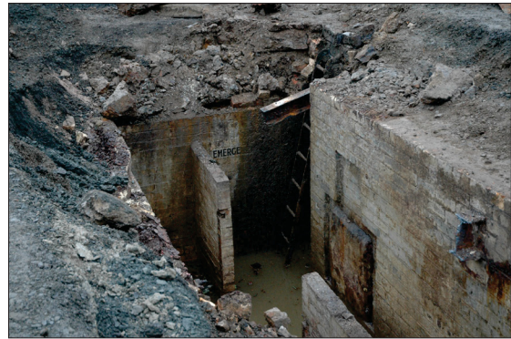
Plate 34: Emergency Exit at west end of shelter
