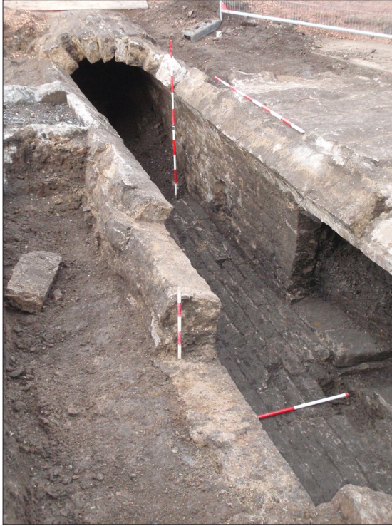
Plate 16: View of Second tunnel
