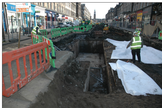
Plate 32: East end of shelter on West Maitland Street
