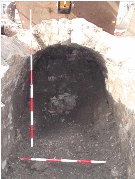
Plate 18: Crawley Tunnel structure
