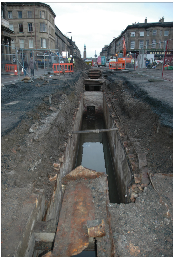
Plate 30: West end of shelter at Haymarket Terrace
