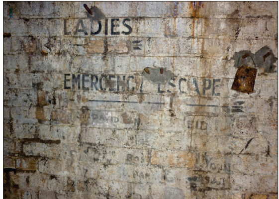
Plate 36: Signage on shelter wall
