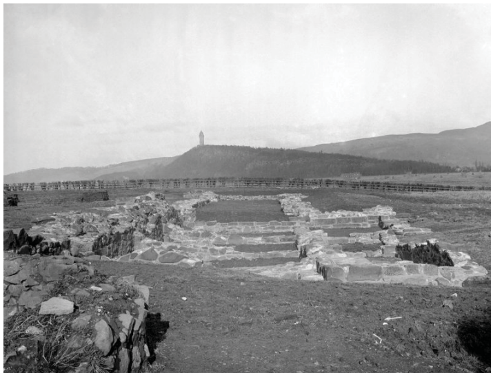
Fig. 4 Photo from 1931 (Canmore) Building A from south, presumably following consolidation
