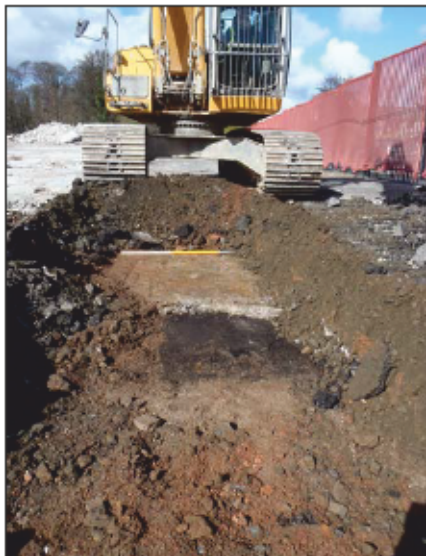
Plate 7: Roughcast concrete floor [012] overlying a mortar screed [013] in Trench 10.
