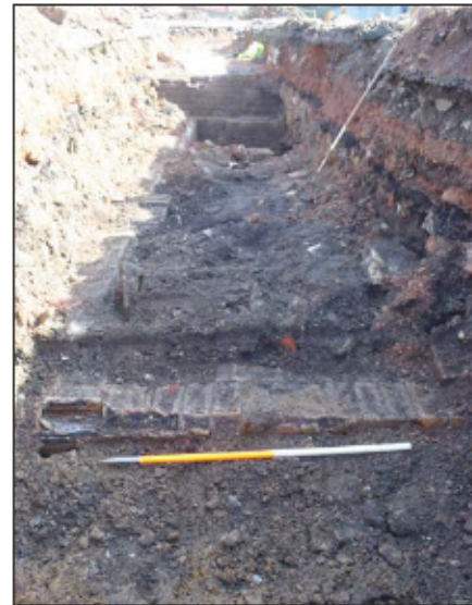
Plate 10: Brick wall [017] forming the north west limit of the brick structure, from the north west.
