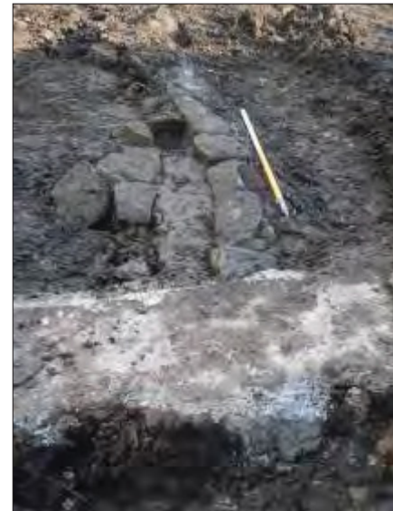
Plate 17: Culvert 1017 from the west.
