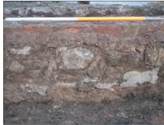
Plate 19: Sandstone wall 1010 with a course of unfrogged brick on top of its upper course, probably a later build, west facing elevation.
