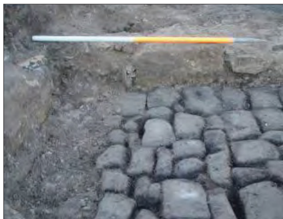
Plate 20: Wall 1006, left of frame cutting cobbled surface 1011 and wall 1008, top right of frame, from the east.
