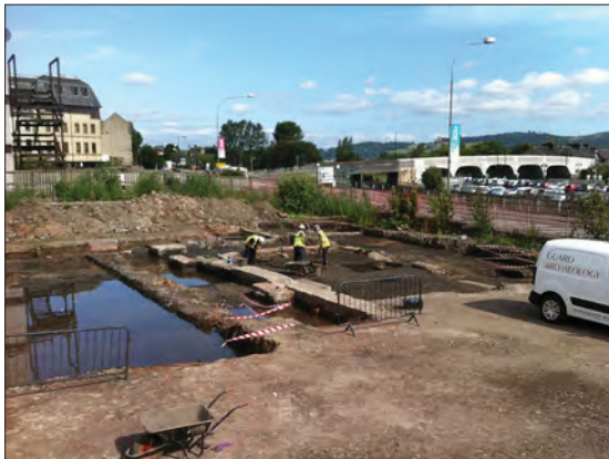
Plate 1: Working shot of preliminary clean up of site prior to excavation.
