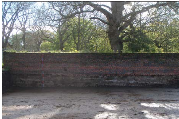
Plate 4 : Shot of wall of slurry pit [003] [004].
