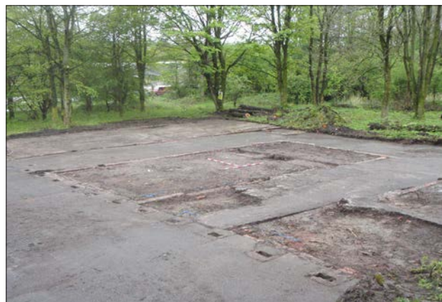
Plate 1: Shot of Woodland House area stripped.
