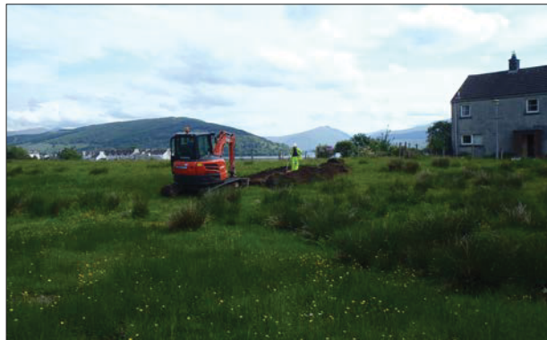
Plate 3: General view of trenching.
