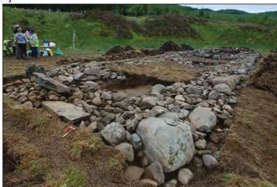
Plate 1: East Gable wall 014 with lintel stone left of centre.
