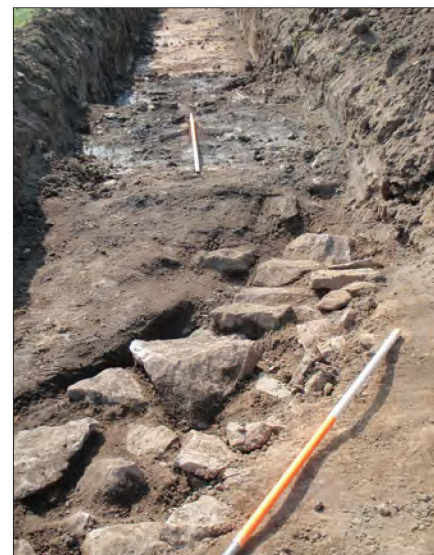
Plate 1: The disturbed basal courses of wall 300 in Trench 22 with associated demolition spread 301 lying along the south side of the wall within a trench cut [302] to receive the demolished wall, view from the east-north-east
