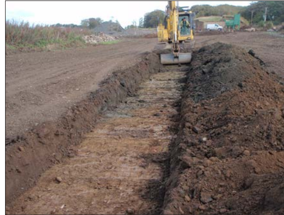
Plate 2: General view of foundation trench for agricultural building, from west.
