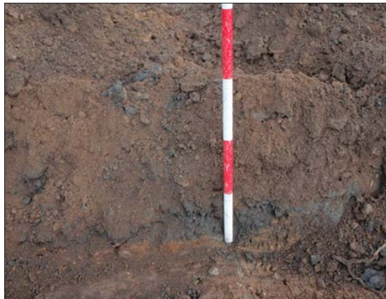
Plate 3: East facing section of strip foundation for agricultural shed. The thin black layer represents the undisturbed topsoil.
