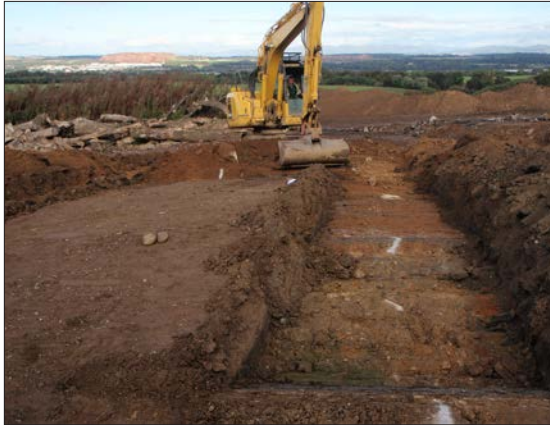
Plate 1: General view of trench foundation for house/lodge, from north-west.
