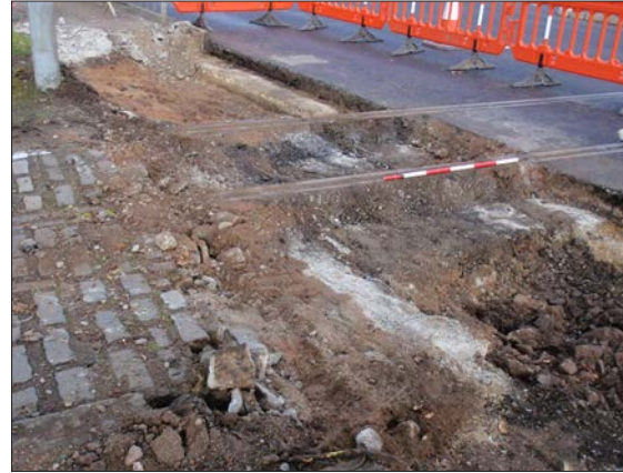
Plate 2: Old tramlines preserved in situ during the ground works.
