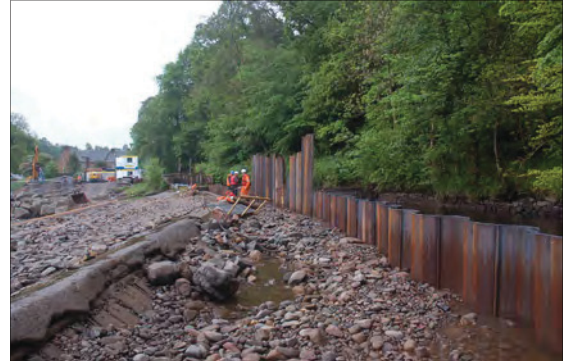
Plate 4: Cofferdam in situ and river bed material pre-excavation.
