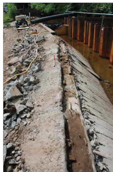
Plate 14: Partially exposed lintel beam 006/018.
