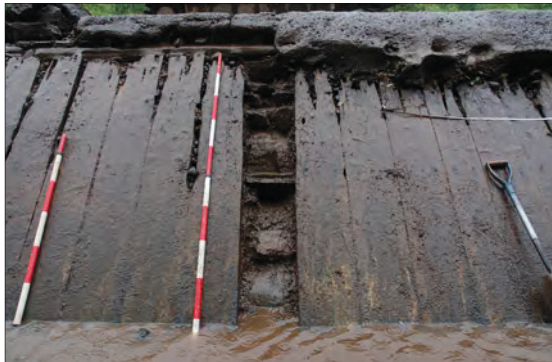
Plate 11: Packing material and structure beneath removed weir face plank 004.
