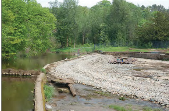
Plate 3: Construction access track across weir spillway.
