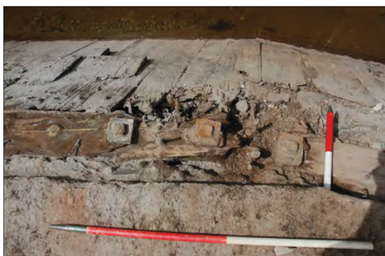
Plate 15: Bolts securing lintel beam at its change in direction near to lade.
