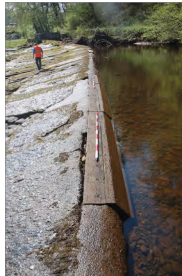
Plate 12: Crest repairs.
