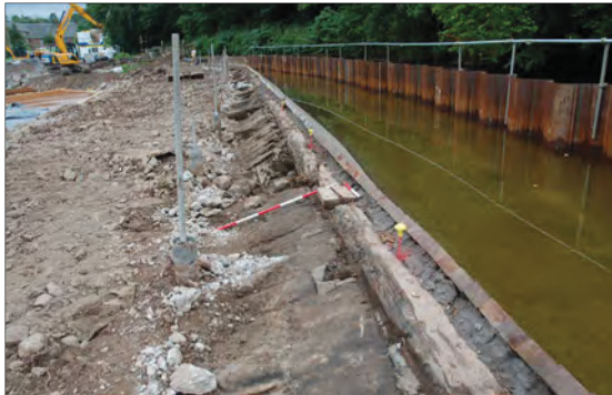
Plate 18: Dressed sandstone blocks in crib to immediate east of penstock
