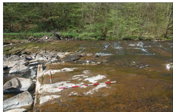
Plate 2: Shot of weir crest and cribs.
